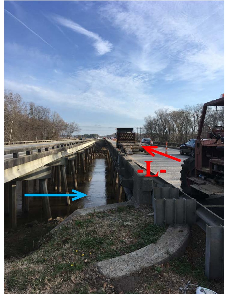
Looking Northeast towards End Bent 2
