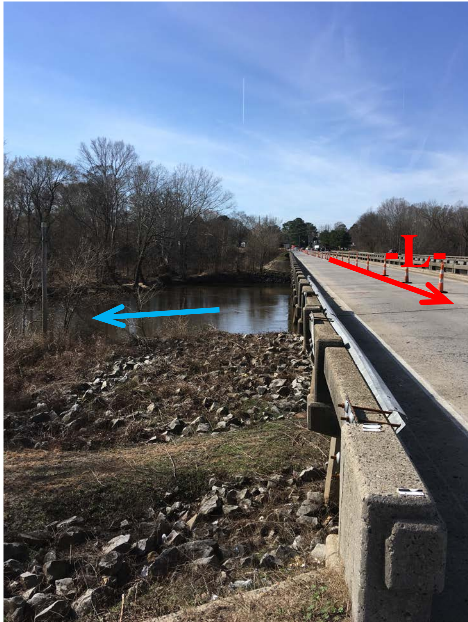
Looking Southwest towards End Bent 1
