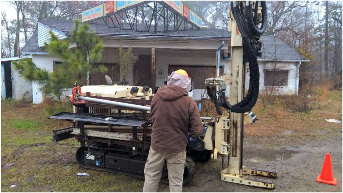
View of drilling activities.
