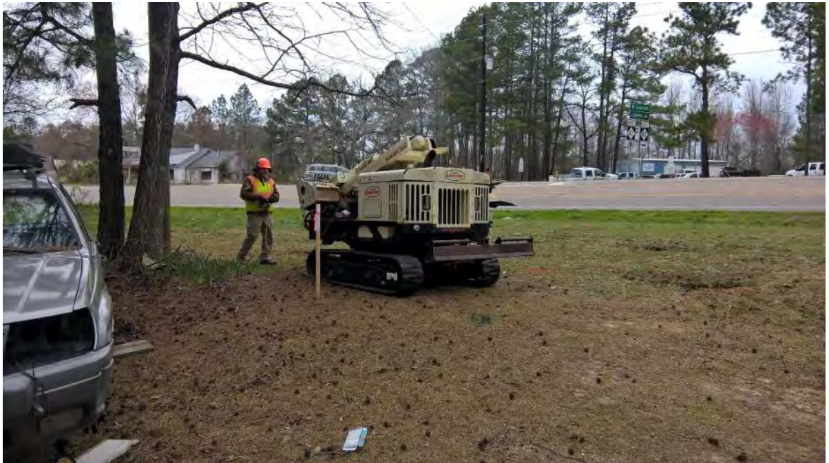
View of drilling on Parcel 117.
