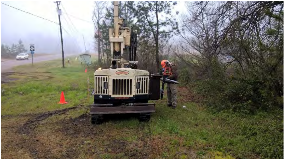
View of drilling activities.
