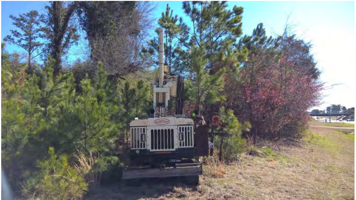
View of drilling on Parcel 77/78/79.
