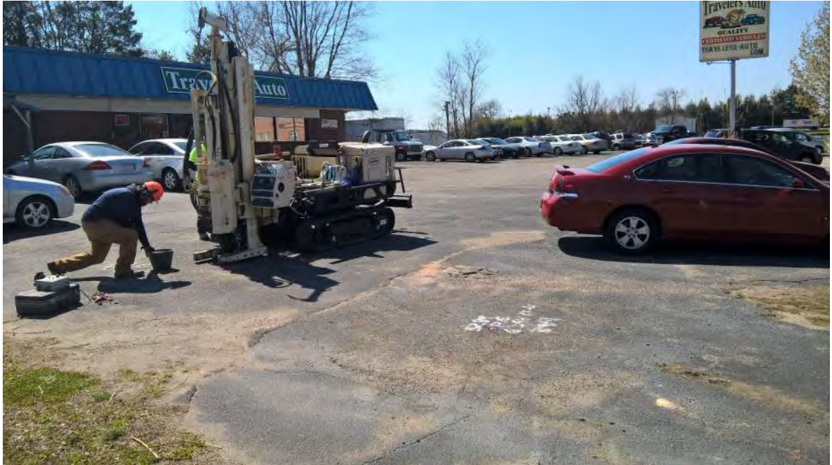
View of former UST Basin.
