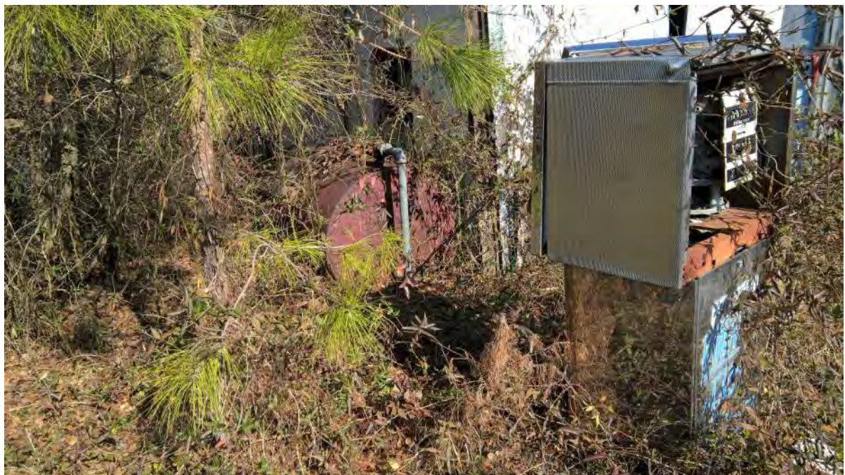
View of kerosene AST and dispenser.
