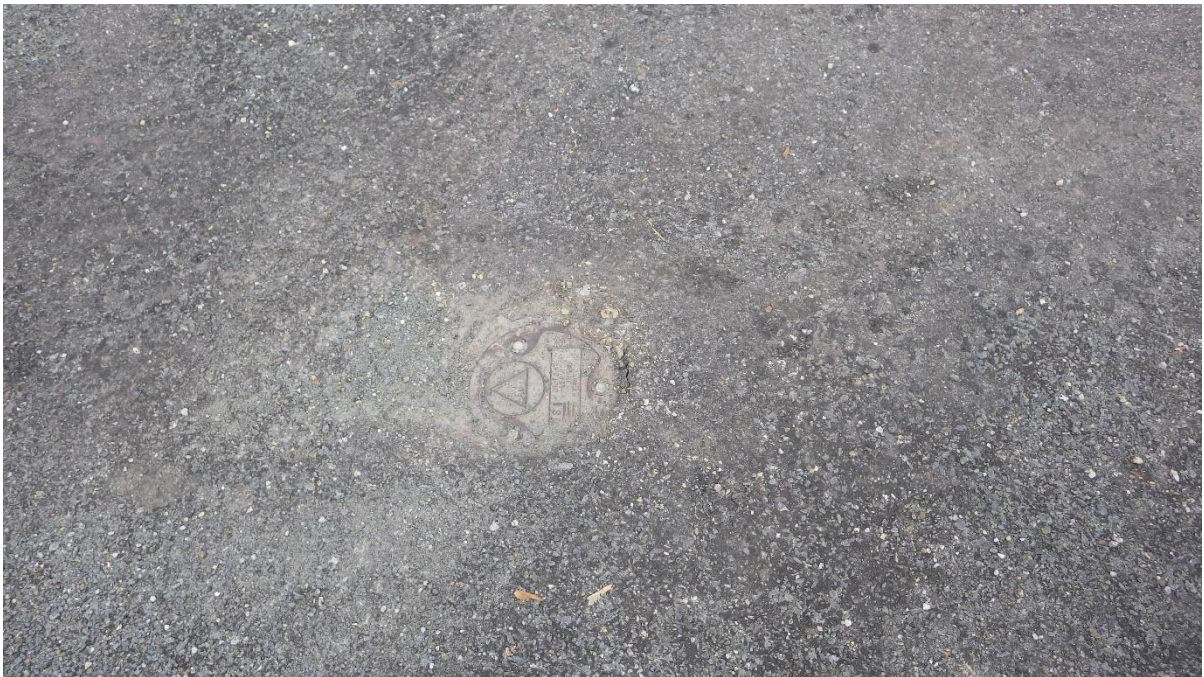
Monitoring well in the former USTs area
