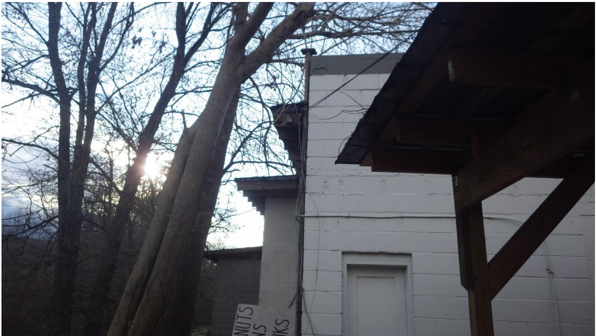
Two vent pipes on the wall.
