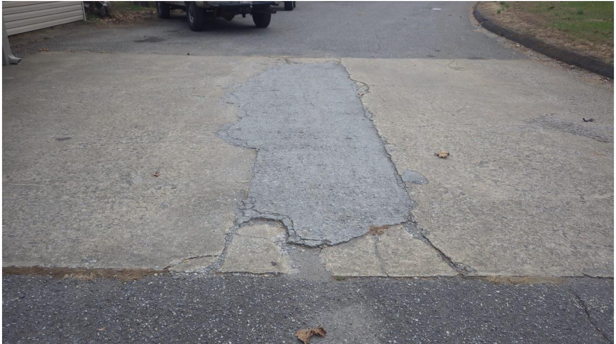
Former Pump island
