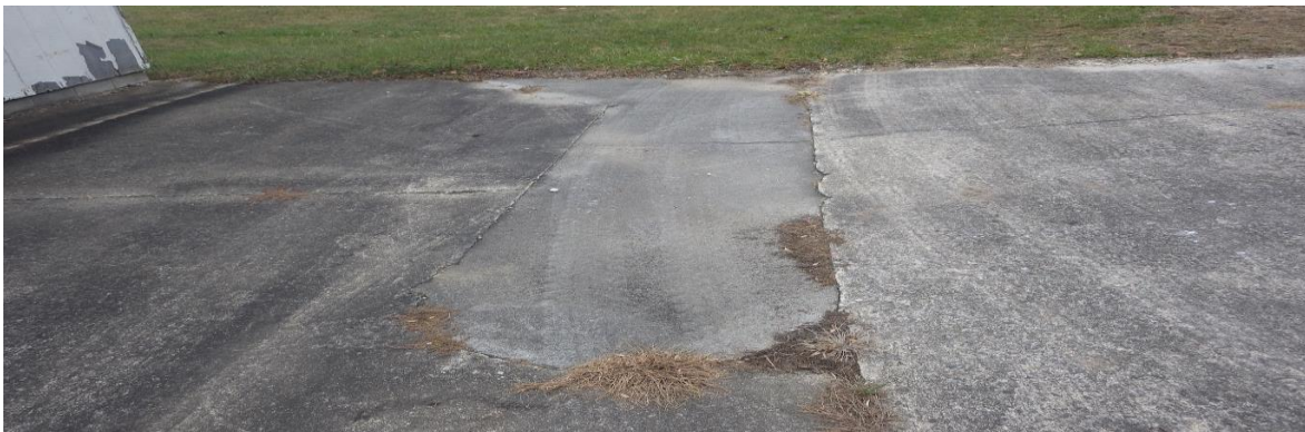
Pump island removed
