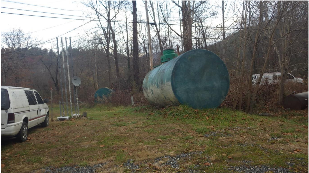
USTs removed from the ground and store on site.
