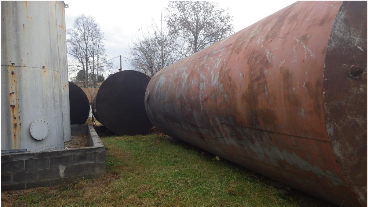
Some USTs removed and store on site.
