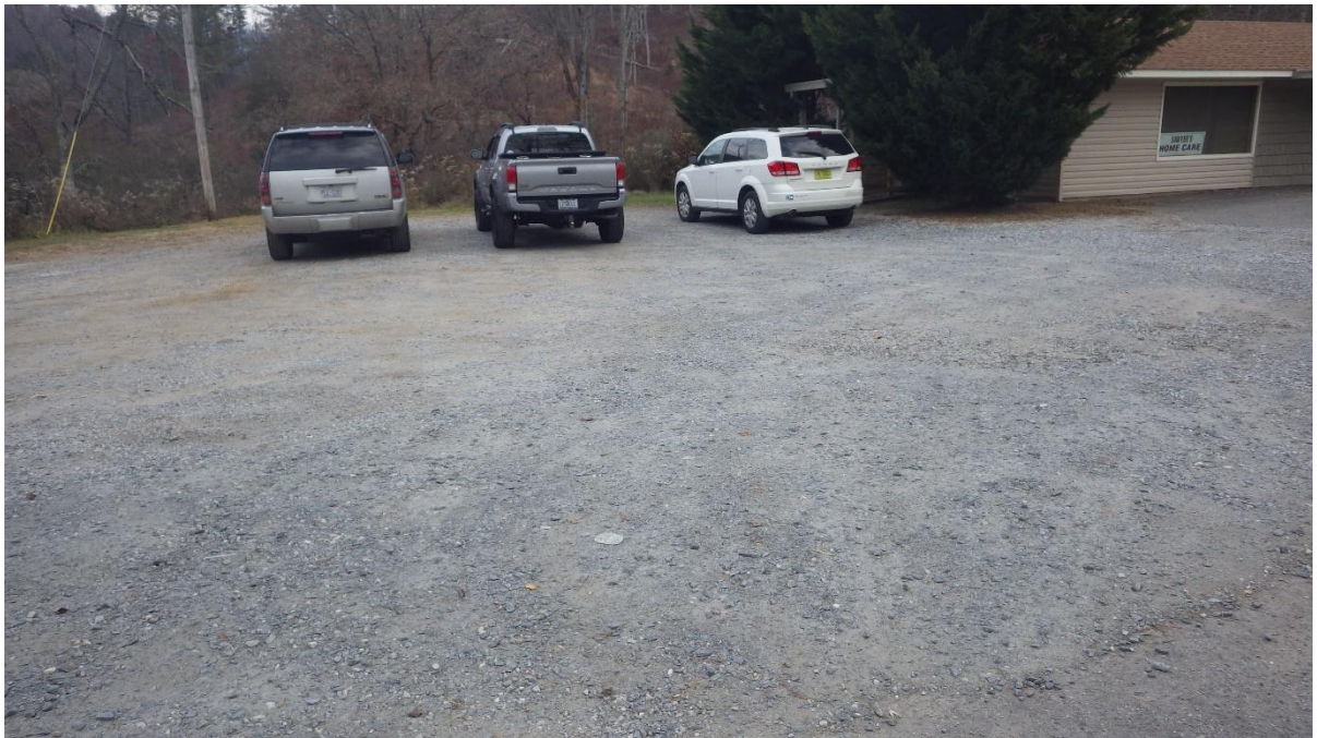
Possible former USTs area
