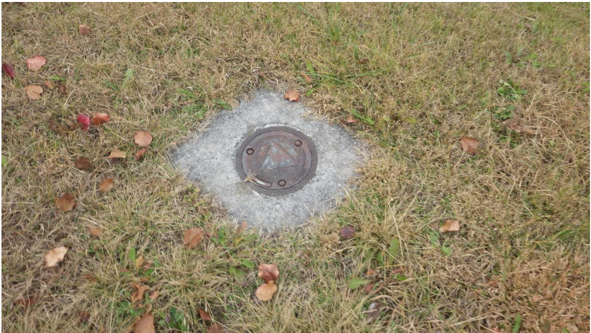
Older Monitoring well
