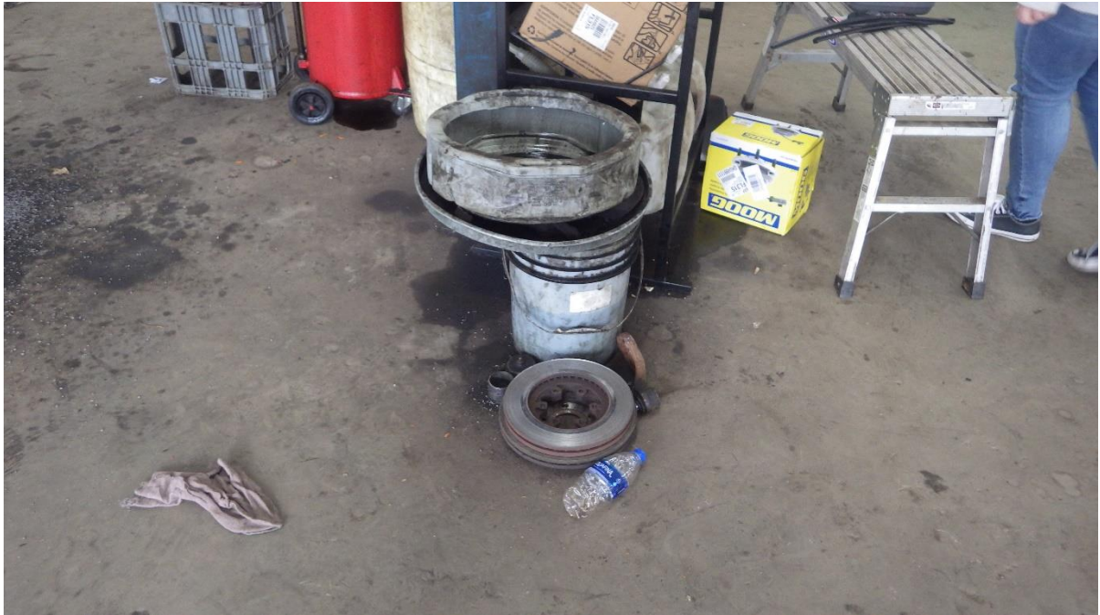
UST fill port inside the building according to an employee on site.
