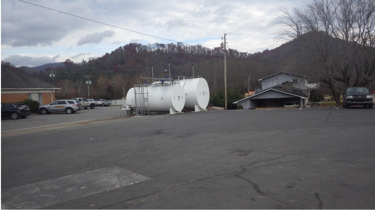
ASTs with concrete internal lining.
