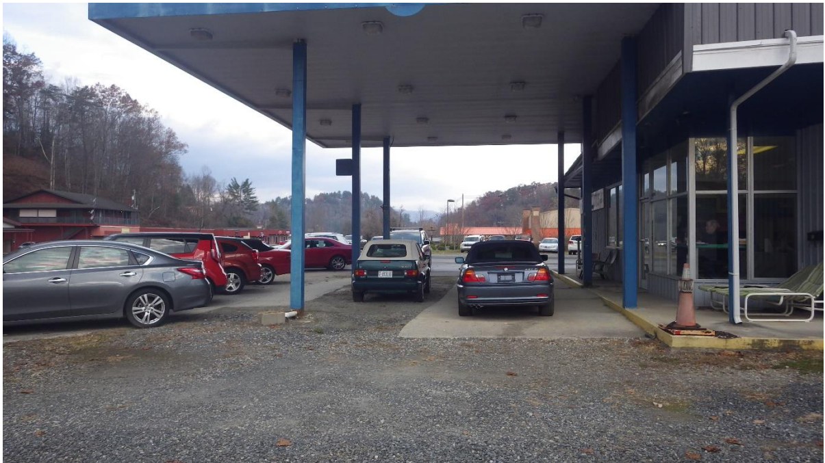
Land disturbance for USTs removal
