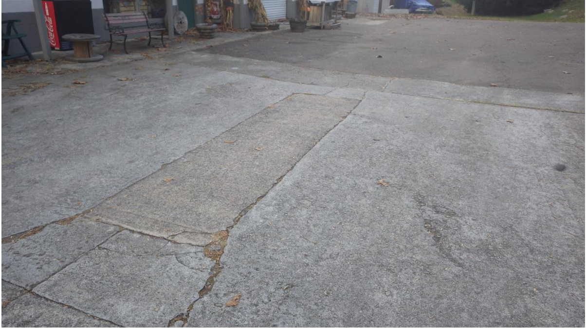
Former dispenser area
