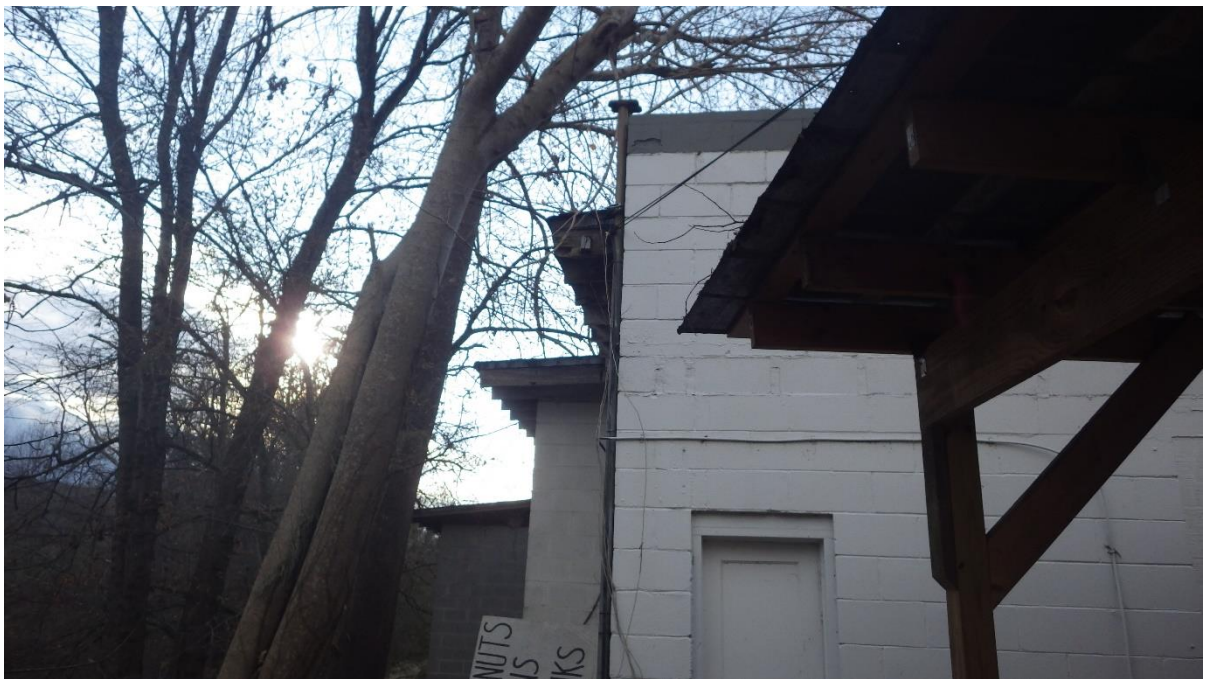
Two vent pipes on the wall.
