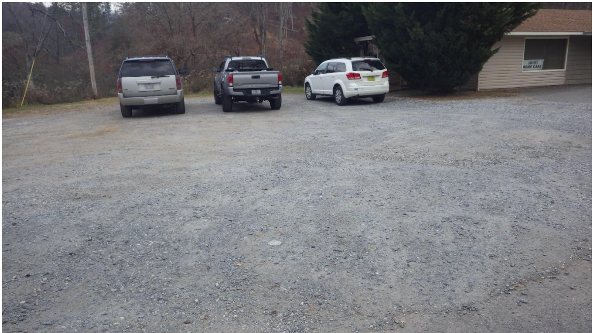
Possible former USTs area
