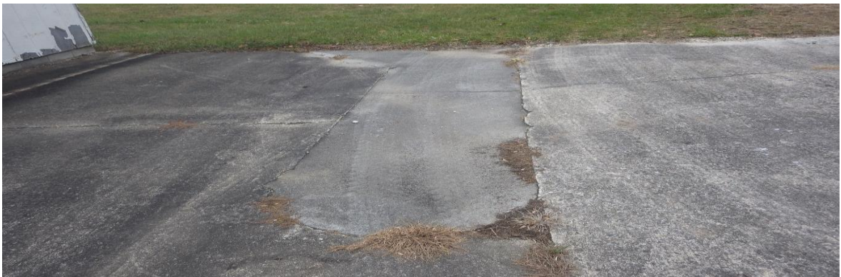
Pump island removed
