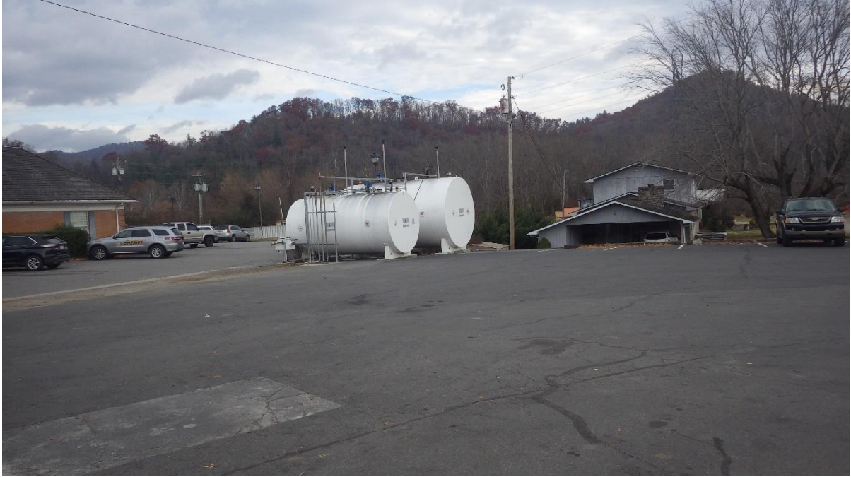
ASTs with concrete internal lining.
