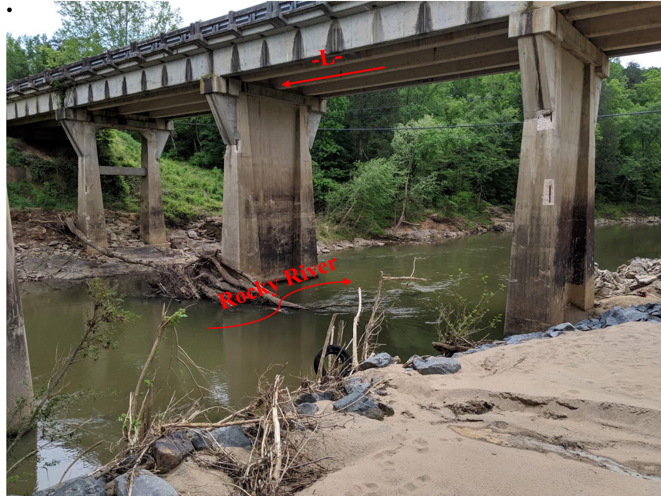
View Looking Downstream
