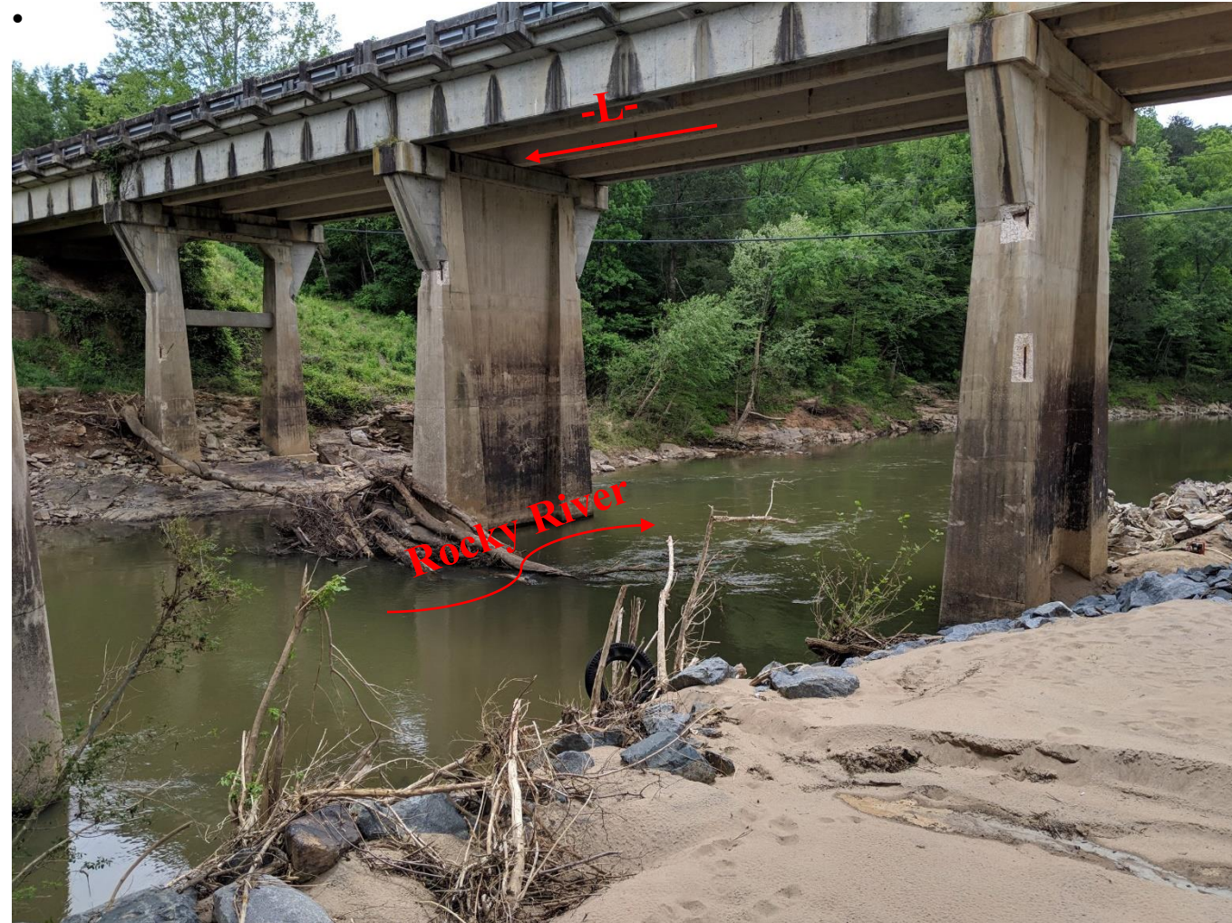
View Looking Downstream
