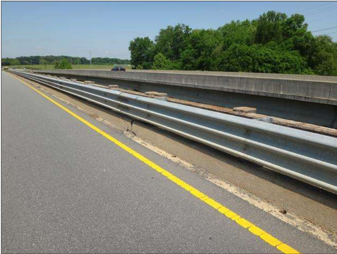
NORTH BARRIER RAIL
