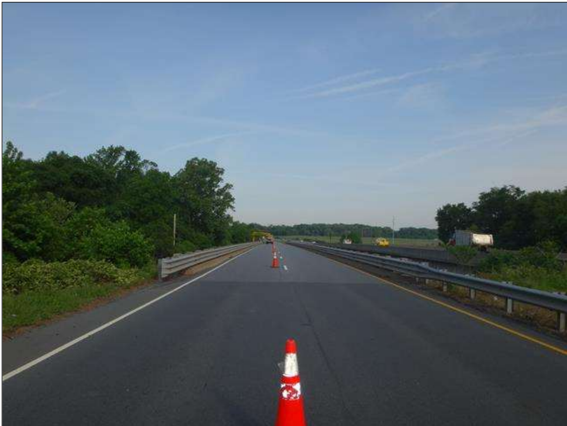
EAST APPROACH LOOKING WEST
