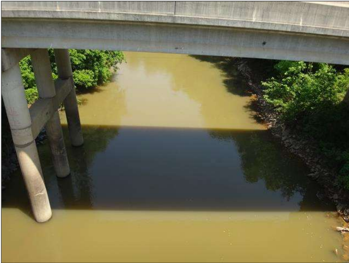
LOOKING UPSTREAM, NORTH
