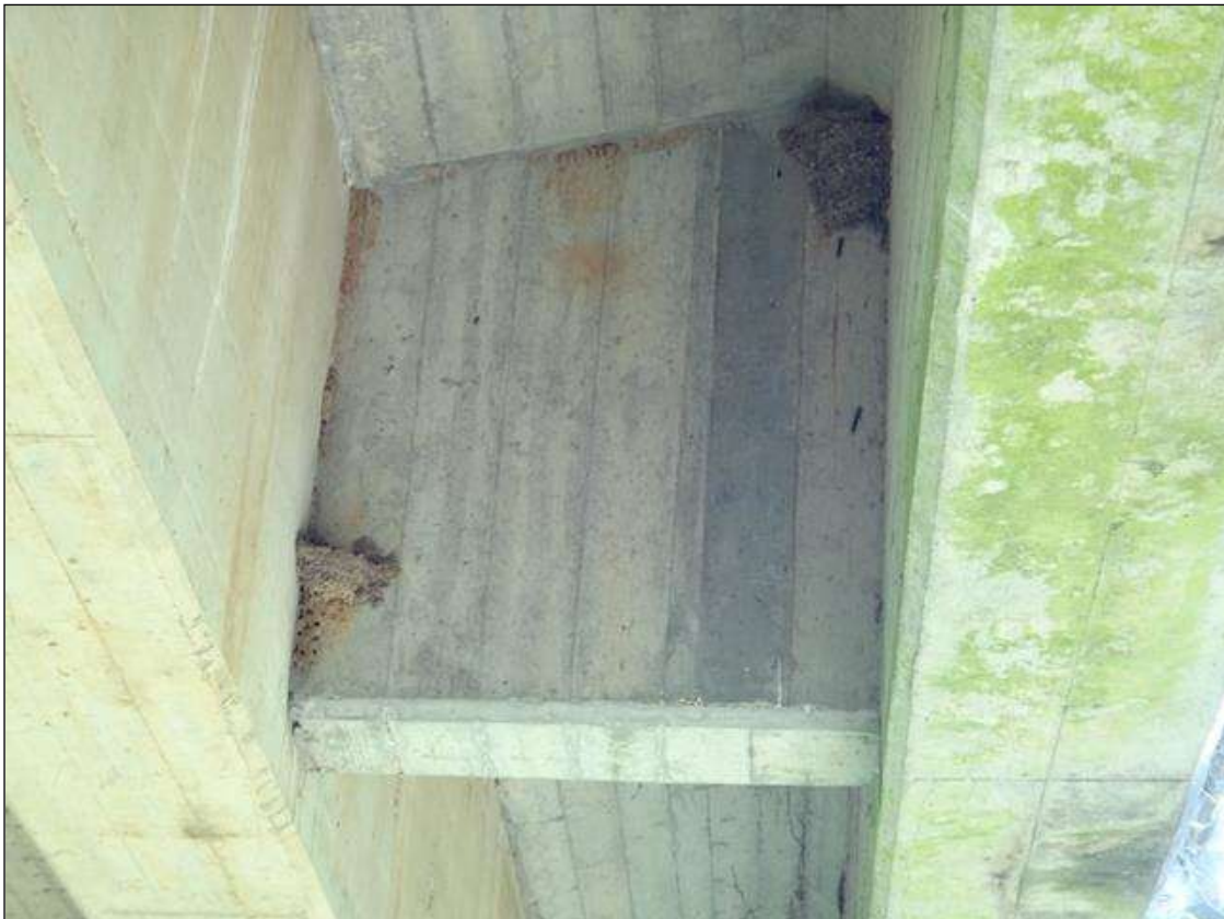
UNDERSIDE OF DECK BAY 1 INTERIOR DIAPHRAGM (SIMILAR AT BAY 5)
