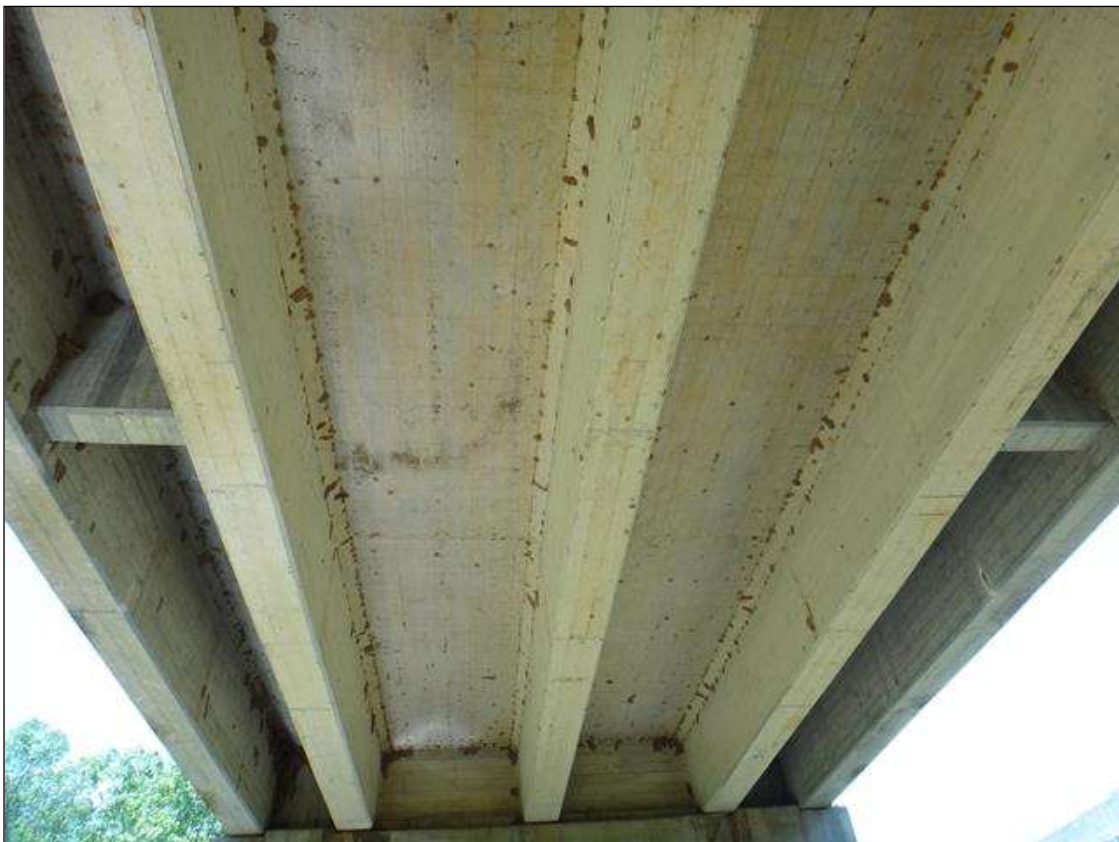
UNDERSIDE OF DECK
