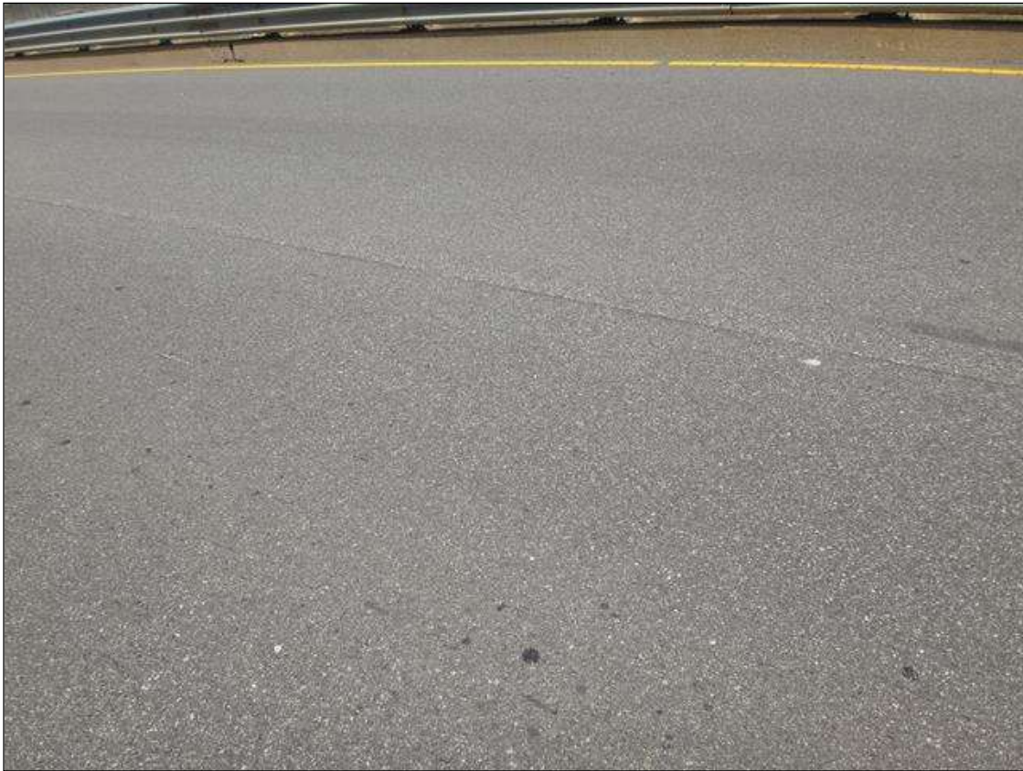
ASPHALT WEARING SURFACE AT SPAN 10
