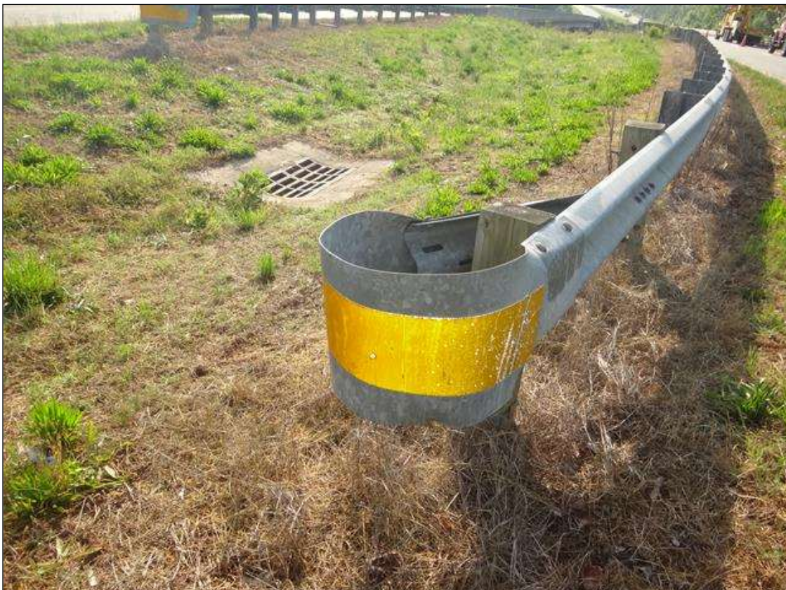
NORTHWEST GUARDRAIL TERMINATION
