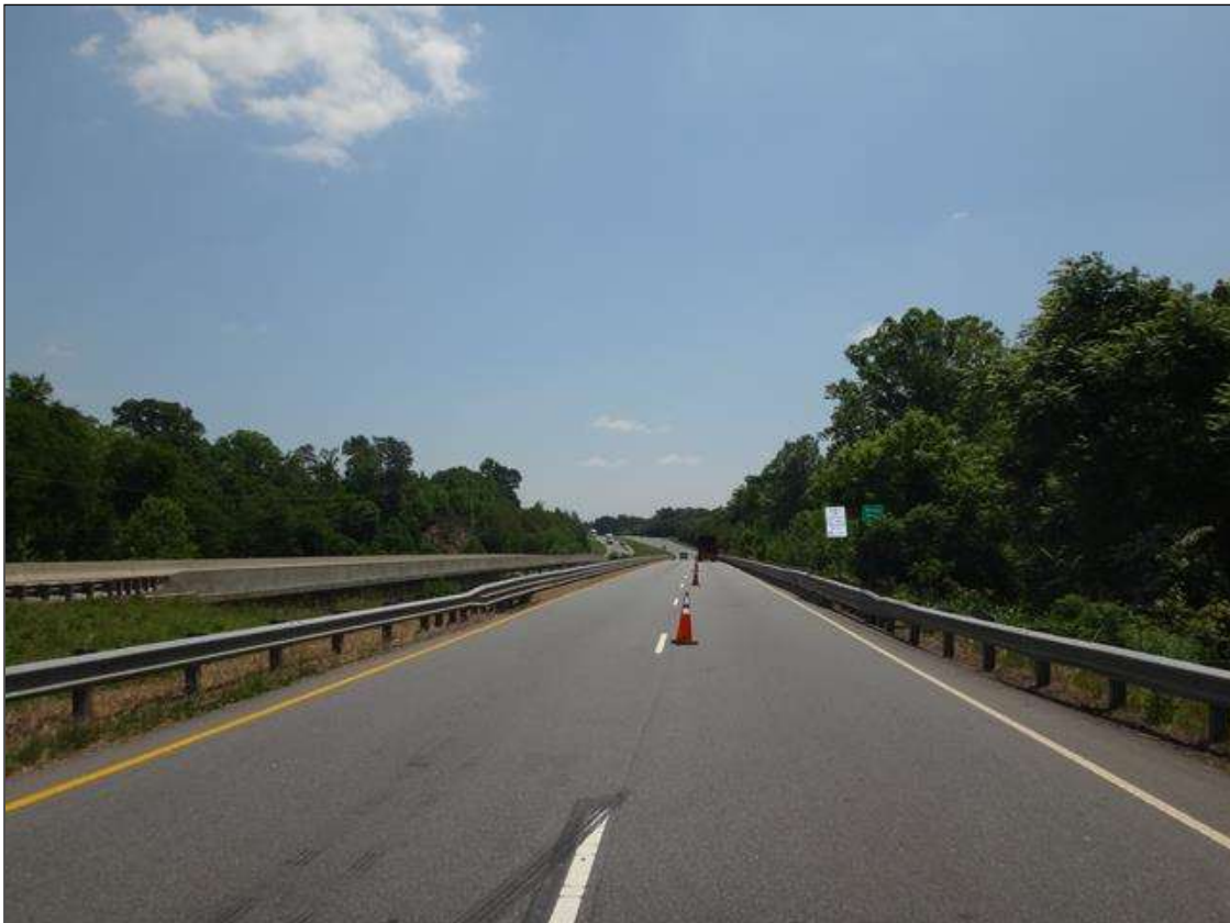
WEST APPROACH LOOKING EAST
