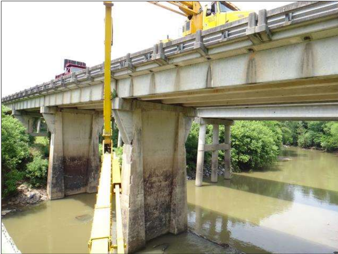
DOWNSTREAM PROFILE, LOOKING NORTH
