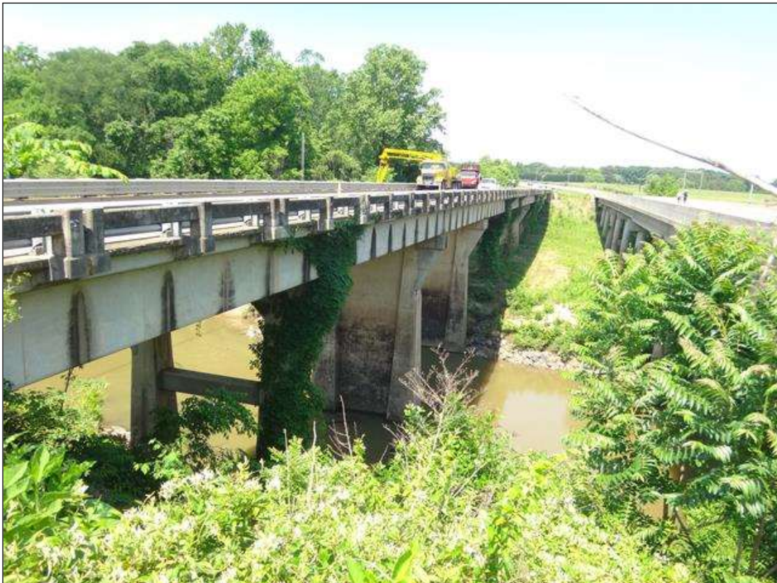
UPSTREAM PROFILE, LOOKING SOUTH
