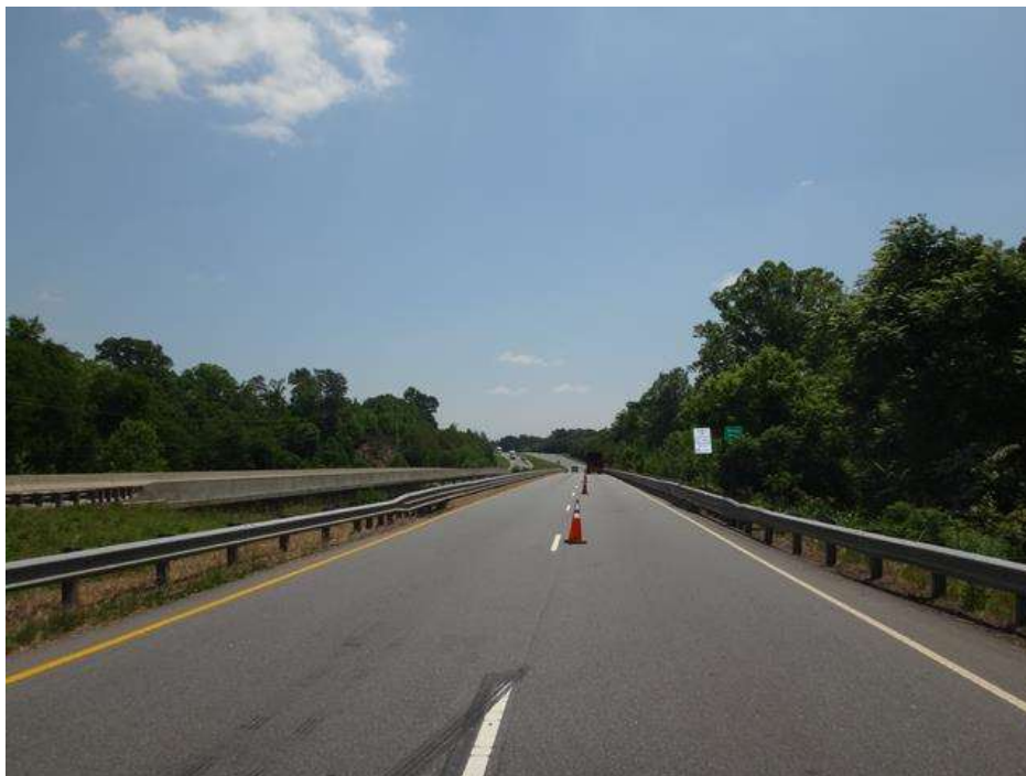
WEST APPROACH LOOKING EAST
