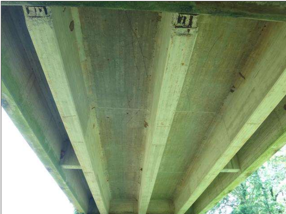
UNDERSIDE OF DECK AT SPAN 2
