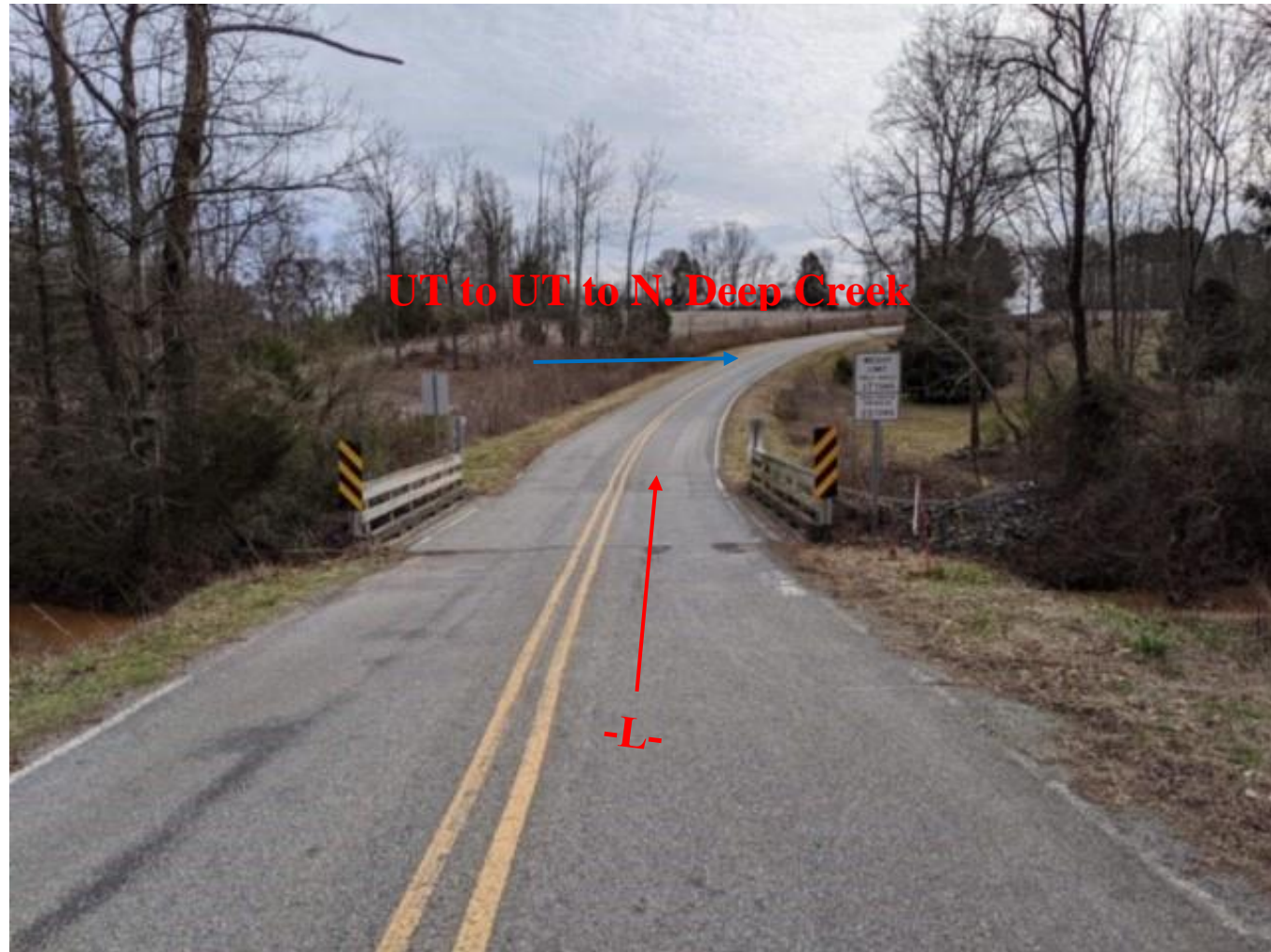
Photograph No. 1: Looking from End Bent 1 towards End Bent 2
