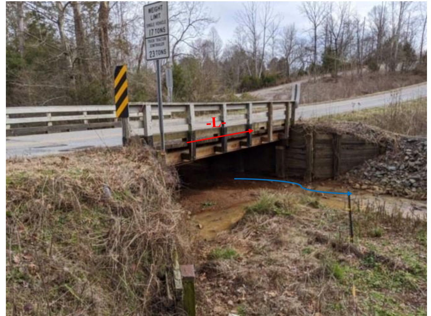
Photograph No. 2: Looking Upstream
