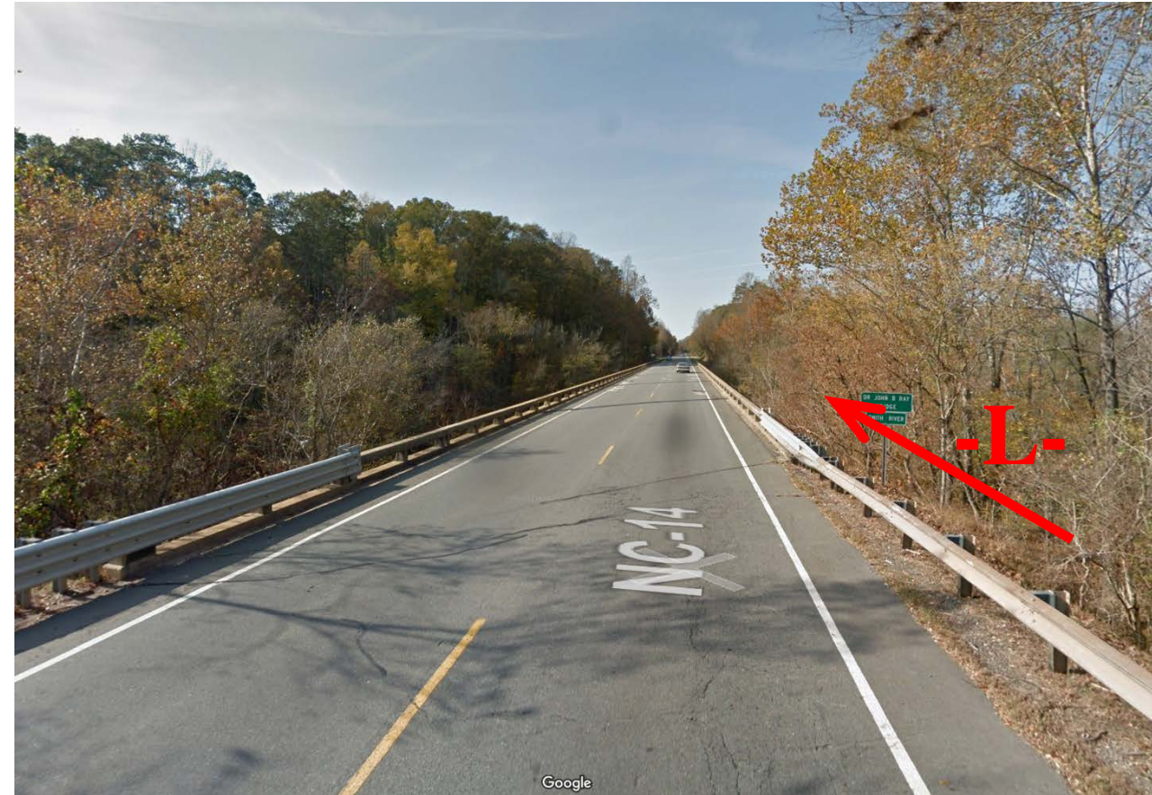
View near existing end bent 2, facing downstation (west)
