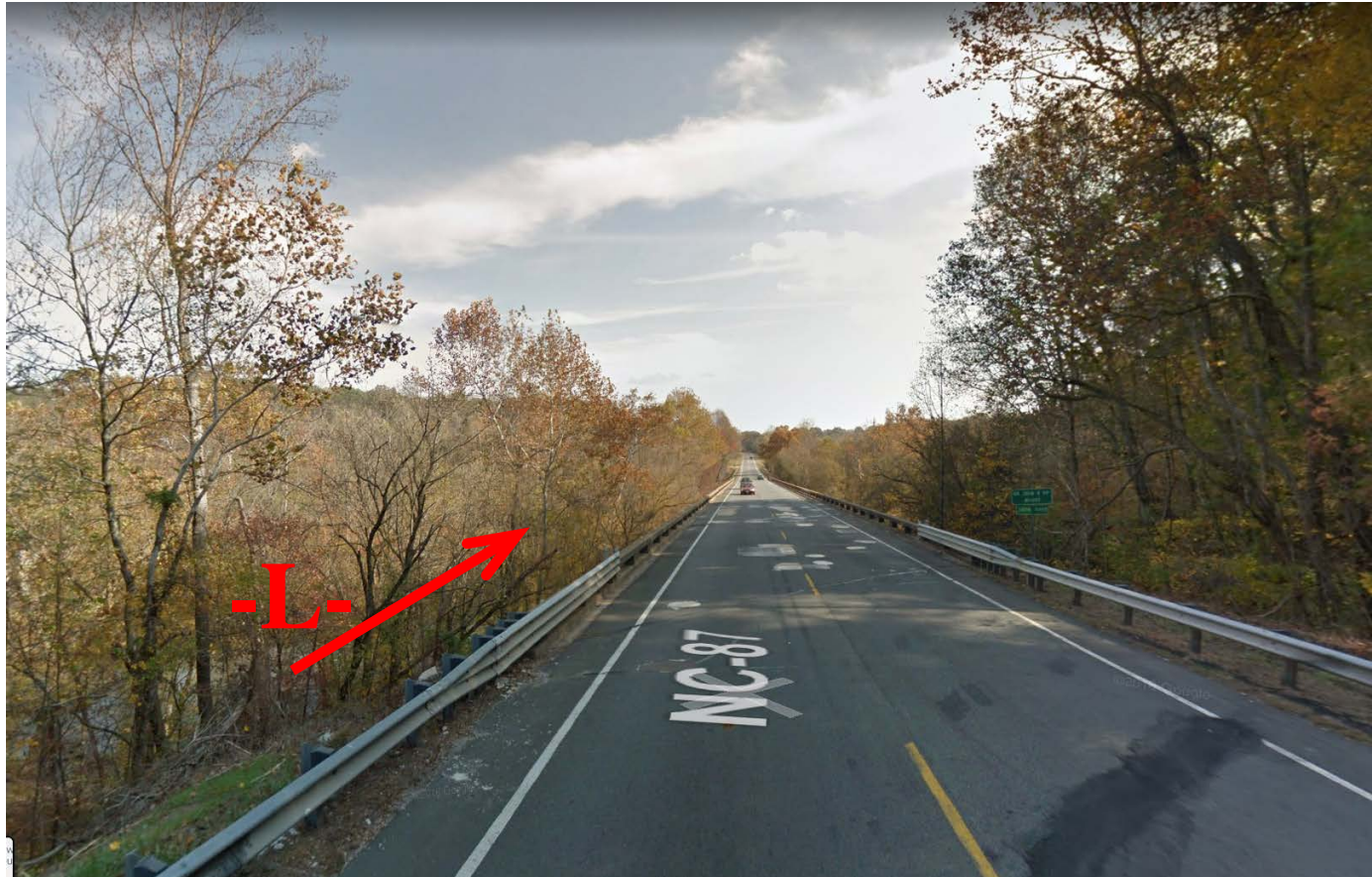
View near existing end bent 1, facing upstation (east)
