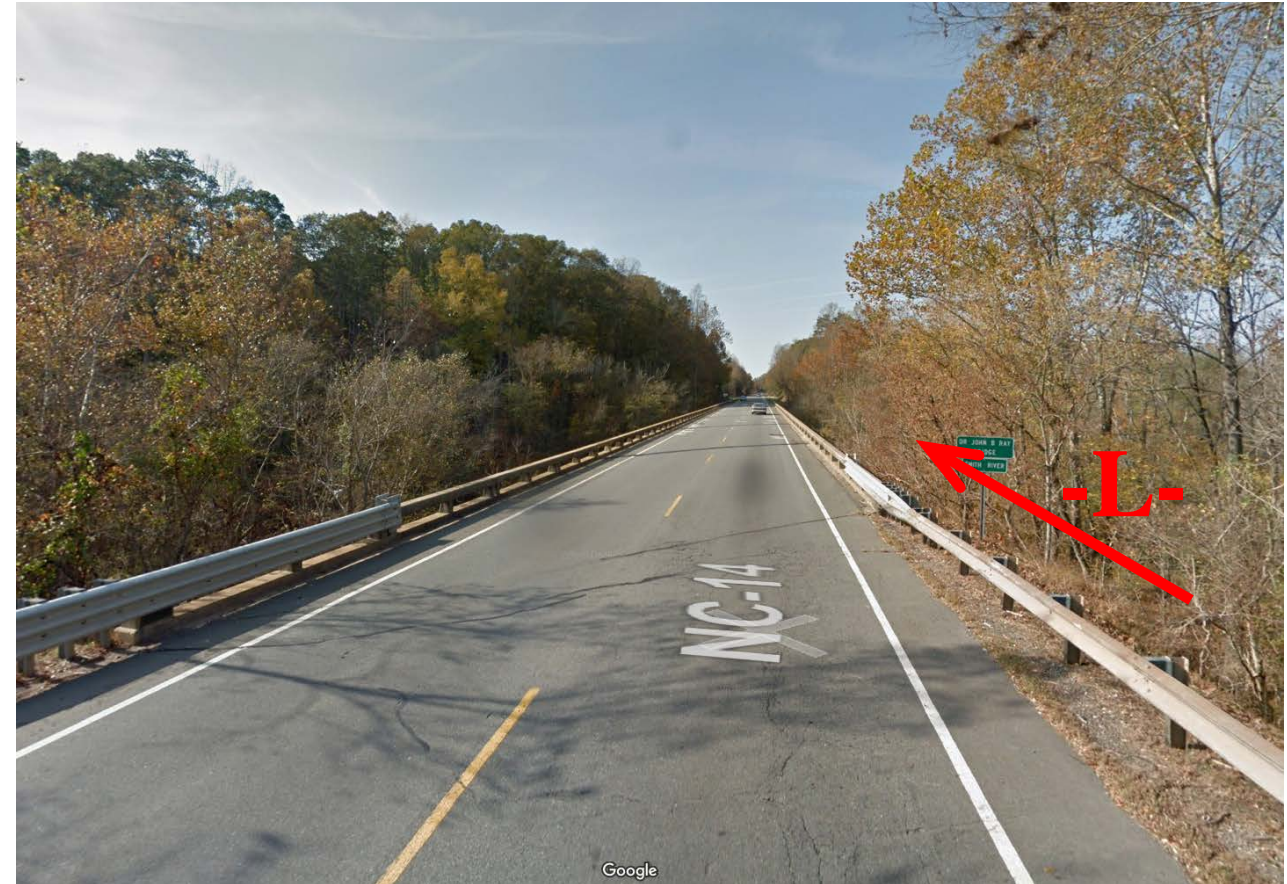
View near existing end bent 2, facing downstation (west)
