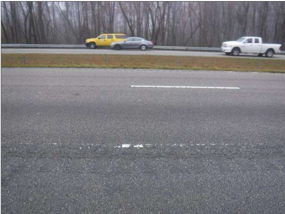
OVERVIEW NORTH BOUND LANES
