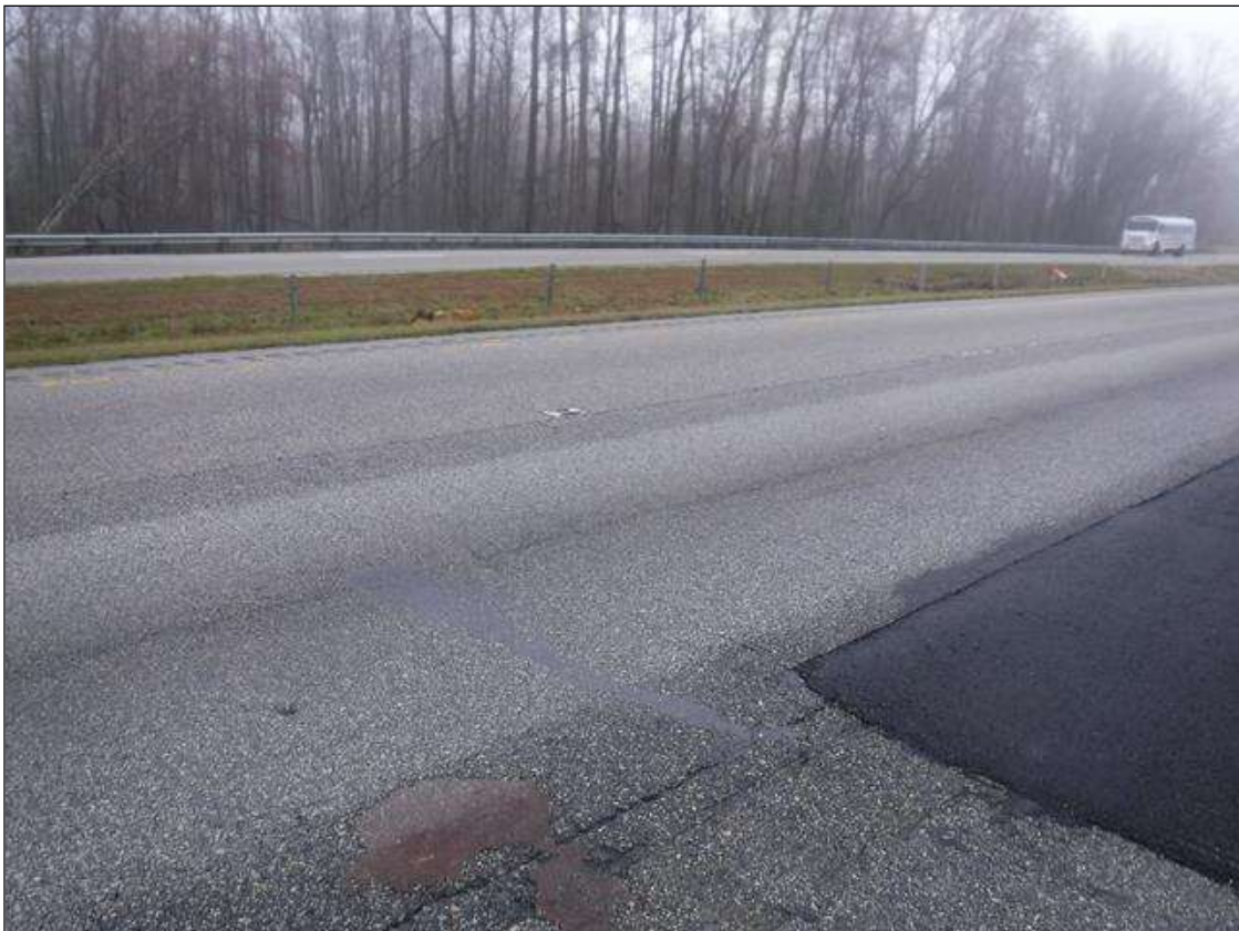
OVERVIEW SOUTH BOUND LANES
