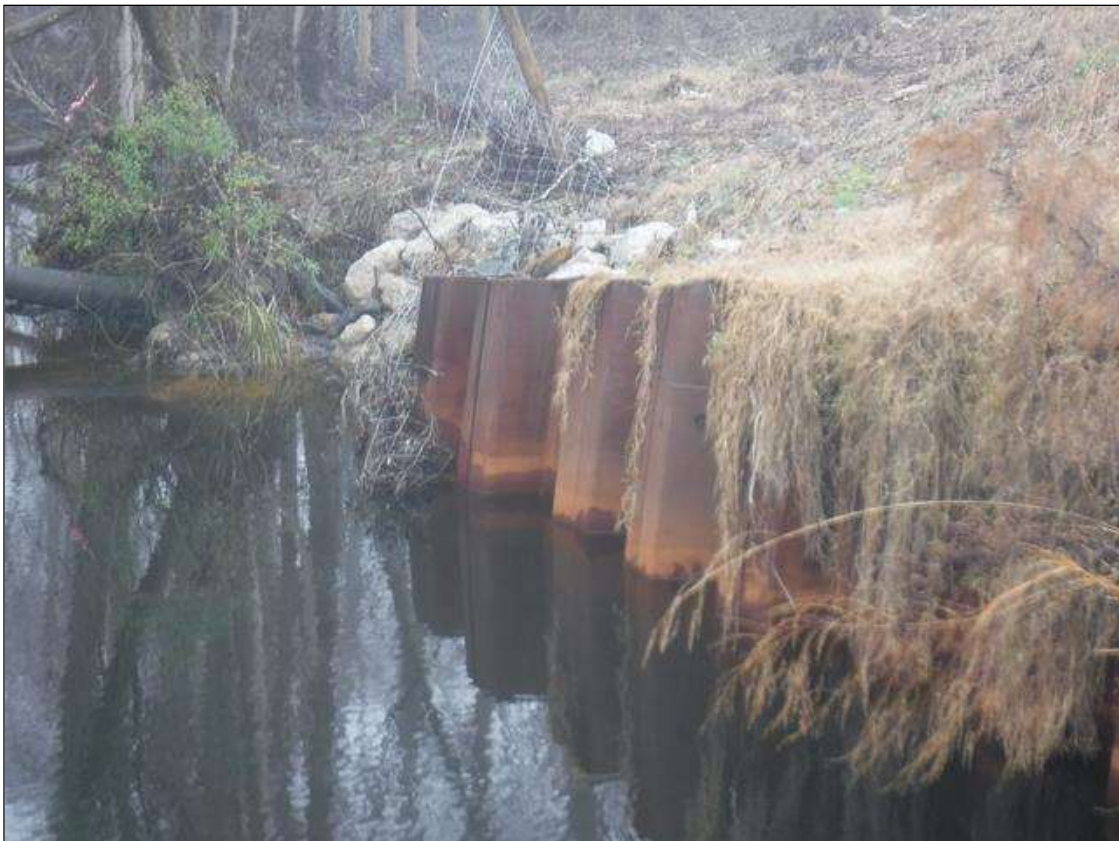
N.W. WING REPLACED WITH STEEL SHEETING
