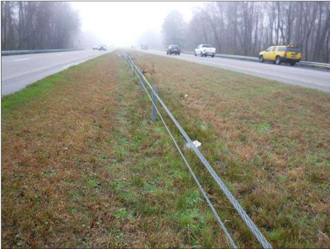
MEDIAN CABLE BARRIER
