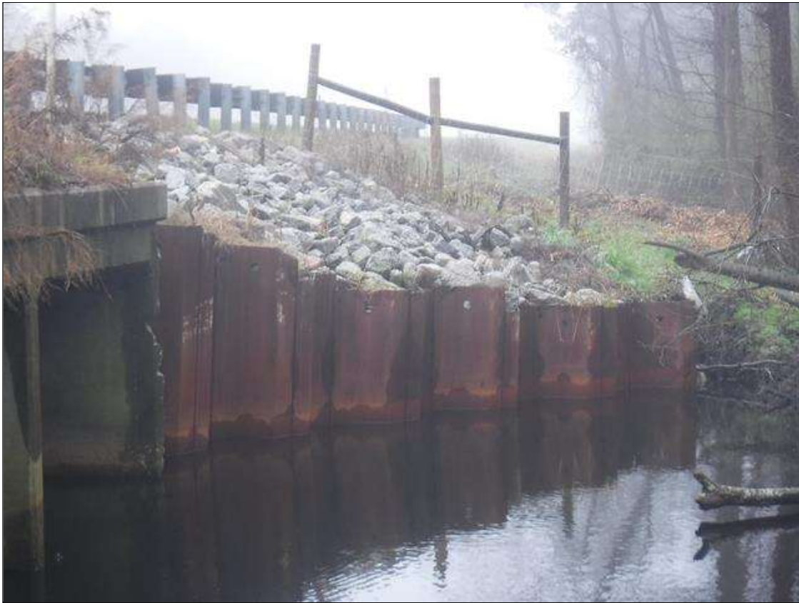
S.W. WING REPLACED WITH STEEL SHEETING
