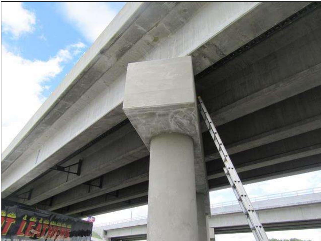
WEST END OF BENT 1 CAP
