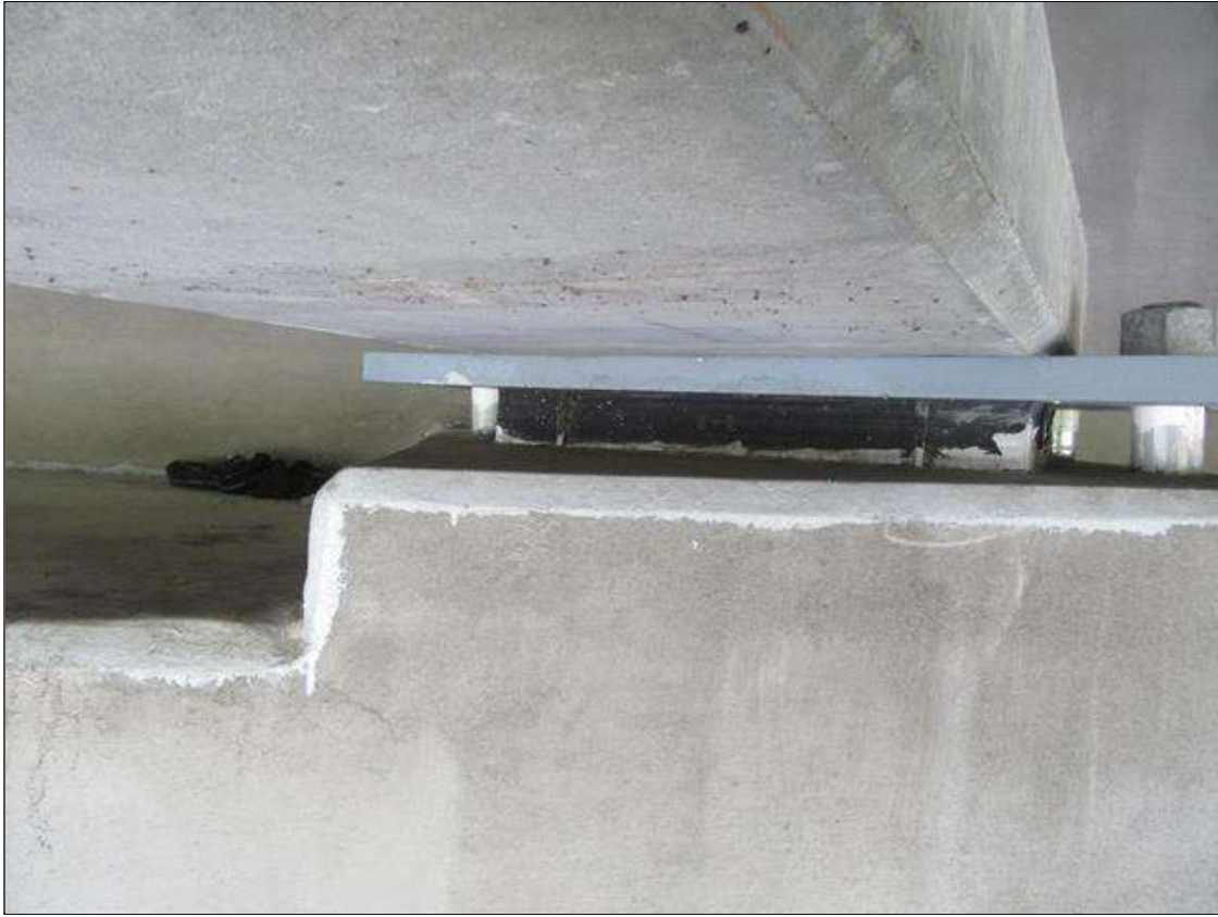
SPAN 1 BEAM 3 NEAR BEARING
