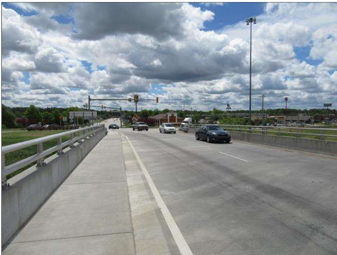
LOOKING SOUTH, OFF BRIDGE
