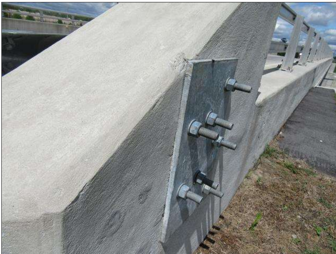
EXTERIOR GUARDRAIL CONNECTION
