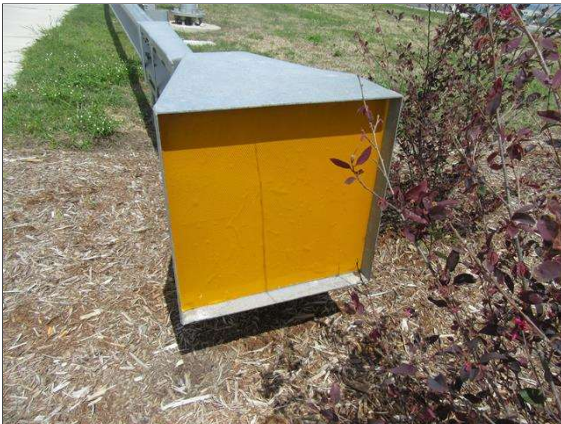
GUARDRAIL END TERMINAL
