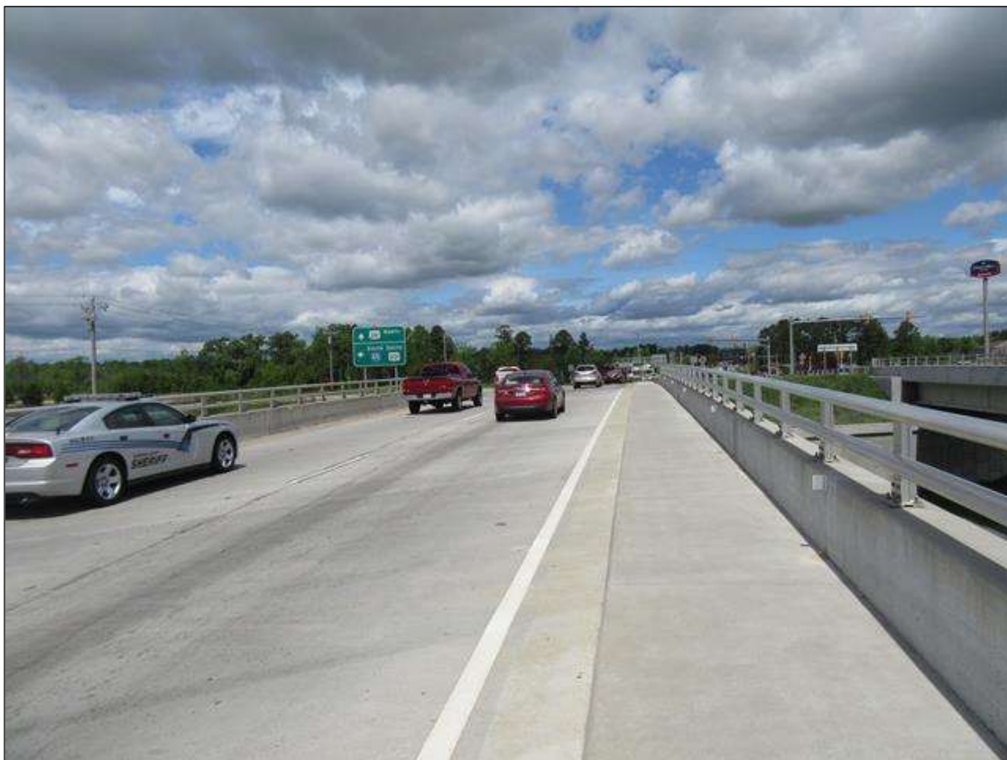
LOOKING NORTH, OFF BRIDGE
