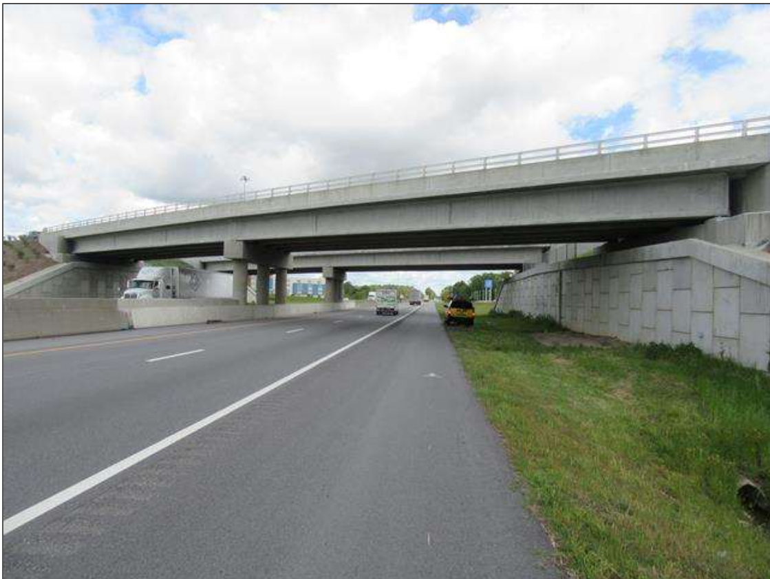
LOOKING EAST, NORTHBOUND LANE I-95 THRU SPAN 1
