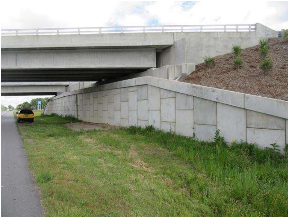
ABUTMENT 1 PPC EARTHWALL
