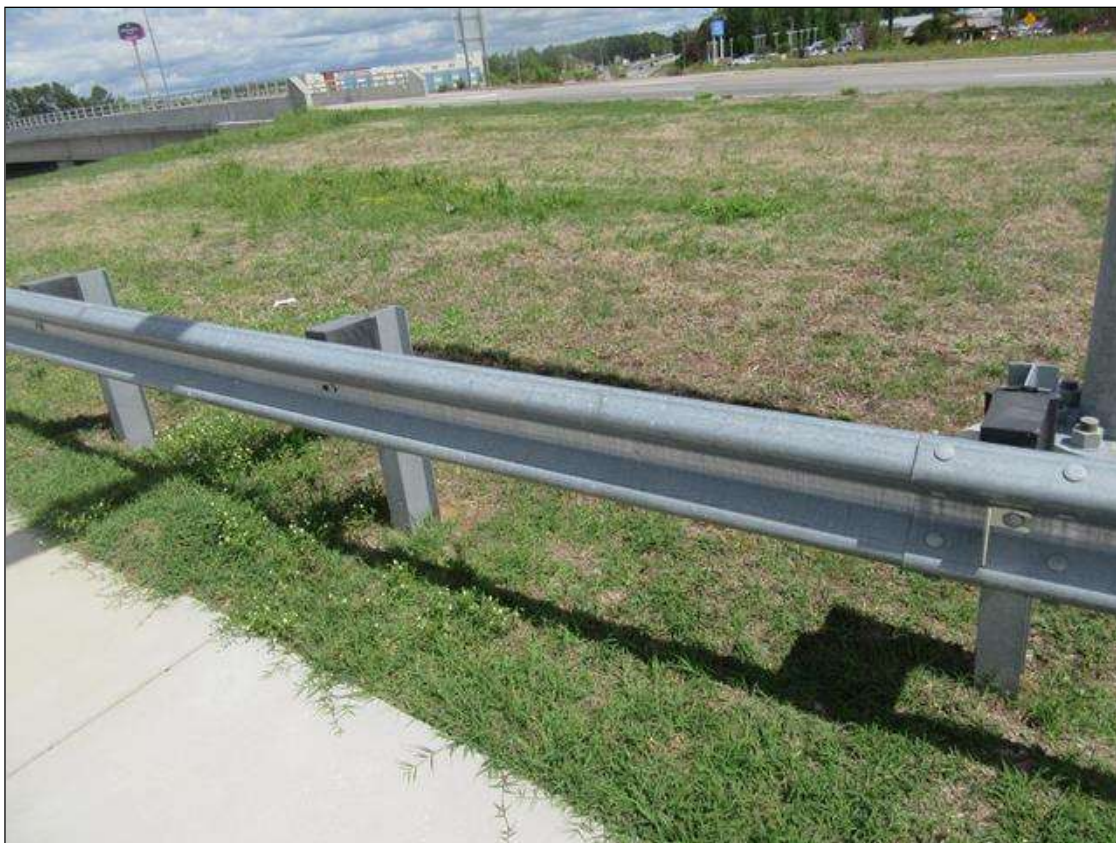
GUARDRAIL POST SPACING AT MID PORTION 6.25 FT.
