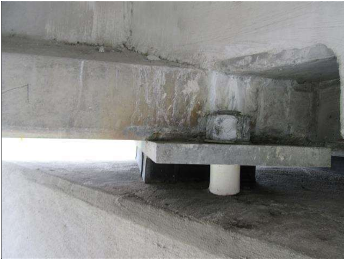
SPAN 1 BEAM 1 FAR BEARING
