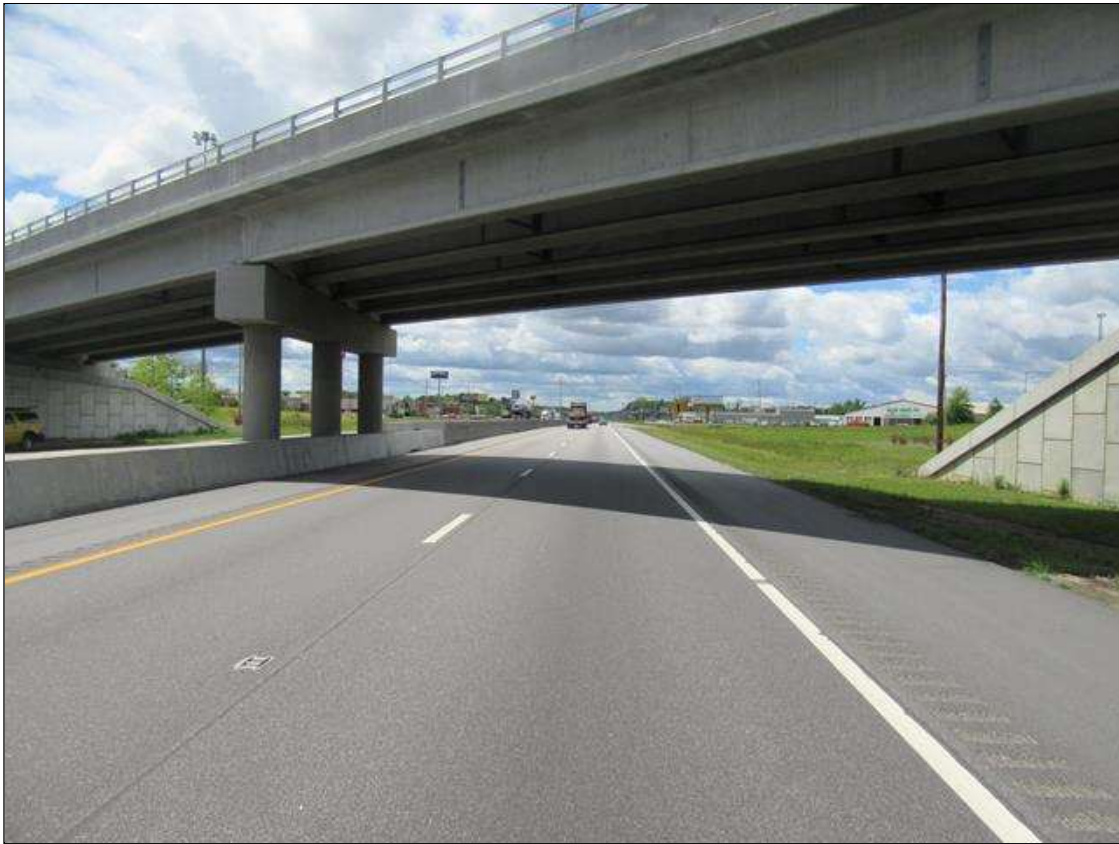
LOOKING WEST, SOUTHBOUND LANE I-95 THRU SPAN 2
