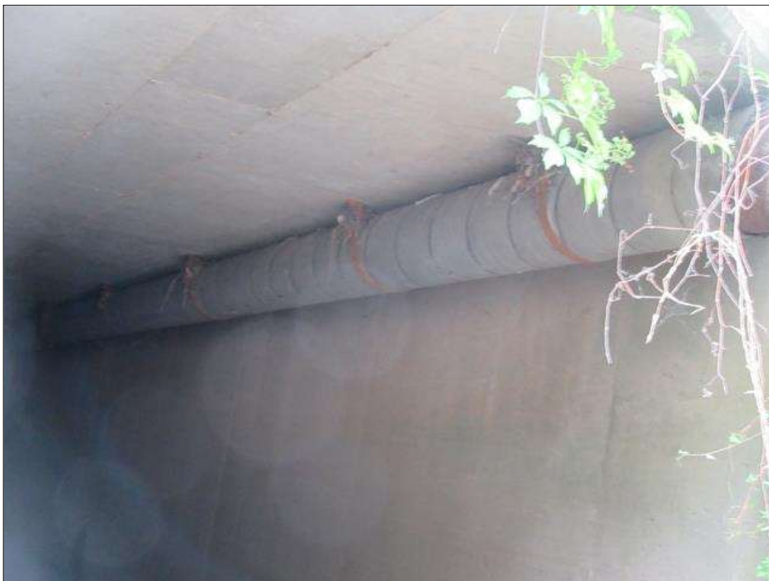
12" CAST IRON UTILITY BARREL 1 ALONG SOUTH WALL
