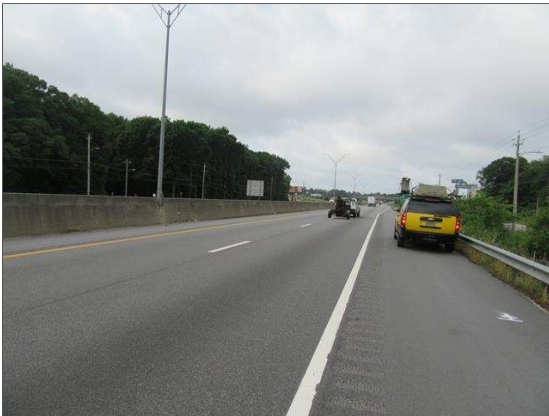
LOOKING SOUTH, SOUTHBOUND LANE I-95
