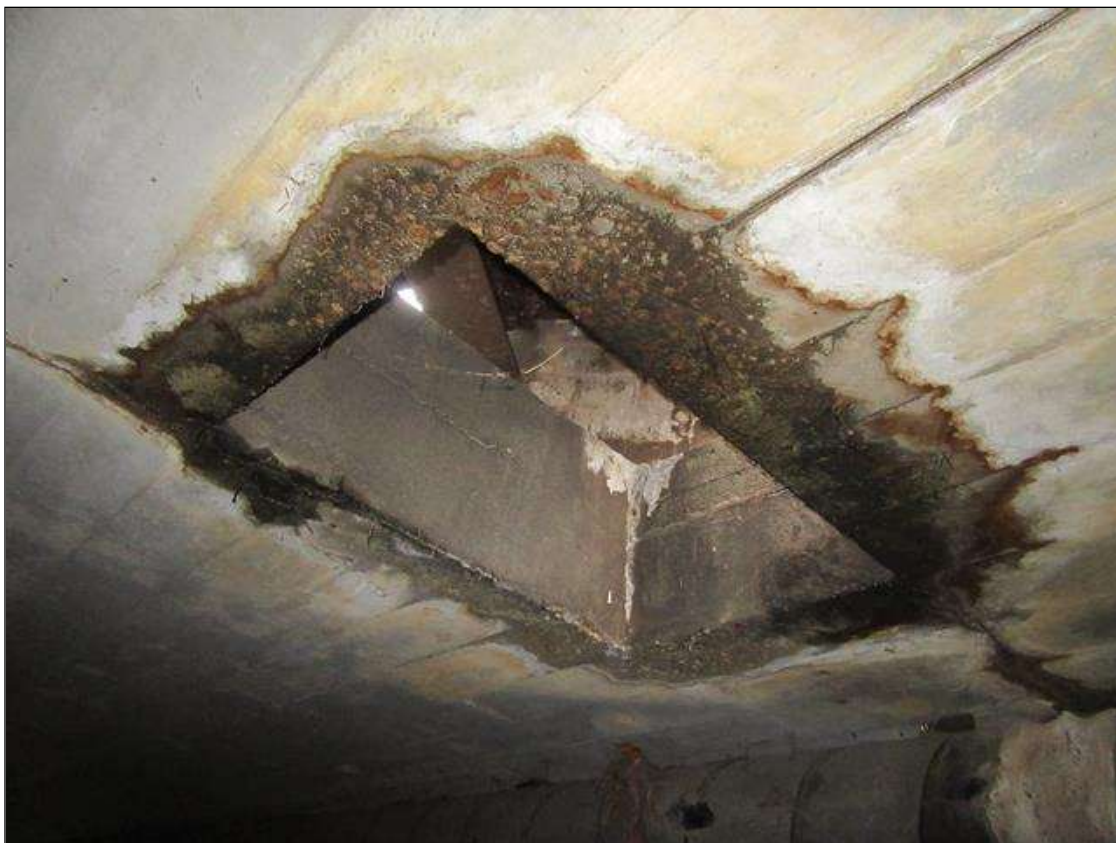
STORM WATER INLET TOP SLAB BARREL 1 AT MID POINT
