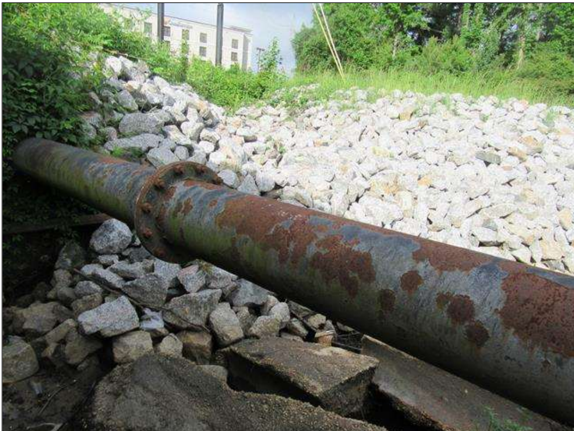
12" CAST IRON UTILITY 8' WEST OF CULVERT
