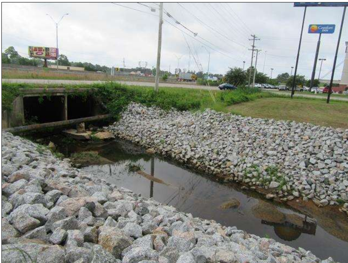
RIP RAP SLOPE PROTECTION , HURRICANE MATTHEW REPAIR
