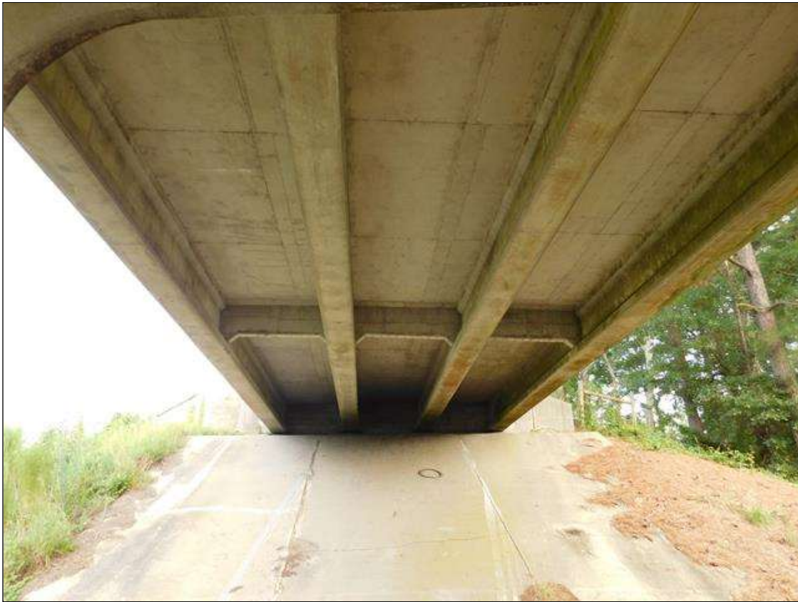
SPAN 4 SUPERSTRUCTURE, SPAN 1 SIMILAR
