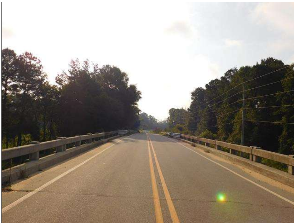
LOOKING EAST, OFF BRIDGE
