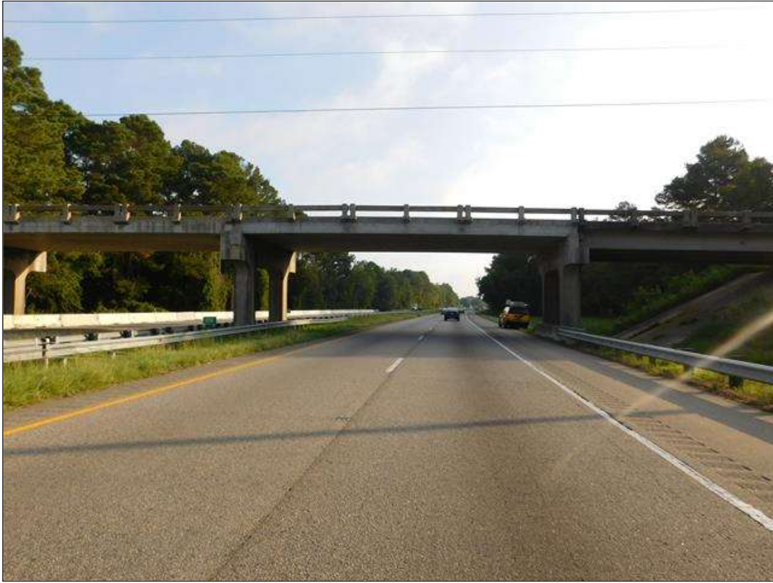
LOOKING NORTH, NORTHBOUND LANE I-95 THRU SPAN 3
