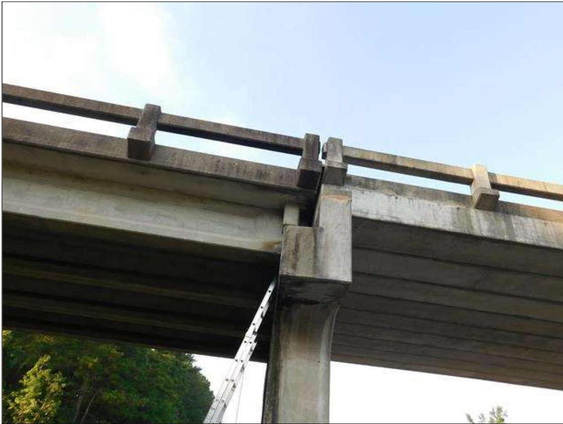
NORTH END OF BENT 3 CAP
