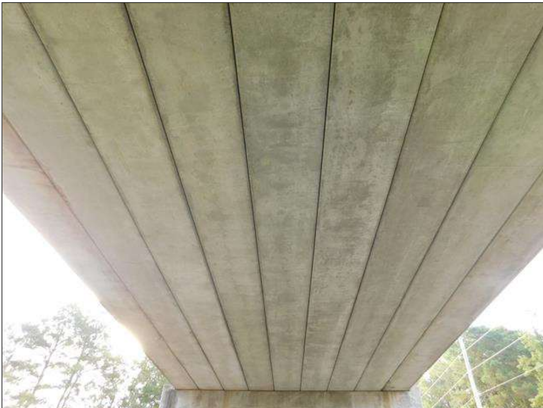
SPAN 3 SUPERSTRUCTURE, SPAN 2 SIMILAR
