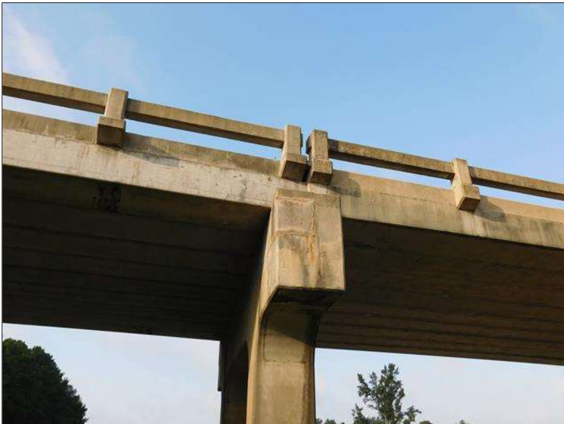
NORTH END OF BENT 2 CAP
