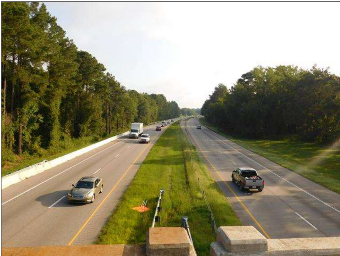
LOOKING NORTH, I-95
