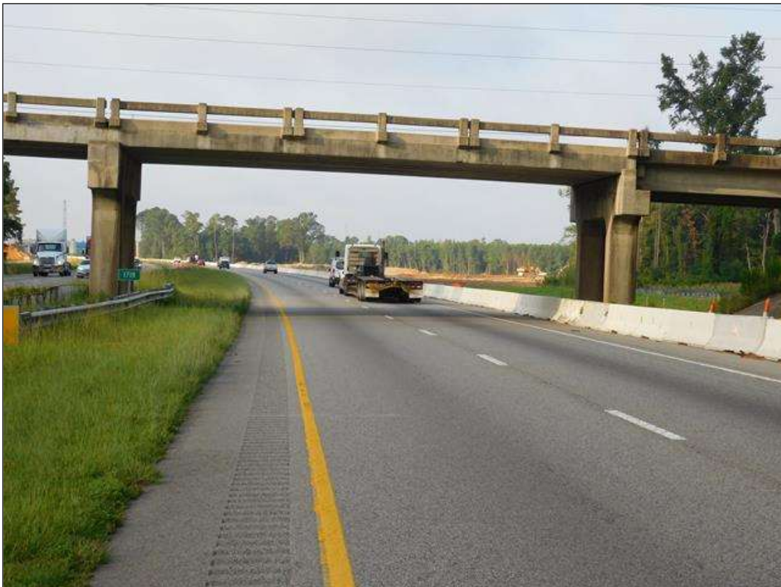
LOOKING SOUTH, SOUTHBOUND LANE I-95 THRU SPAN 2
