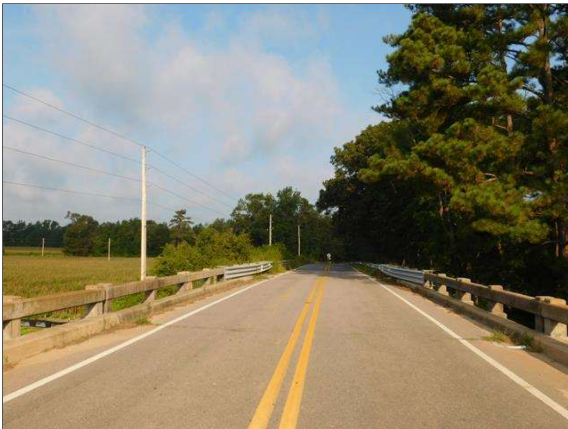
LOOKING WEST, OFF BRIDGE
