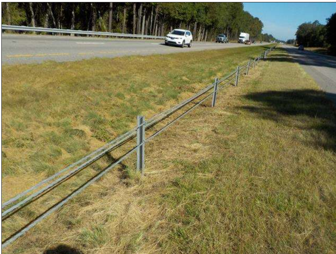
MEDIAN CABLE RAIL
