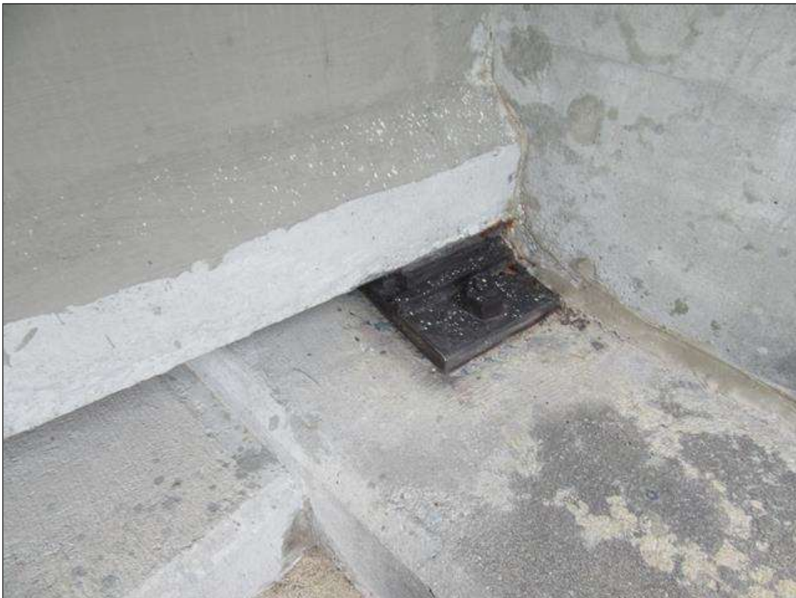
SPAN 4 BEAM 4 FAR BEARING, ALL BEARINGS IN SPANS 1 AND 4 ARE SIMILAR
