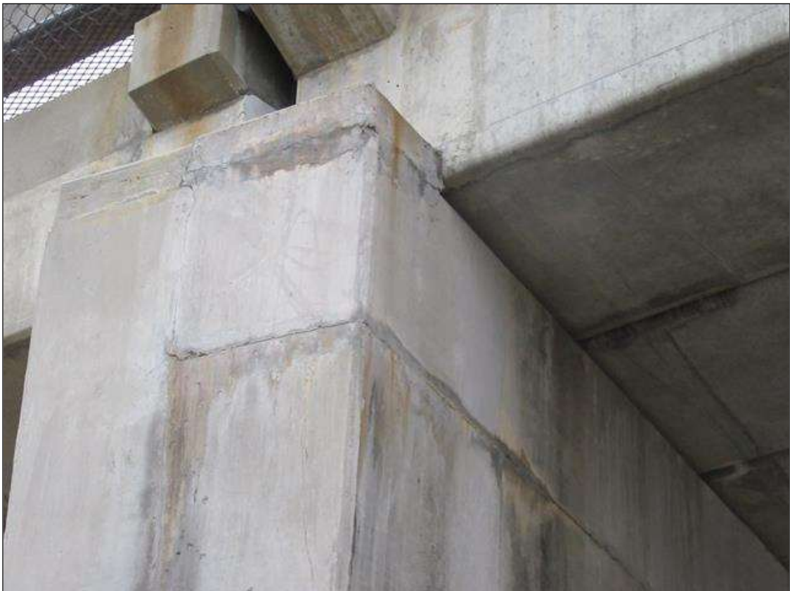
CONSTRUCTION JOINT IN BENT 2 CAP
