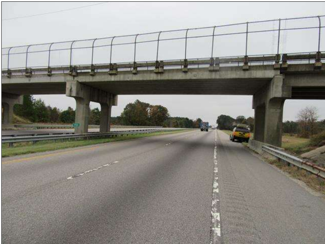
LOOKING SOUTH, SOUTHBOUND LANE I-95 THRU SPAN 2
