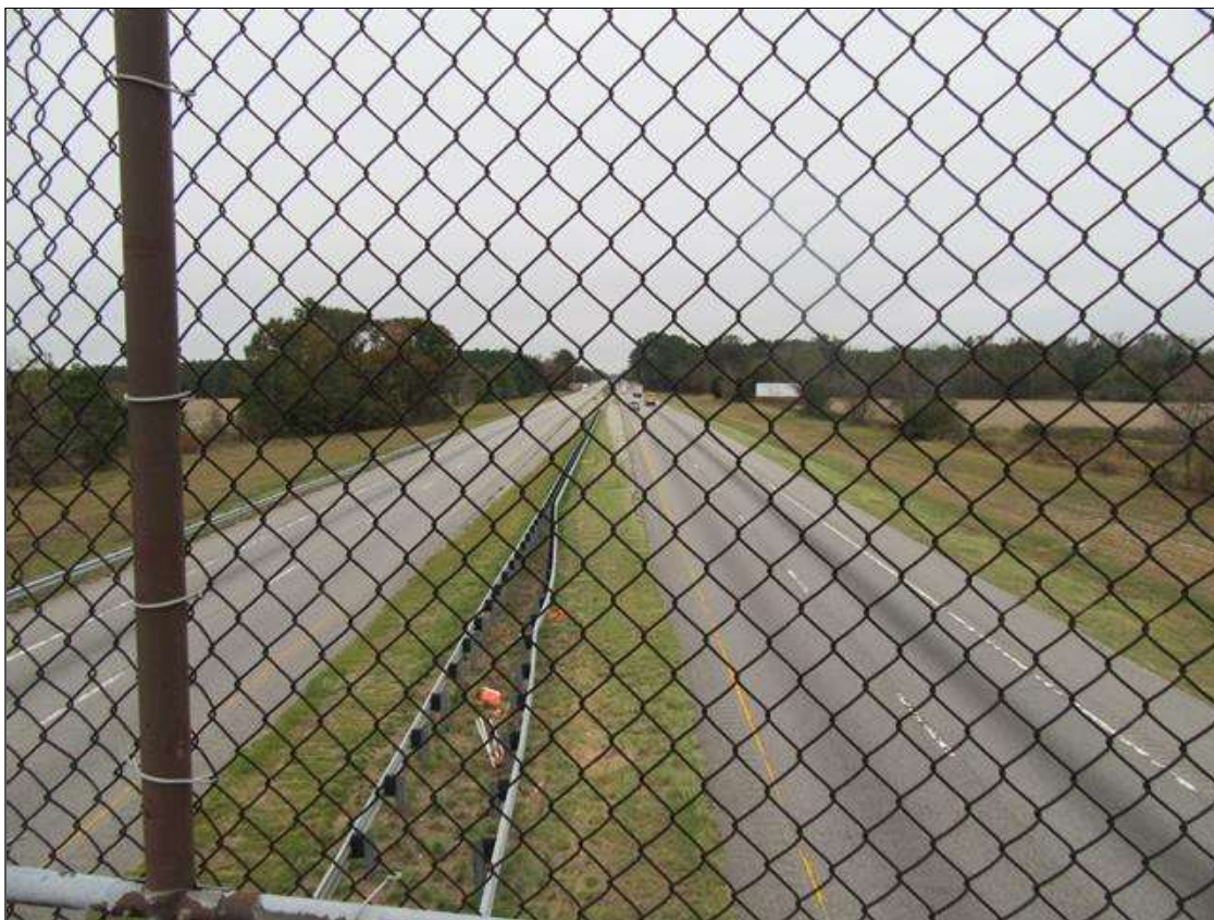
LOOKING SOUTH, I - 95
