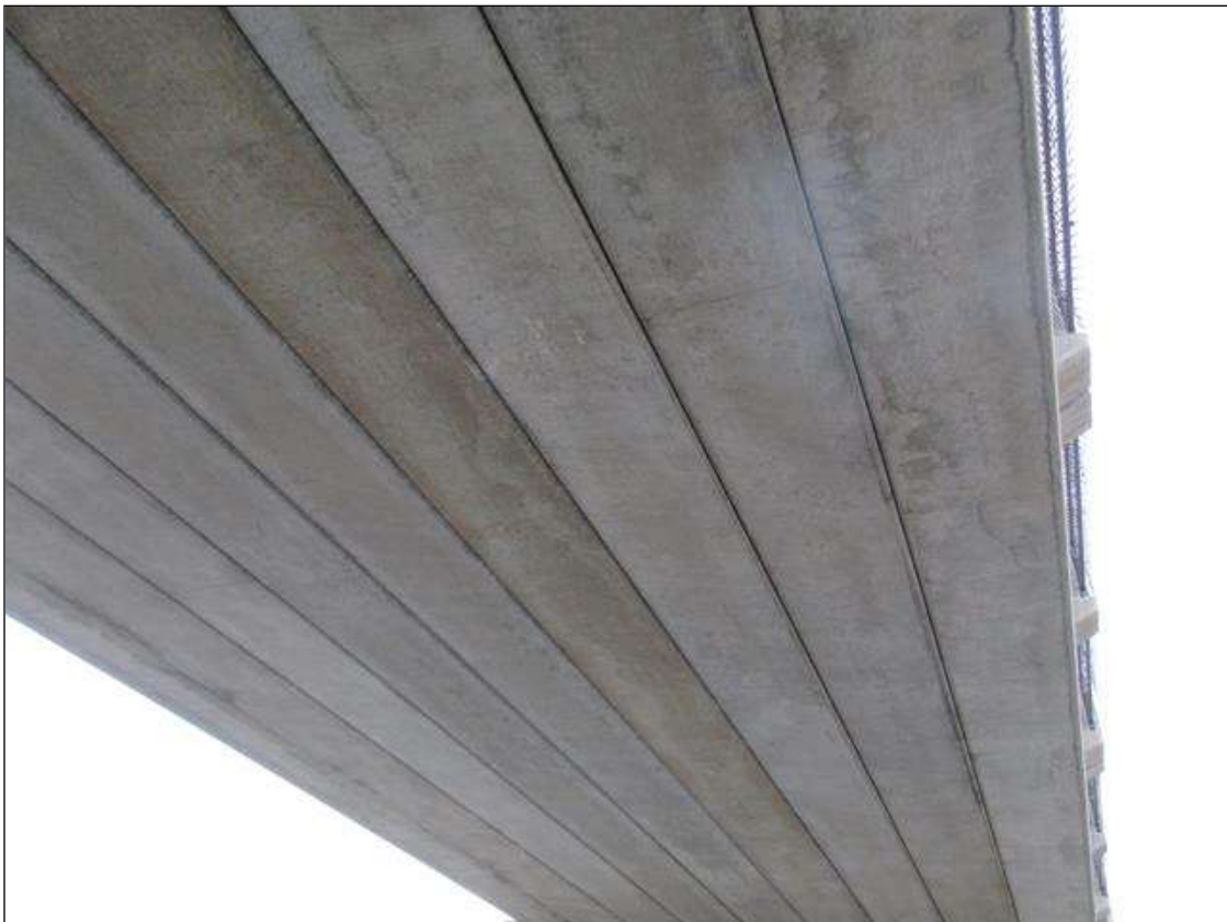
SPAN 3 SUPERSTRUCTURE, SPAN 2 SIMILAR
