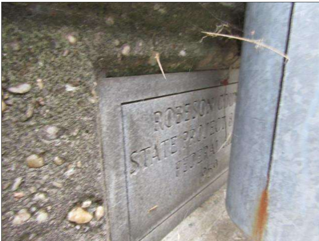
DATA PLATE IN RAIL AT SOUTHWEST CORNER
