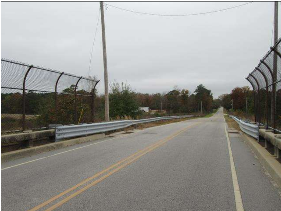
LOOKING WEST, OFF BRIDGE
