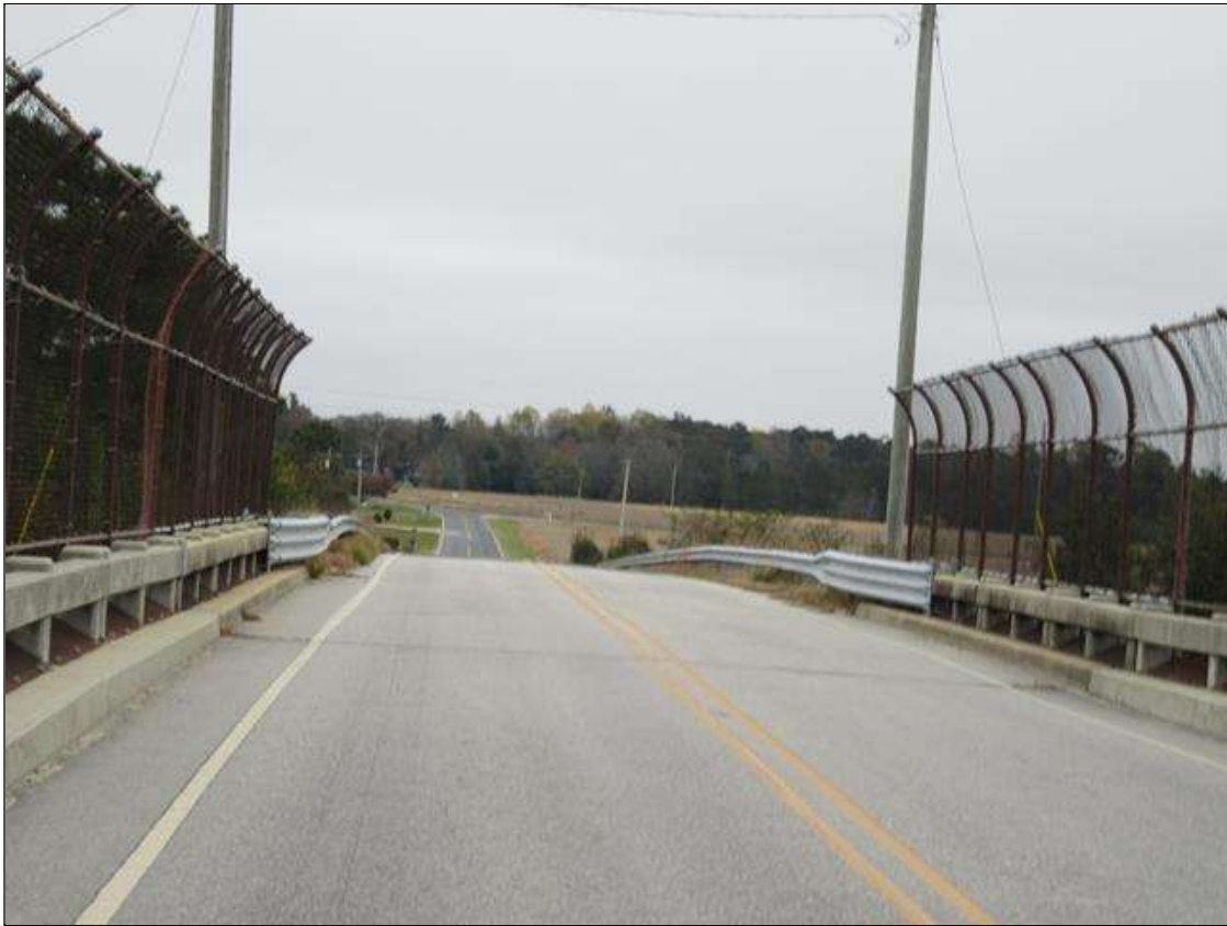
LOOKING EAST, OFF BRIDGE
