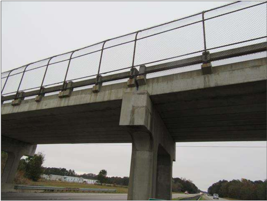
SOUTH END OF BENT 2 CAP
