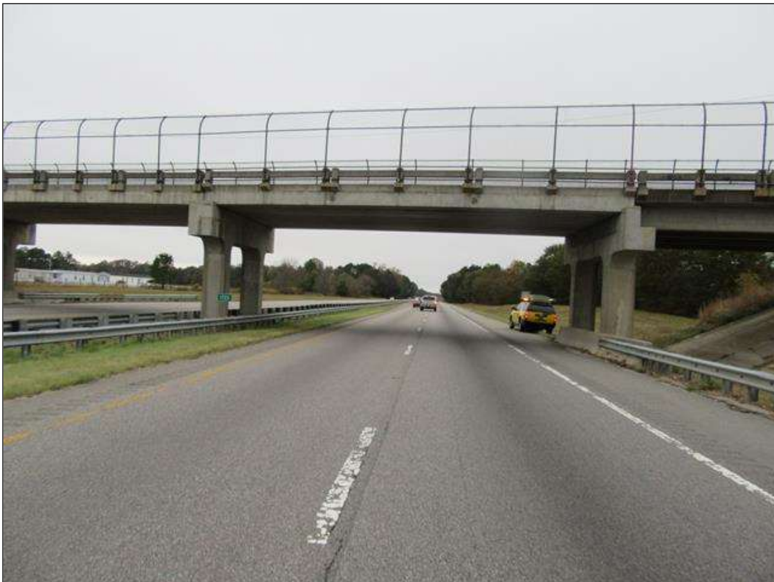
LOOKING NORTH, NORTHBOUND LANE I- 95 THRU SPAN 3
