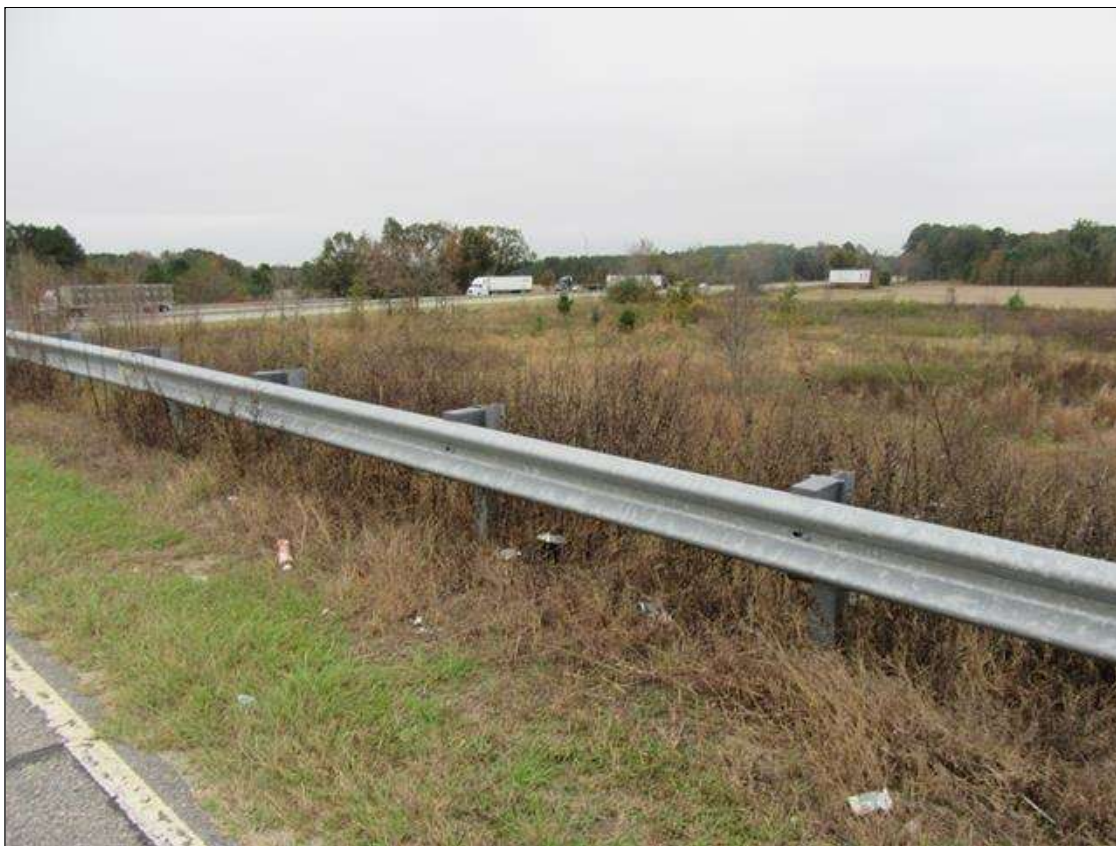
GUARDRAIL POST SPACING AT MIDPORTION
