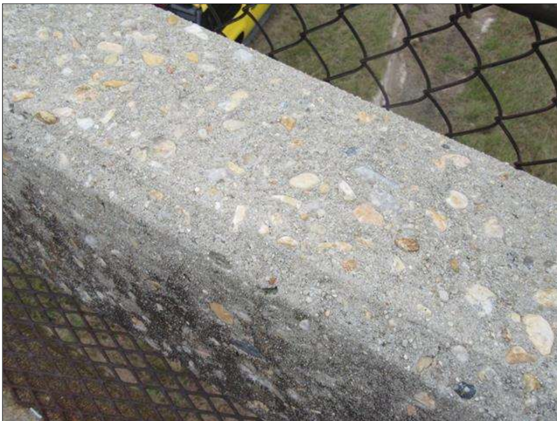
SPAN 1 RIGHT RAIL 35 FT OF EXPOSED AGGREGATE
