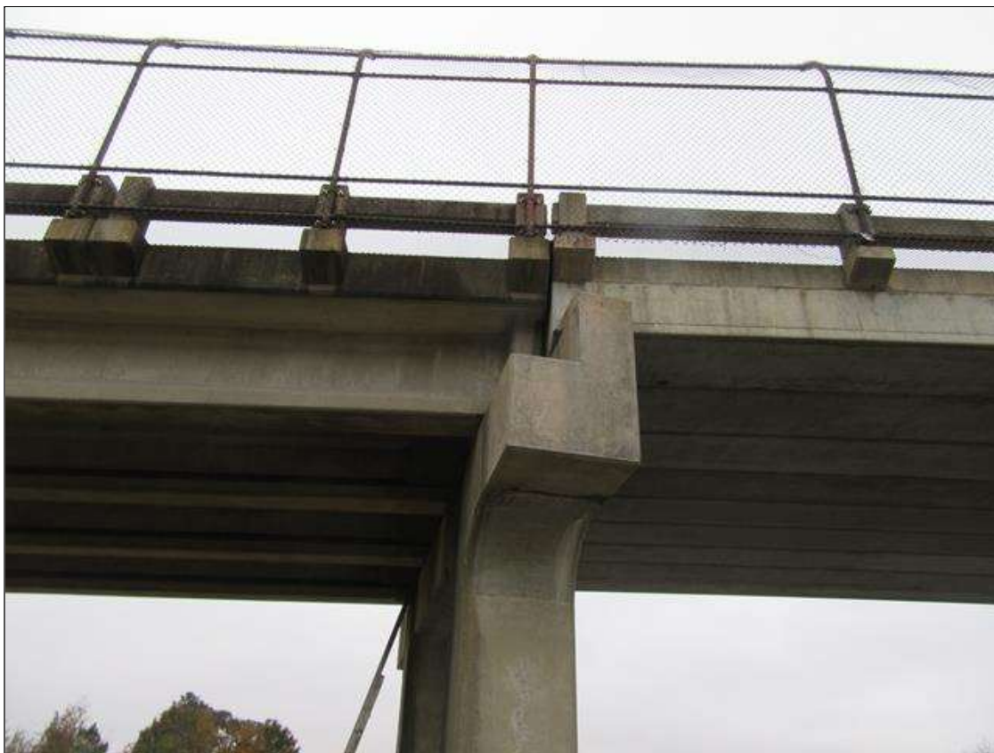
NORTH END OF BENT 3 CAP
