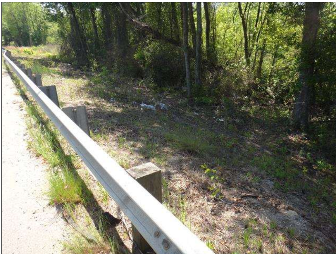
Southwest guardrail looking South
