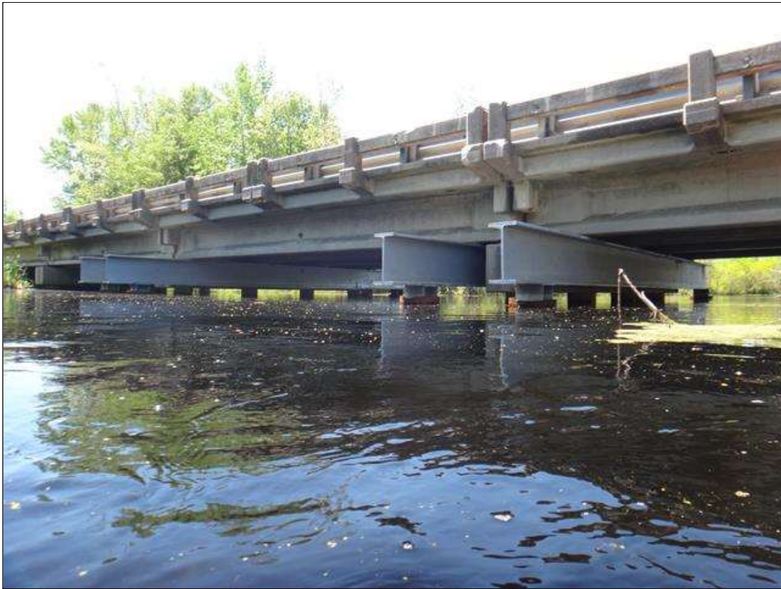
East profile looking West
