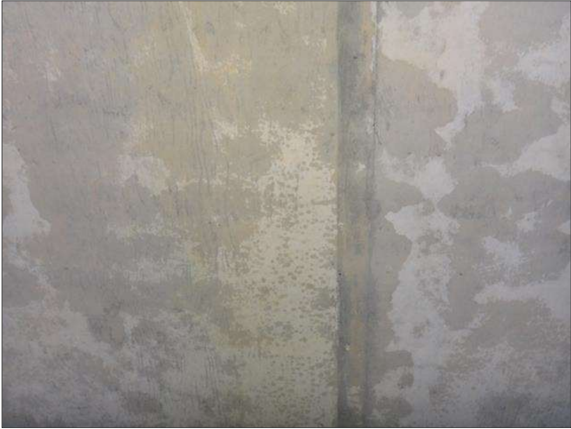
typical underside of deck
