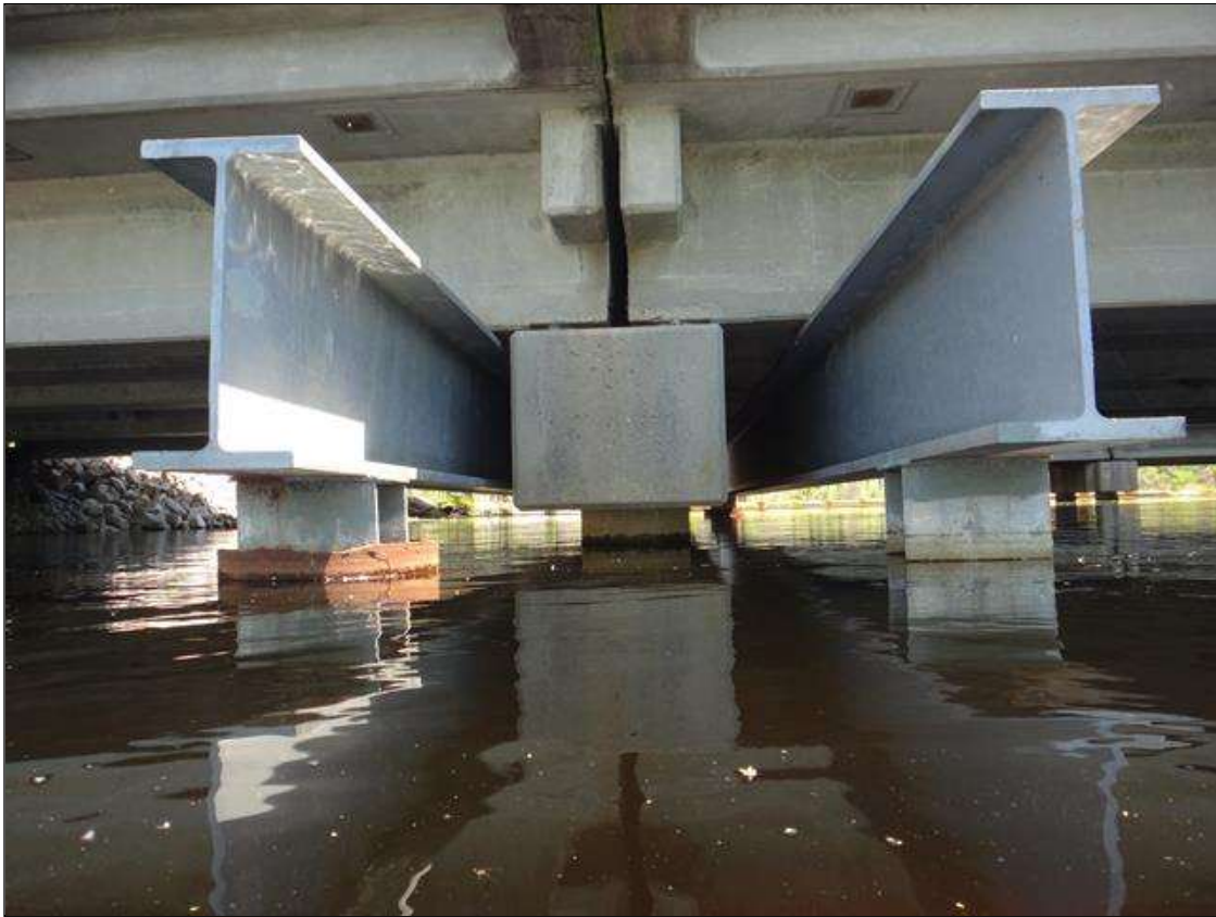
looking [East] at bent 3
