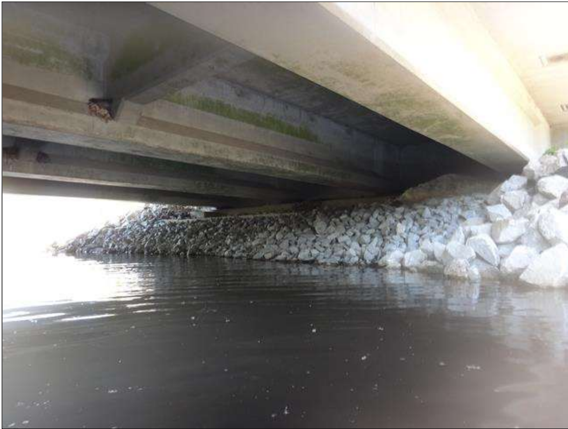
end bent 2 and slope protection
