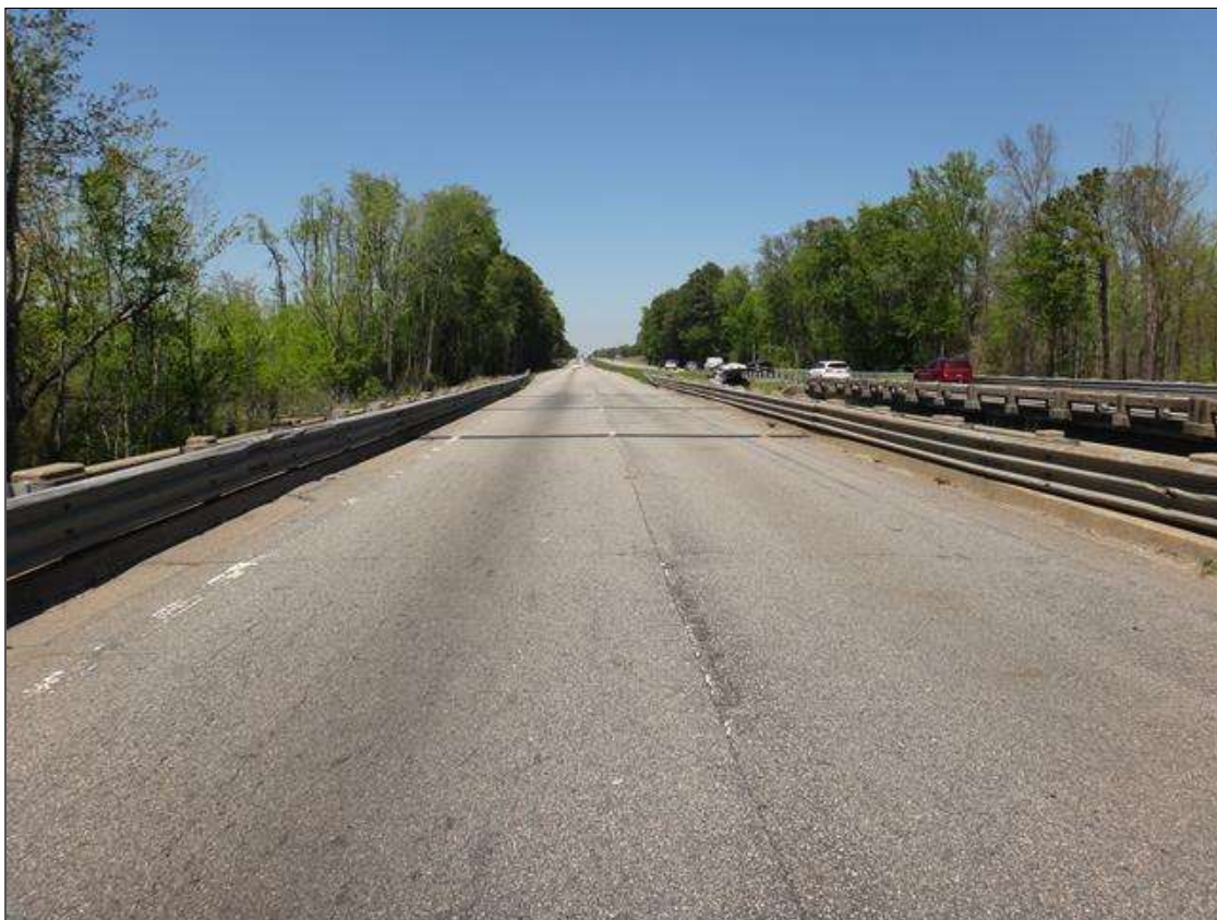
South approach looking North
