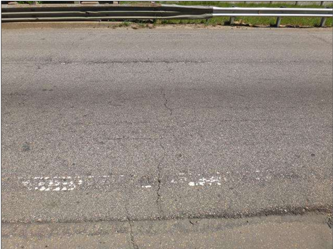
South approach asphalt
