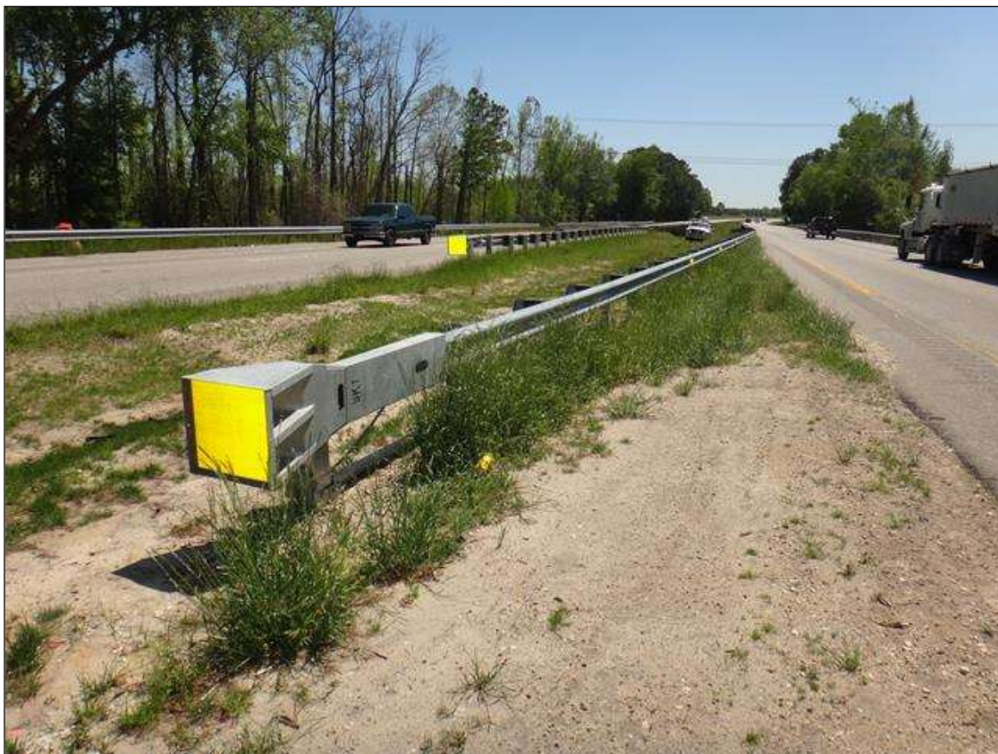
Northeast guardrail and end treatment
