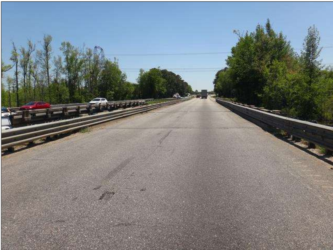
North approach looking South
