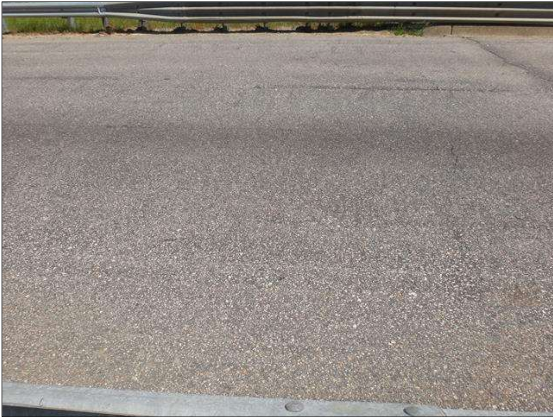
North approach asphalt
