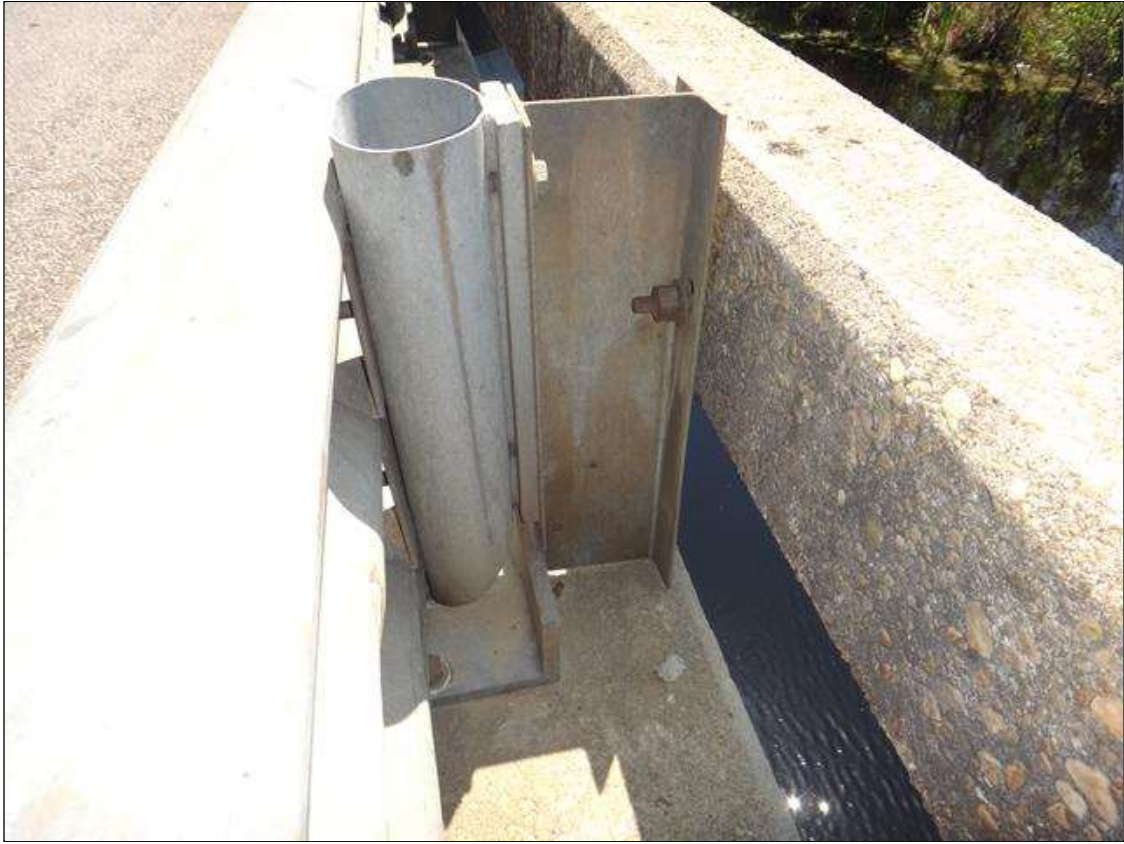
typical guardrail attachment to bridge rail
