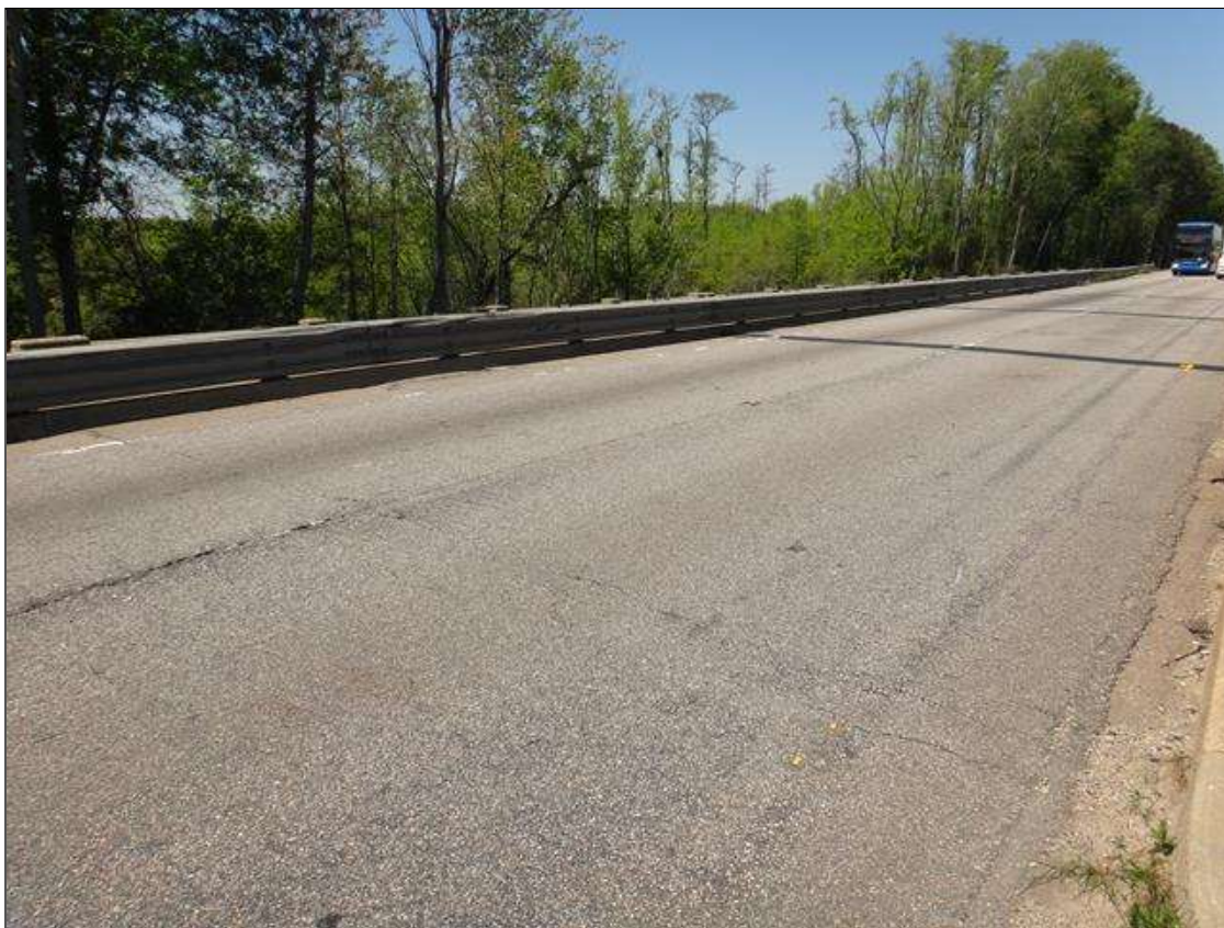
left bridge rail
