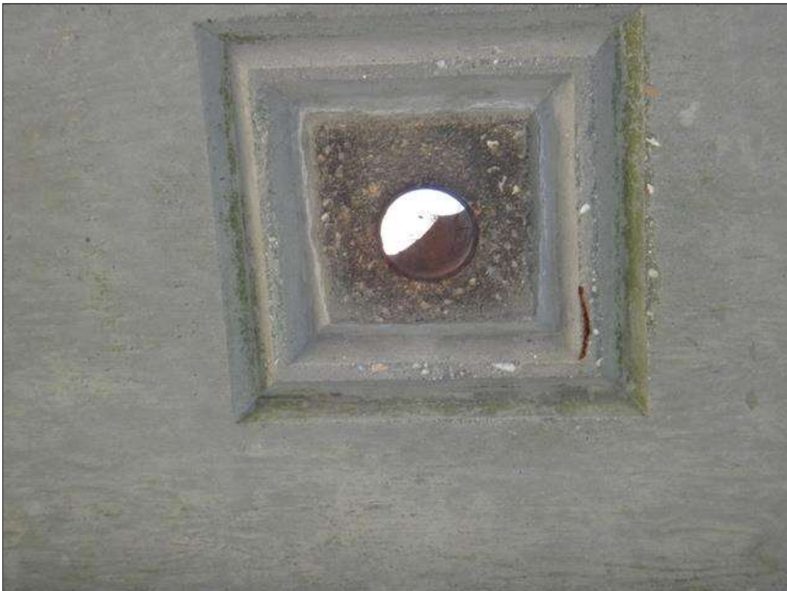
typical deck drain
