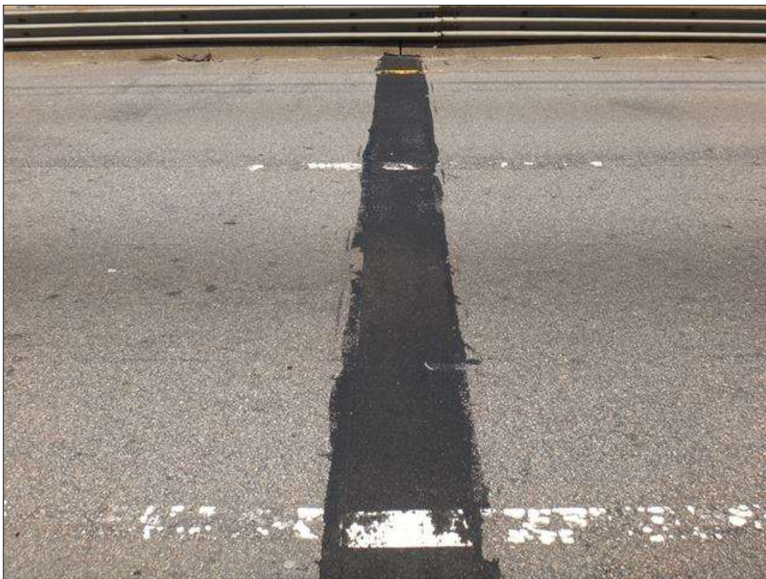
asphalt over bent 1
