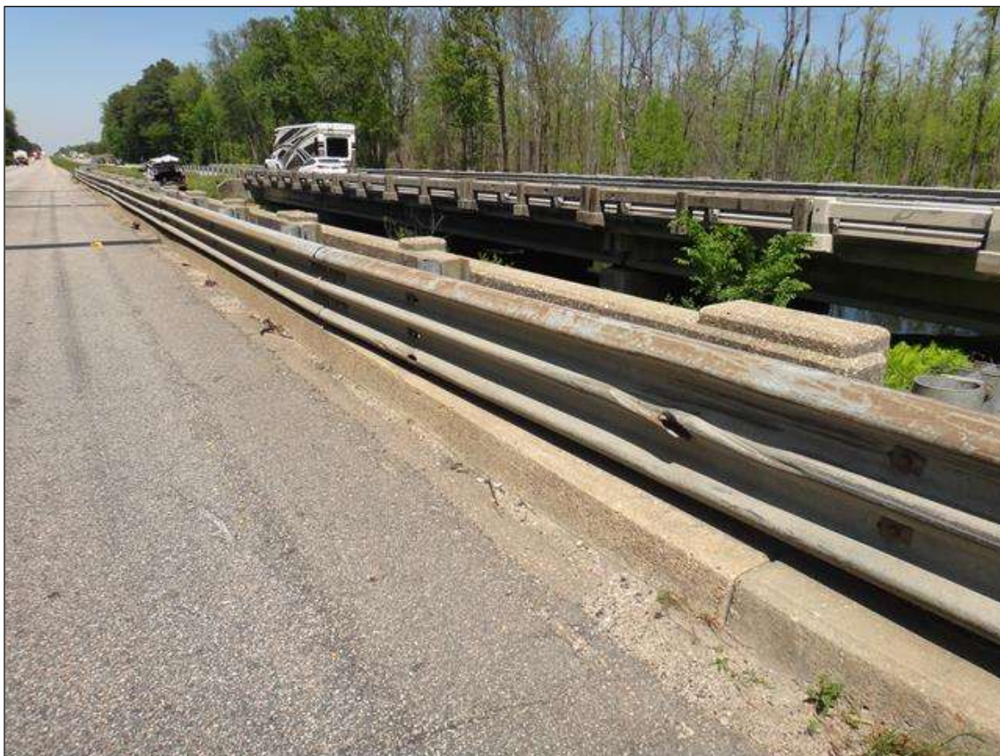
right bridge rail
