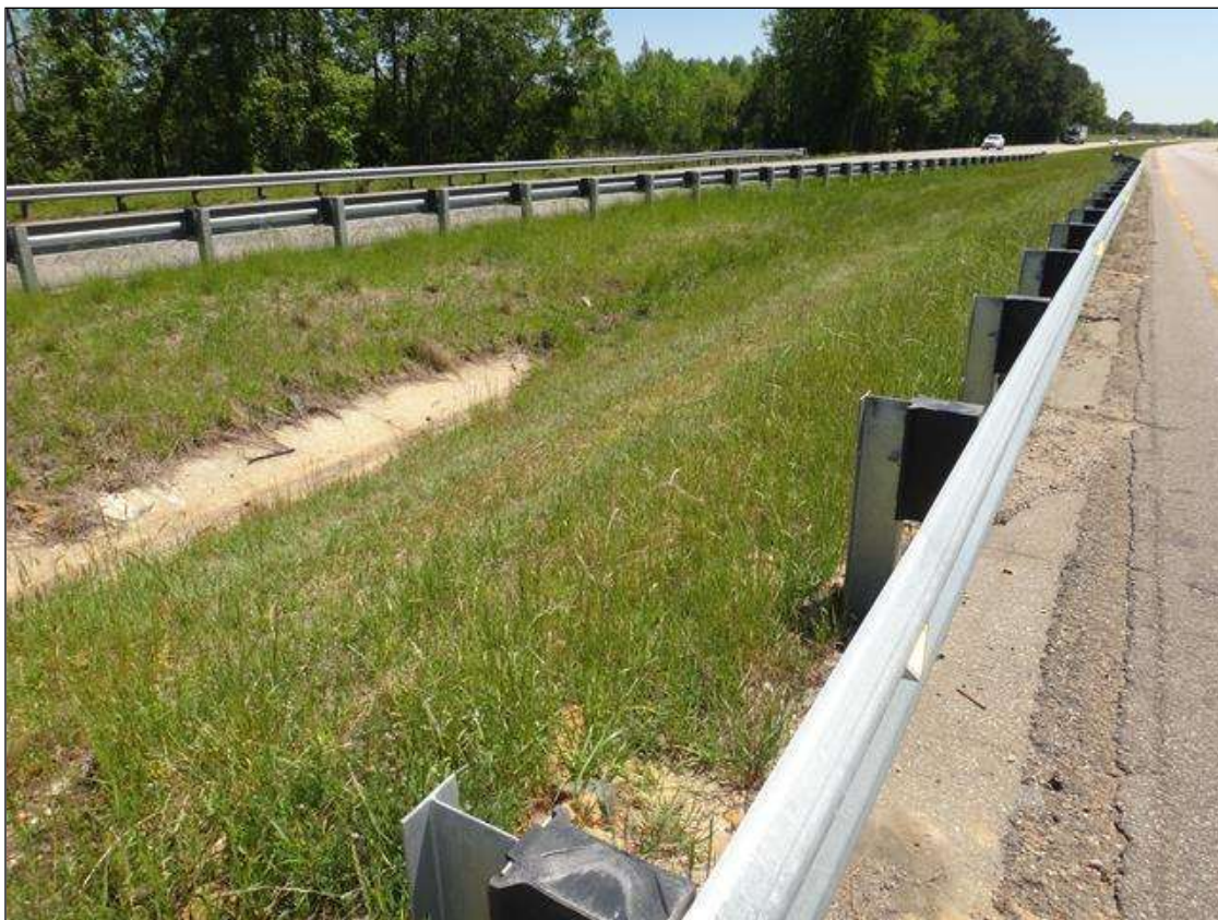
Southeast guardrail looking South
