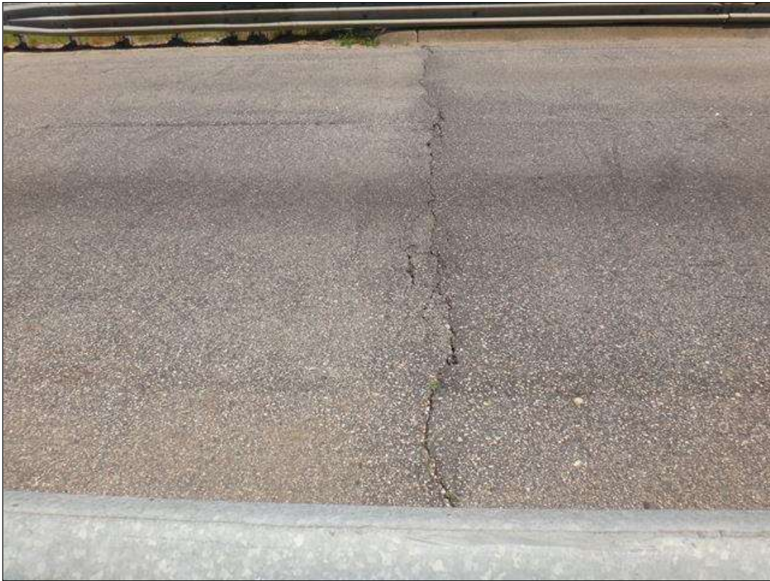
asphalt over end bent 2
