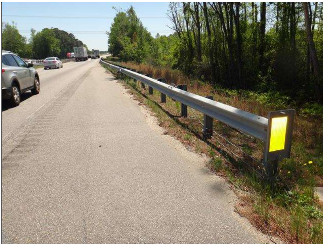
Northwest guardrail and end treatment
