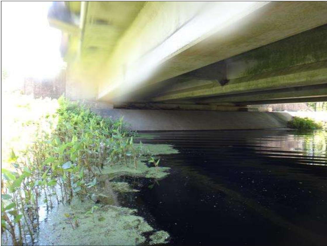
end bent 1 and slope protection
