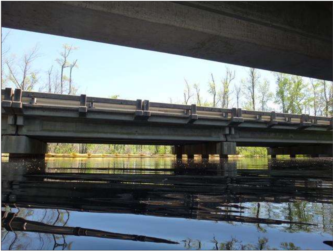
looking downstream [East] from underneath bridge
