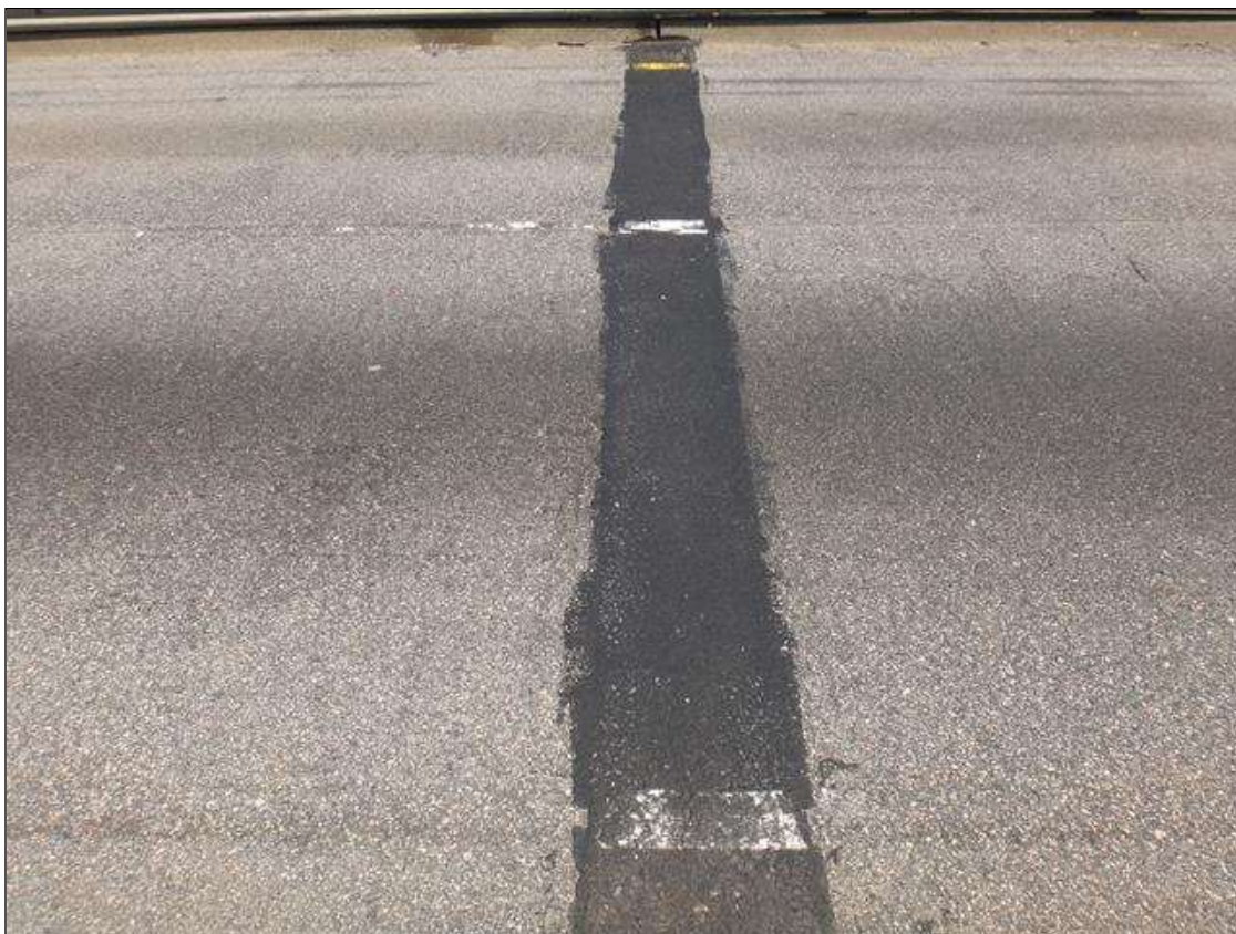
asphalt over bent 3
