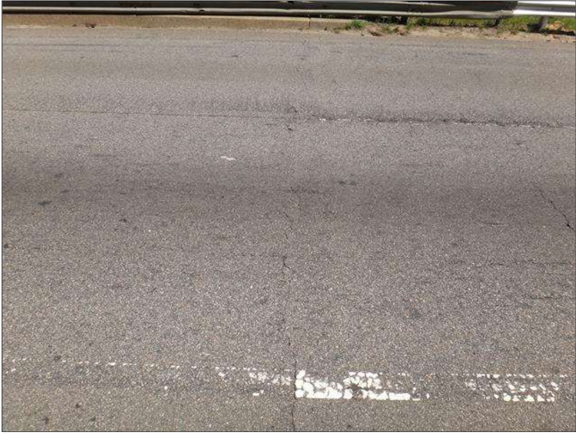
asphalt over end bent 1
