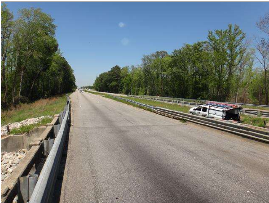
North approach looking North
