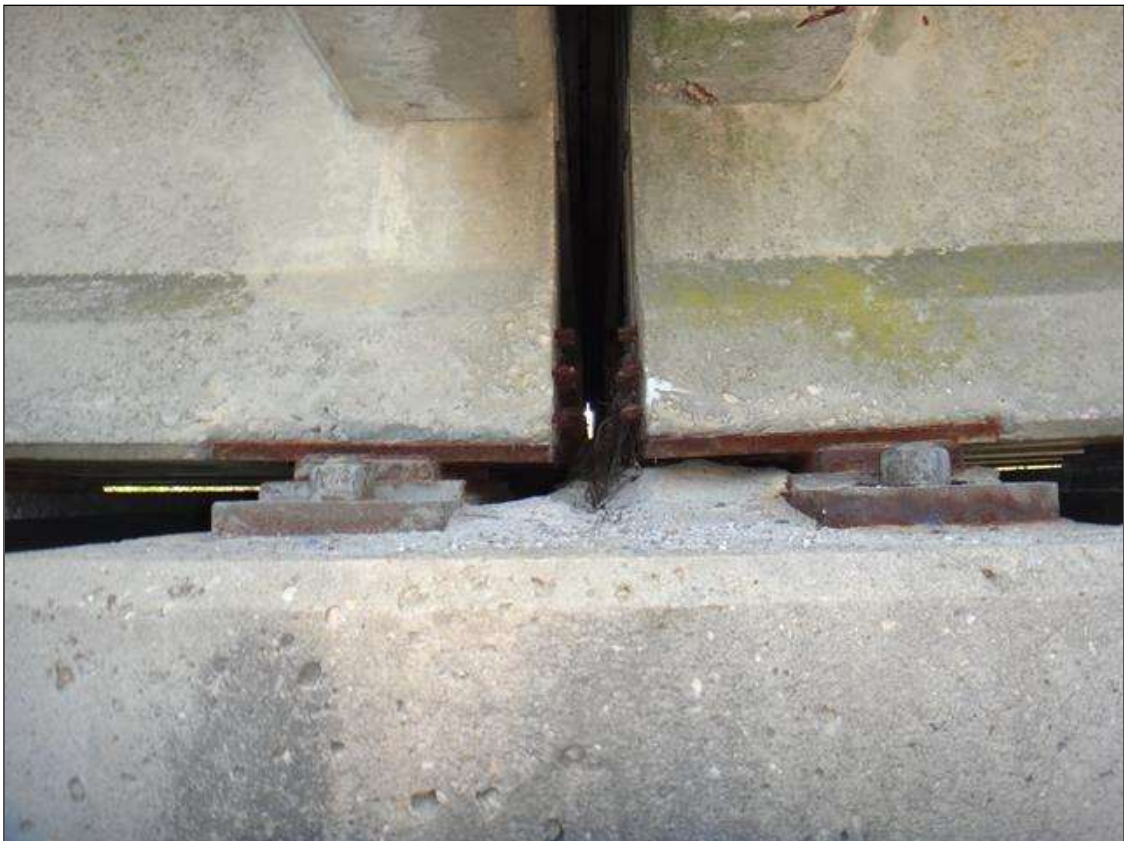
typical beam over interior bent
