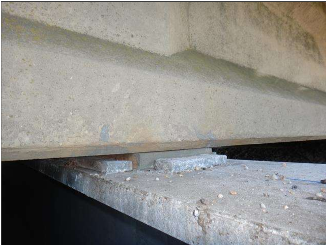
typical bearing at crutch bent
