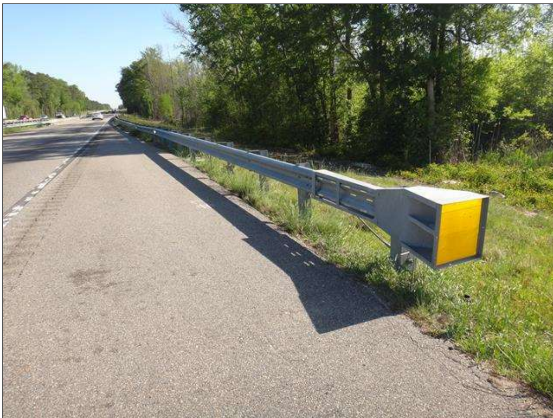
Southeast guardrail and end treatment
