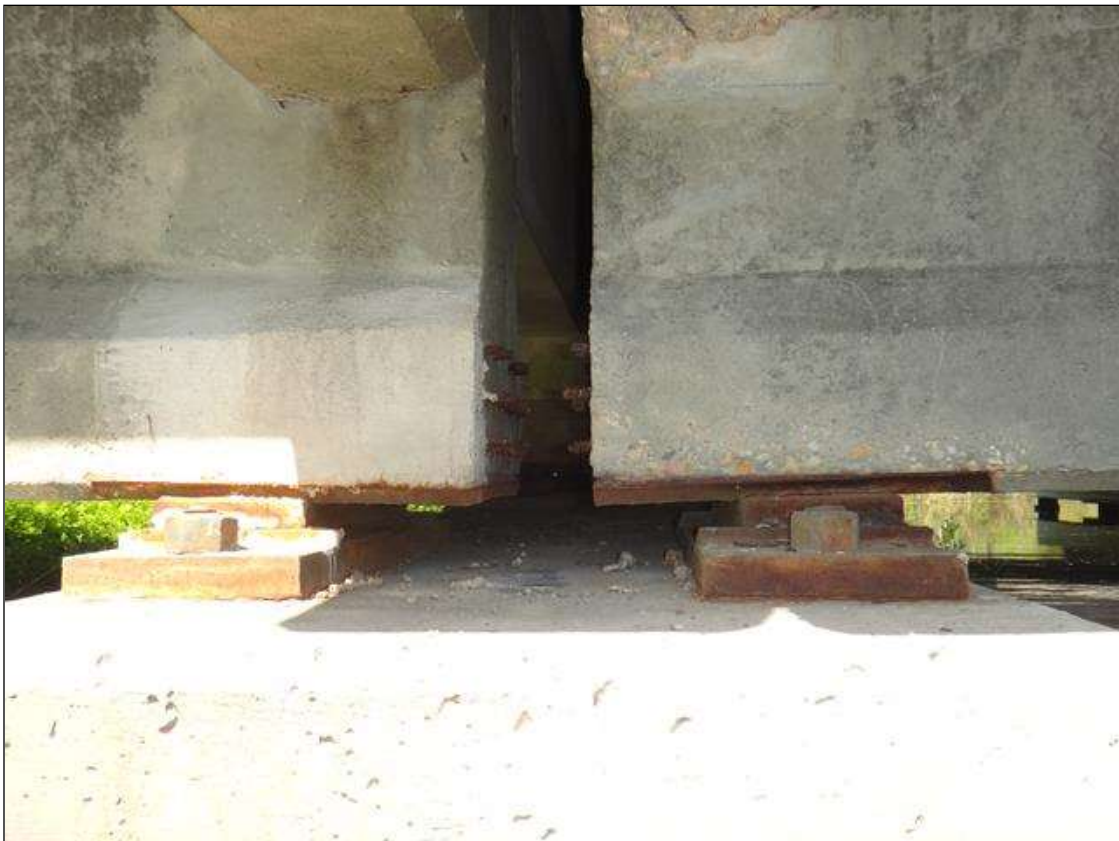
typical beam over interior bent
