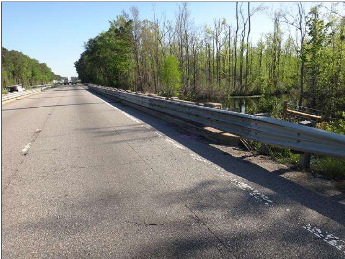
right bridge rail
