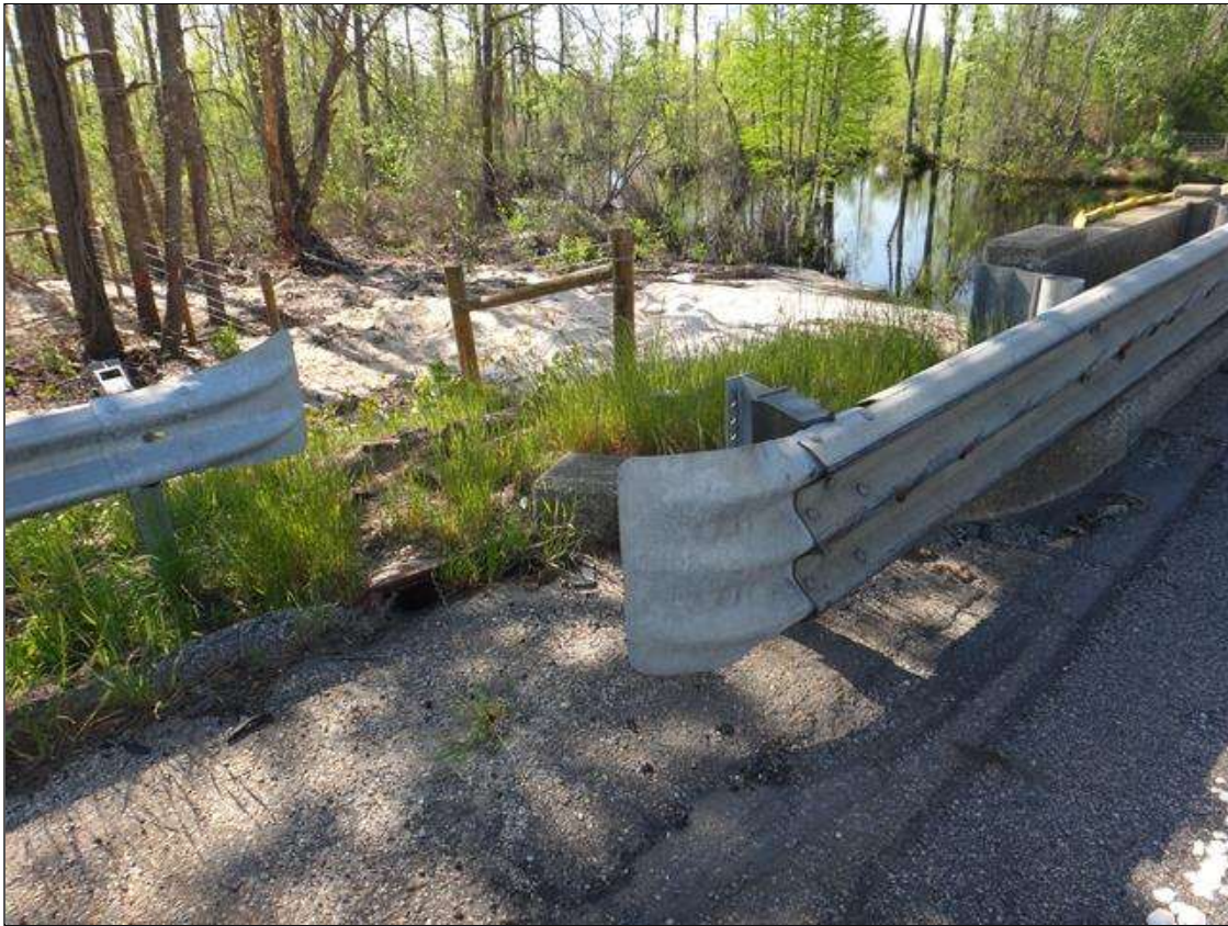
guardrail at Northeast corner [not connected to bridge rail]
