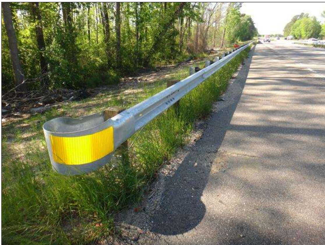
Northeast guardrail and end treatment
