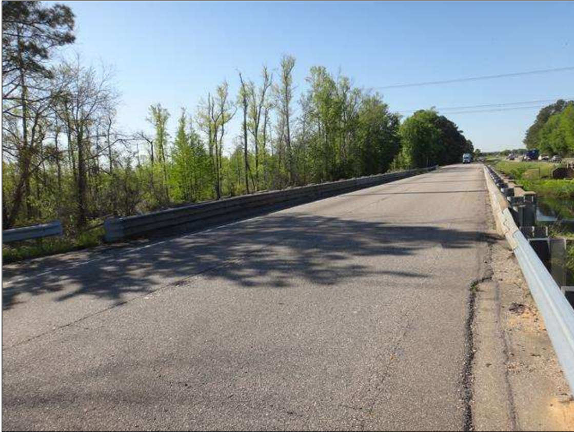
North approach looking South
