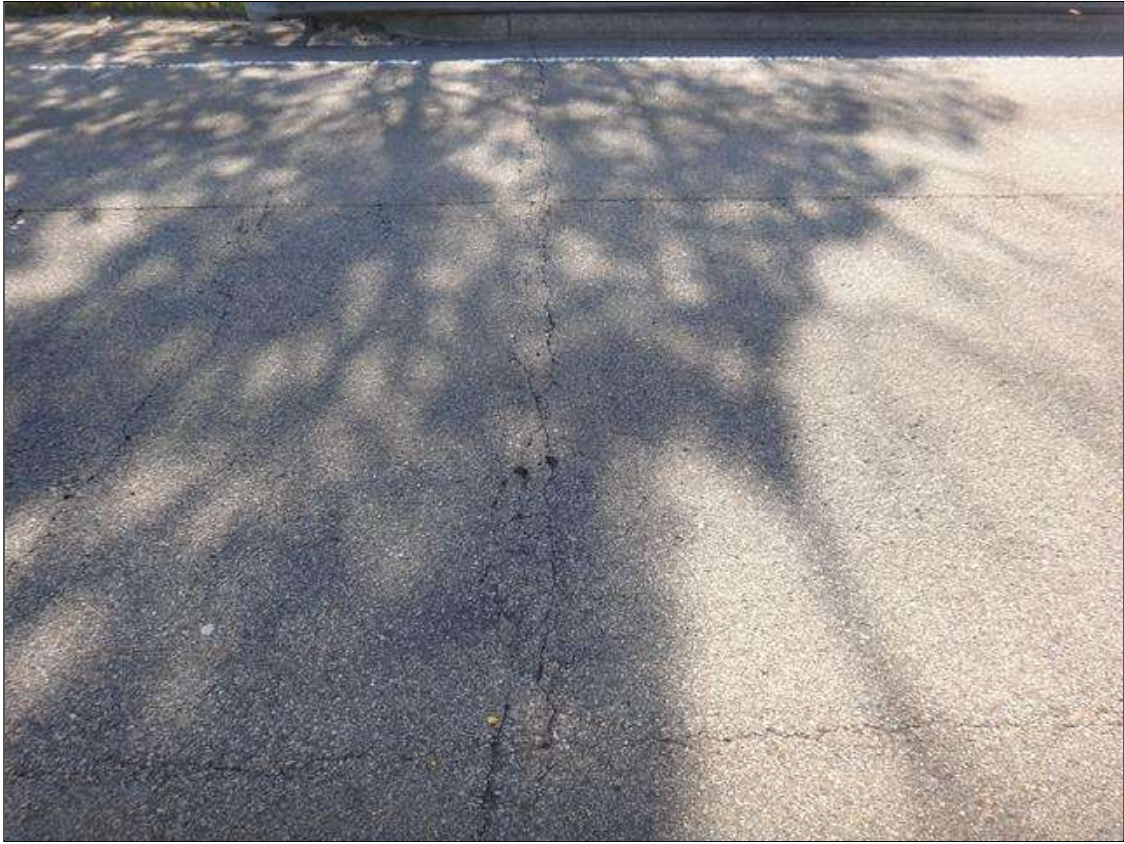
asphalt over end bent 2
