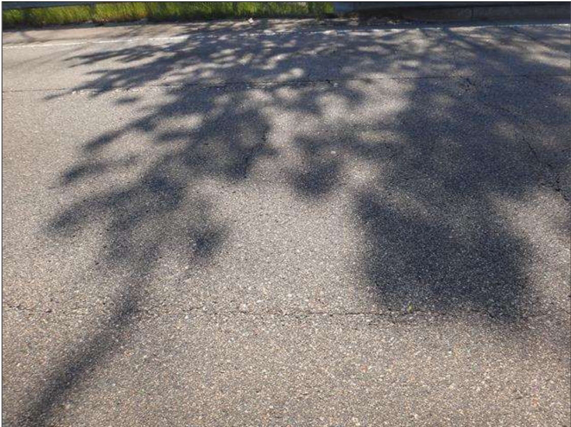
North approach asphalt
