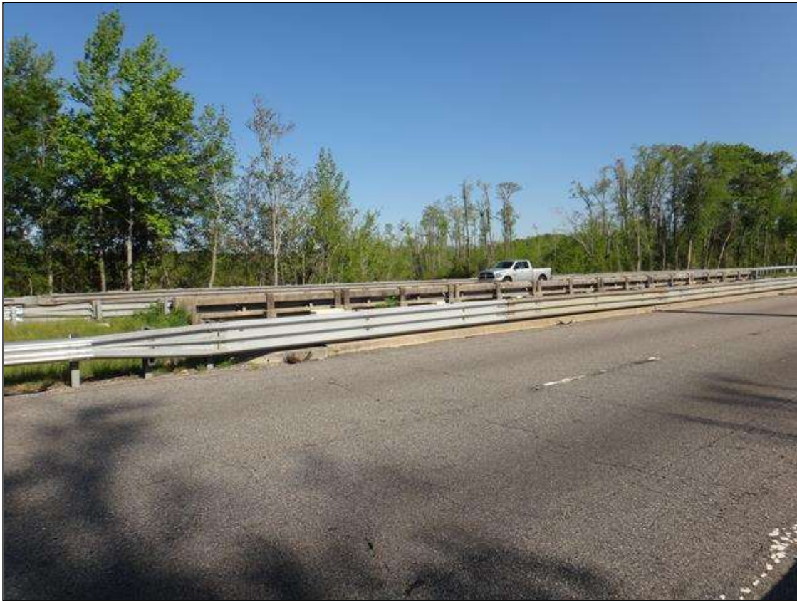
left bridge rail
