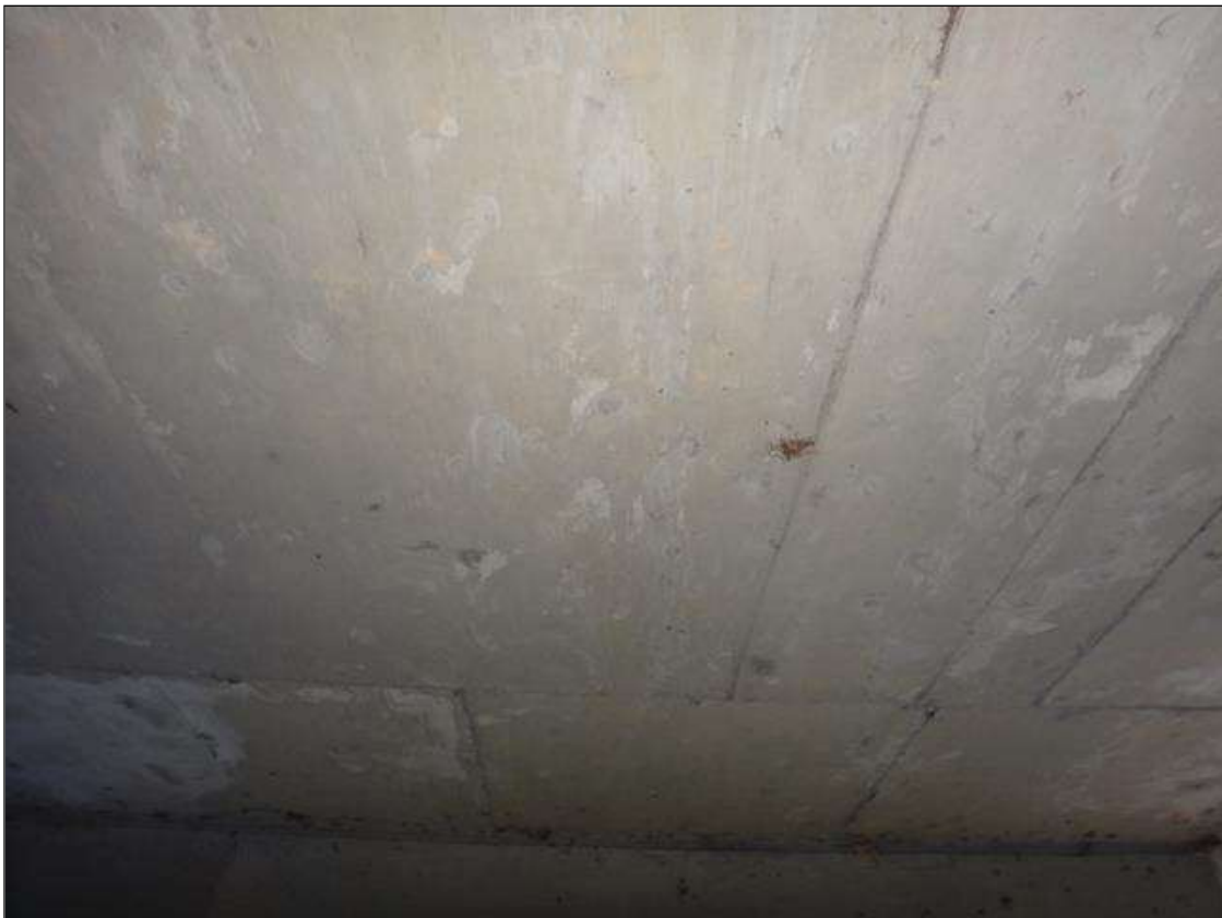
typical underside of deck
