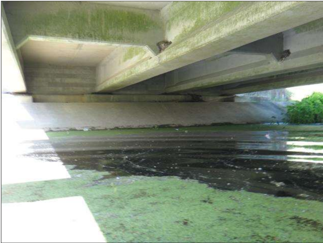
end bent 1 and slope protection
