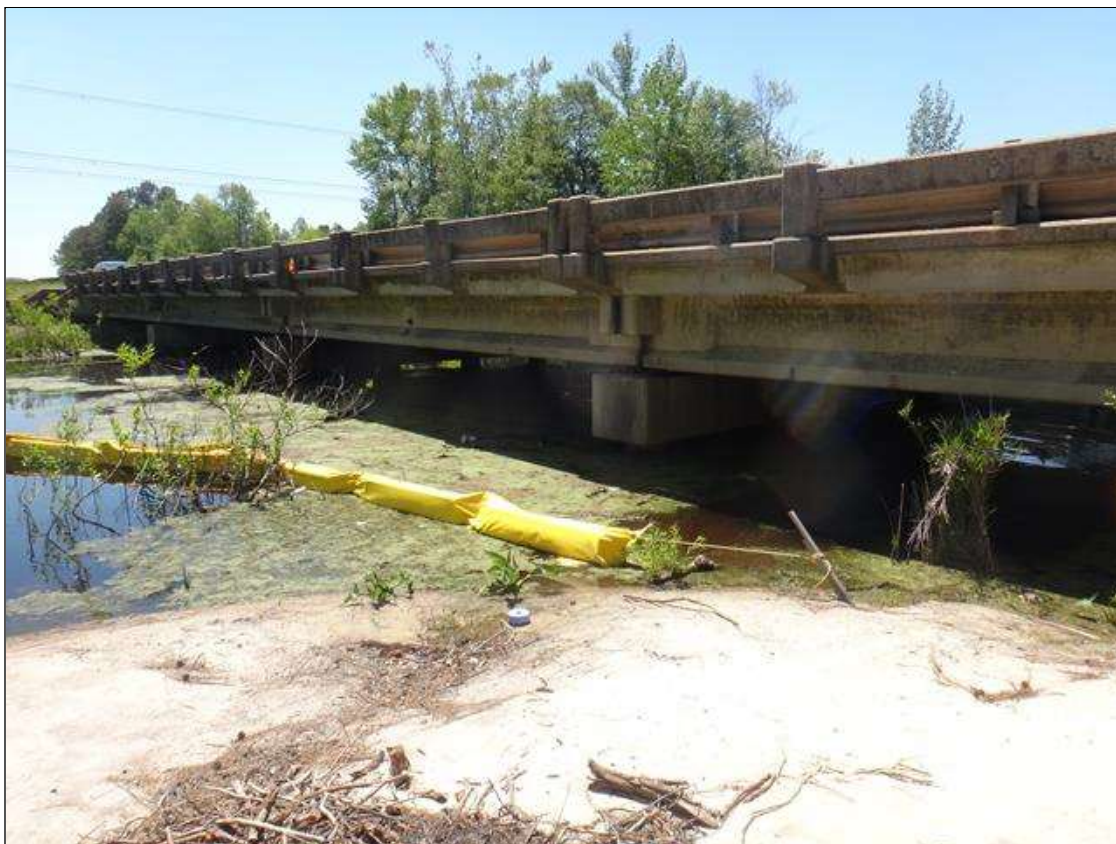
East profile looking West
