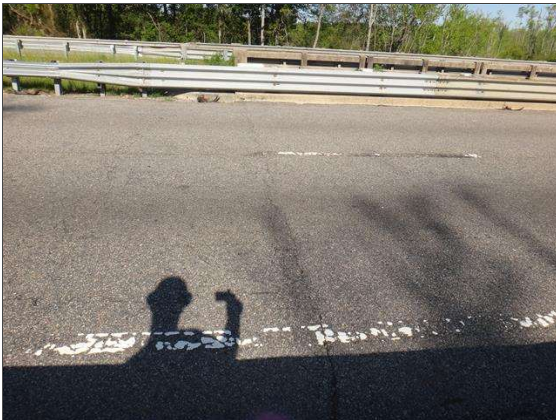
asphalt over end bent 1
