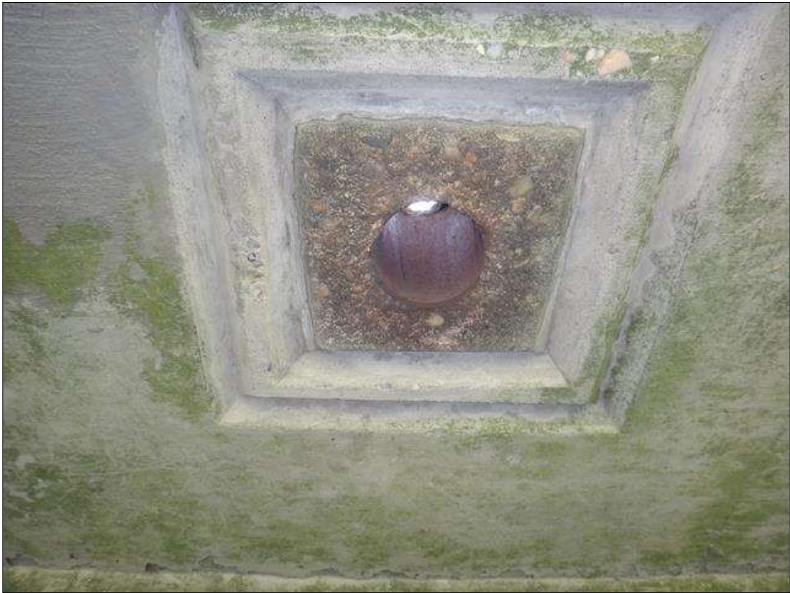
typical deck drain
