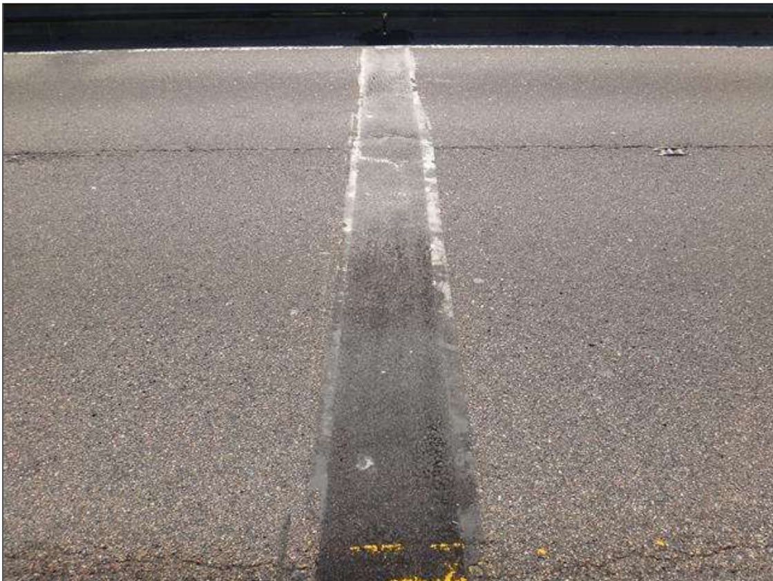
joint over bent 3
