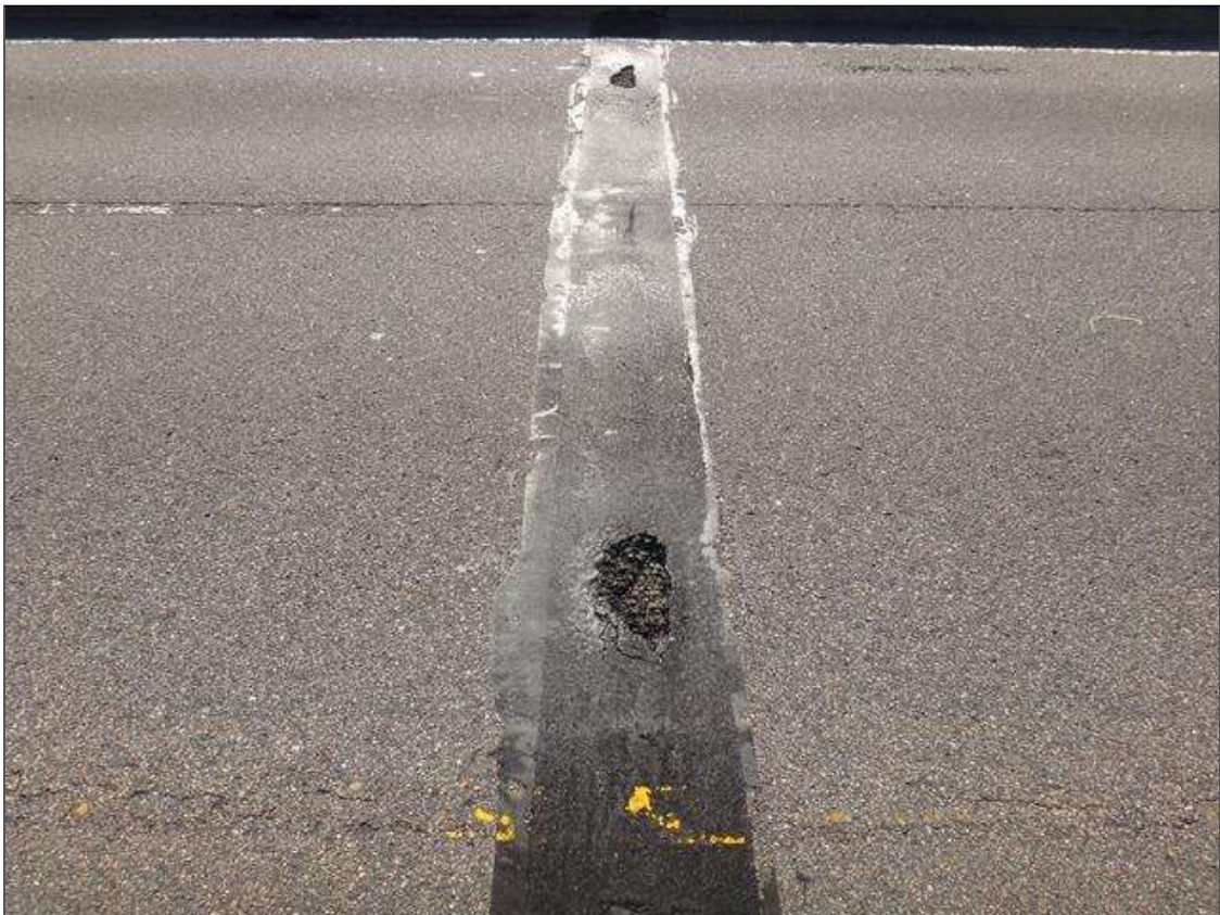
joint over bent 2
