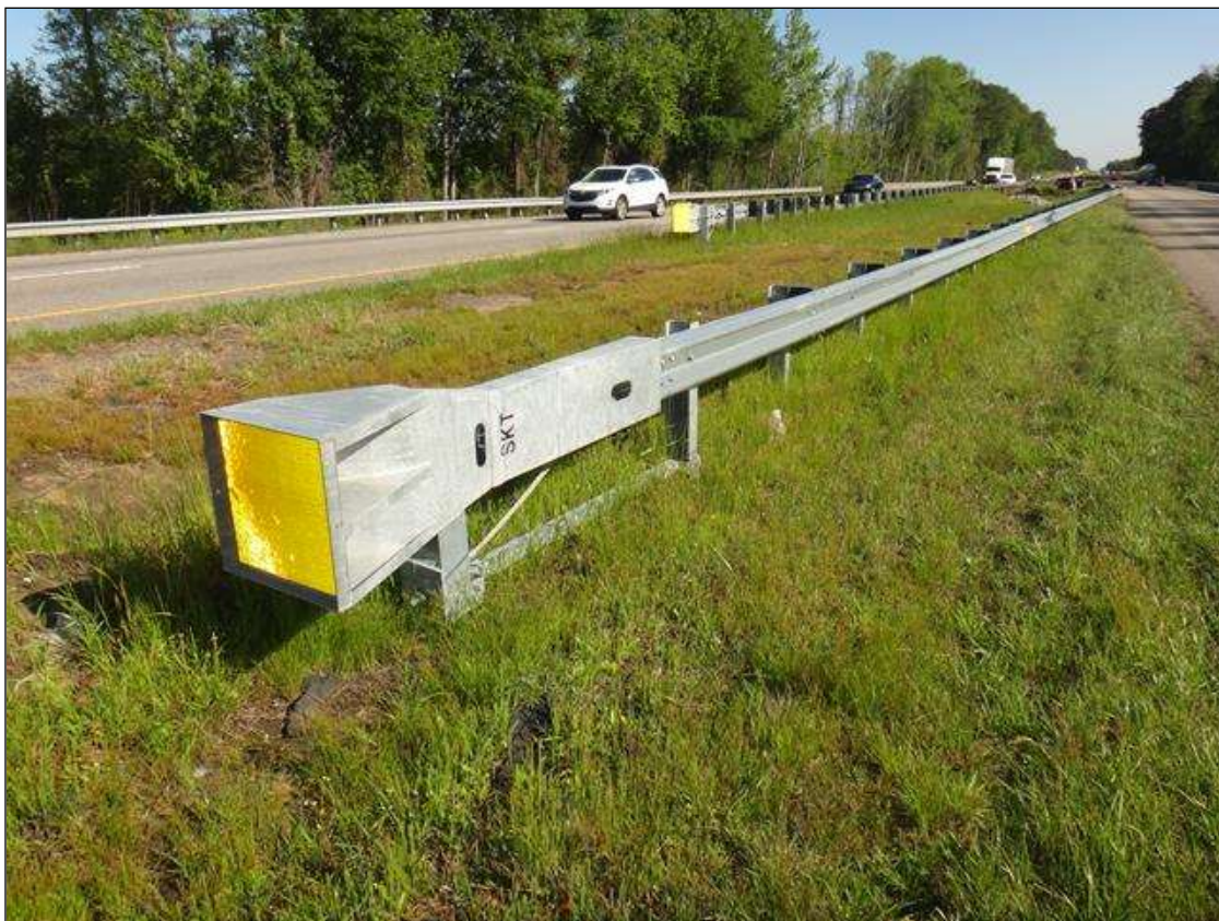
Southwest guardrail and end treatment
