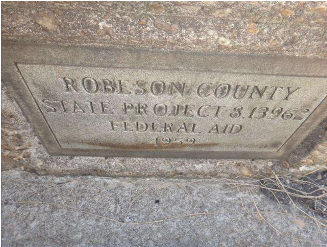
bridge plaque at Southeast corner
