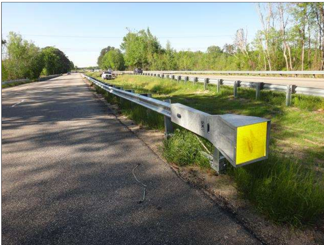
Northwest guardrail and end treatment
