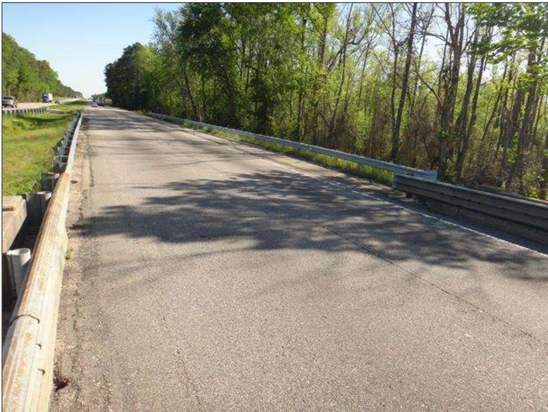
North approach looking North
