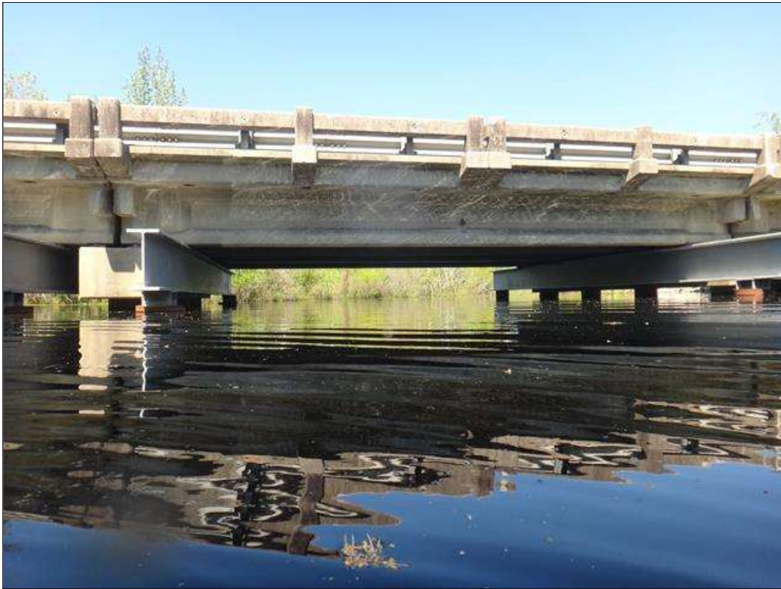
looking upstream [West] from under bridge
