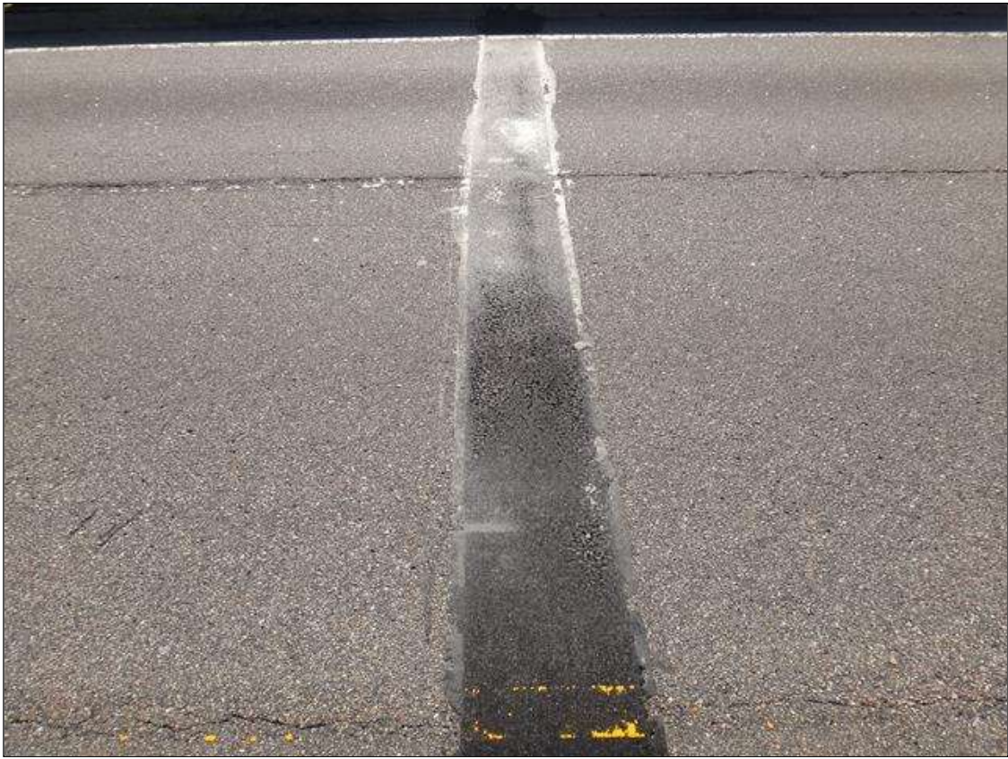
joint over bent 1
