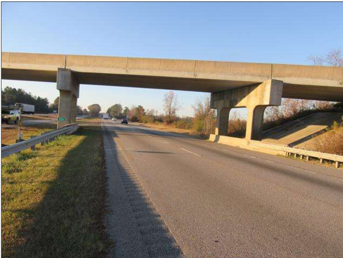
LOOKING SOUTH, SOUTHBOUND LANE THRU SPAN 2
