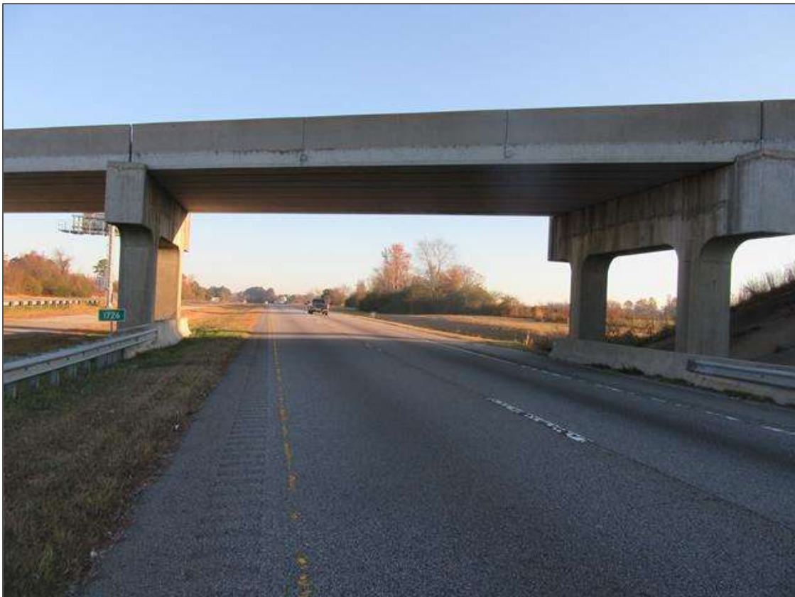
LOOKING NORTH, NORTHBOUND LANE THRU SPAN 4
