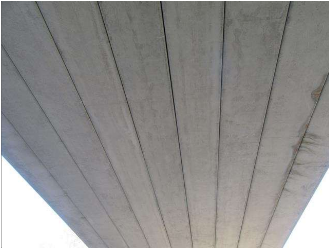
SPAN 2 SUPERSTRUCTURE, ALL SPANS ARE SIMILAR
