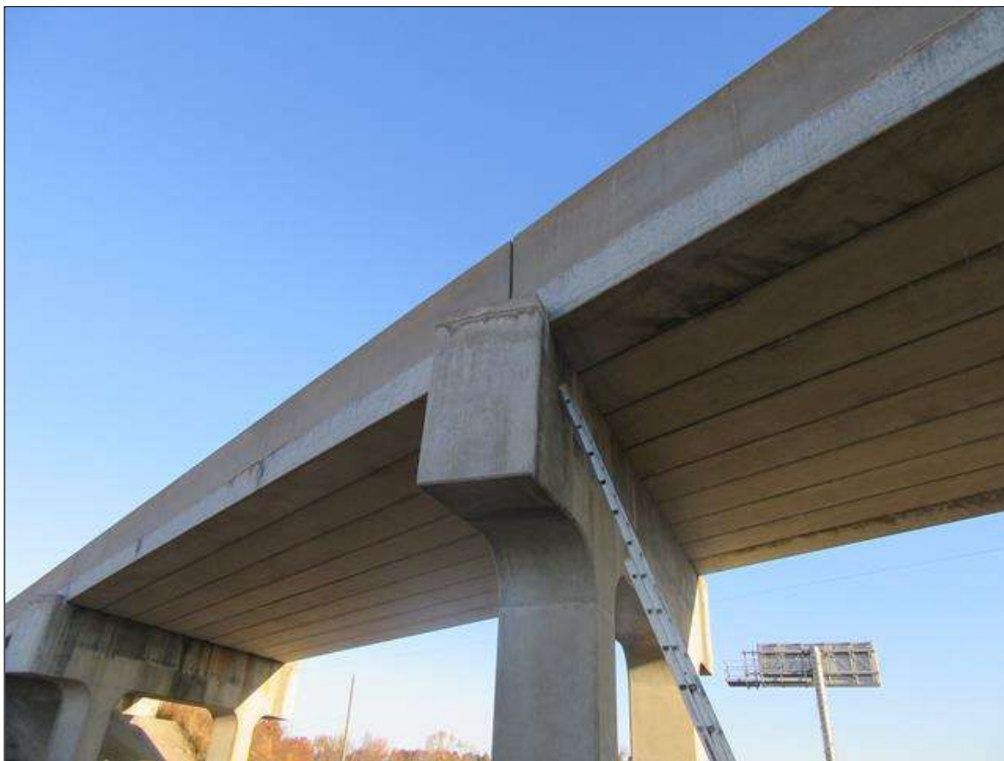
SOUTH END OF BENT 2 CAP, SIMPLE SPANS
