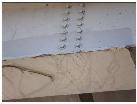
Span 2 Beam 4: BOTTOM FLANGE OF BEAM 4 IN SPAN 2 IS BOWED DOWNWARD 1/4" OVER WEST BOUND THRU LANE.
