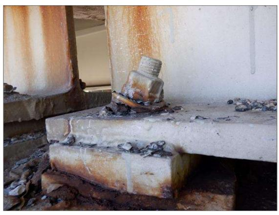
Span 1 Beam 1 Far Bearing: EAST ANCHOR BOLT LEANING TOWARDS SOUTH PAR
