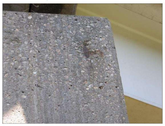
Bent 2 Cap 1: 3" DIAMETER X 1" DEEP SPALL WITH EXPOSED REBAR IN EAST FACE
