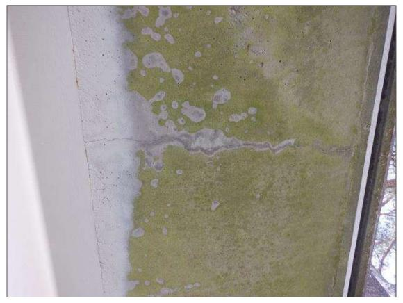
Span 1 Deck: 12 - 2 FT. TRANSVERSE HAIRLINE CRACKS WITH EFFLORESCENCE IN BOTTOM OF DECK WEST OVERHANG
