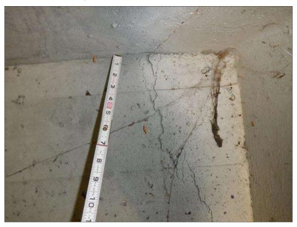
End Bent 1 Abutment/Backwall: 8" X 3" DELAMINATION IN BAY 1
