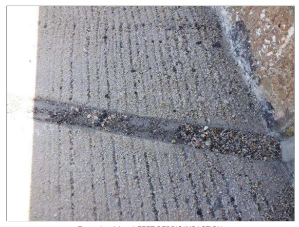
Expansion Joint: 3 FEET DEBRIS IMPACTION
