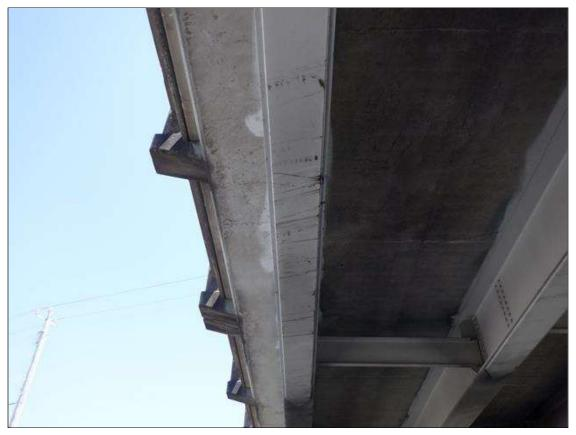
Span 2 Beam 1: 10 FT. OF VEHICLE SCRAPES WITH GOUGES UP TO 3" X 1/2" IN BOTTOM FLANGE AND BOTTOM FLANGE COVER PLATE 25 FT. FROM BENT 2
