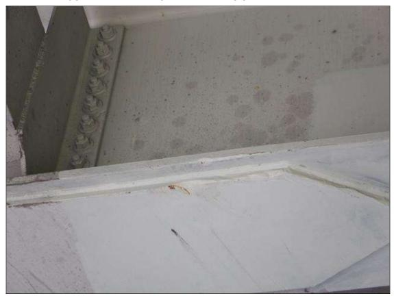
Span 2 Beam 3: BEAM 3 IN SPAN 2 OVER WEST BOUND LANE IS BOWED 1" @ POINT OF IMPACT OF 19FT FROM NORTH END OF BEAM.
