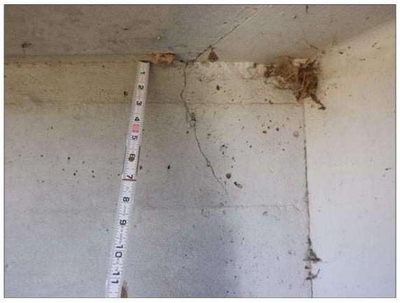
End Bent 2 Abutment/Backwall: 10" X 4" DELAMINATION UNDER WEST OVERHANG
