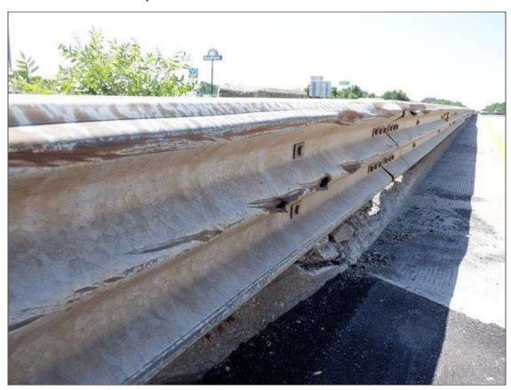
Span 3 Right Bridge Rail: MULTIPLE GOUGES UP TO 6" X 1" IN RAIL
