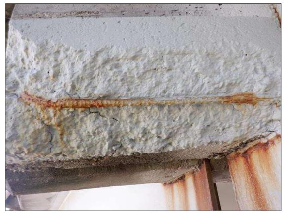
END DIAPHRAGM WEST OVERHANG AT BENT 1: 24" X 8" X 5" DEEP SPALL WITH EXPOSED REBAR IN SOUTH FACE
