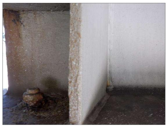
Span 2 Beam 1: 1 FOOT OF PAINTED OVER PITTING UP TO 1/16" DEEP WITH RUST BLEEDING IN WEB AROUND END DIAPHRAGM AND BEARING STIFFENER AT BENT 1
