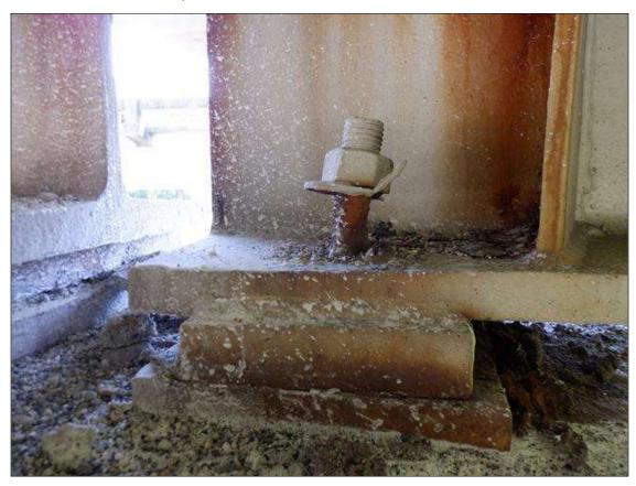
Span 1 Beam 4 Far Bearing: WEST ANCHOR BOLT LEANING TOWARDS SOUTH PAR
