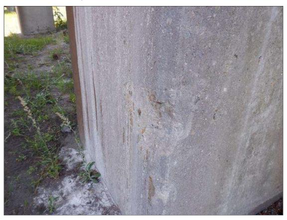
Bent 1 Pile 1: 8" DIAMETER X 1" DEEP SPALL IN NORTHWEST CORNER
