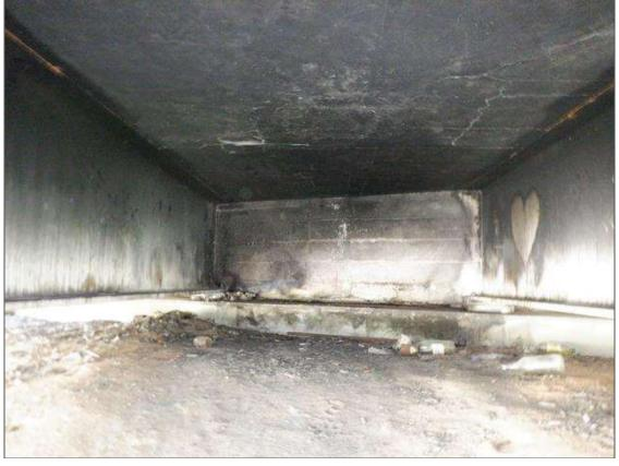
FIRE DAMAGE IN BAY 2 ABUTMENT 2
