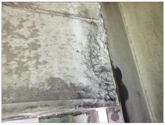
END DIAPHRAGM BAY 2 AT BENT 2: 12" X 4" X 1" DEEP SPALL IN NORTH FACE
