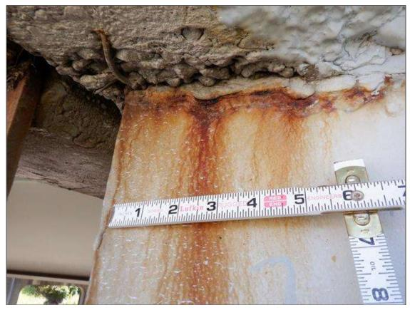
Span 1 Beam 1: 1 FOOT OF CORROSION WITH 11/16" REMAINING SECTION IN WEB AROUND END DIAPHRAGM AT BENT 1 PAR
