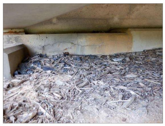
End Bent 2 Cap 1: 2 S.F. OF VERTICAL AND HORIZONTAL CRACKS UP TO 1/16" WIDE UNDER BAY 1
