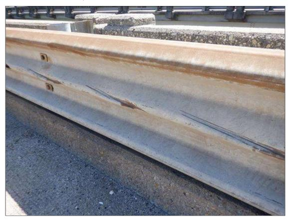
Span 2 Right Bridge Rail: MULTIPLE GOUGES UP TO 6" X 1" IN RAIL
