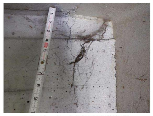
End Bent 1 Abutment/Backwall : 12" X 3" DELAMINATION IN BAY 3
