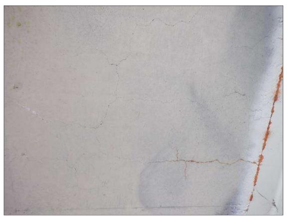
Span 1 Deck: 500 SF. OF TRANSVERSE AND LONGITUDINAL CRACKS UP TO 1/16" WIDE WITH EFFLORESCENCE IN BOTTOM OF DECK
