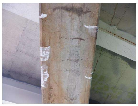
Bent 1 Cap 1: 6 - 24" LONGITUDINAL HAIRLINE CRACKS WITH EFFLORESCENCE IN BOTTOM OF CAP BETWEEN COLUMNS 1 AND 2
