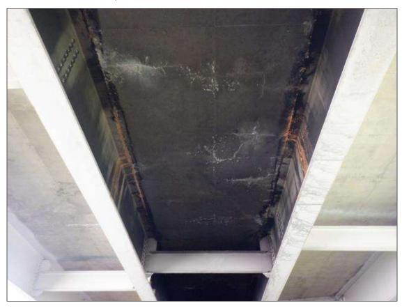
FIRE DAMAGE IN SPAN 3 BAY 2 BOTTOM OF DECK
