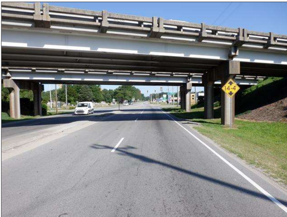
SPAN 2 WEST BOUND THRU LANE
