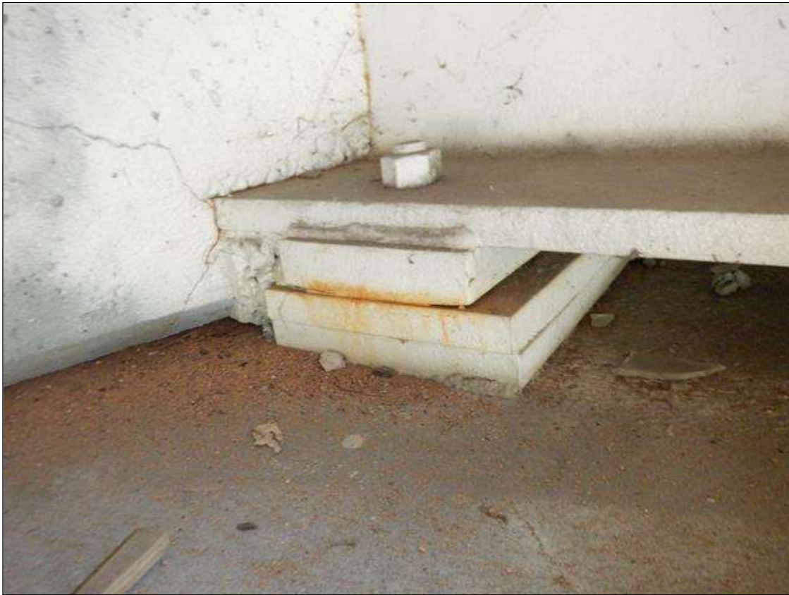
ABUTMENT 1 BEAM 3 BEARING
