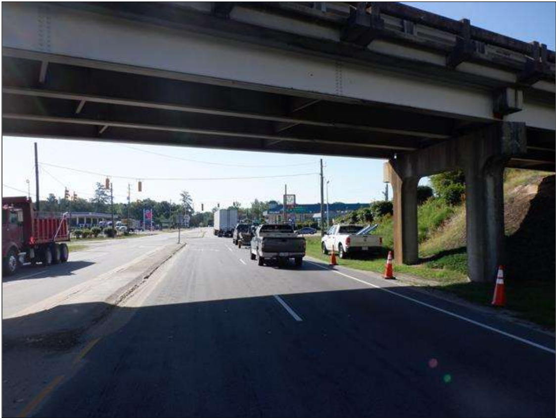
SPAN 2 EAST BOUND THRU LANE
