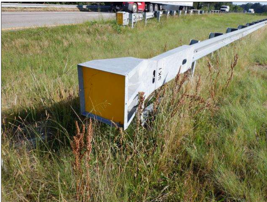
SOUTHWEST GUARDRAIL END TERMINAL
