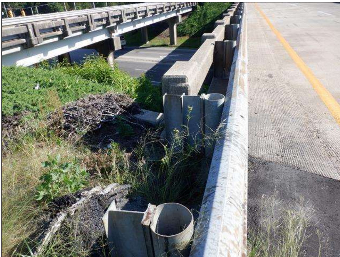
SW GUARDRAIL TRANSITION
