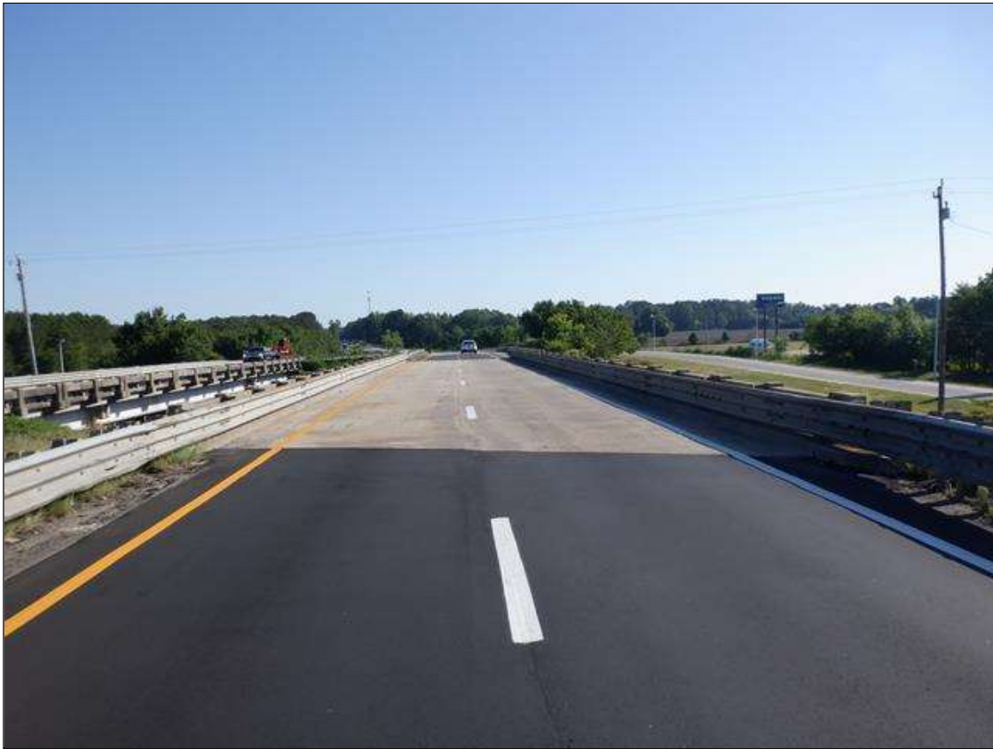
COVER SHEET PHOTO LOOKING NORTH
