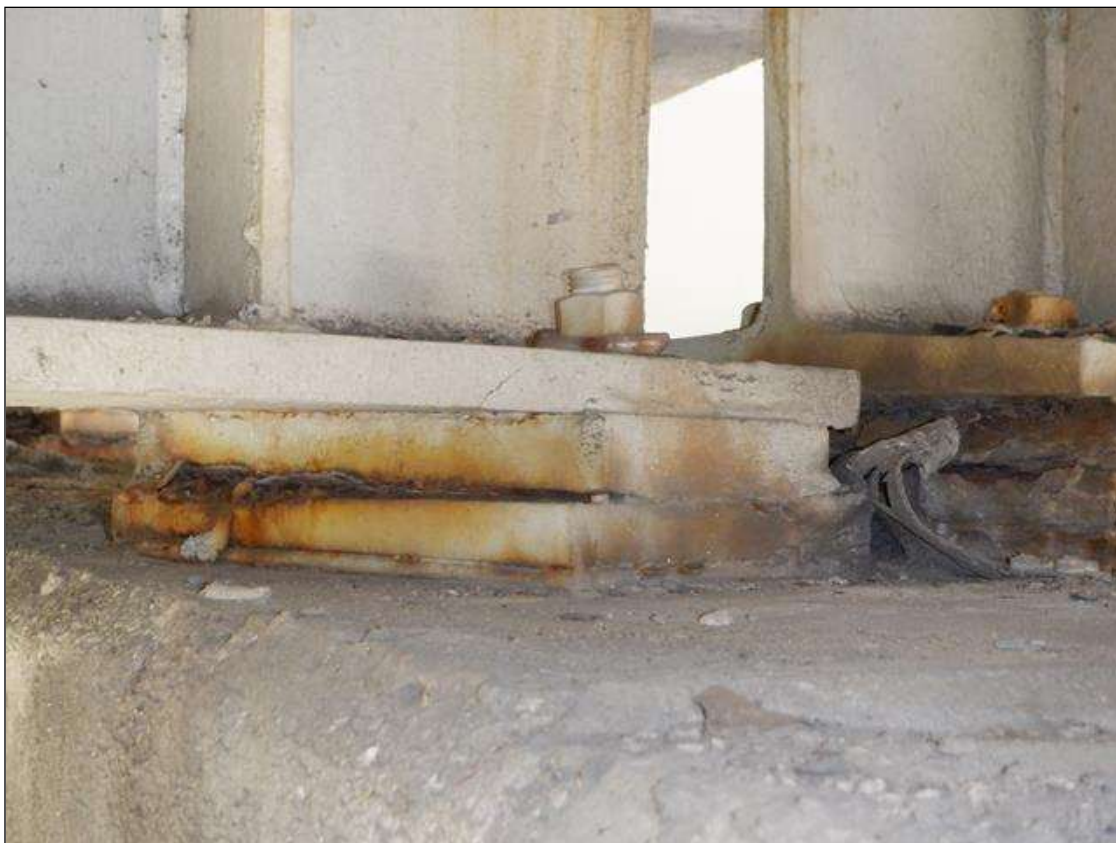
BENT 1 BEAM 3 BEARING
