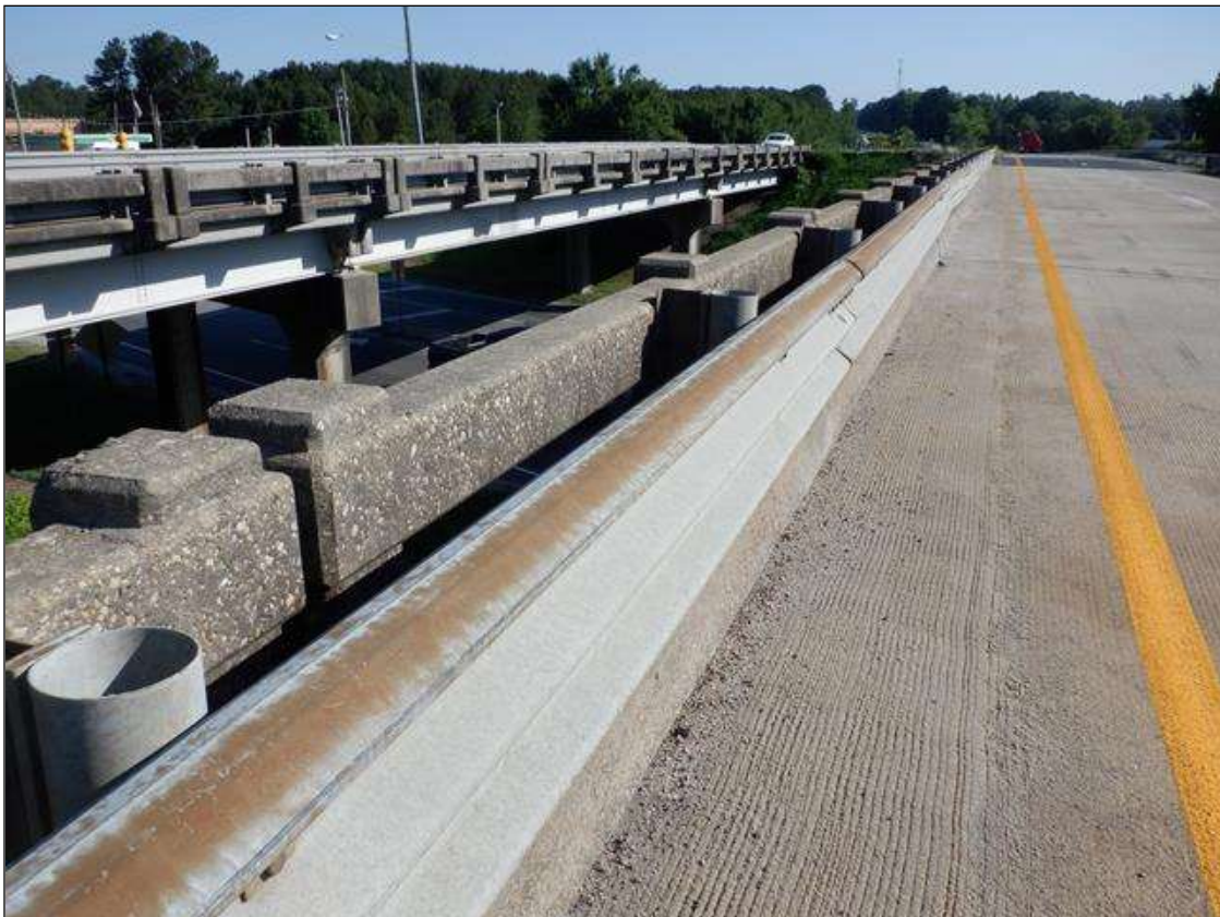
LEFT RAIL RIGHT RAIL SIMILAR
