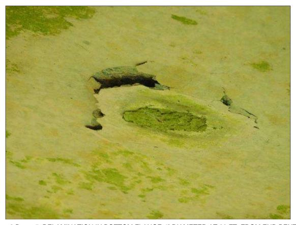
Span 3 Beam 5: DELAMINATION IN BOTTOM FLANGE 4" DIAMETER AT 20 FT. FROM END BENT 2
