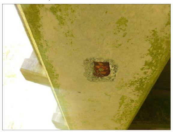
Span 3 Beam 1: 4" DIAMETER X 1/2" DEEP SPALL WITH EXPOSED PLATE AT HOLD-DOWN POINT IN BOTTOM FLANGE
