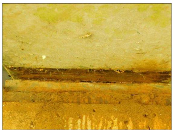
Span 1 Beam 2 Far Bearing: RUST WITH FLAKING, NO SECTION LOSS
