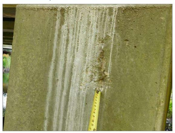
Bent 1 Cap 1: SURFACE SPALL 6" DIAMETER X 1" DEEP ON WEST END
