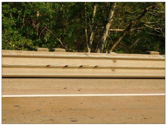
Span 1 Left Bridge Rail: MULTIPLE GOUGES UP TO 3" X 1" IN RAIL
