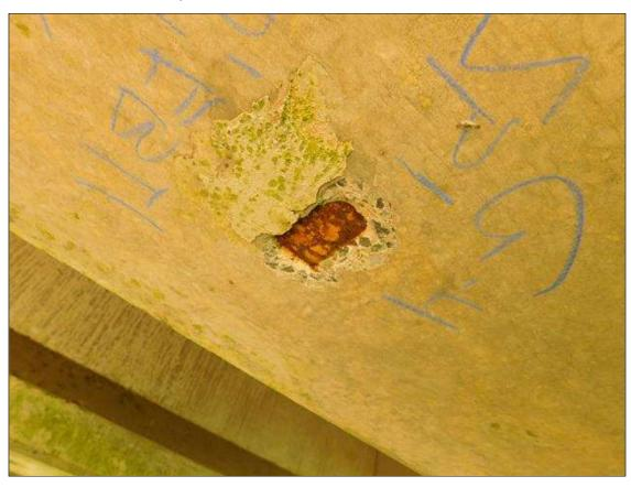
Span 1 Beam 4: SURFACE SPALL 4" DIAMETER X 1/2" DEEP IN BOTTOM FLANGE AT 20 FT. FROM END BENT 1 CAP
