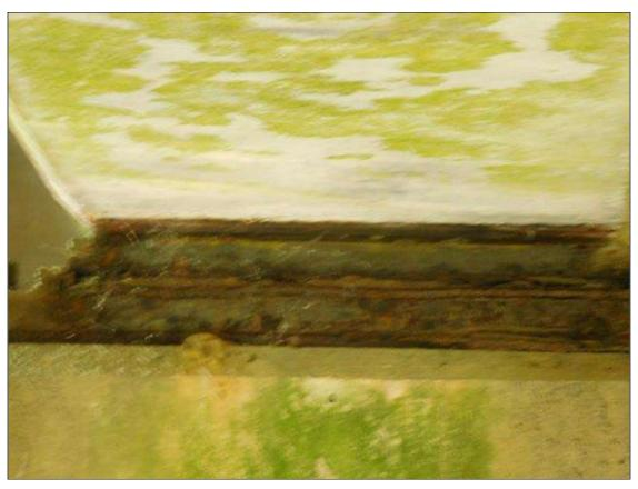
Span 3 Beam 4 Near Bearing: SURFACE CORROSION
