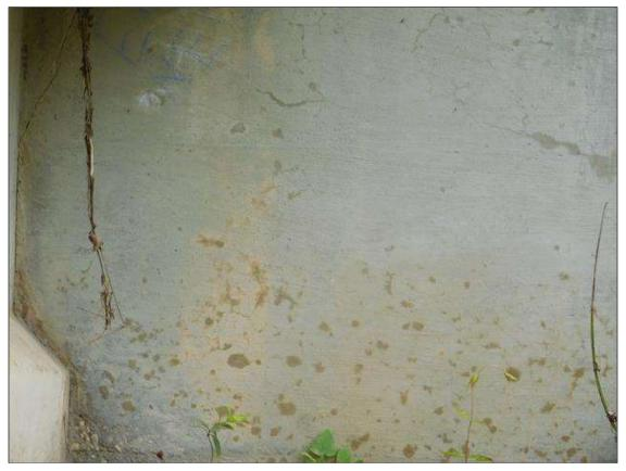
End Bent 2 Abutment/Backwall : 6 SF. OF HAIRLINE MAP CRACKING AT EAST END
