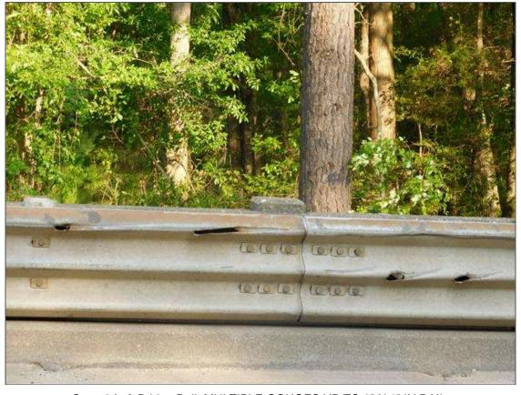
Span 3 Left Bridge Rail: MULTIPLE GOUGES UP TO 8" X 1" IN RAIL
