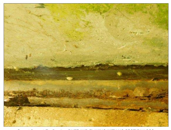
Span 1 Beam 1 Far Bearing: RUST AND FLAKING WITH NO SECTION LOSS
