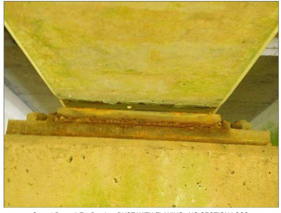
Span 1 Beam 3 Far Bearing: RUST WITH FLAKING, NO SECTION LOSS
