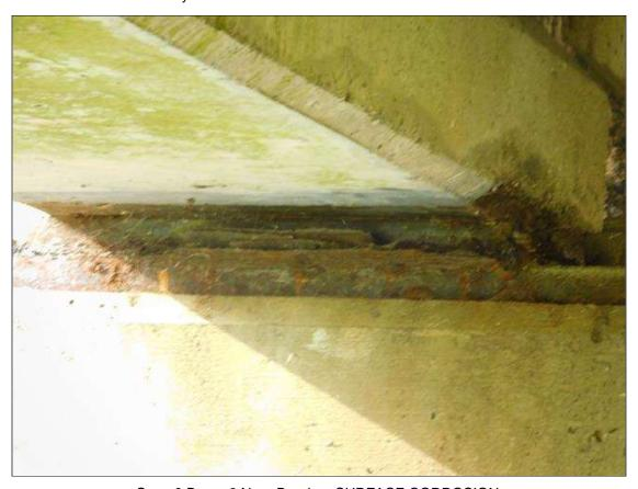
Span 3 Beam 6 Near Bearing: SURFACE CORROSION
