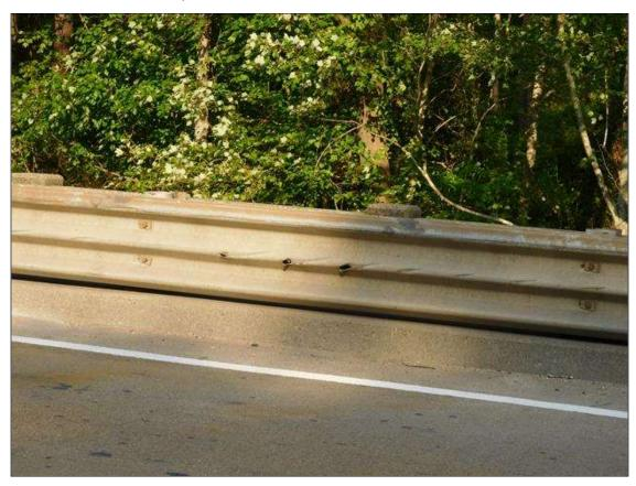
Span 2 Left Bridge Rail: MULTIPLE GOUGES UP TO 3" X 1" IN RAIL
