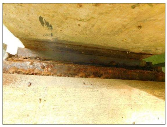
Span 3 Beam 6 Near Bearing: RUST AND FLAKING WITH NO SECTION LOSS
