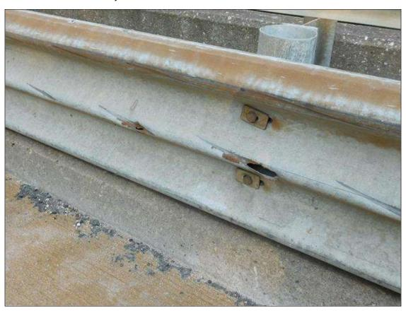
Span 1 Left Bridge Rail: MULTIPLE GOUGES UP TO 6" X 3" IN RAIL
