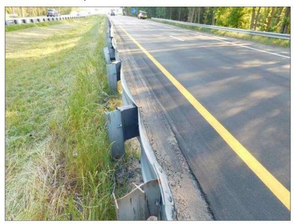
DAMAGED GUARDRAIL (40 FT.) IN NORTH WEST CORNER
