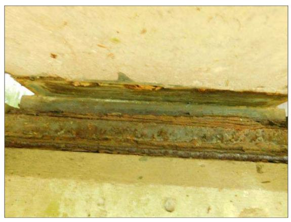
Span 3 Beam 2 Near Bearing: RUST AND FLAKING WITH NO SECTION LOSS
