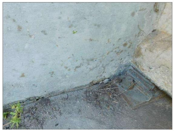
End Bent 2 Abutment/Backwall : HAIRLINE MAP CRACKING AT WEST END , SIMILAR THROUGHOUT ABUTMENT IN ALL BAYS
