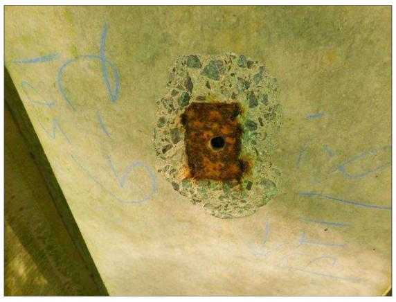
Span 1 Beam 2: 4" DIAMETER X 1/2" DEEP SPALL WITH EXPOSED PLATE AT HOLD-DOWN POINT IN BOTTOM FLANGE
