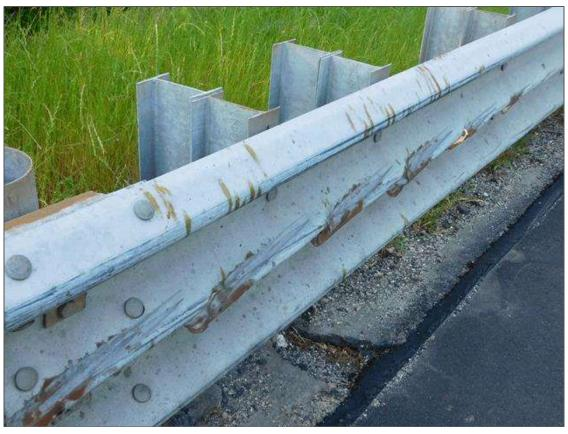
DAMAGED GUARDRAIL AT SOUTHEAST CORNER 20 FT.
