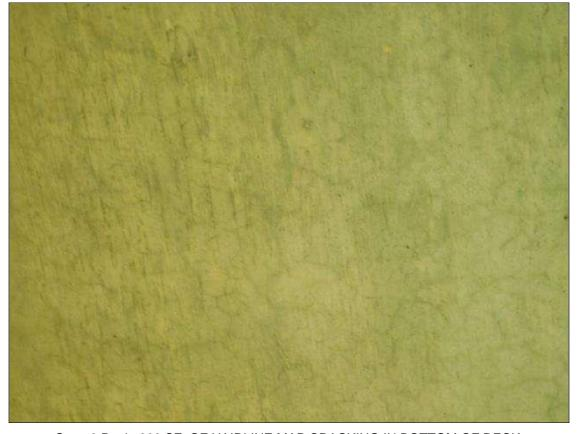
Span 3 Deck: 300 SF. OF HAIRLINE MAP CRACKING IN BOTTOM OF DECK
