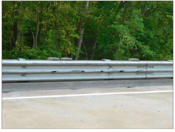
Span 3 Right Bridge Rail: IMPACT GOUGES IN STEEL RAIL
