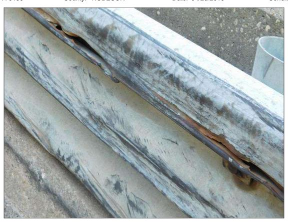
Span 3 Left Bridge Rail: MULTIPLE GOUGES UP TO 12" X 1" IN RAIL
