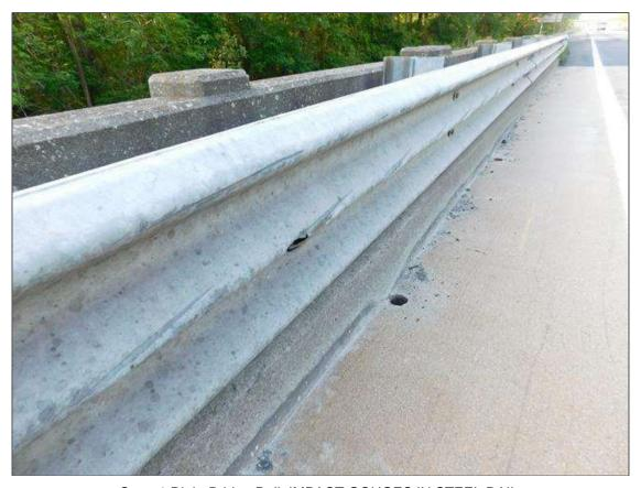
Span 1 Right Bridge Rail: IMPACT GOUGES IN STEEL RAIL
