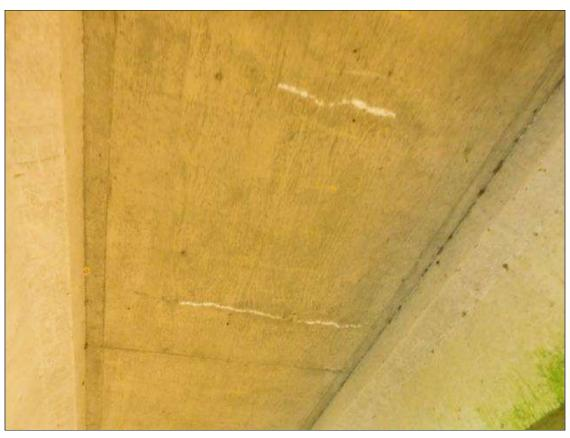
Span 3 Deck: 24" AND 12" TRANSVERSE HAIRLINE CRACKS WITH EFFLORESCENCE IN BOTTOM OF DECK BAY 3, 10 FT. FROM BENT 2
