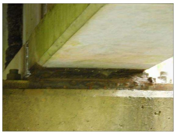
Span 1 Beam 6 Far Bearing: RUST AND FLAKING WITH NO SECTION LOSS
