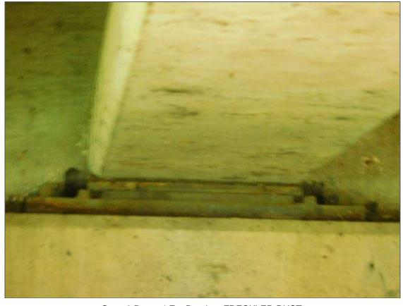
Span 3 Beam 4 Far Bearing: FRECKLED RUST
