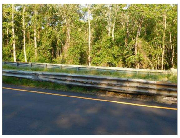
DAMAGED GUARDRAIL AT SOUTHWEST CORNER 20 FT.
