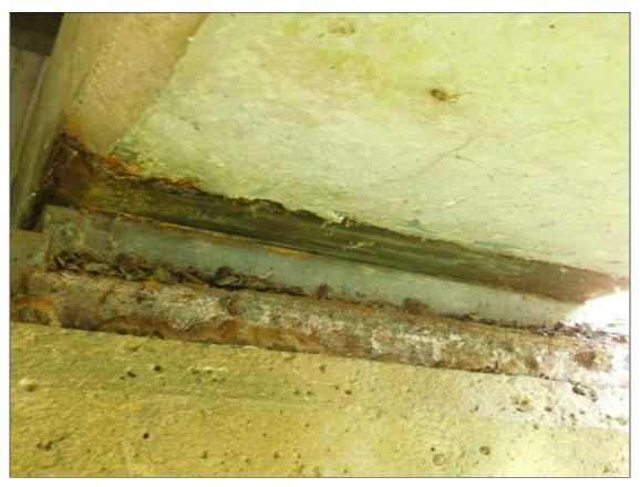
Span 2 Beam 1 Near Bearing: 1/8" OF PACK RUST
