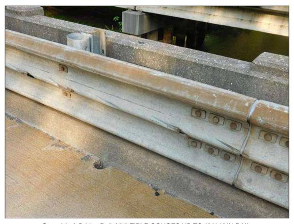
Span 2 Left Bridge Rail: MULTIPLE GOUGES UP TO 6" X 3" IN RAIL
