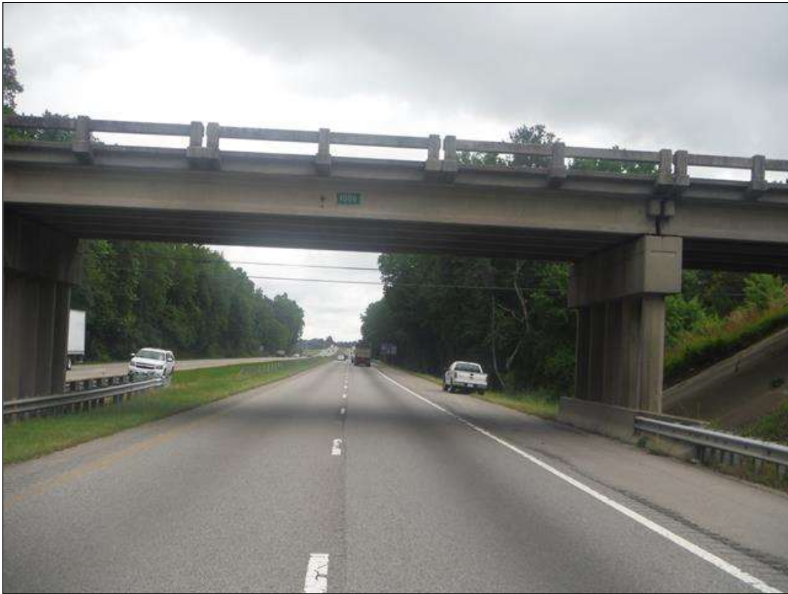
SPAN 3 UNDERCLEARANCE LOOKING NORTH
