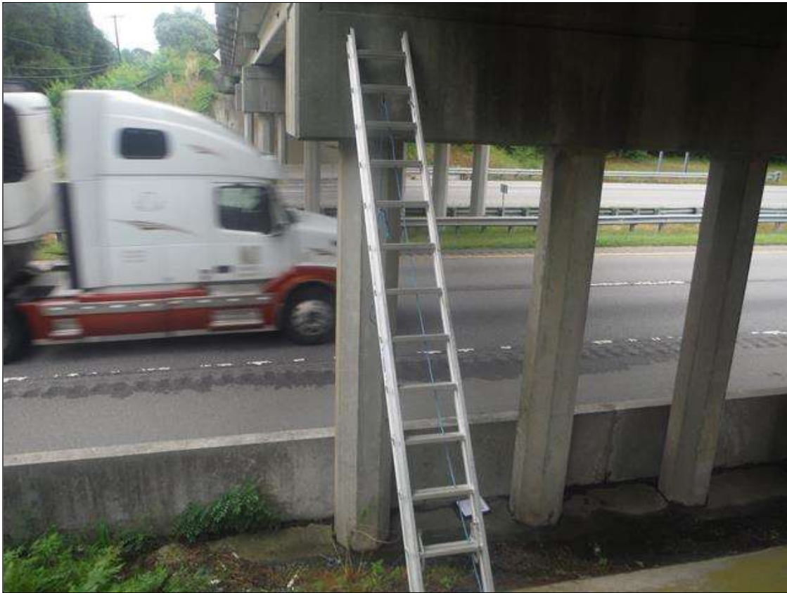
LADDER USED DURING INSPECTION
