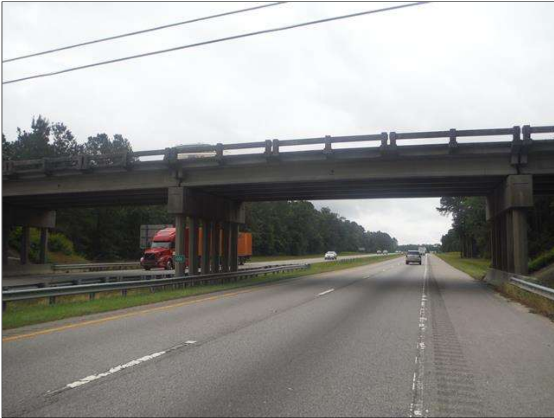
SPAN 2 UNDERCLEARANCE LOOKING SOUTH
