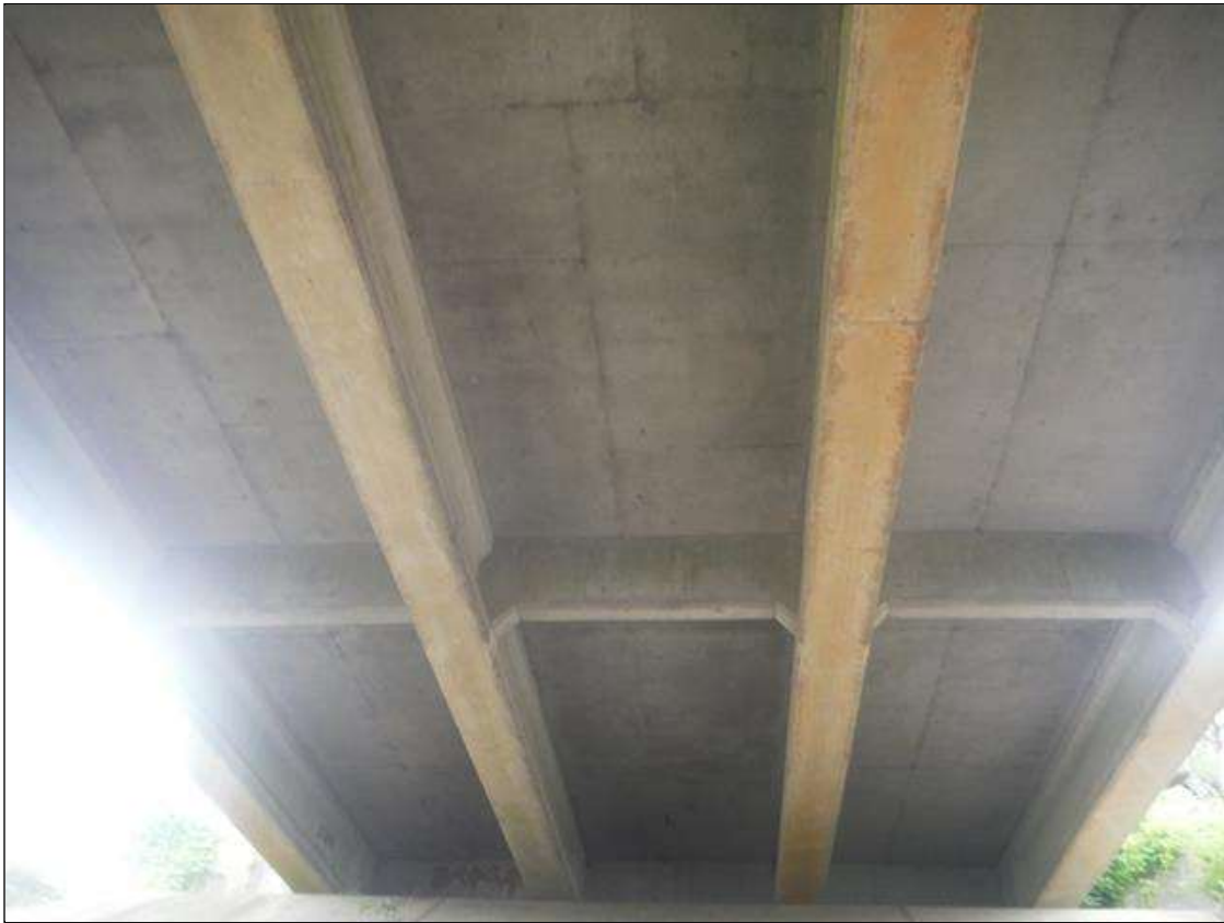
SPAN 4 SUPERSTRUCTURE, SPAN 1 SIMILAR
