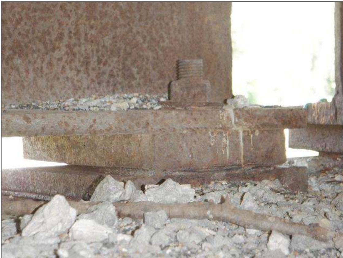
BENT 4 BEAM 1 BEARING
