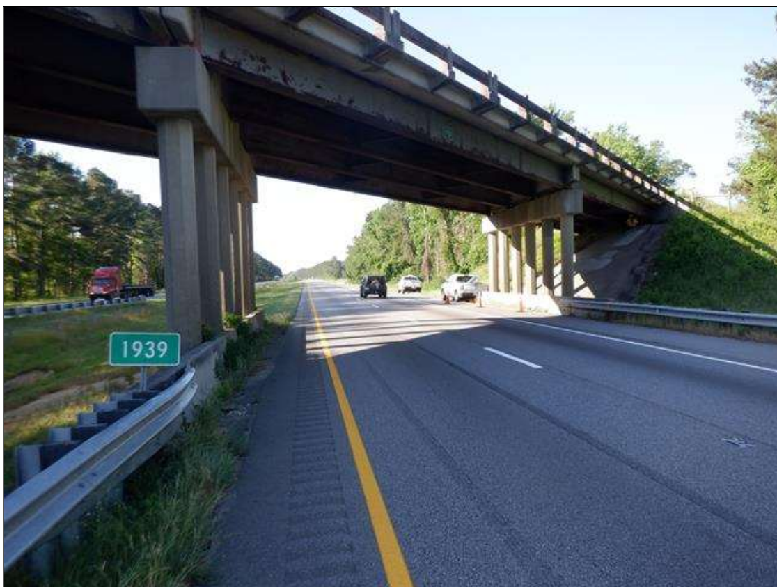
SPAN 2 THRU LANES LOOKING SOUTH
