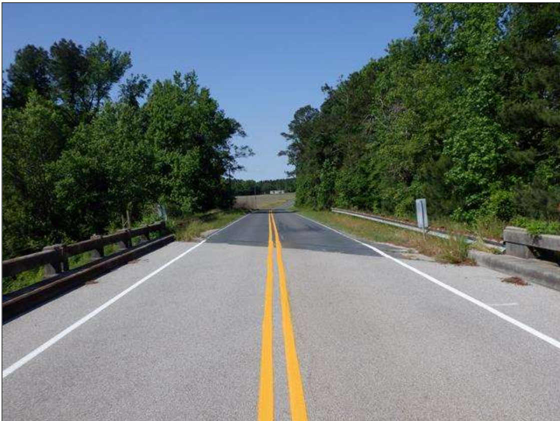
WEST APPROACH LOOKING WEST
