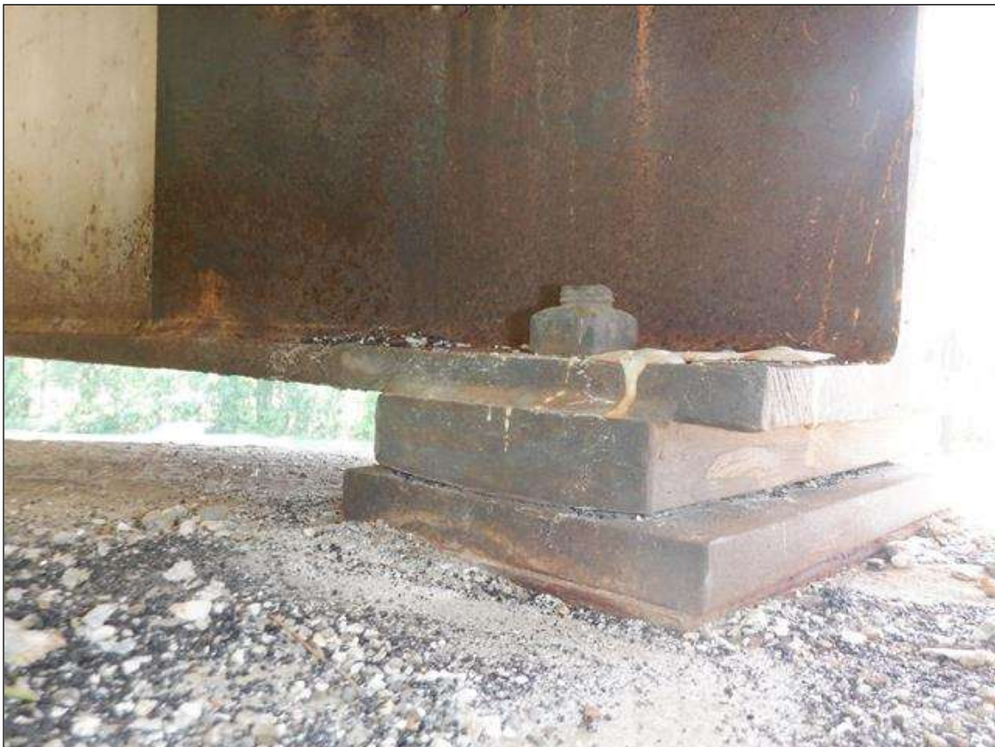
BENT 1 BEAM 4 BEARING
