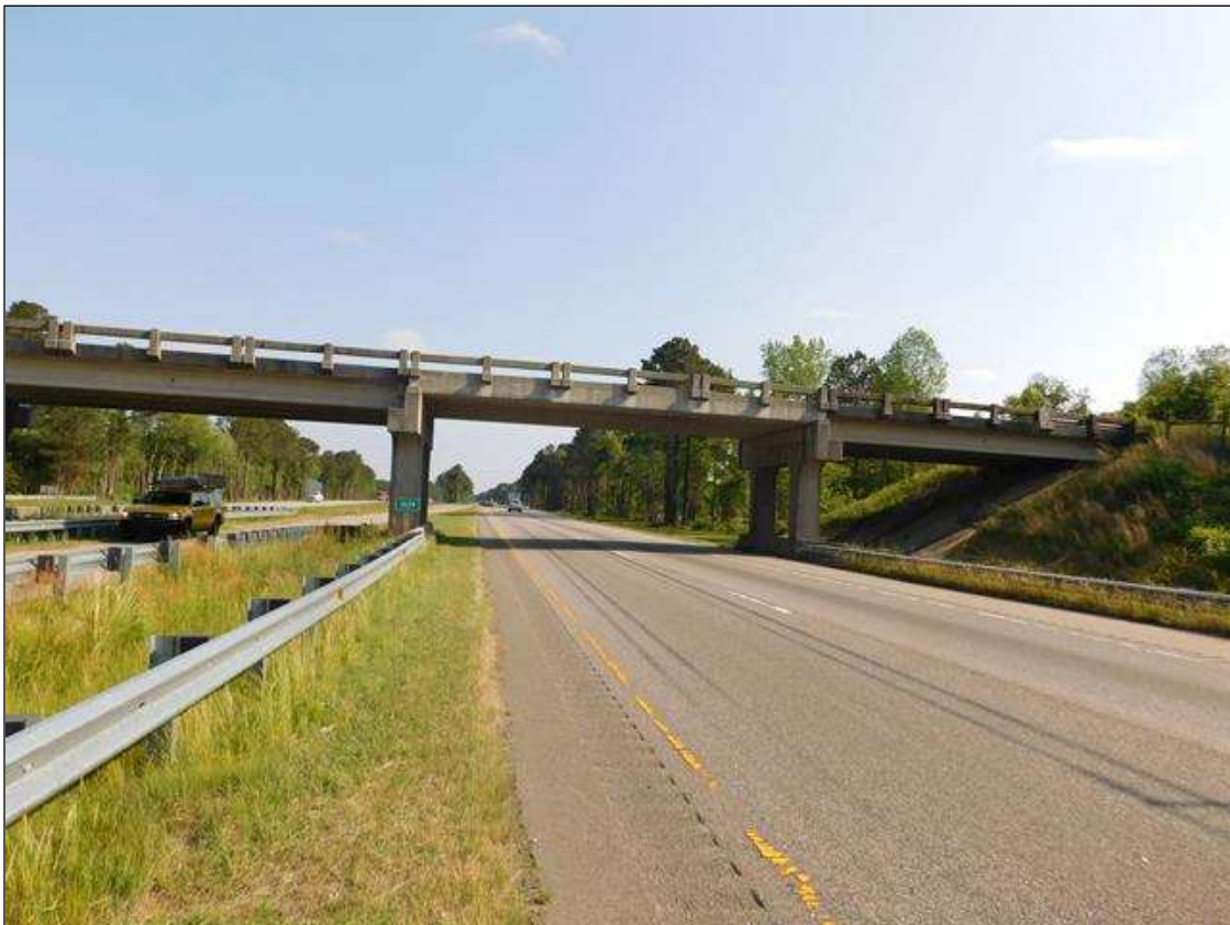
LOOKING NORTH, NORTHBOUND LANE I-95 THRU SPAN 4
