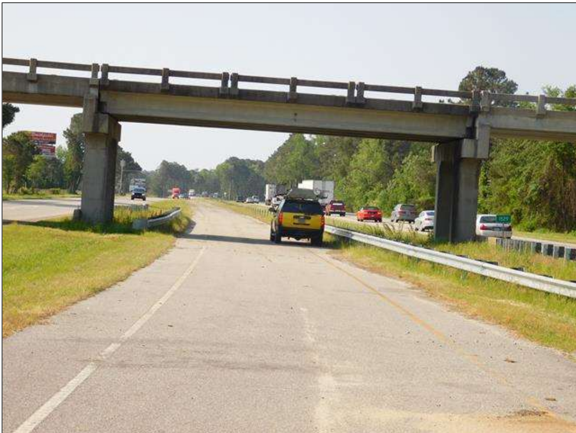
LOOKING SOUTH, SERVICE ROAD THRU SPAN 3
