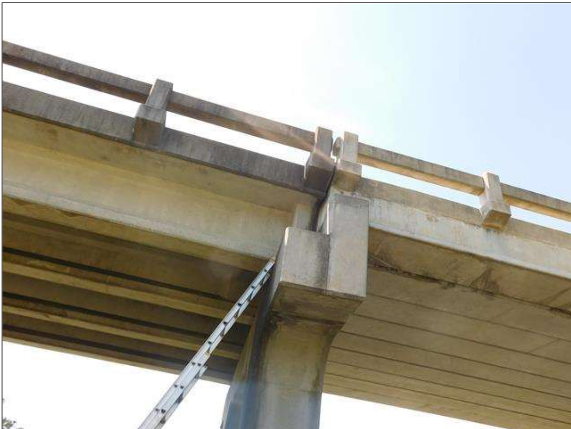
NORTH END OF BENT 2 CAP, SIMPLE SPANS
