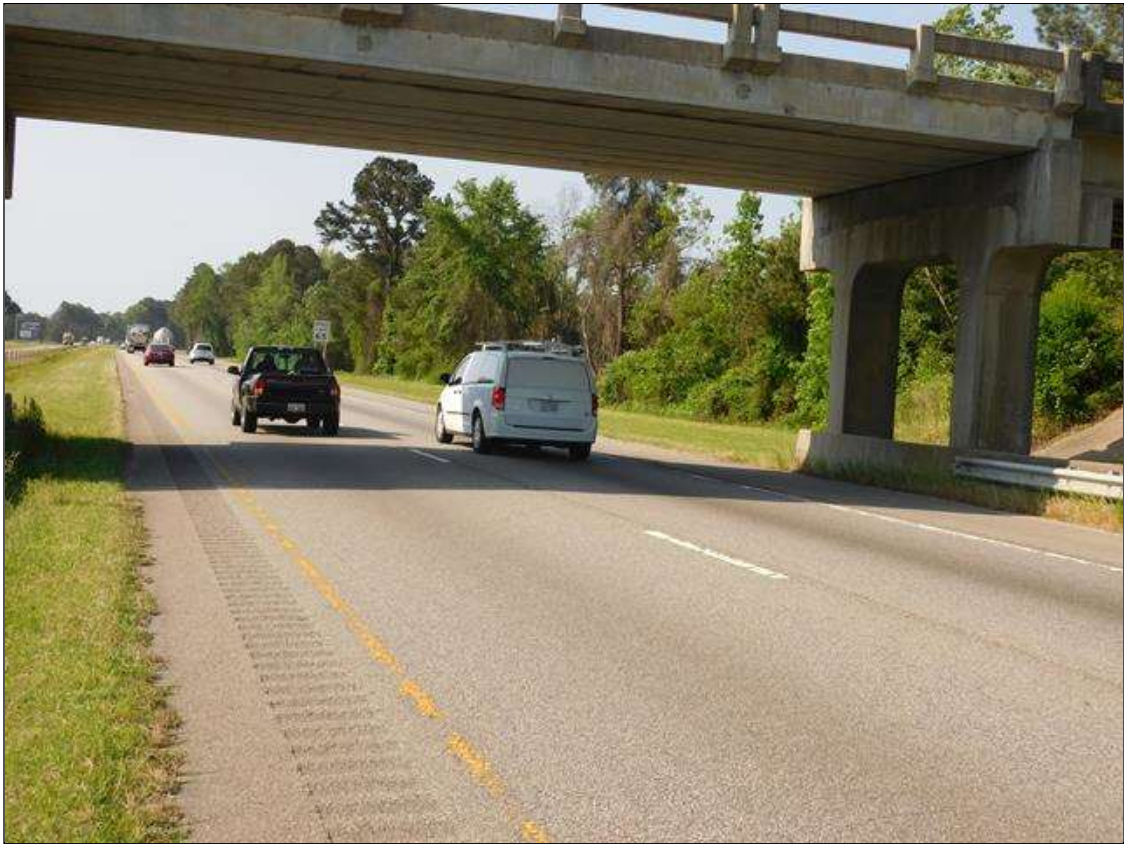
LOOKING SOUTH, SOUTHBOUND LANE I-95 THRU SPAN 2
