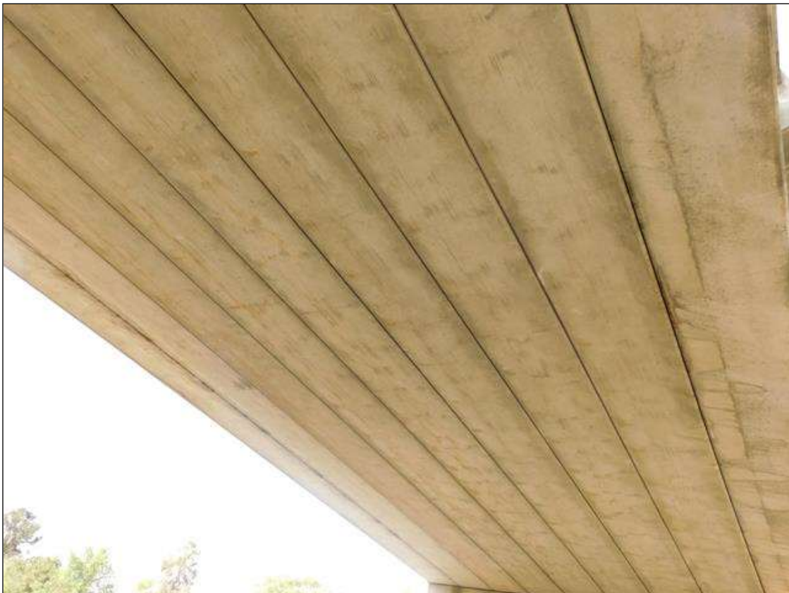
SPAN 4 SUPERSTRUCTURE, SPAN 2 IS SIMILAR
