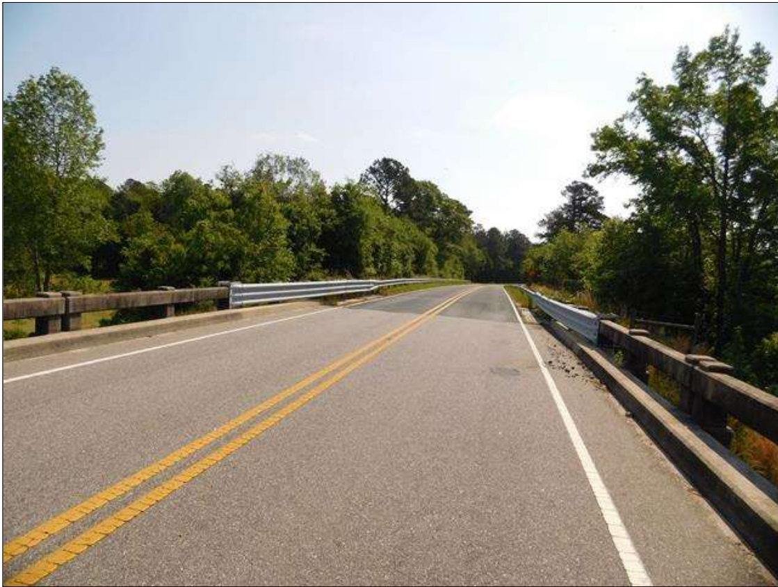
LOOKING EAST, OFF BRIDGE
