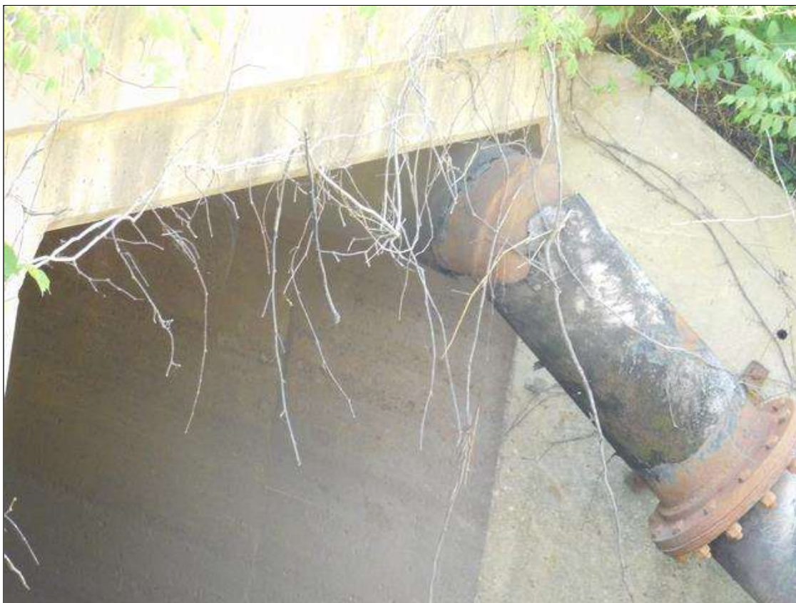
12" CAST UTILITY PIPE ALONG SOUTH WALL OF BARREL 1
