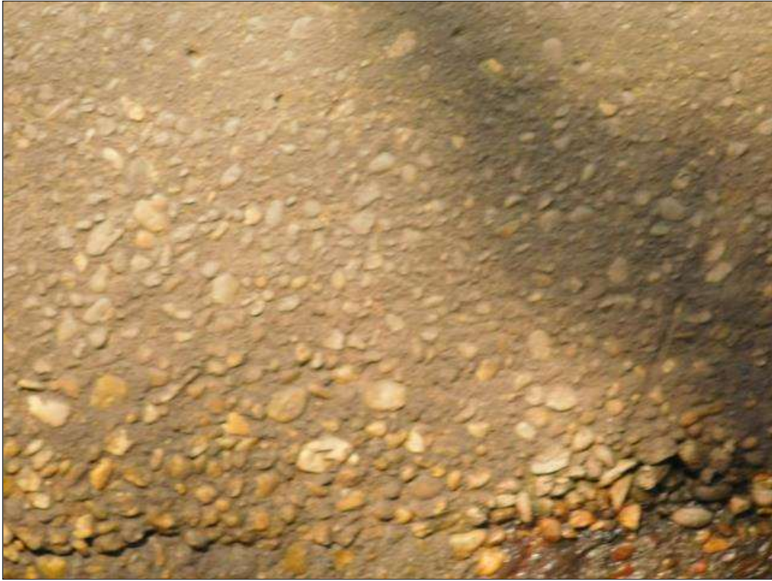
Barrel 1 Section 1: SOUTH WALL EXPOSED AGGREGATE
