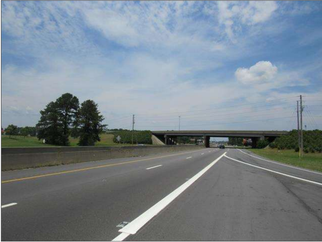
LOOKING NORTH IN NBL
