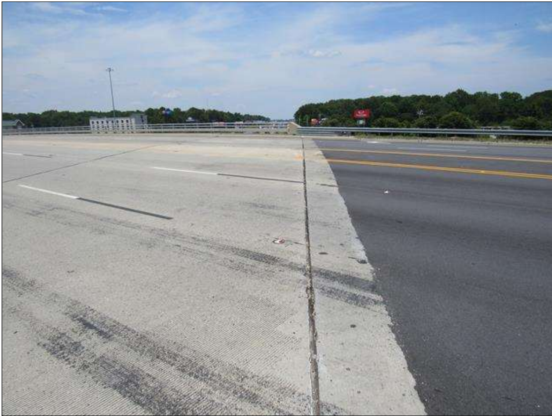
EXPANSION JOINT AT END BENT 2
