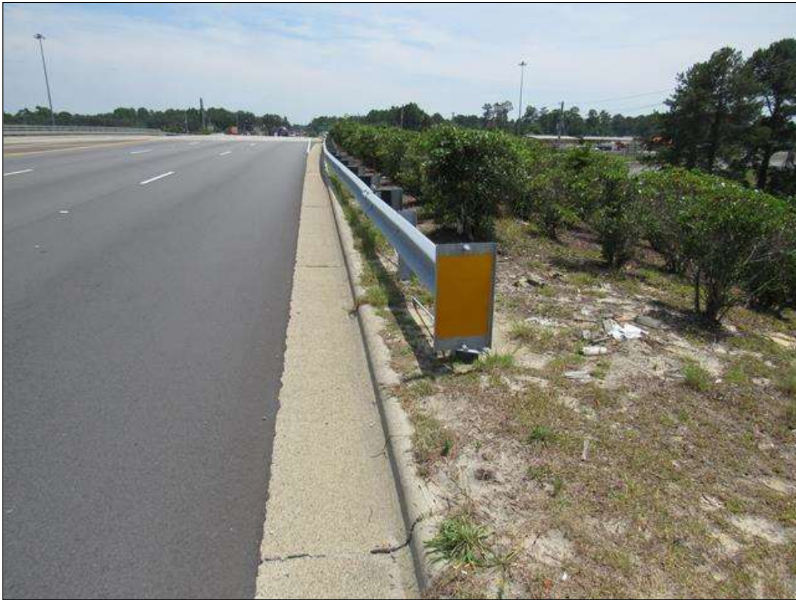
GUARD RAIL TERMINAL END
