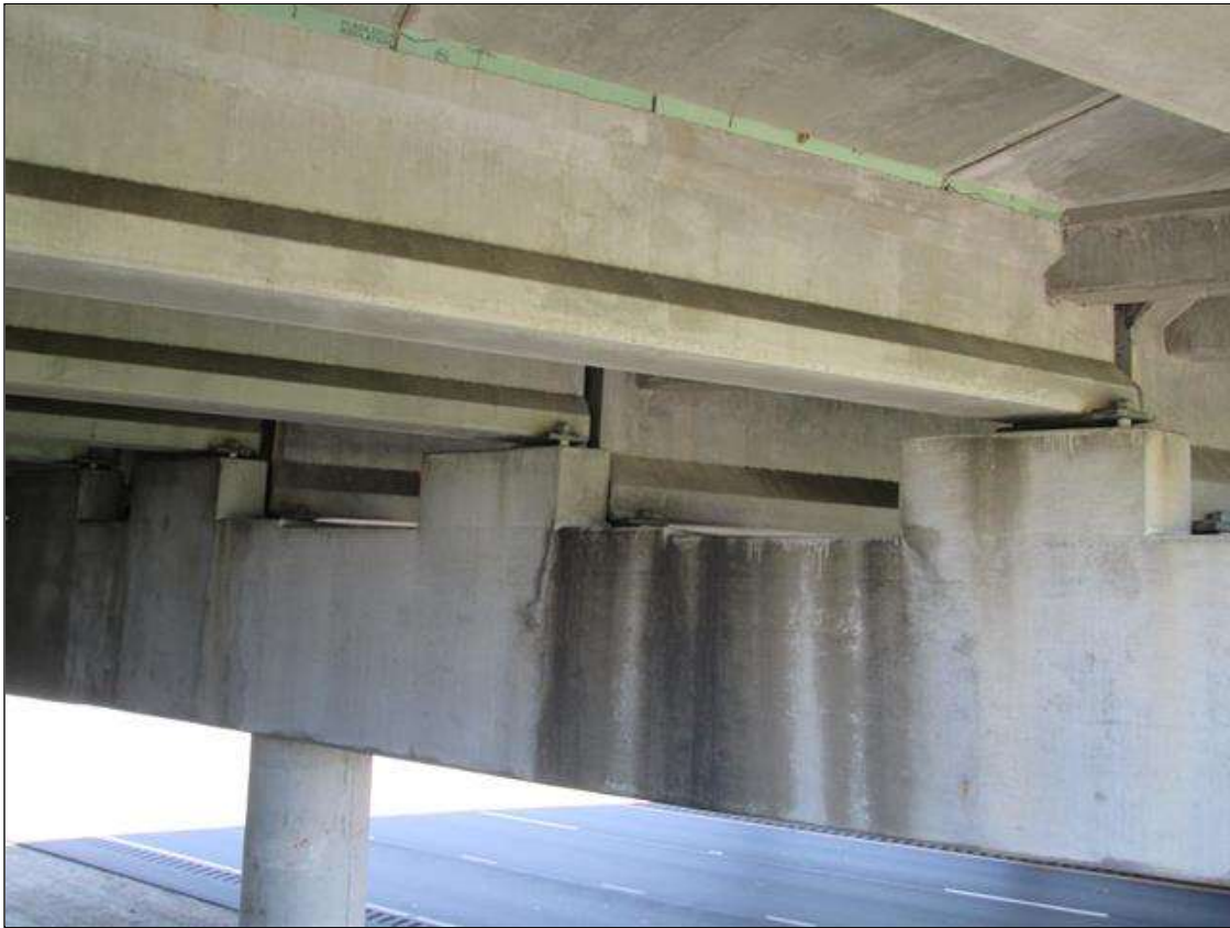
BENT 1 VIEW OF CAP RISERS UNDER GIRDERS.
