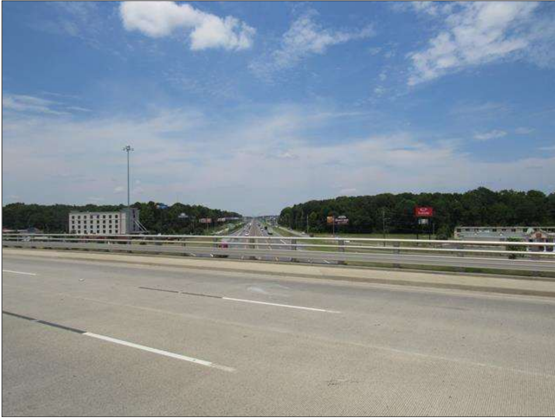
FROM BRIDGE LOOKING NORTH
