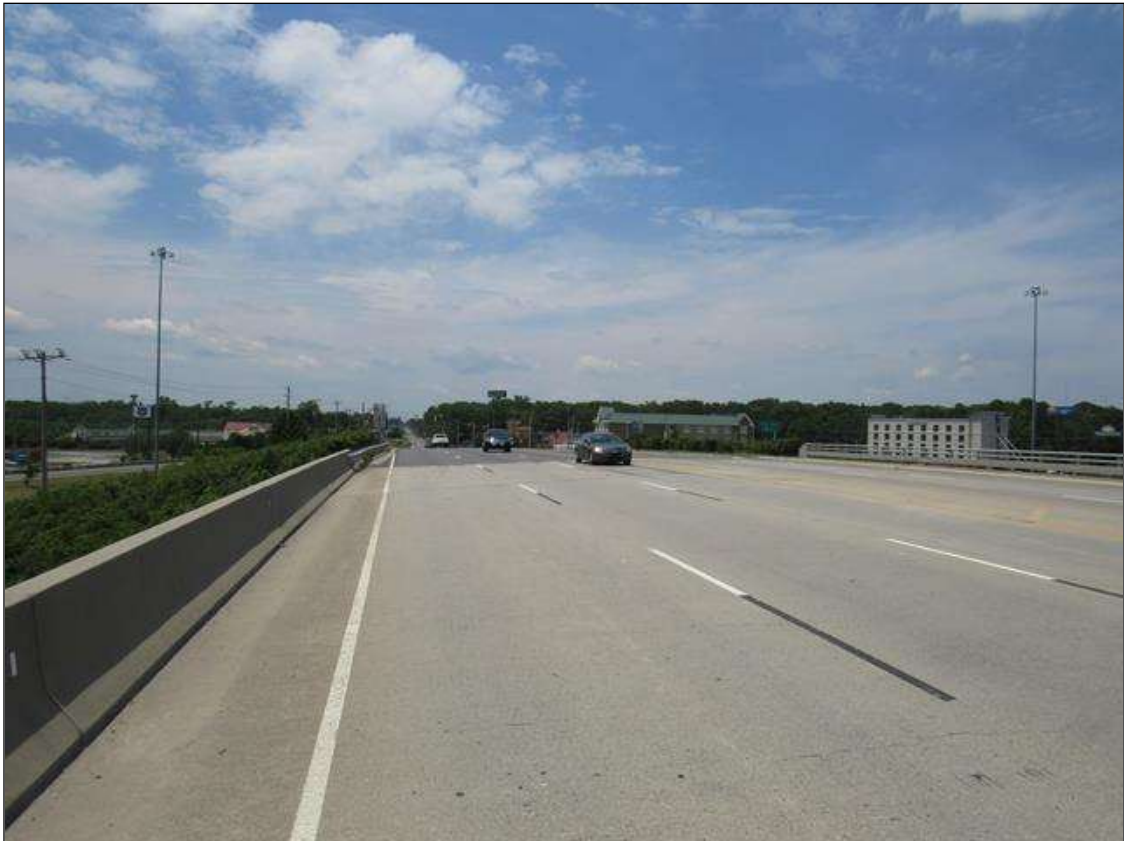
FROM BRIDGE LOOKING WEST
