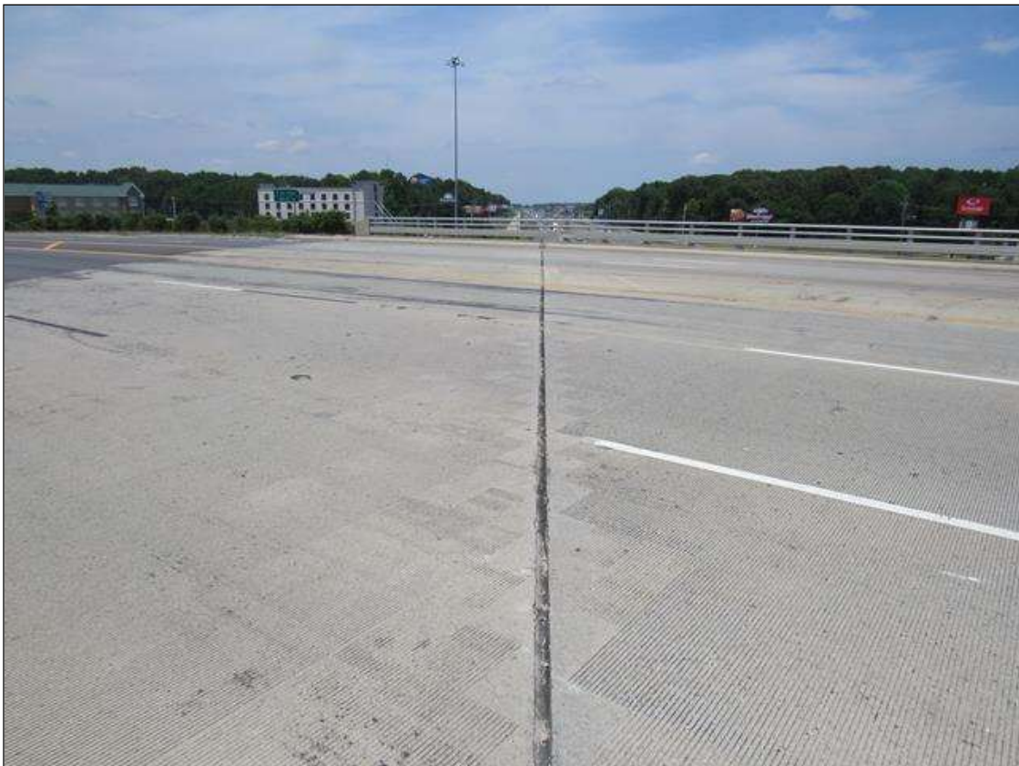
EXPANSION JOINT AT BENT 1
