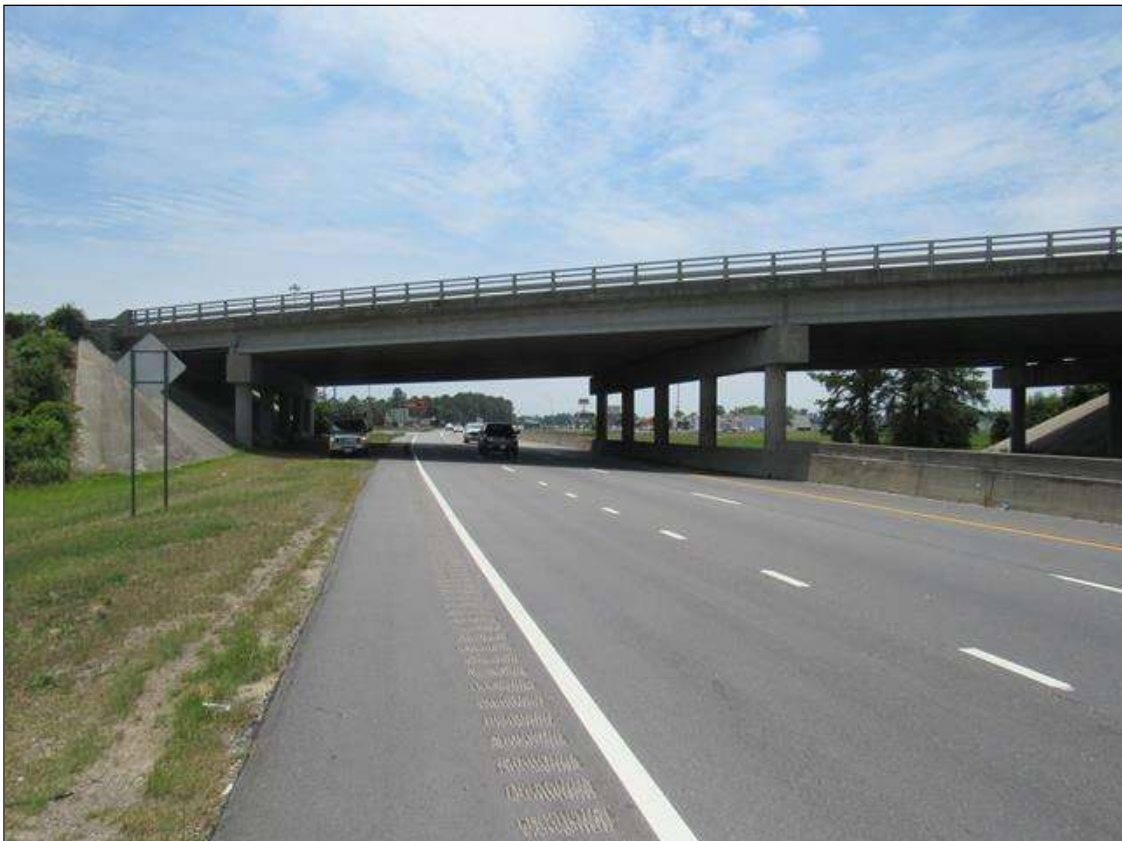
LOOKING SOUTH IN NBL
