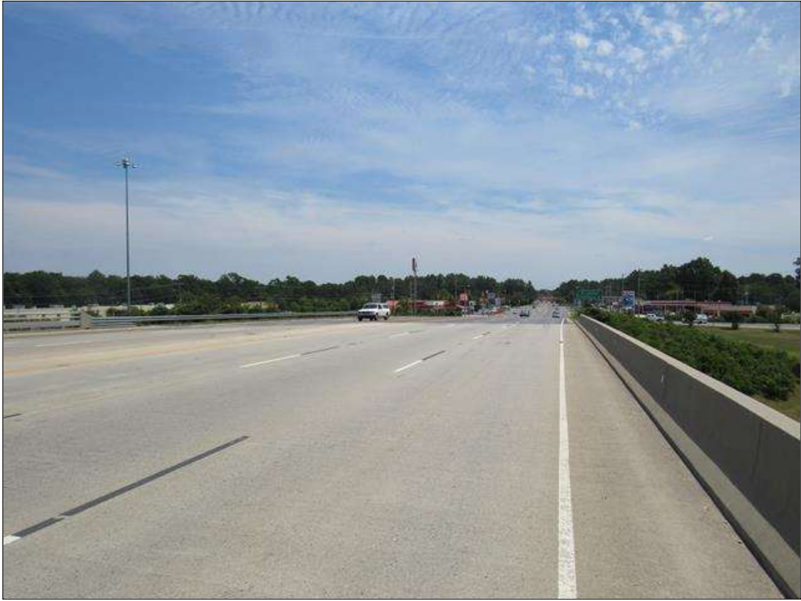
FROM BRIDGE LOOKING EAST
