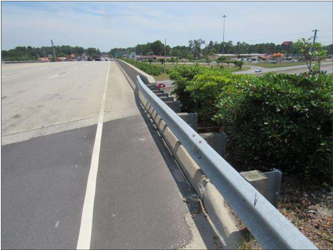
GUARD RAIL TRANSITION
