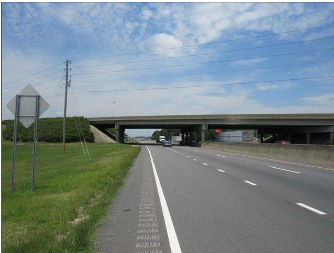
LOOKING NORTH IN SBL
