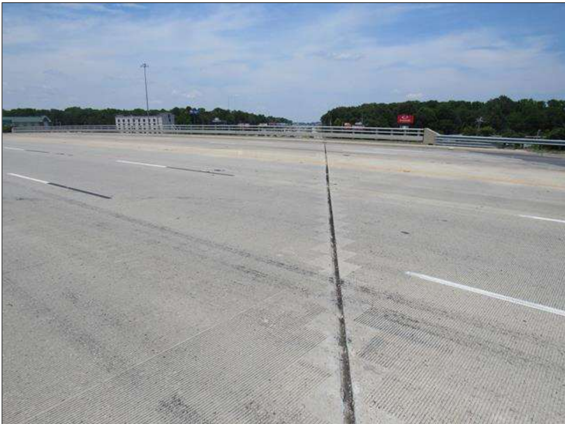
EXPANSION JOINT OVER BENT 3
