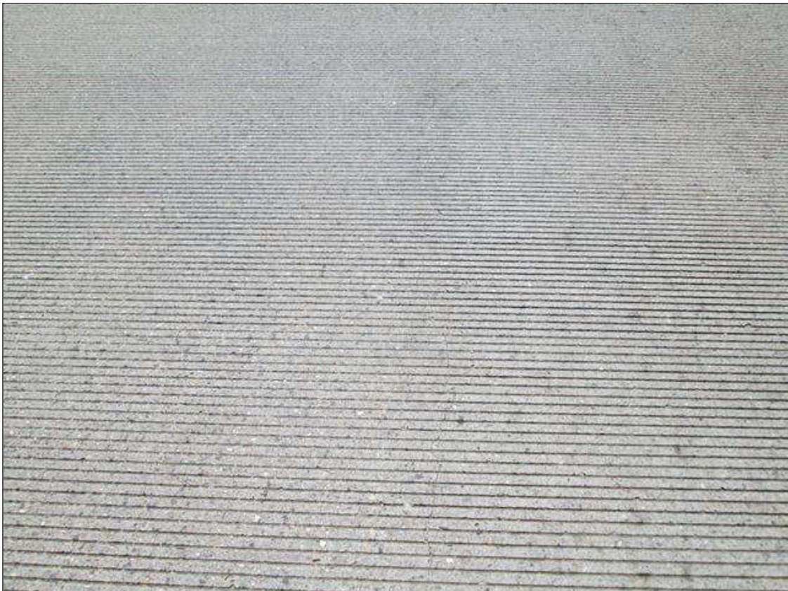
Span 2 Deck: SOME SCATTERED LONGITUDINAL CRACKS IN TOP OF DECK OF EBLs.
