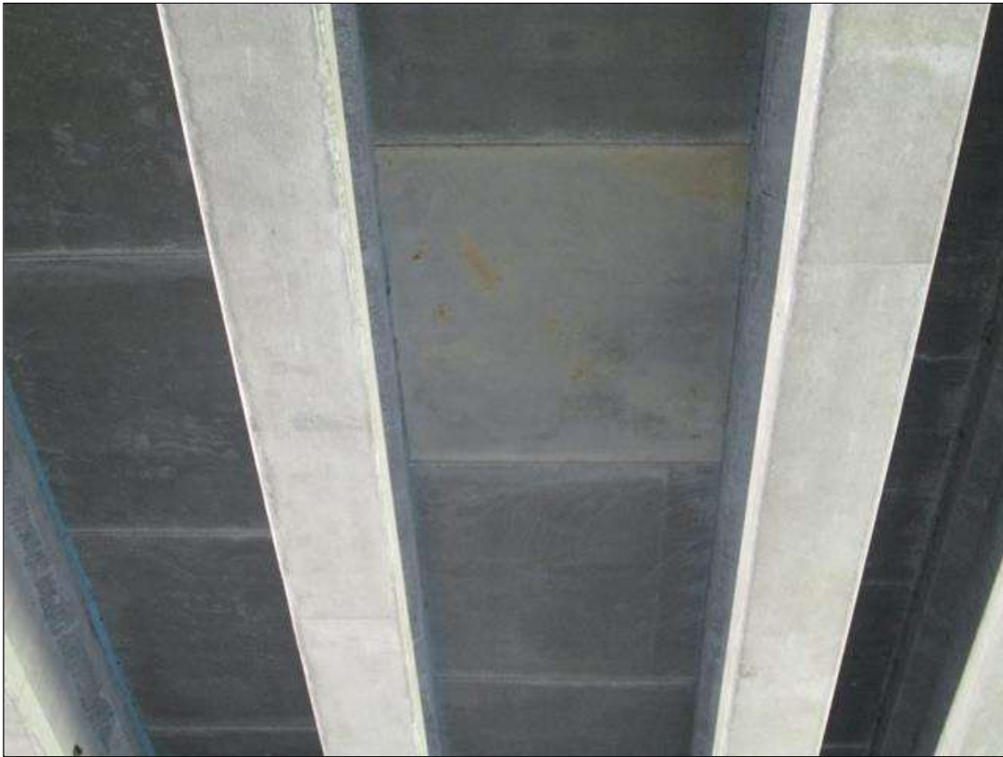
BOTTOM OF DECK HAS CONCRETE SIP FORMS
