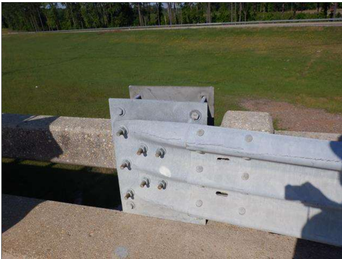
NW GUARD RAIL BRIDGE ATTACHMENT
