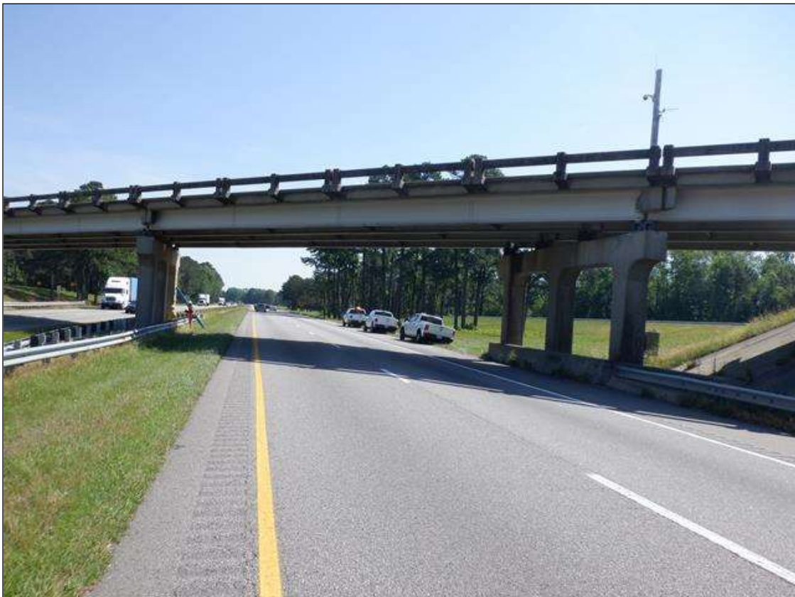
SPAN 2 THRU LANES
