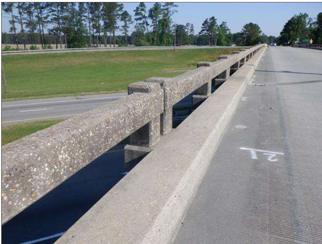
LEFT GUARD RAIL RIGHT RAIL SIMILAR
