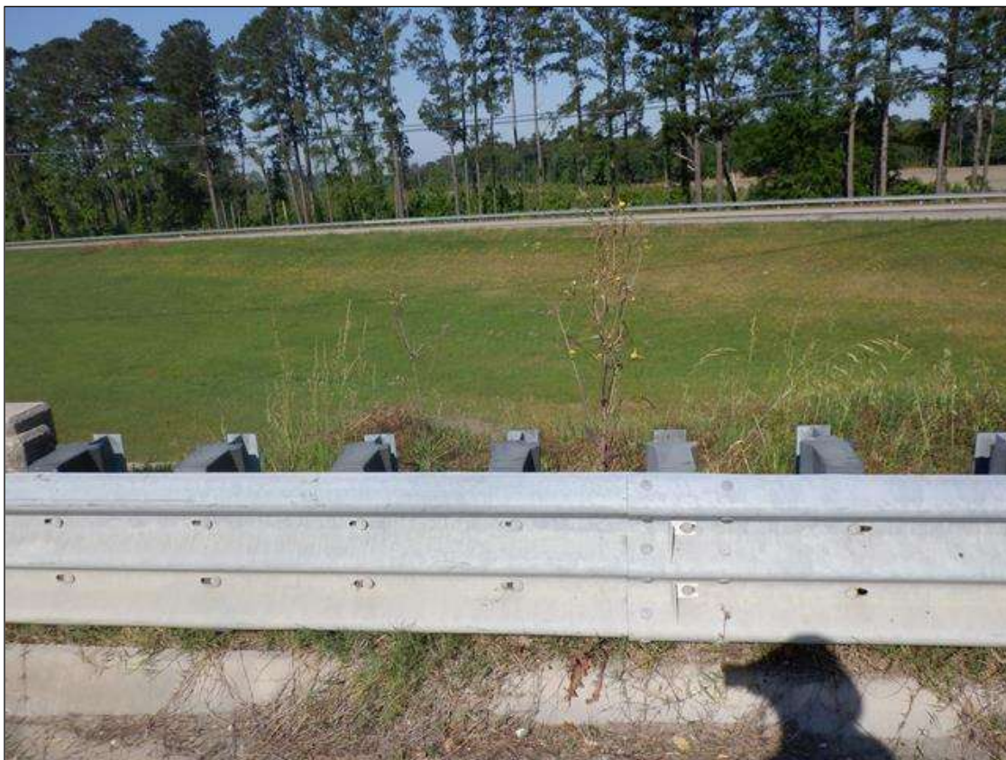
NW GUARD RAIL POST SPACING AT BRIDGE ATTACHMENT
