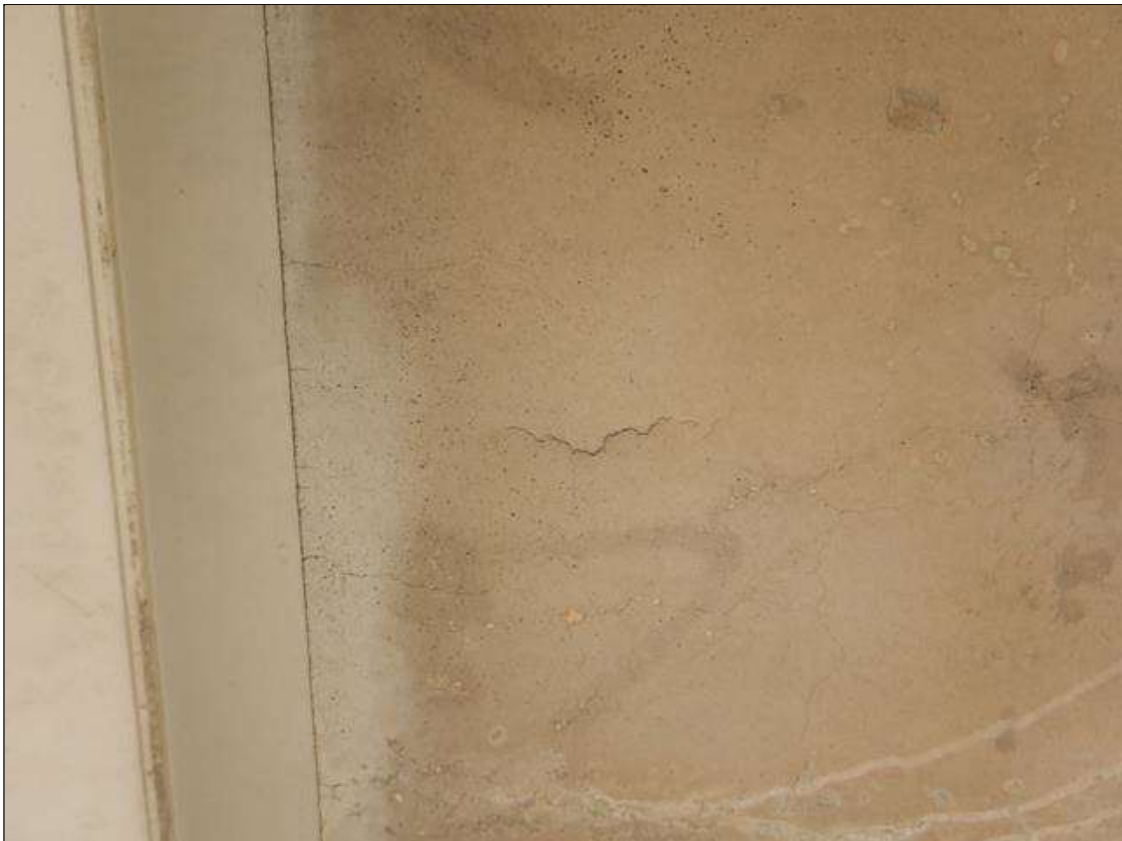
Span 3 Deck: 1 SF DELAMINATION IN BOTTOM OF DECK BAY 3 30 FT FROM BENT 2
