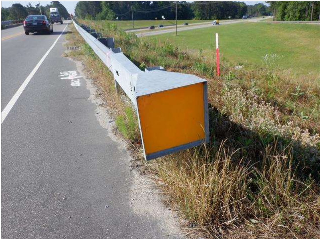
NW GUARD RAIL END TERMINAL
