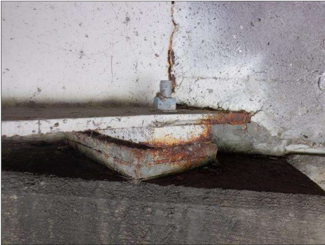
ABUTMENT 1 BEAM 3 BEARING
