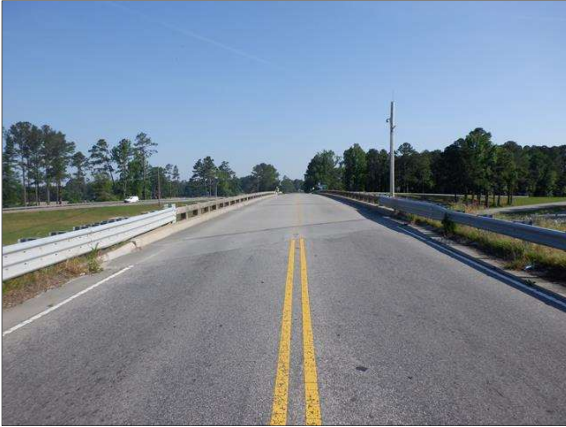
COVER SHEET PHOTO LOOKING NORTH
