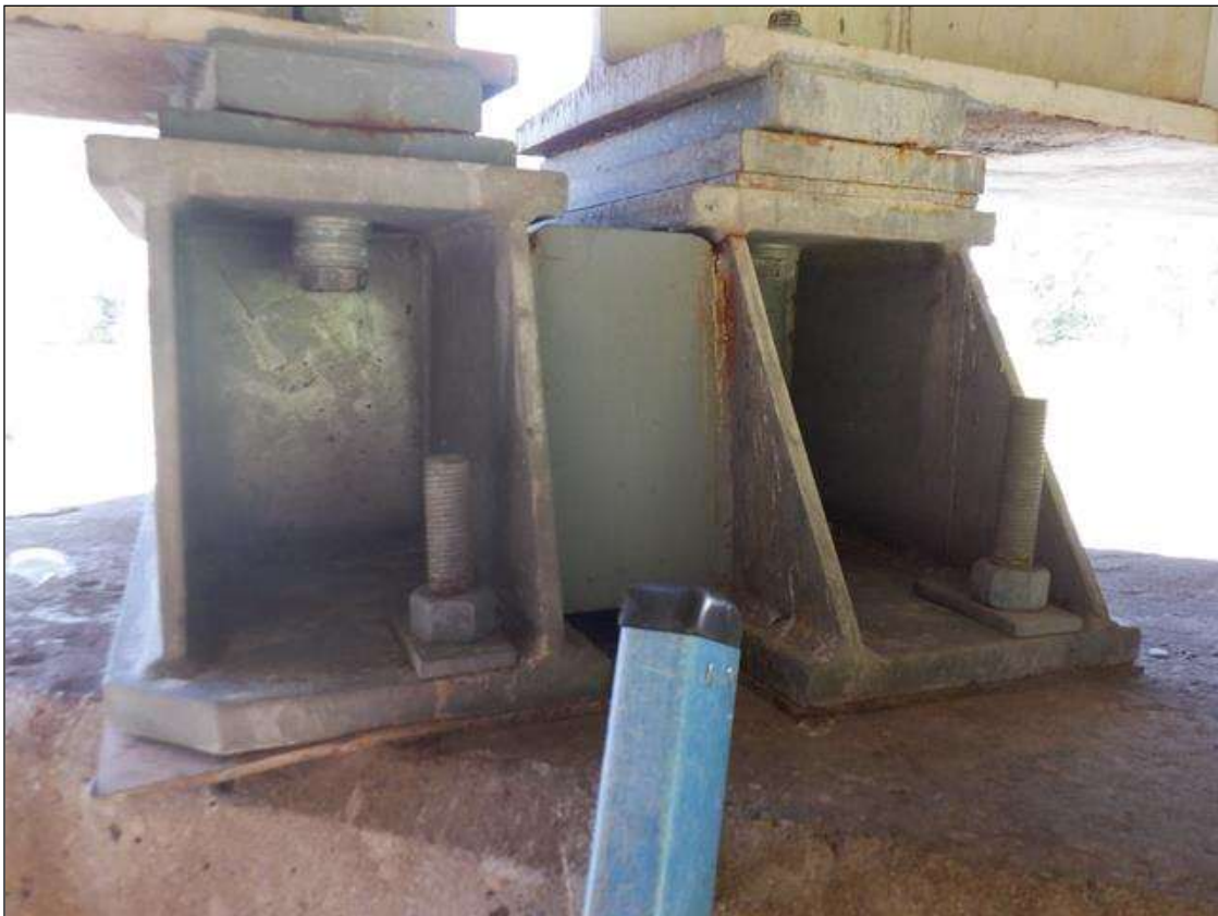
BENT 1 BEAM 1 BEARING
