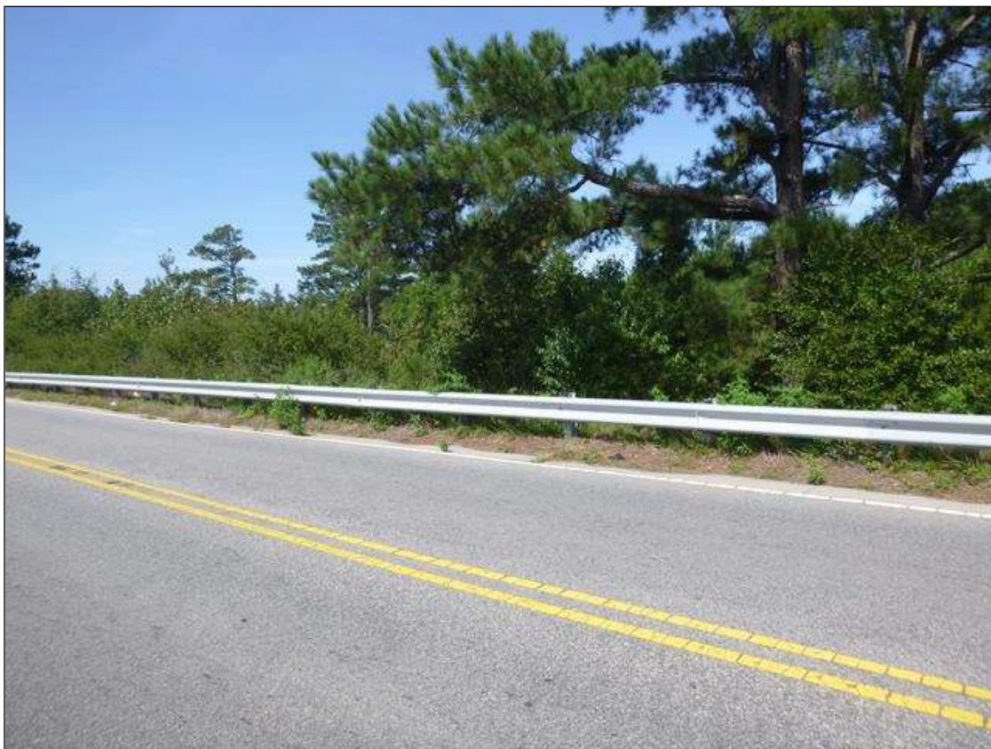
TYPICAL GUARDRAIL, NORTHWEST SHOWN
