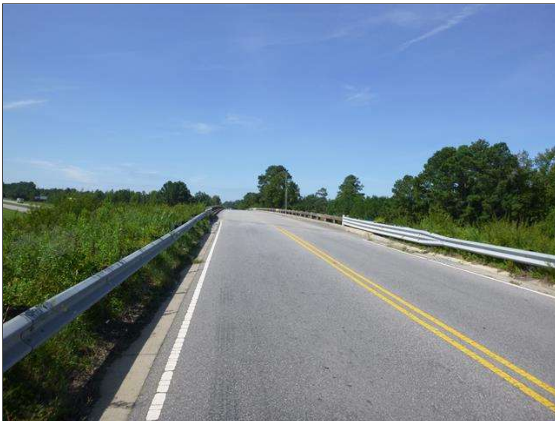
EAST APPROACH, LOOKING WEST
