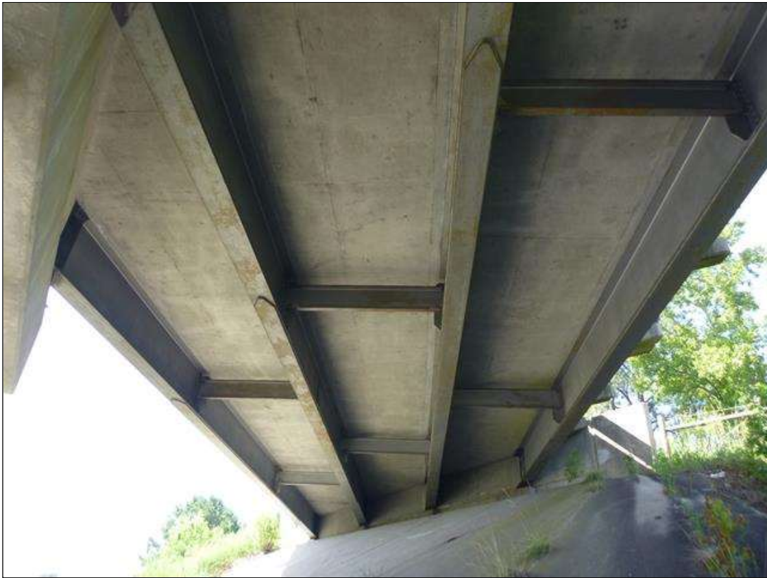
SUPERSTRUCTURE UNDERSIDE, SPAN 1, LOOKING WEST
