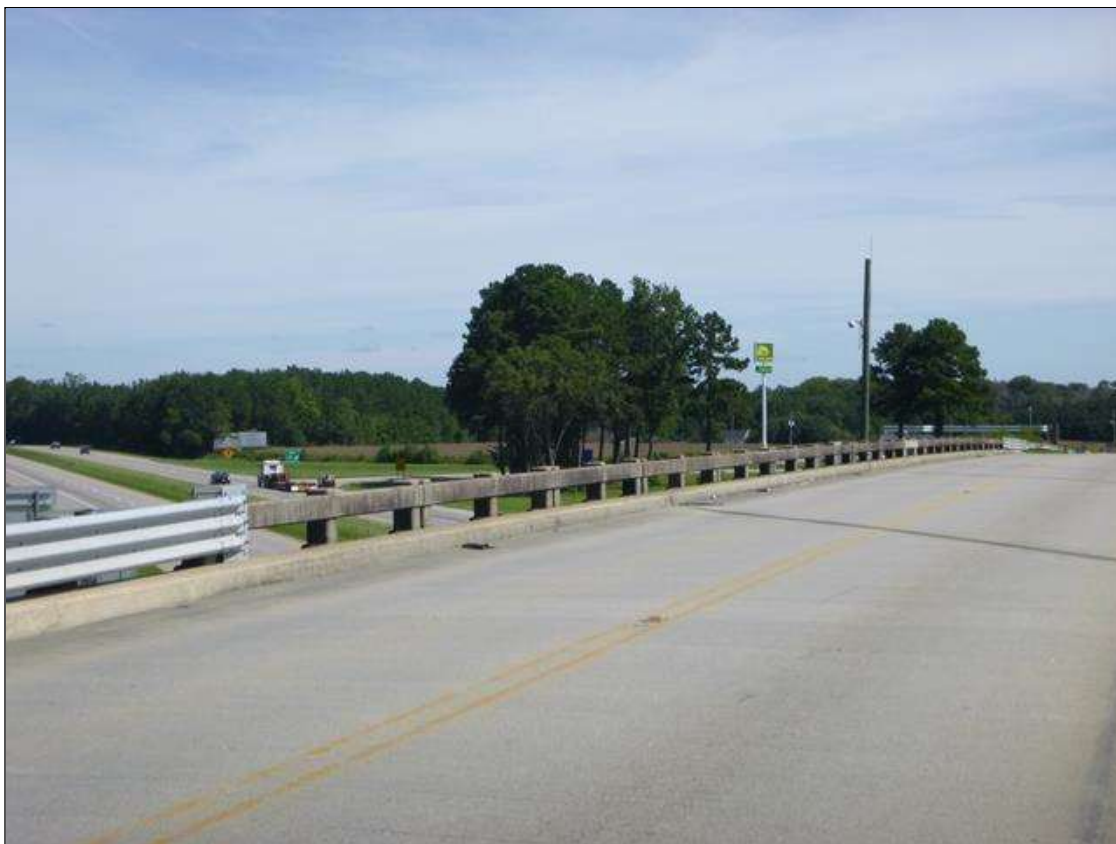
NORTH BRIDGE RAIL
