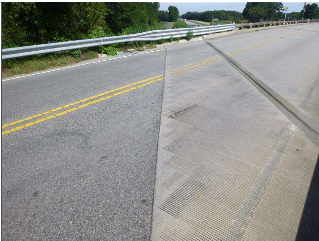
TRANSITION BETWEEN WEST APPROACH ROADWAY AND WEST APPROACH SLAB, LOOKING NORTH
