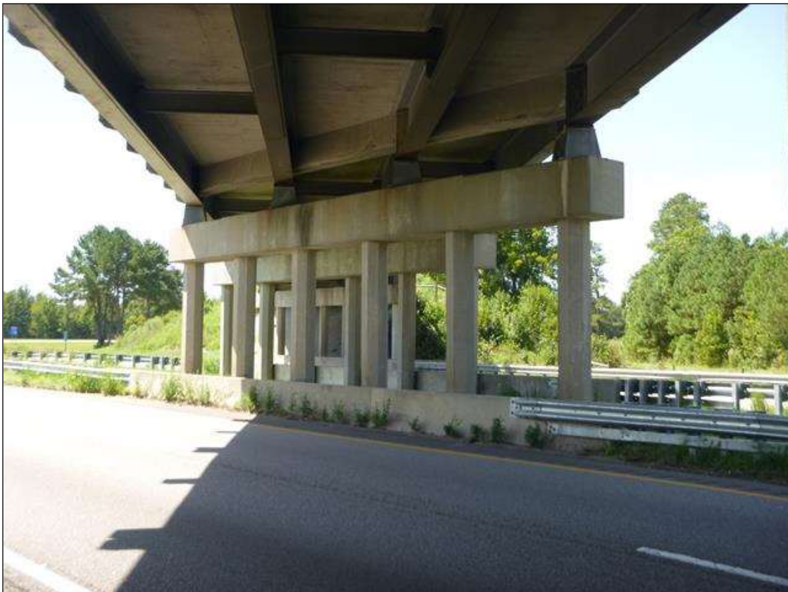
BENT 3 ELEVATION, LOOKING WEST
