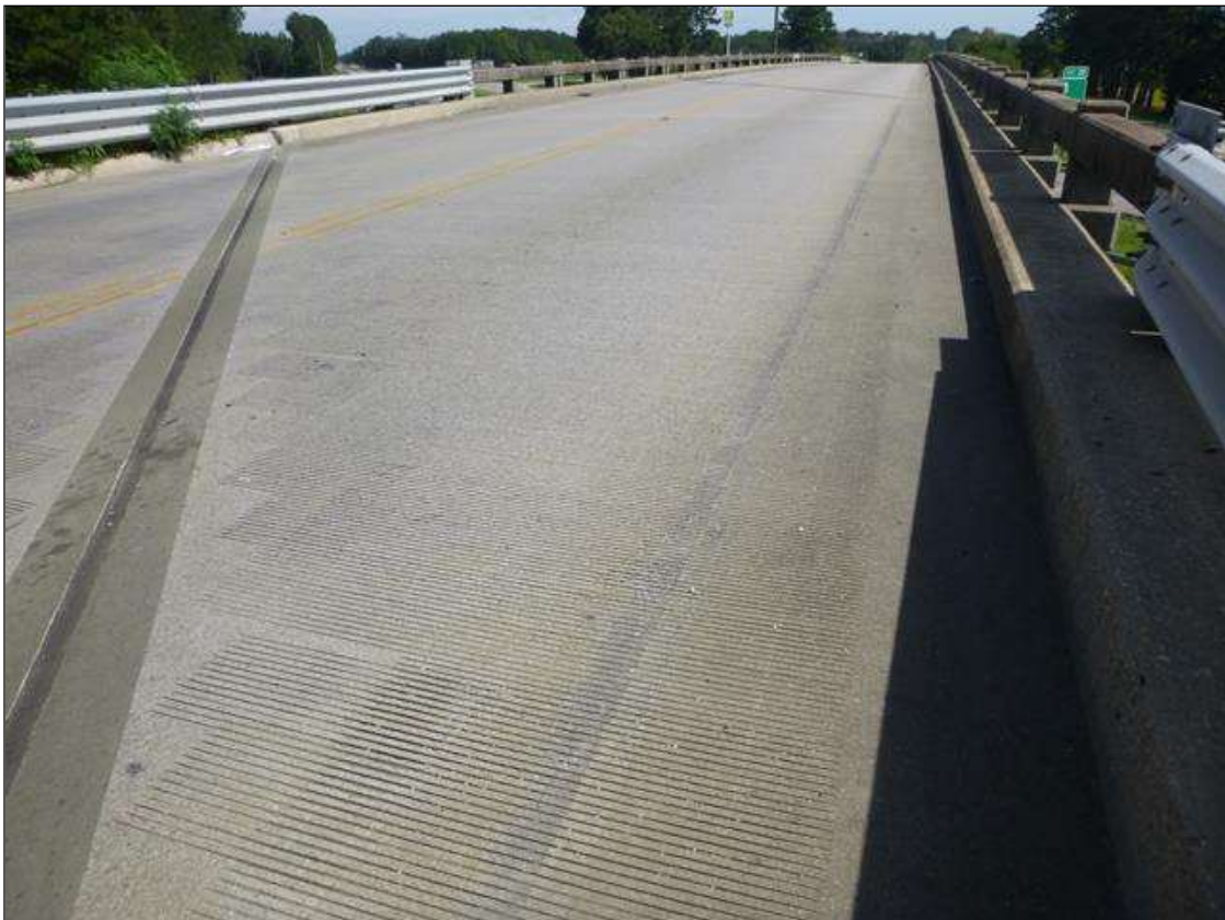
CONCRETE BRIDGE DECK
