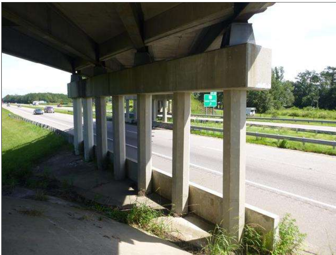
BENT 1 ELEVATION, LOOKING EAST
