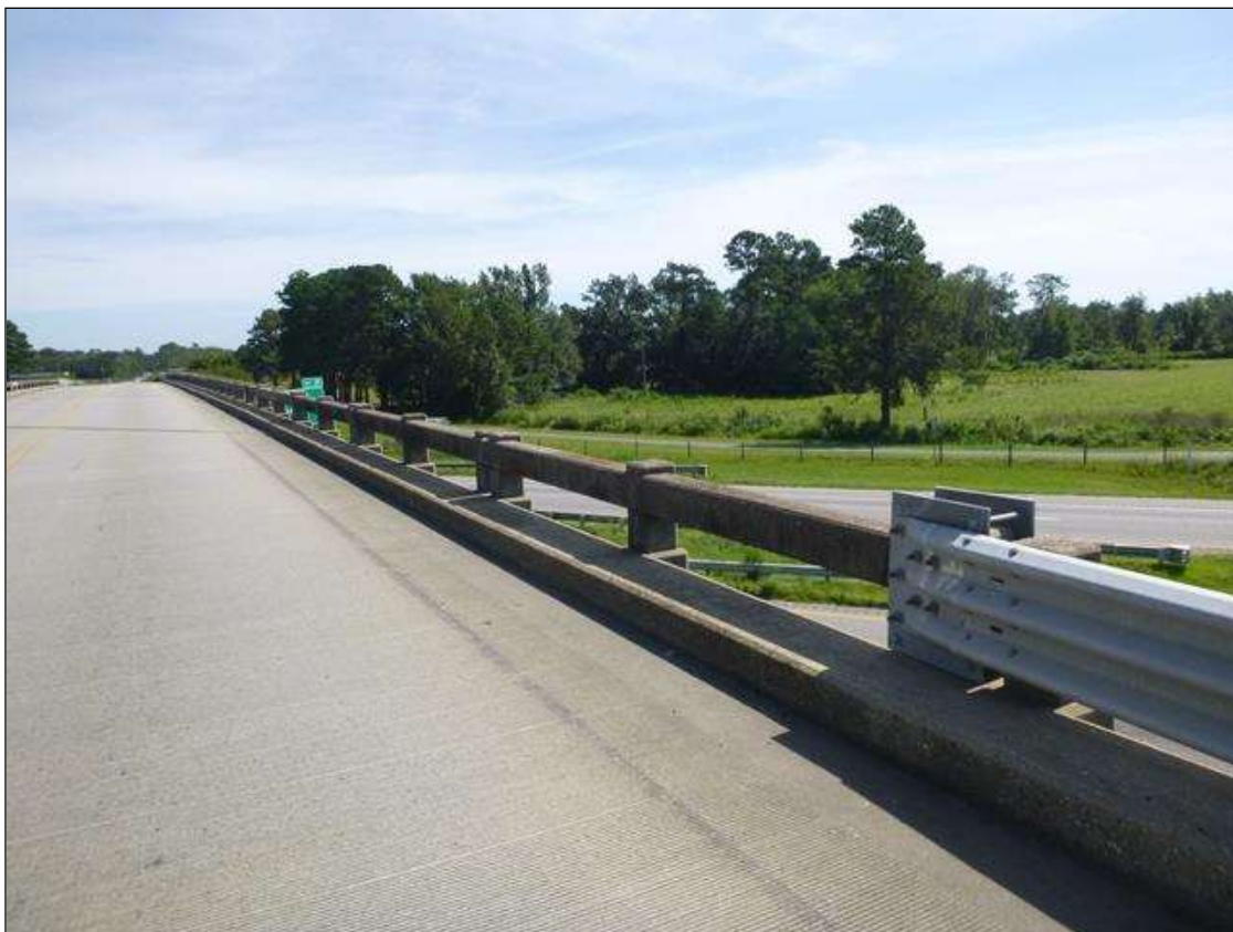
SOUTH BRIDGE RAIL
