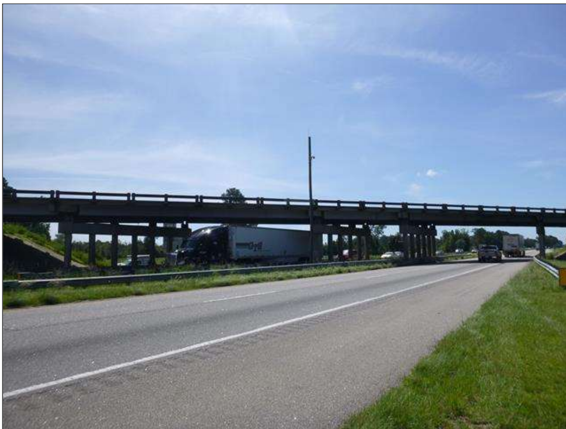
NORTH PROFILE, LOOKING SOUTH
