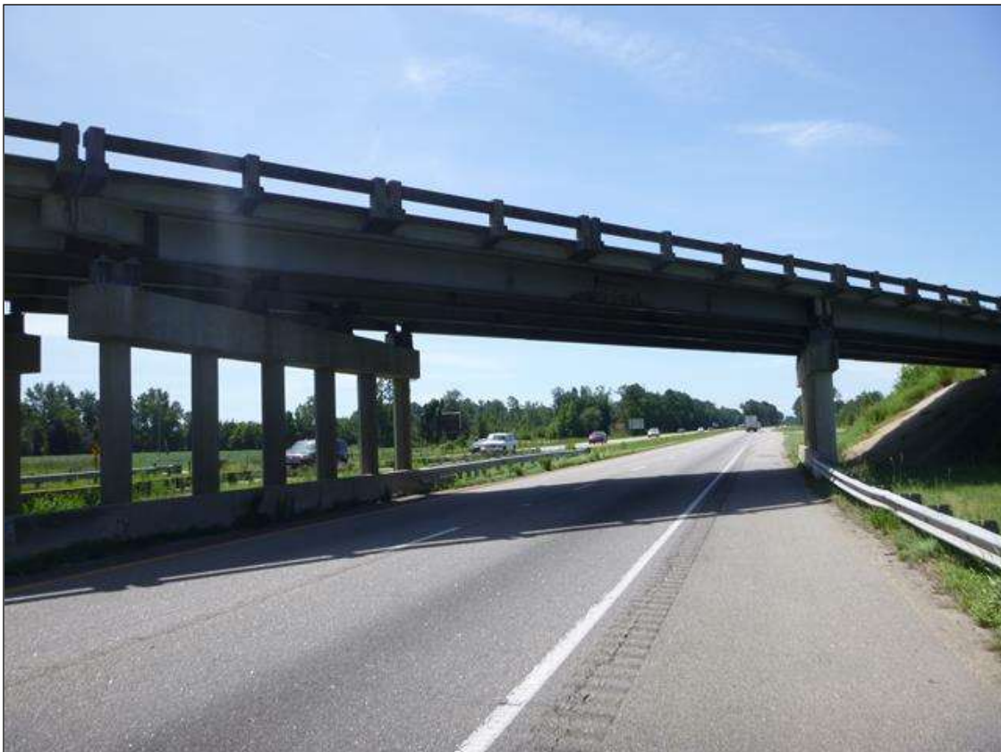
SPAN 2 CLEARANCE, LOOKING SOUTH
