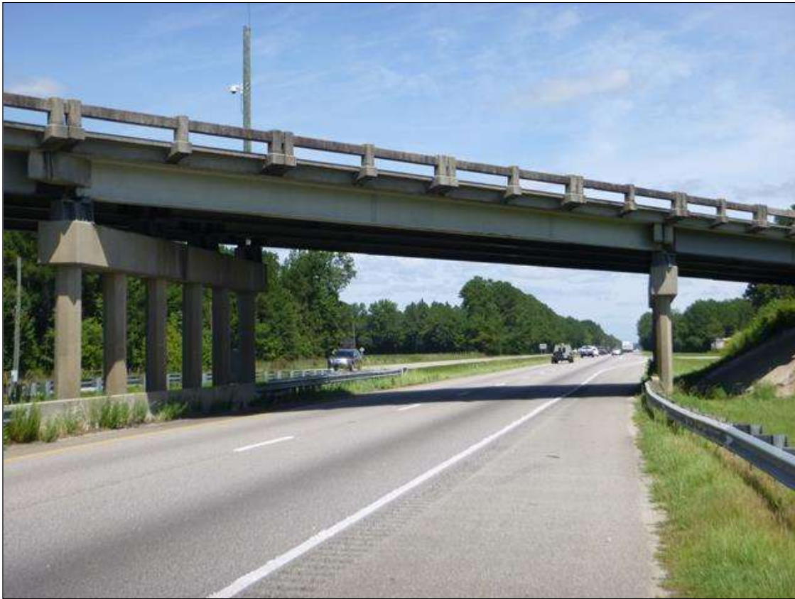
SPAN 4 CLEARANCE, LOOKING NORTH
