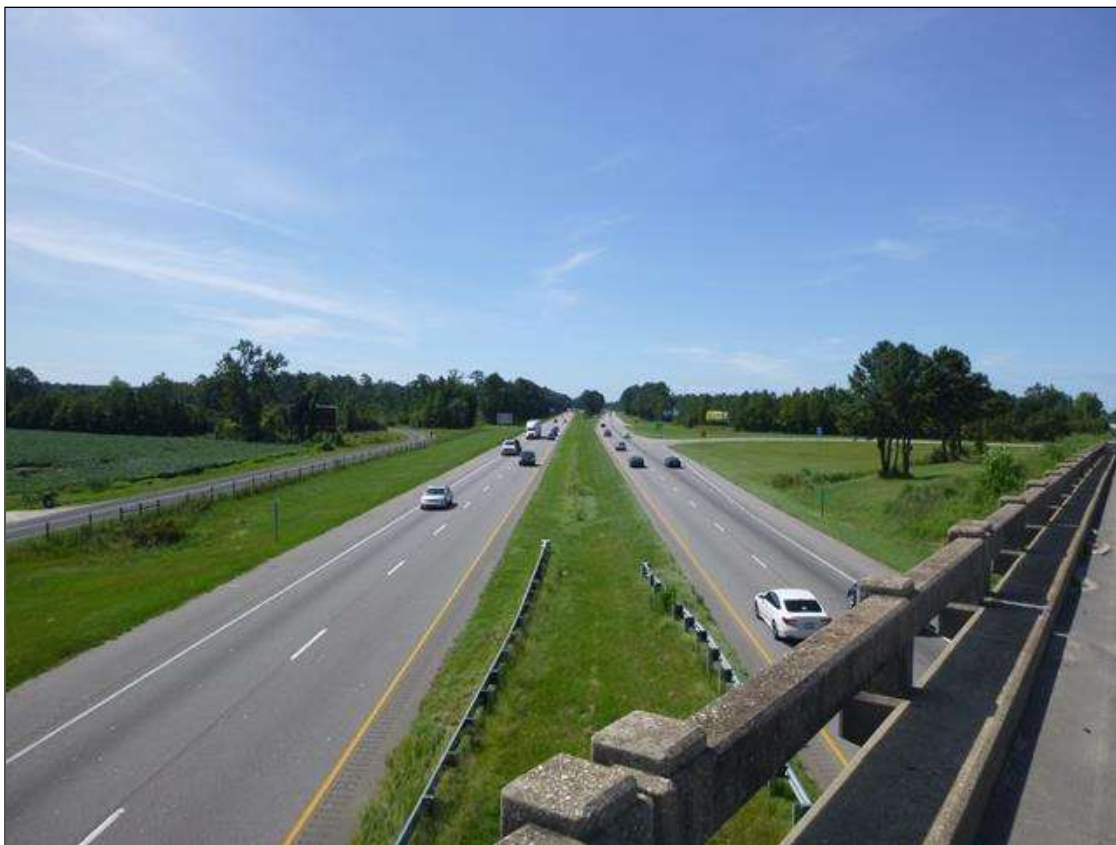
ROADWAY VIEW FROM BRIDGE DECK, LOOKING SOUTH
