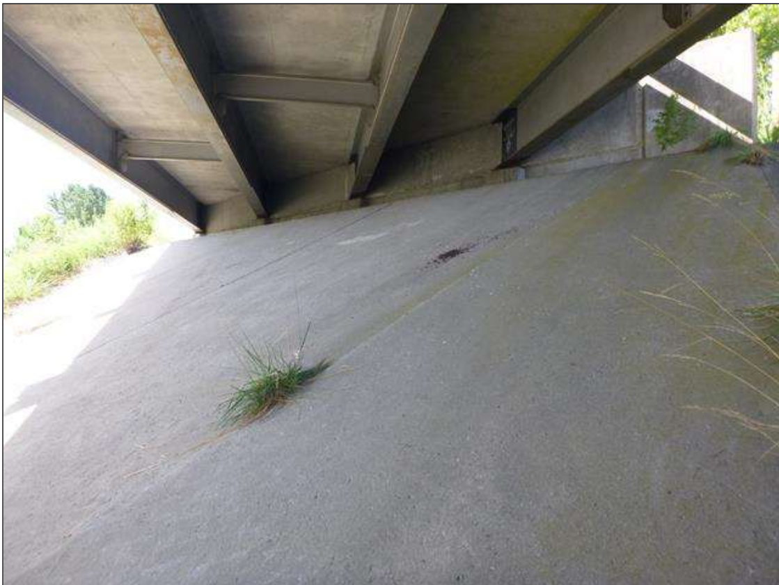
END BENT 1 SLOPE PROTECTION, LOOKING WEST
