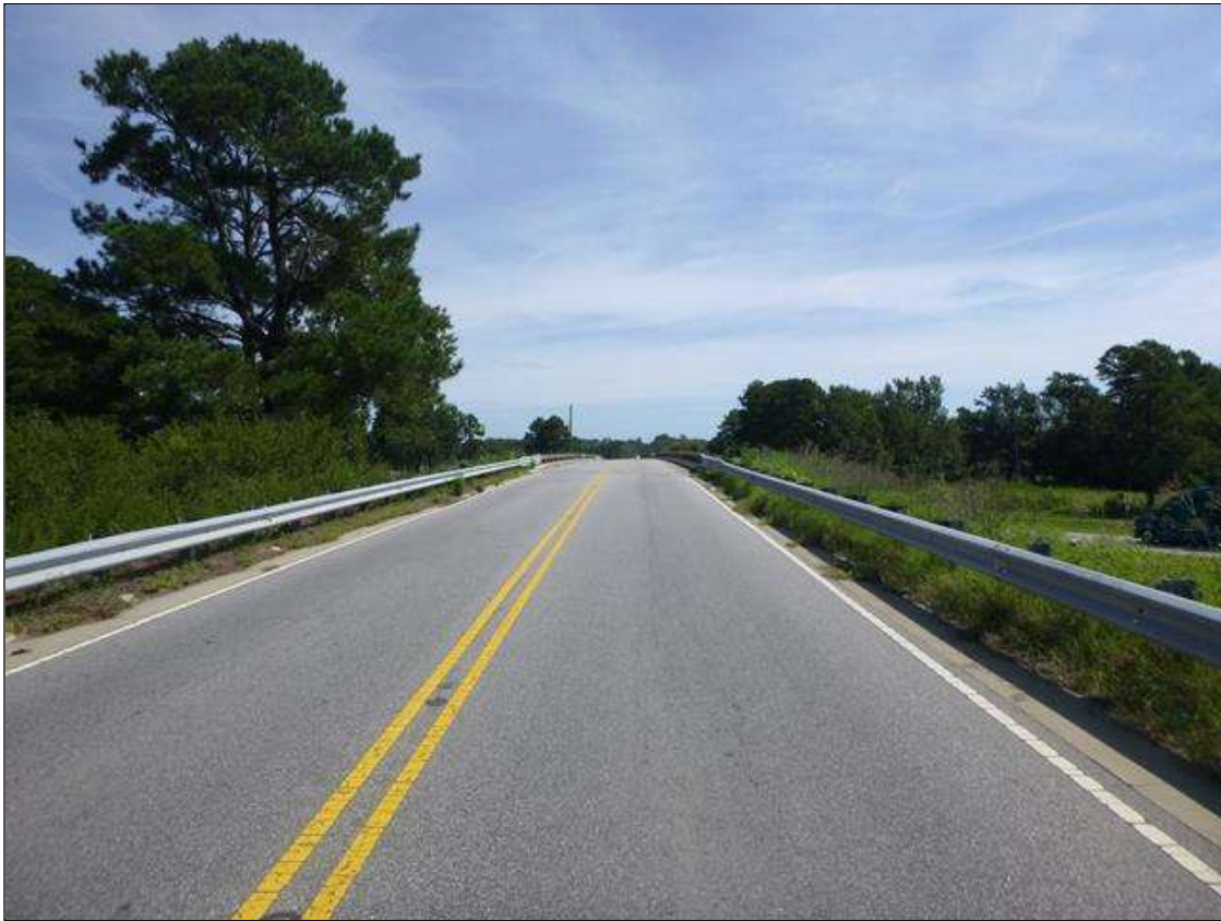
WEST APPROACH, LOOKING EAST
