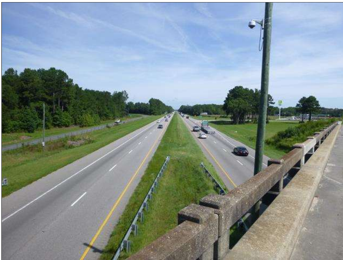
ROADWAY VIEW FROM BRIDGE DECK, LOOKING NORTH
