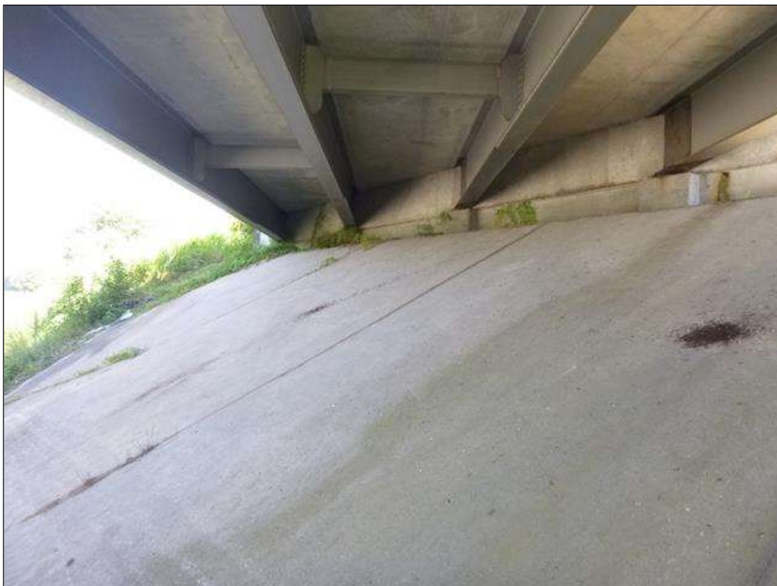
END BENT 2 SLOPE PROTECTION, LOOKING EAST
