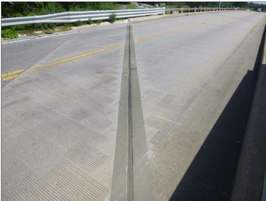
TYPICAL EXPANSION JOINT, END BENT 1 SHOWN, LOOKING NORTH, (ALL BENTS SIMILAR)
