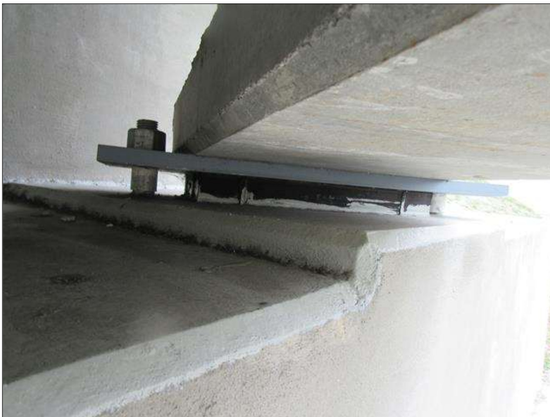
SPAN 1 BEAM 1 NEAR BEARING
