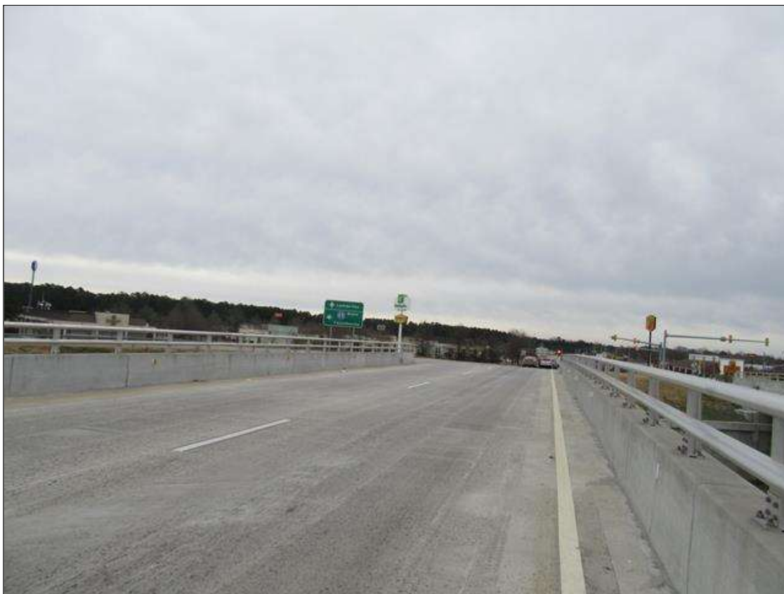
LOOKING SOUTH, OFF BRIDGE
