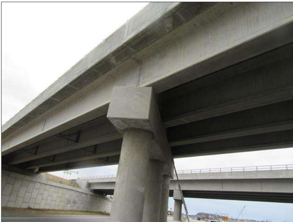
EAST END OF BENT 1 CAP
