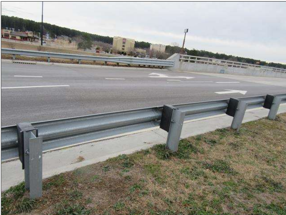
GUARDRAIL POST SPACING AT MID PORTION
