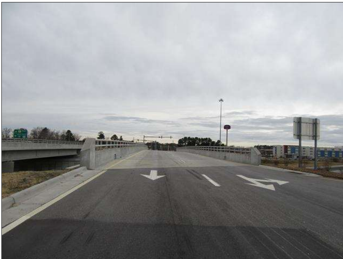
LOOKING NORTH, SOUTHBOUND LANE
