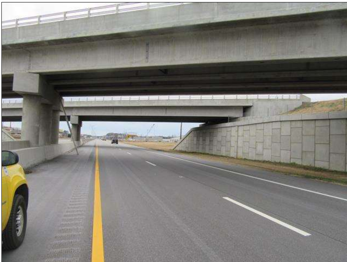
LOOKING WEST, SOUTHBOUND LANE I 95 THRU SPAN 2
