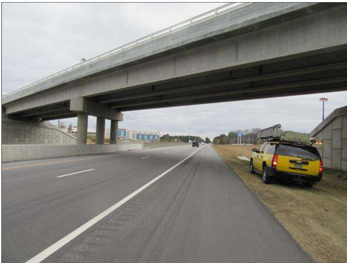
LOOKING EAST, NORTHBOUND LANE I 95 THRU SPAN 1
