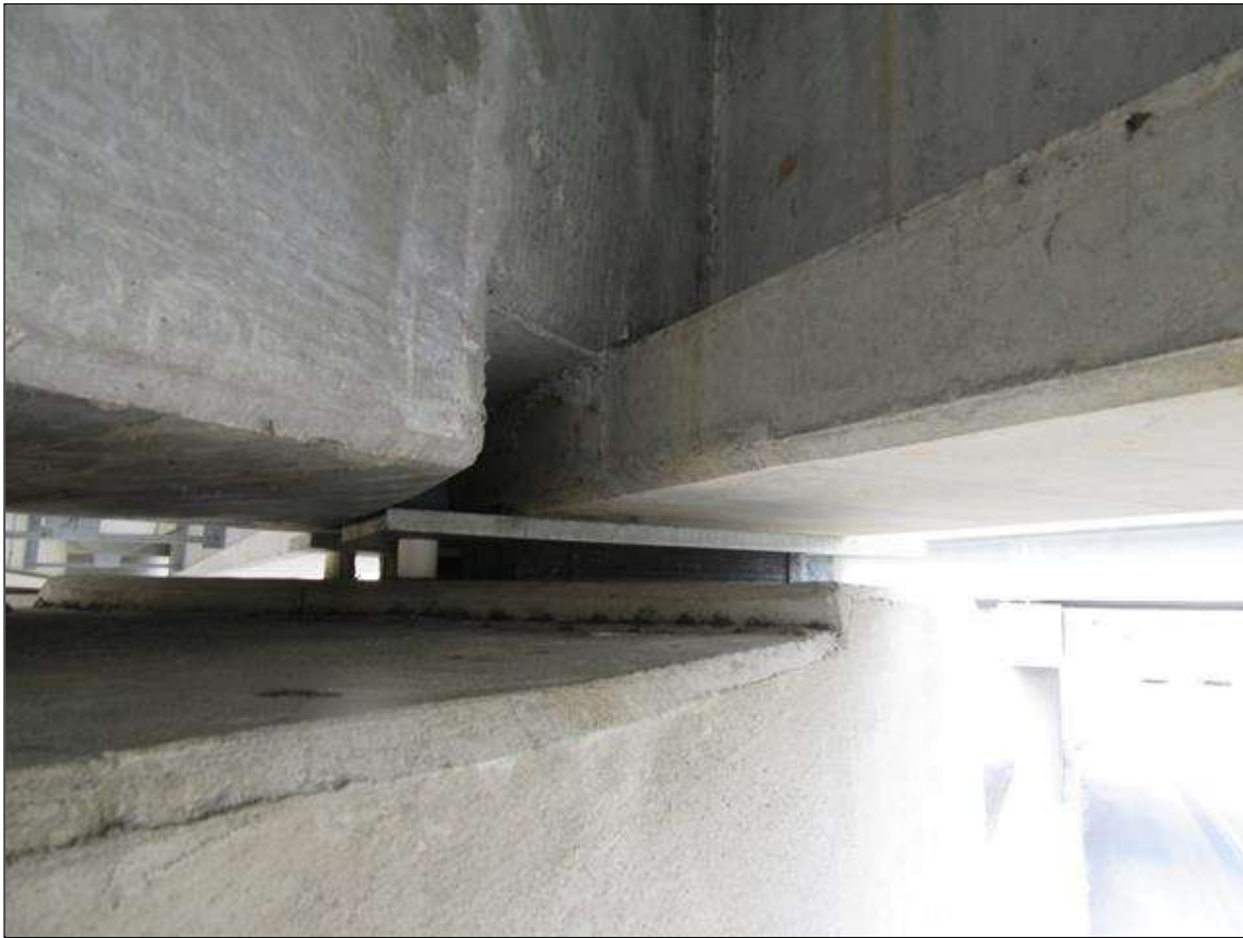
SPAN 2 BEAM 1 NEAR BEARING
