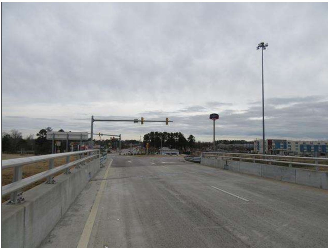
LOOKING NORTH, OFF BRIDGE
