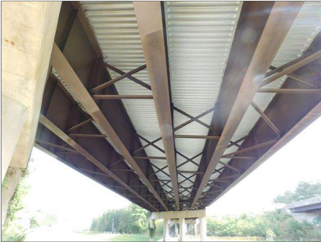
SPAN 2 SUPERSTRUCTURE, SPAN 3 SIMILAR
