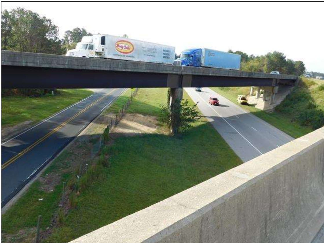
LOOKING WEST, NORTH 95 BUS.
