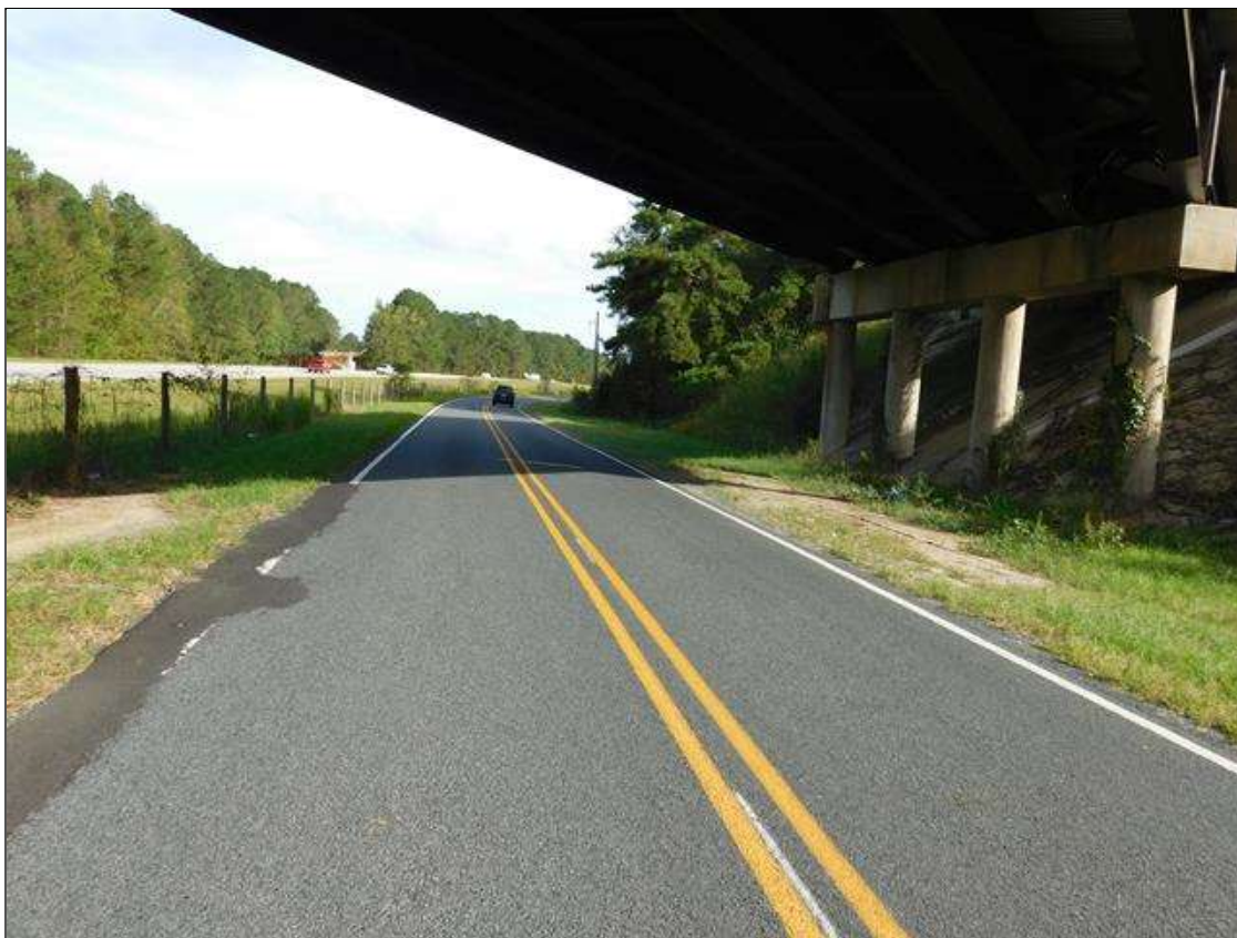
LOOKING WEST, SR 2284 THRU SPAN 3
