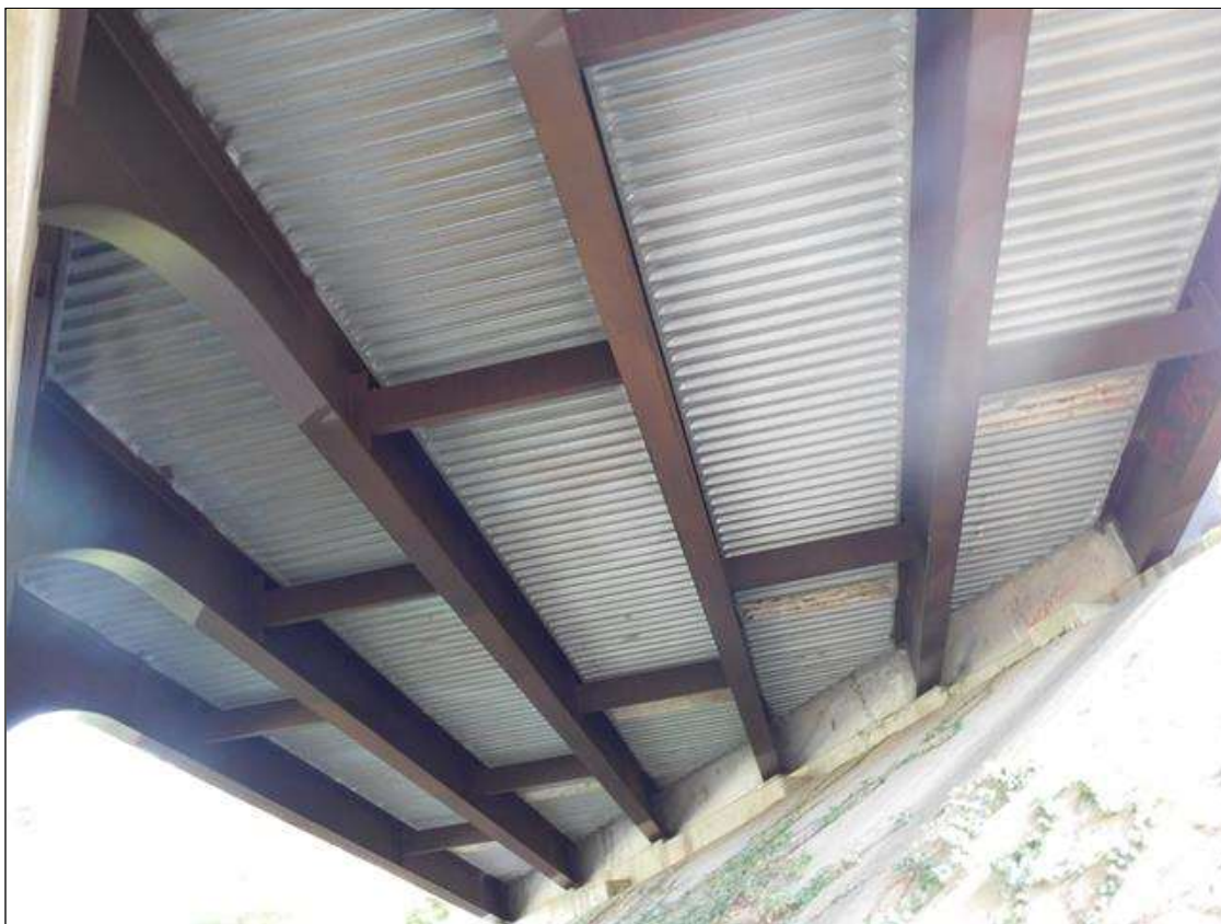
SPAN 4 SUPERSTRUCTURE, SPAN 1 SIMILAR
