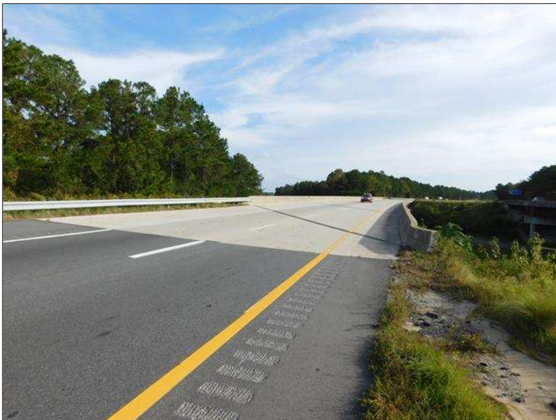
LOOKING NORTH, SOUTHBOUND LANE
