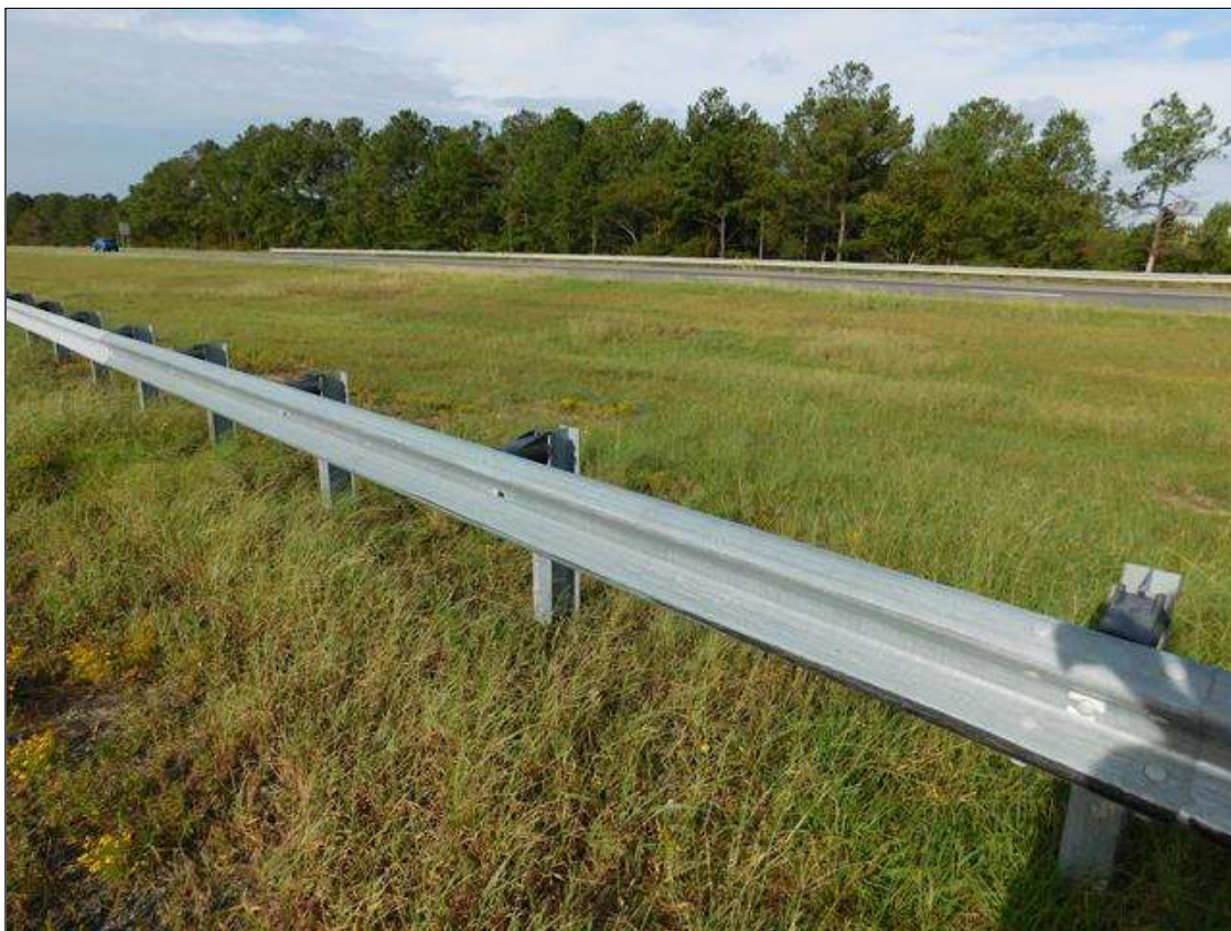
GUARDRAIL POST SPACING AT MID PORTION
