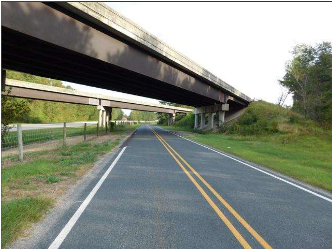
LOOKING WEST, SR 2284 THRU SPAN 3
