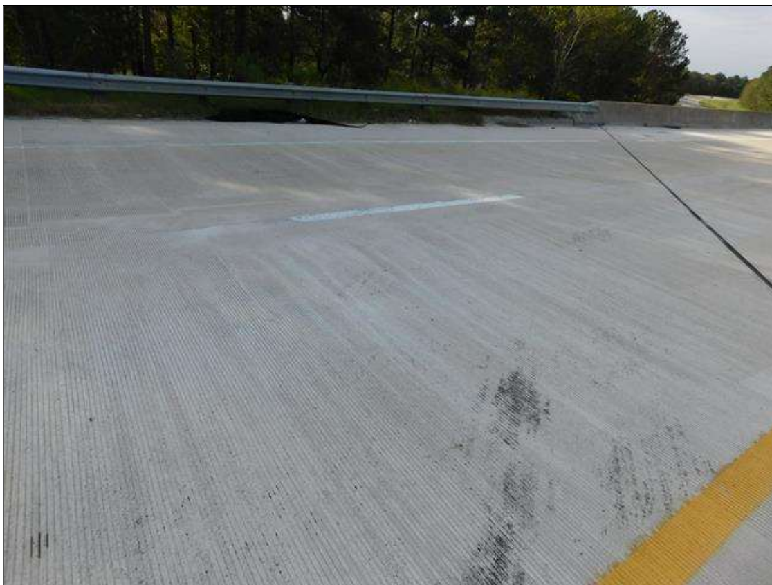
NORTH APPROACH SLAB MILLED AND RESURFACED, SAME MEASUREMENTS
