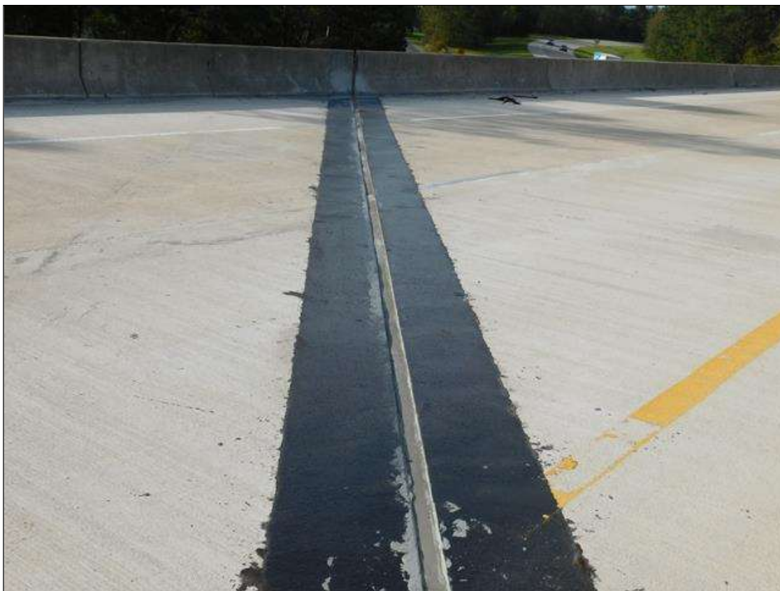
BENT 3 JOINT, NEW
