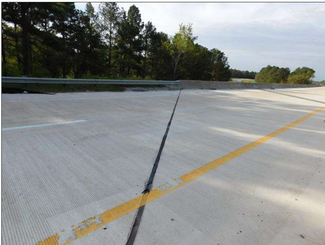
END BENT 2 JOINT NEW
