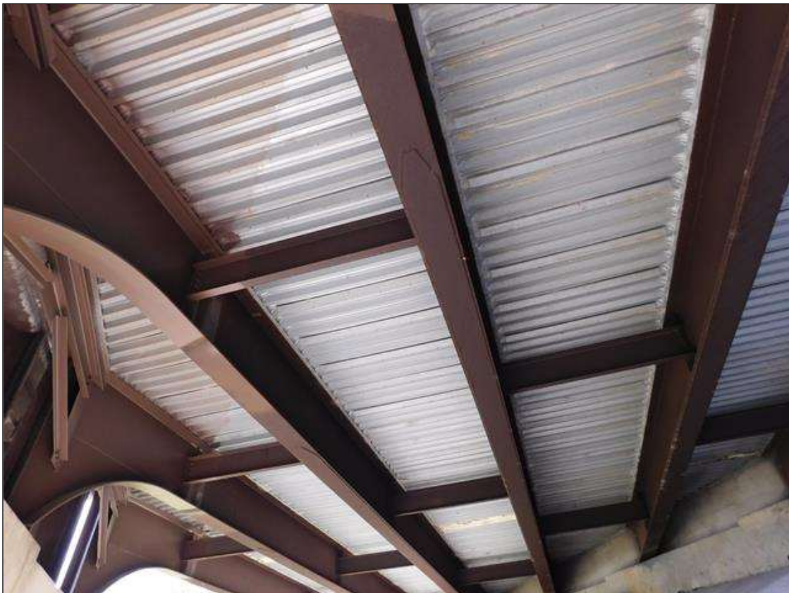
SPAN 1 SUPERSTRUCTURE, SPAN 4 SIMILAR
