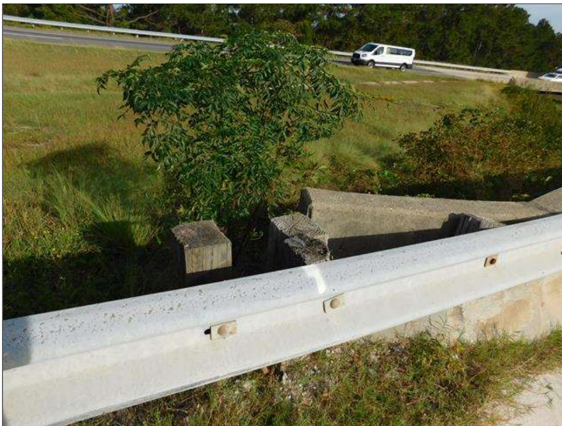
GUARDRAIL POST SPACING AT TRANSITION
