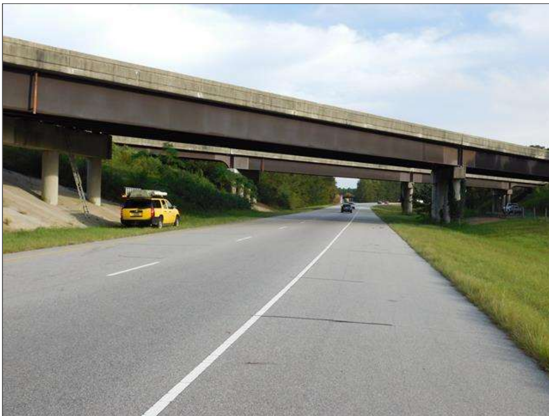
LOOKING WEST, NORTHBOUND LANE 95 BUSINESS THRU SPAN 2
