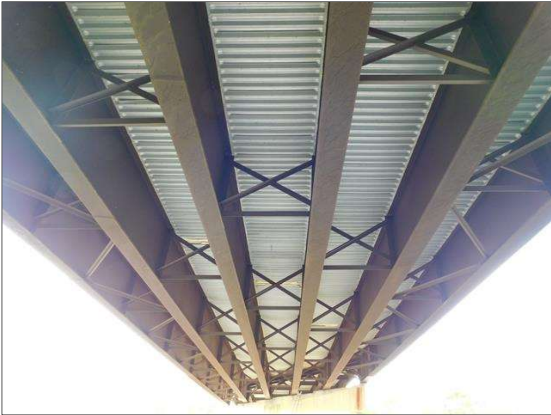
SPAN 2 SUPERSTRUCTURE, SPAN 3 SIMILAR
