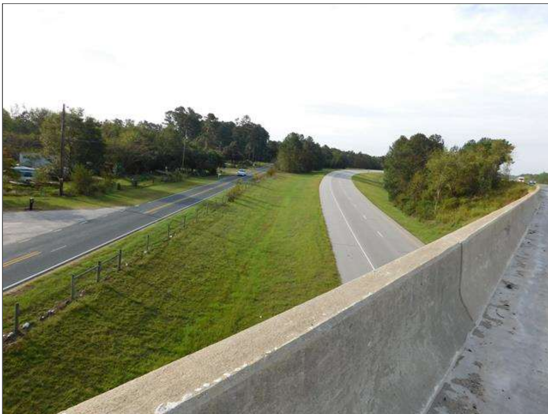
LOOKING EAST, ON RAMP 95 BUS.
