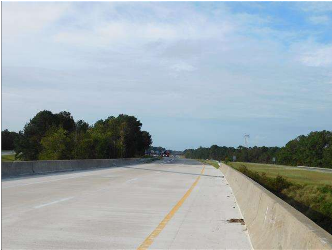
LOOKING SOUTH, OFF BRIDGE
