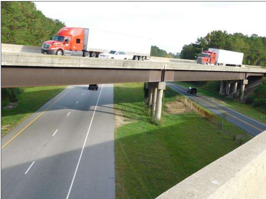
LOOKING WEST, NORTH 95 BUS.
