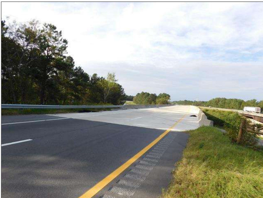
LOOKING SOUTH, NORTHBOUND LANE
