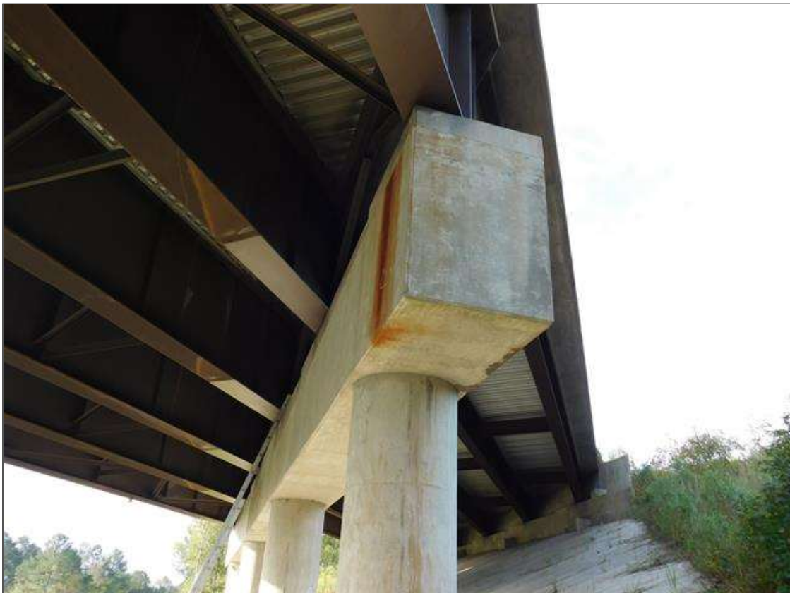
WEST END OF BENT 1 CAP, SIMPLE SPANS
