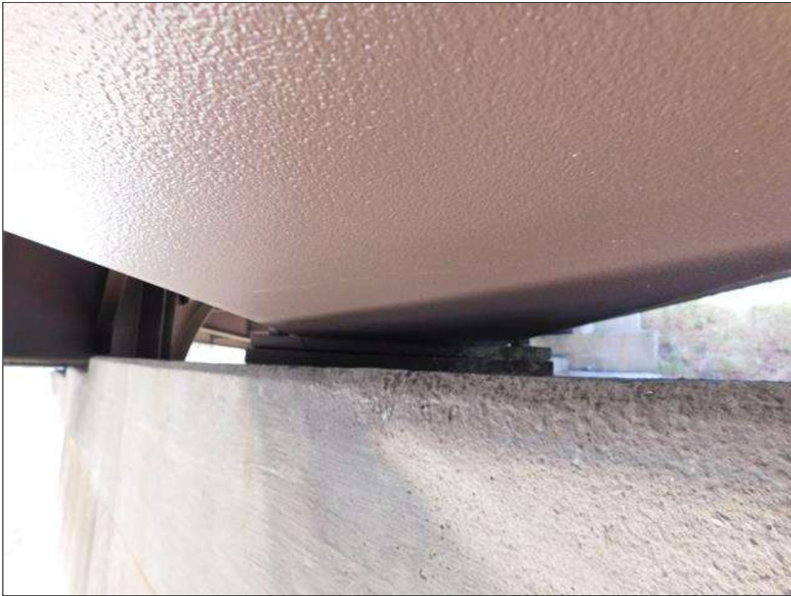
SPAN 2 BEAM 3 NEAR BEARING
