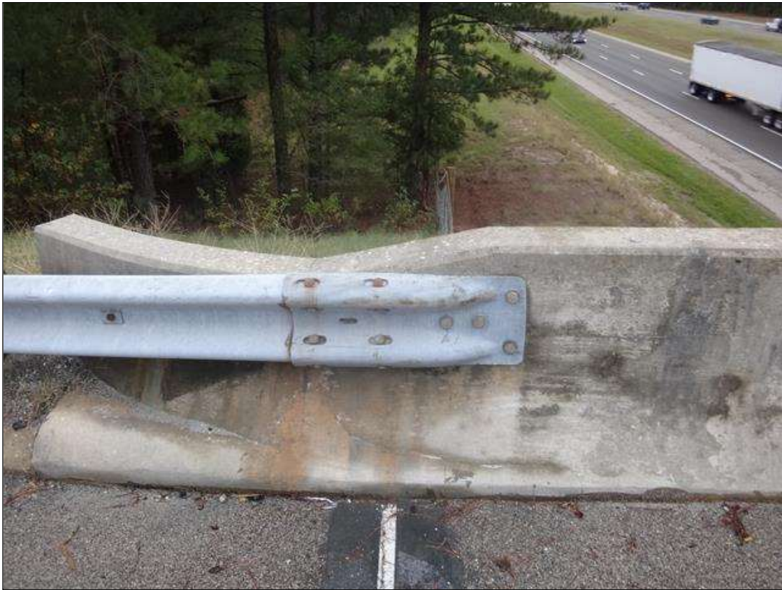
southeast guardrail attachment
