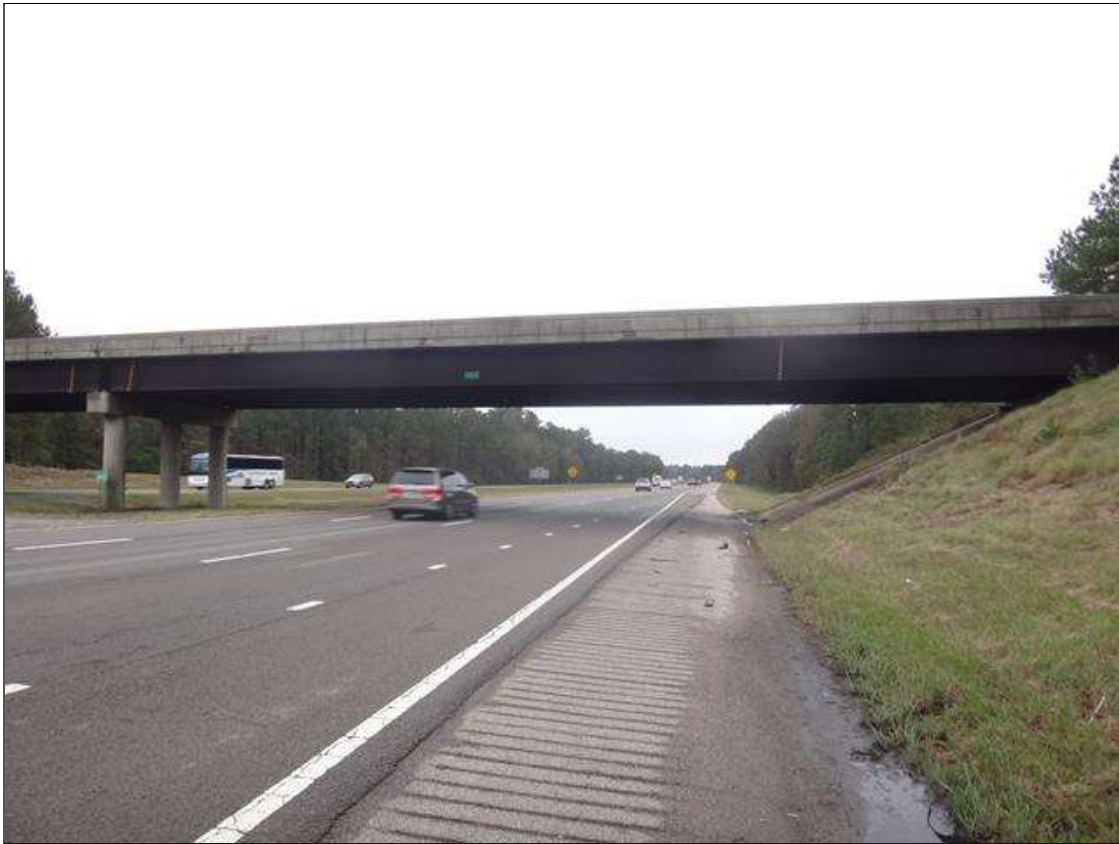
looking south through (span 1)
