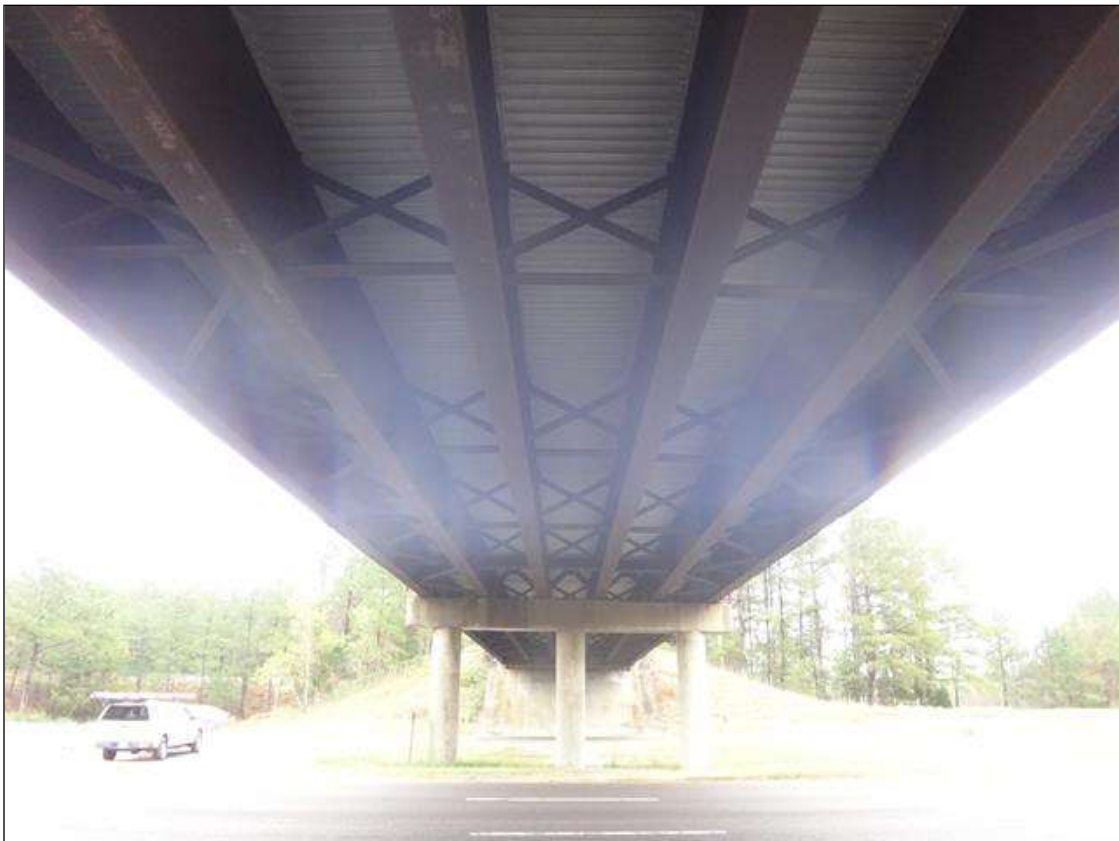
underside of deck
