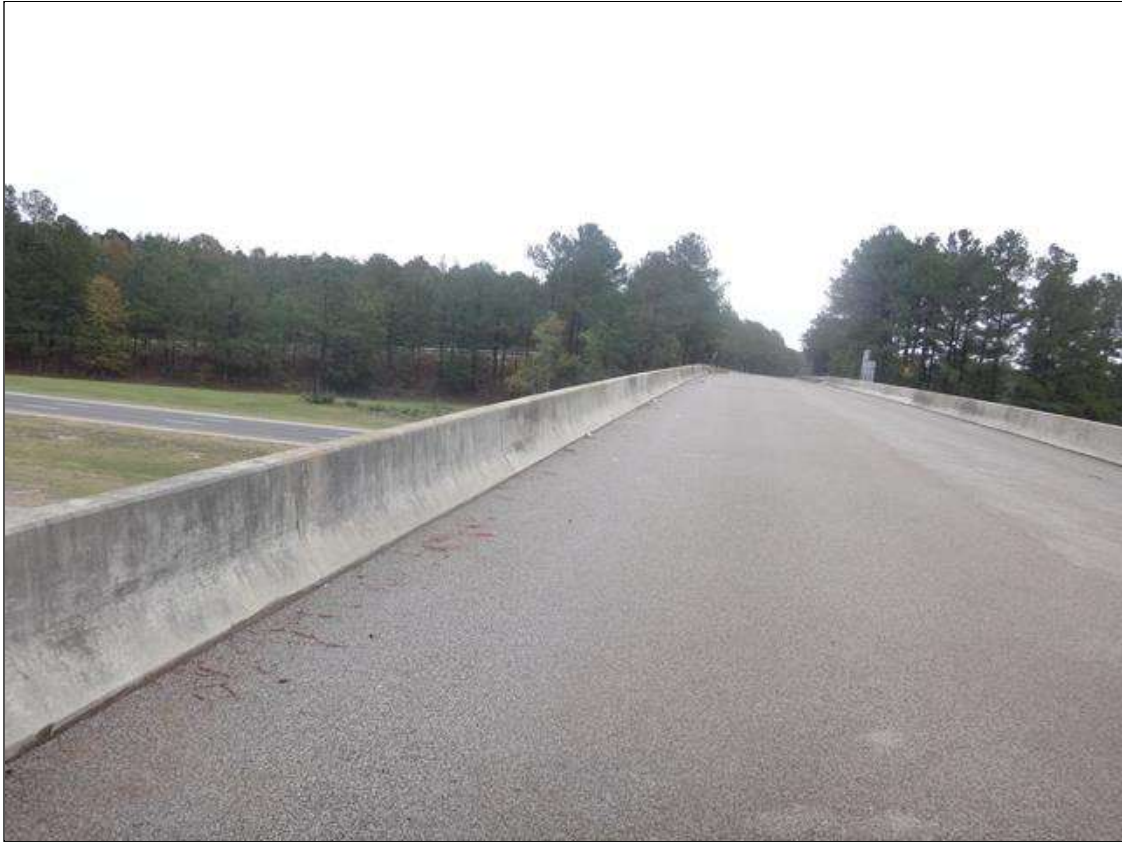
north bridge rail
