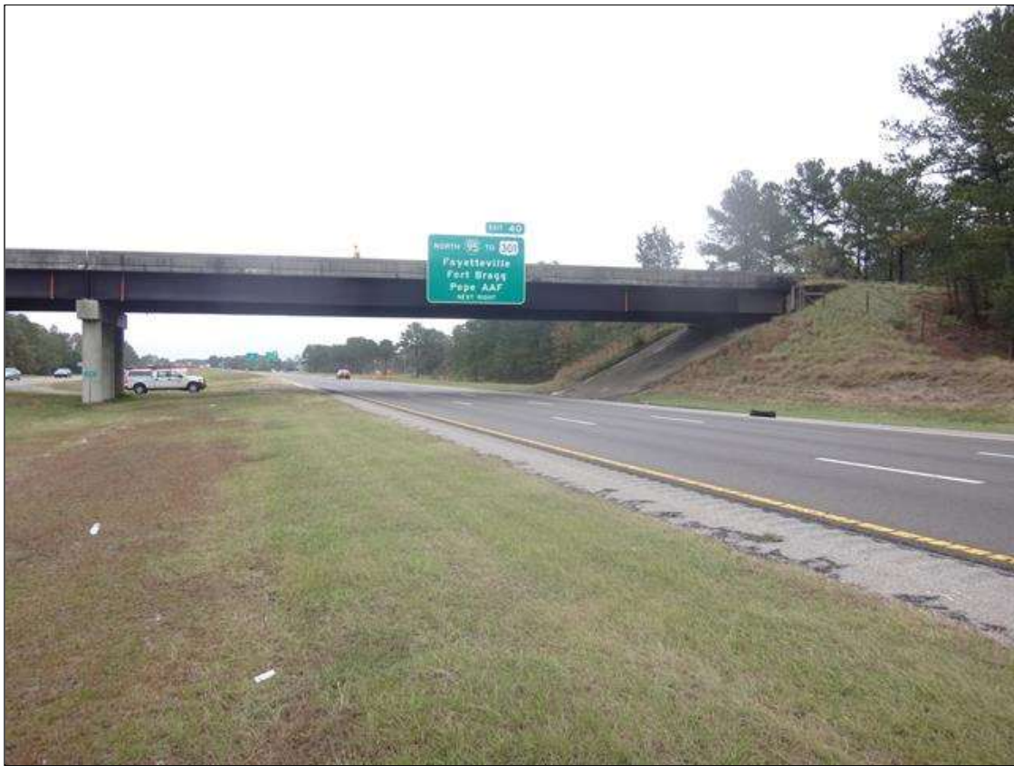
looking north through span 2
