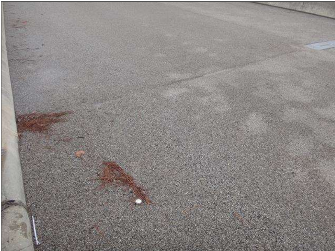
Expansion Joint 1: at north end, joint covered with epoxy overlay (17-1/2ft)
