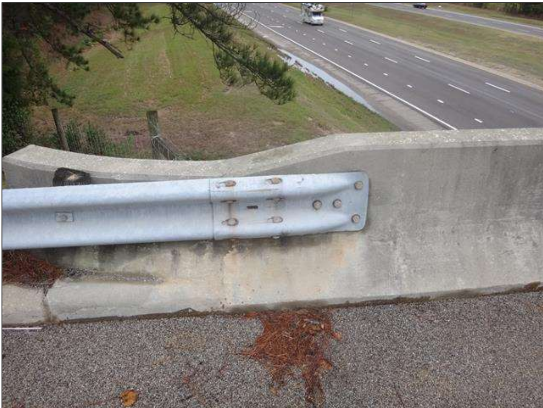
northwest guardrail attachment
