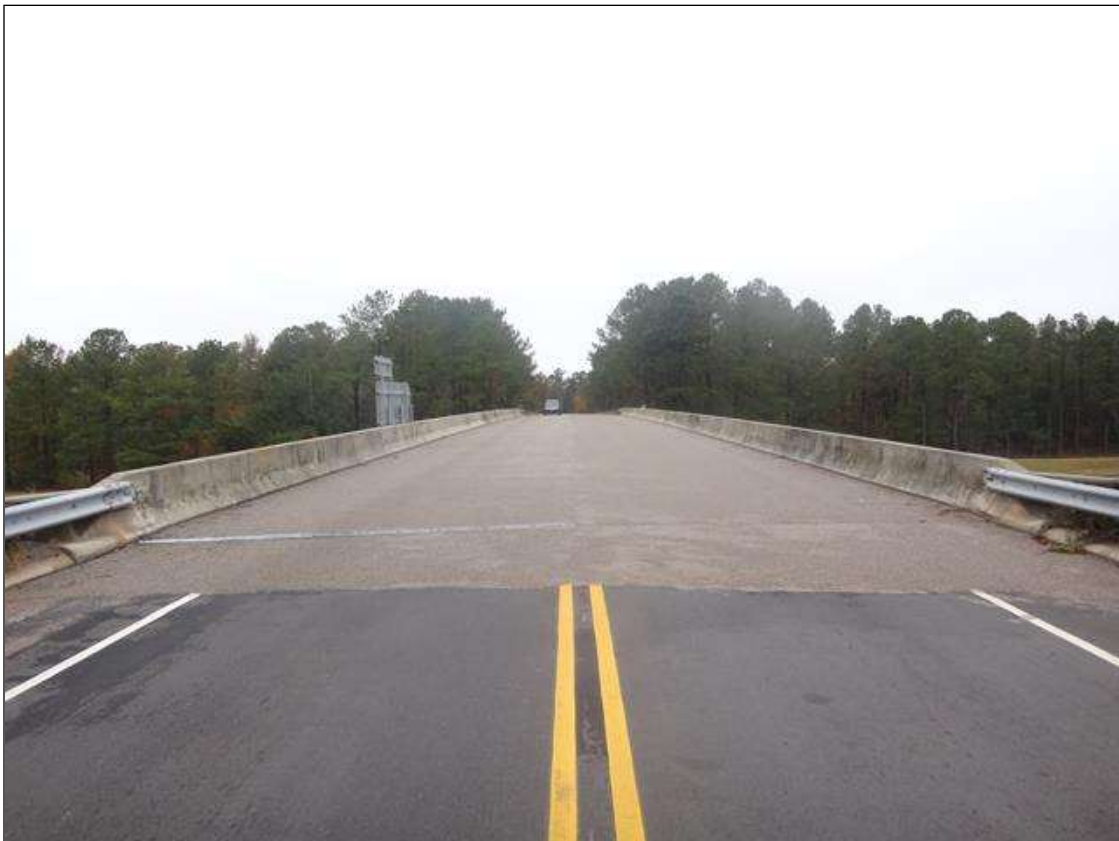
east approach looking west
