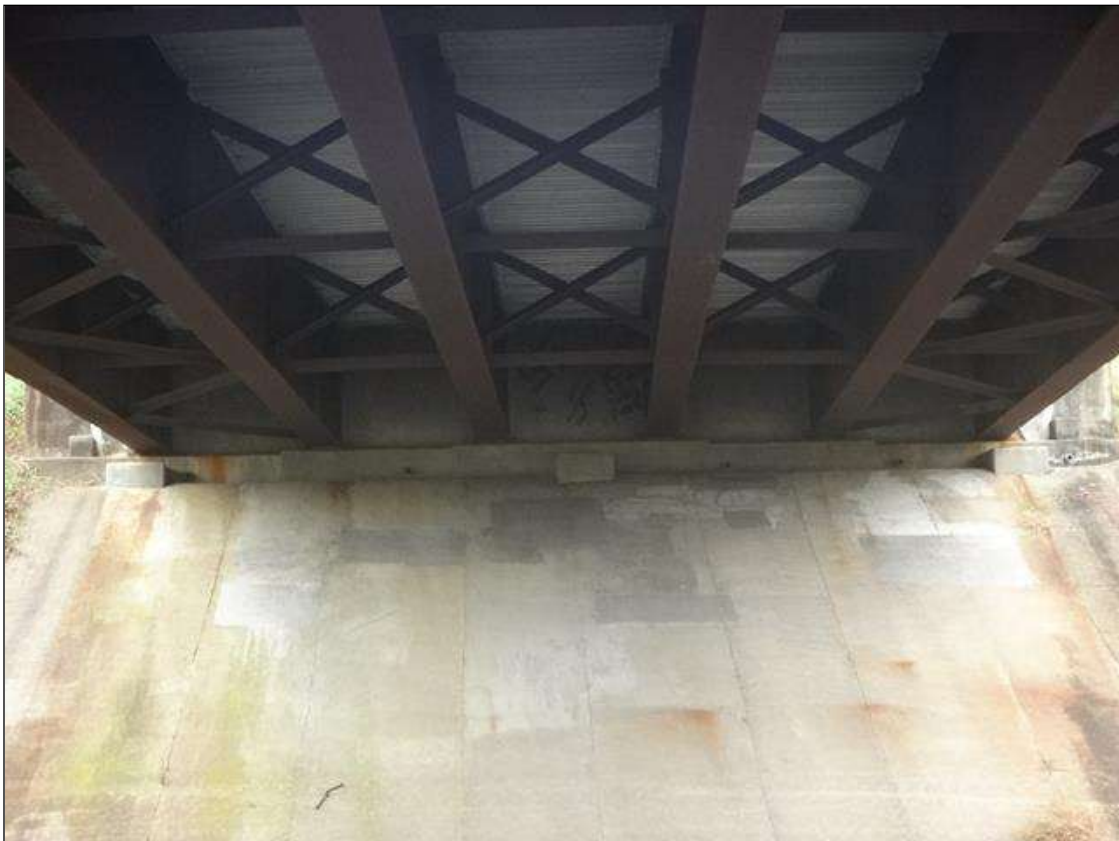
end bent 2 and slope protection
