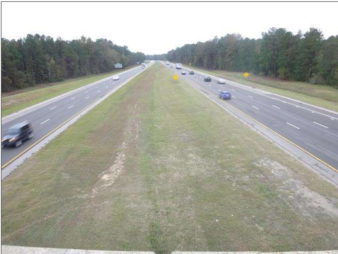
looking south from deck
