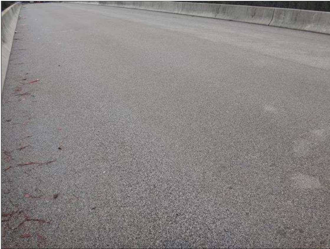
Span 1 Wearing Surface: new epoxy wearing surface installed since last inspection
