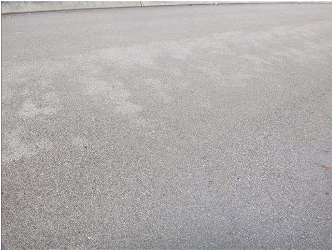
epoxy wearing surface
