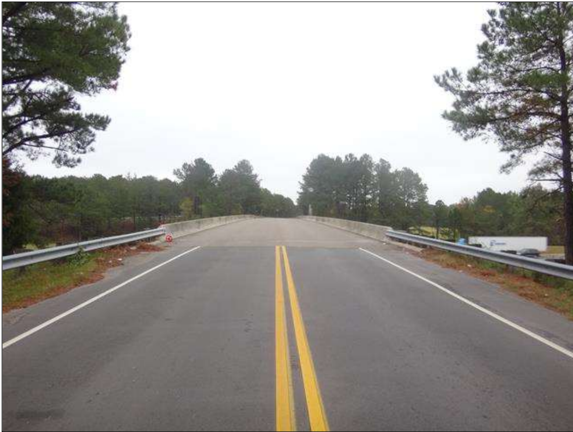
west approach looking east
