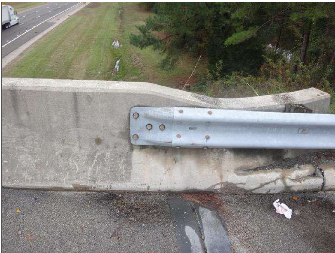
southwest guardrail attachment
