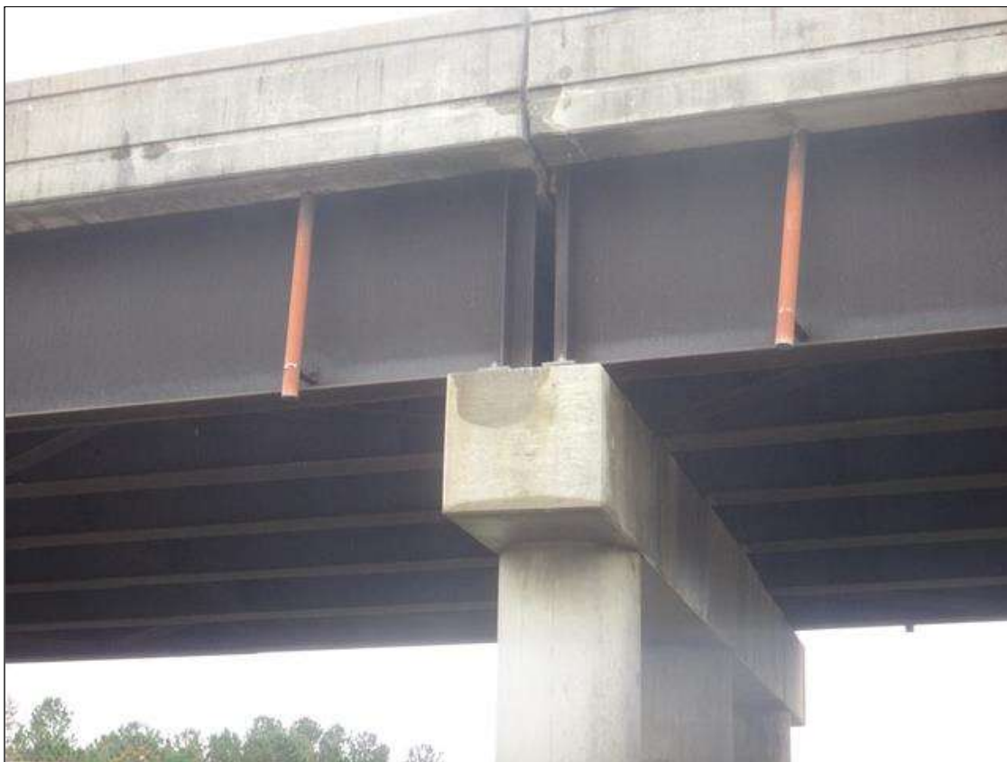
beams over bent 1
