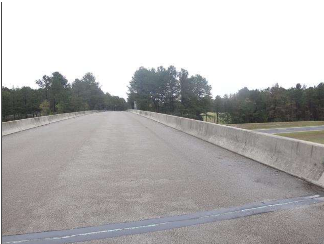
south bridge rail
