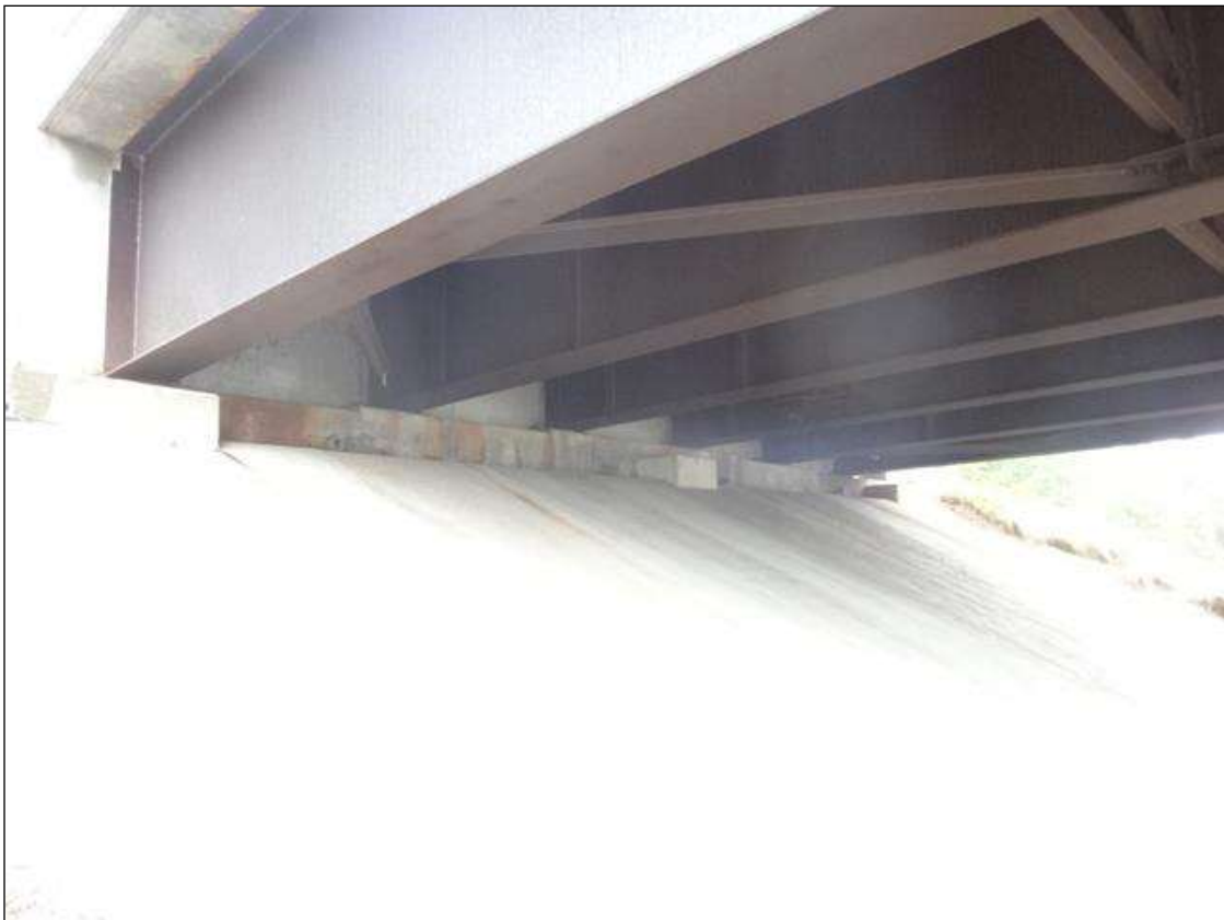
end bent 1 and slope protection
