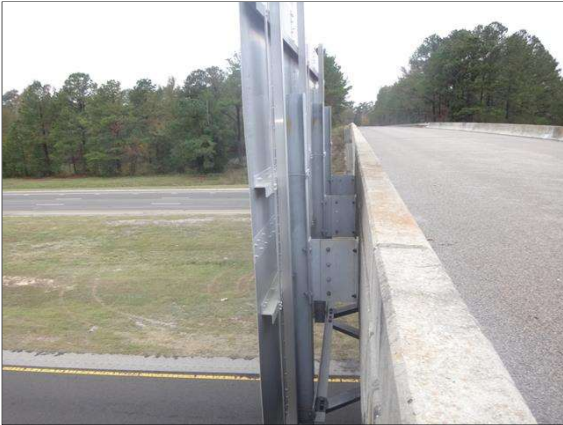
span 2 overhead sign attachment to rail
