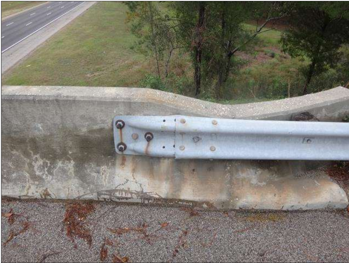
northeast guardrail attachment
