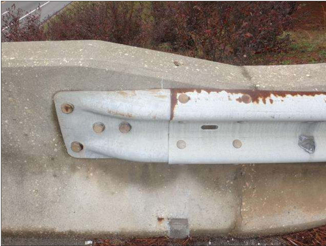
southeast guardrail attachment
