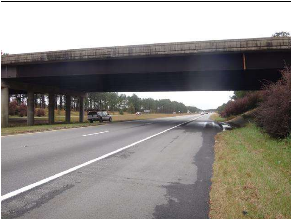
looking west through span 2
