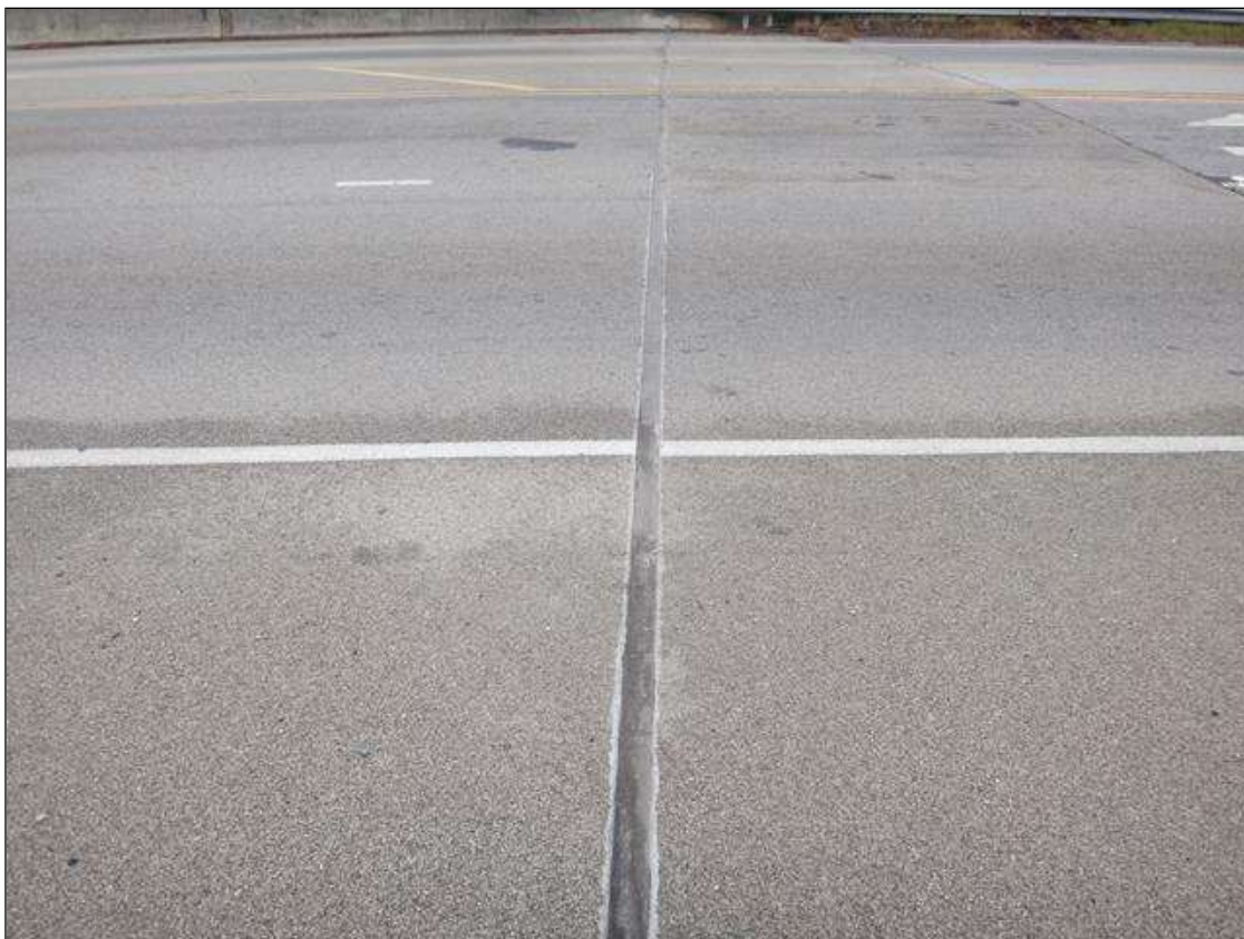
end bent 1 joint
