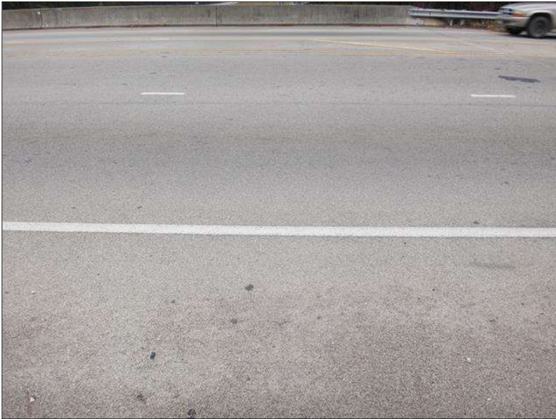
epoxy wearing surface
