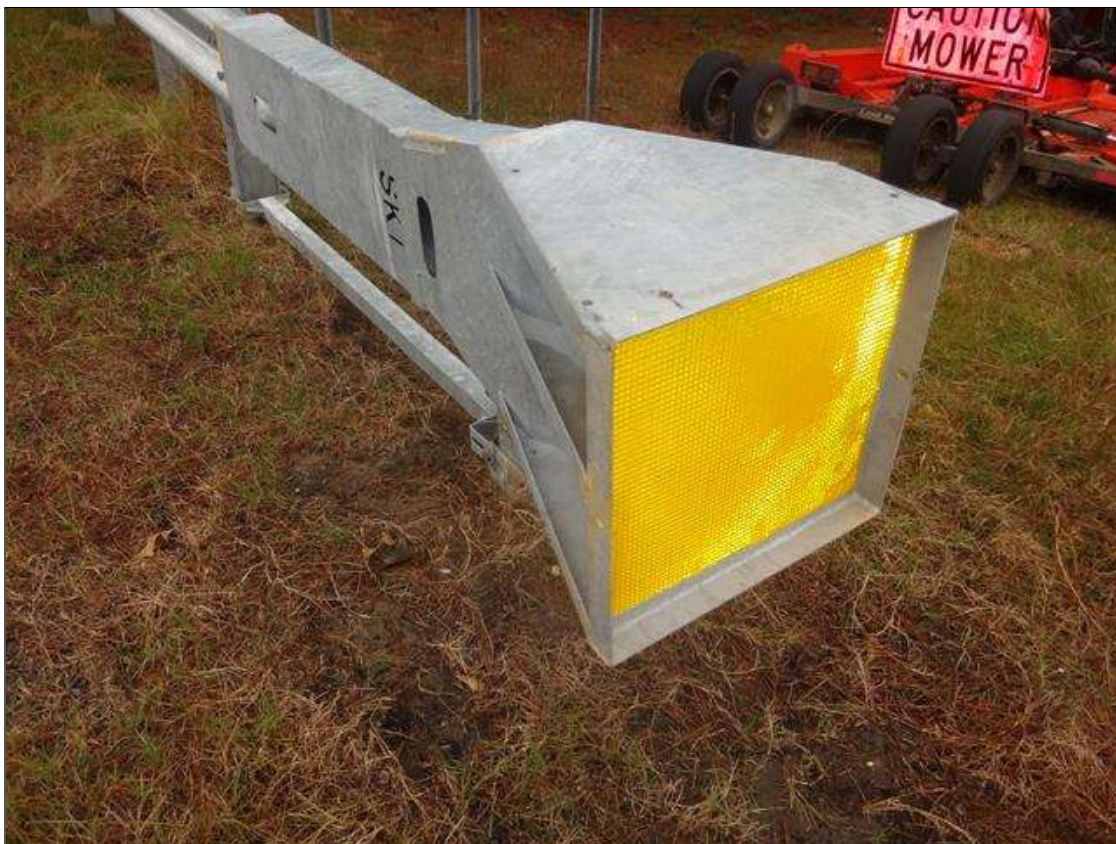
southeast guardrail termination
