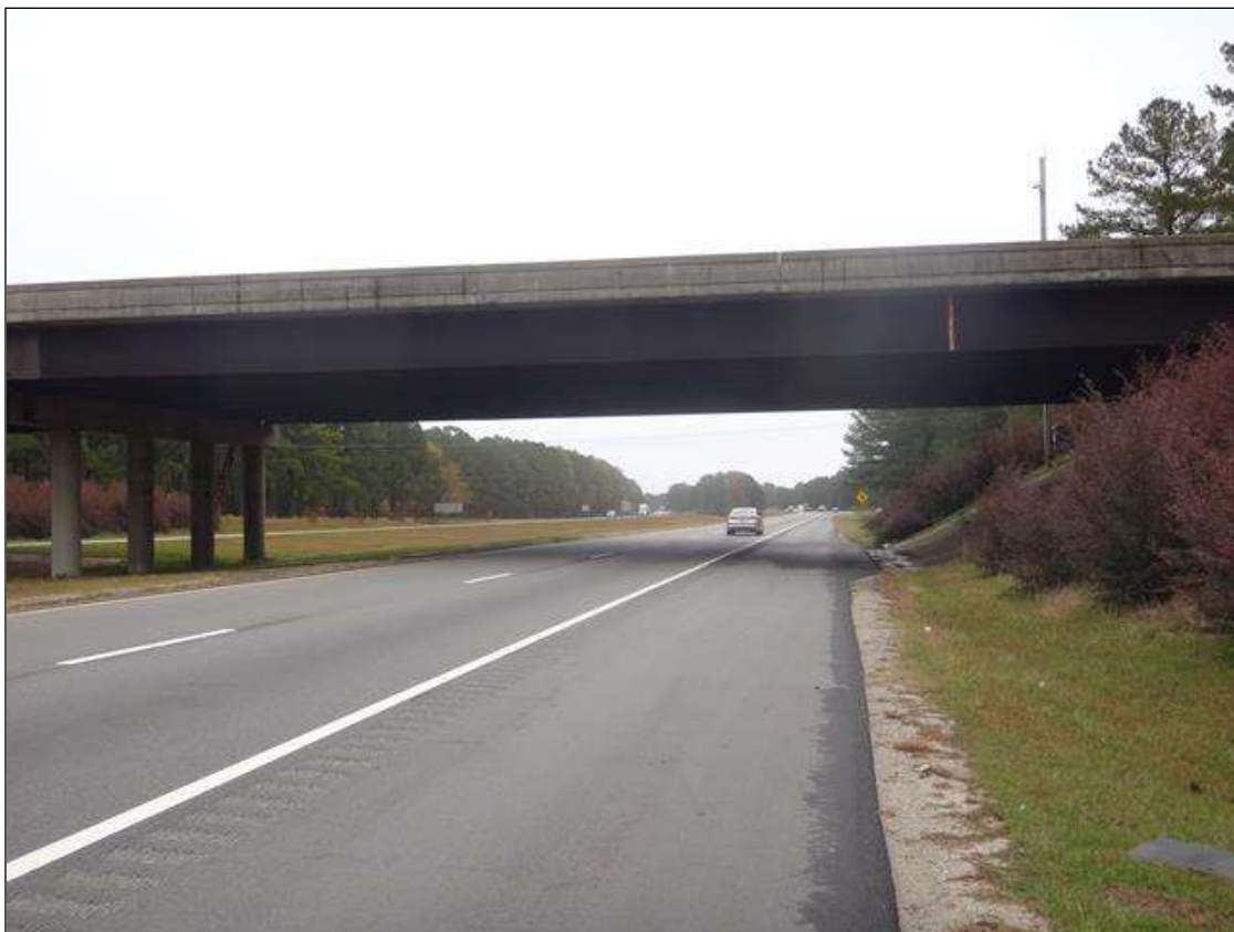
looking east through span 1
