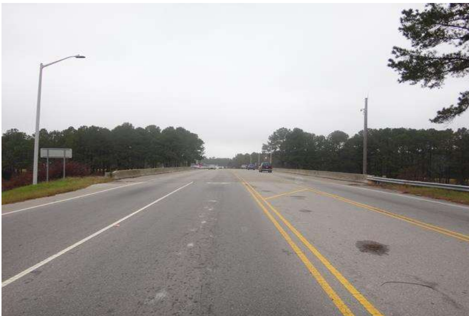
south approach looking north
