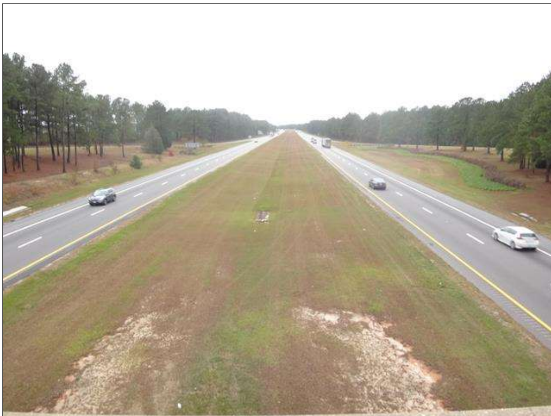
looking west from deck
