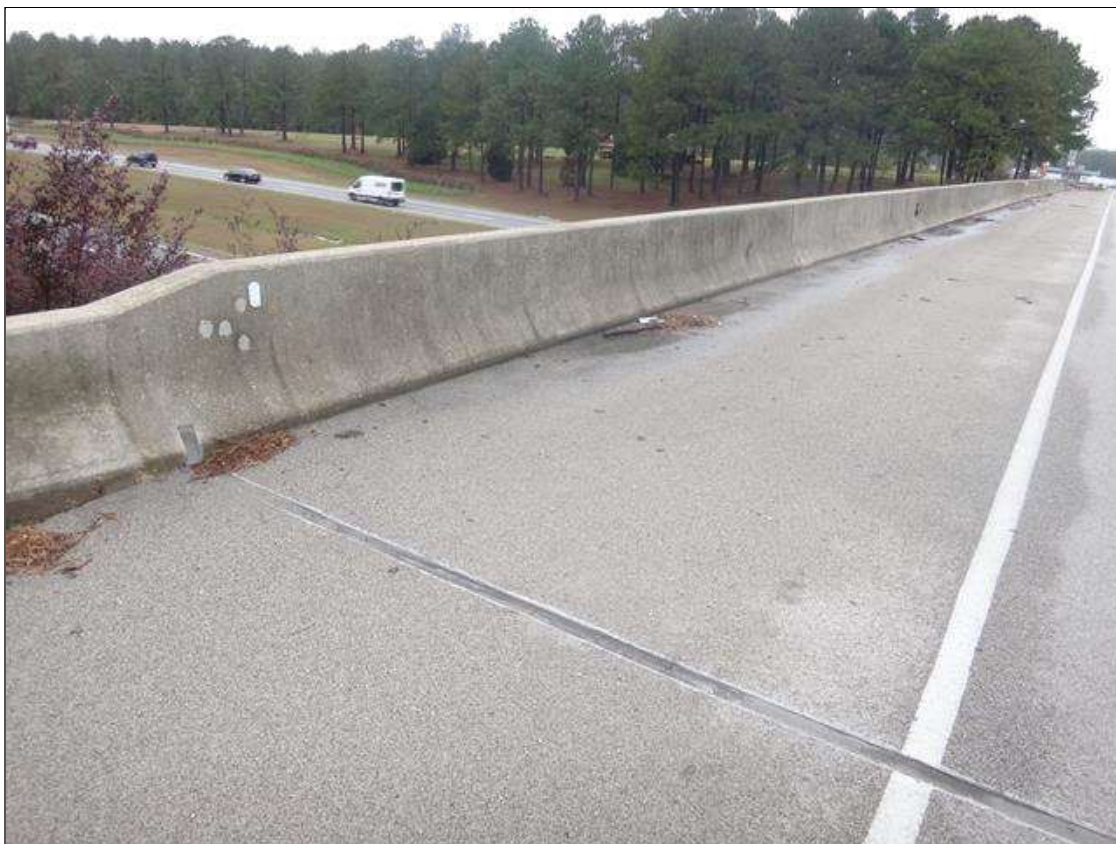
west bridge rail
