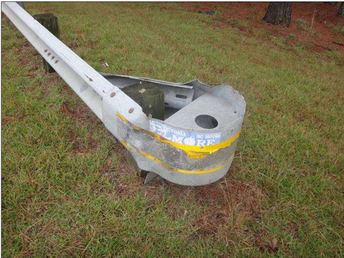
northwest guardrail termination
