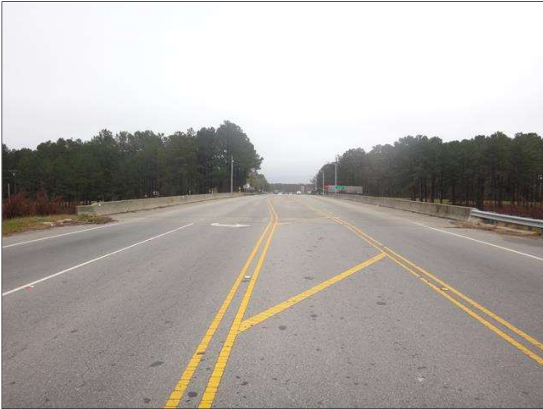
north approach looking south
