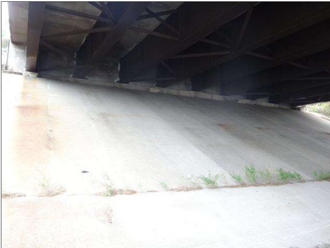
end bent 2 and slope protection
