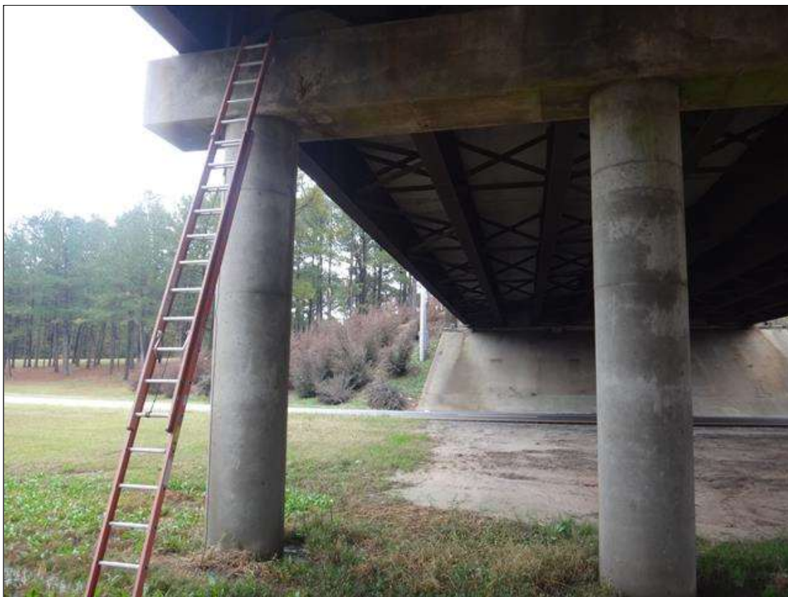
ladder on bent
