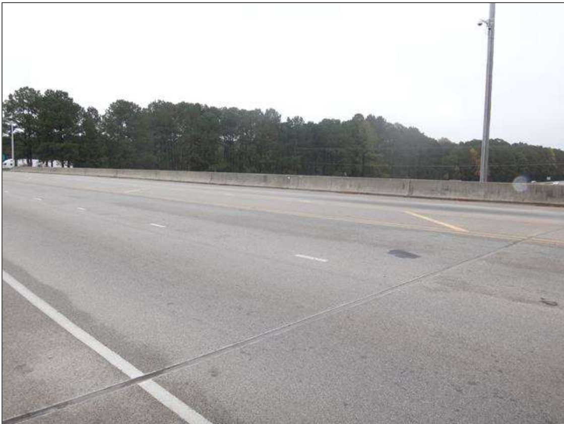
east bridge rail
