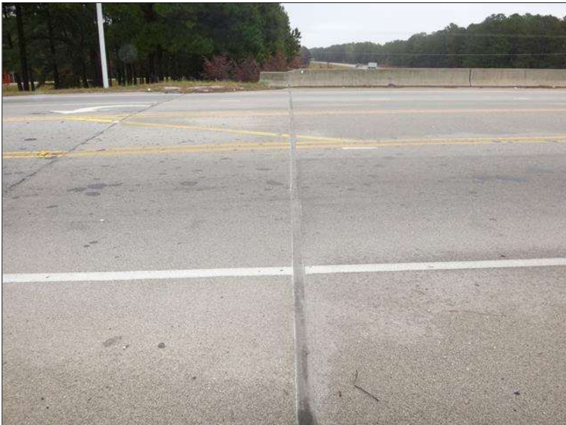
end bent 2 joint
