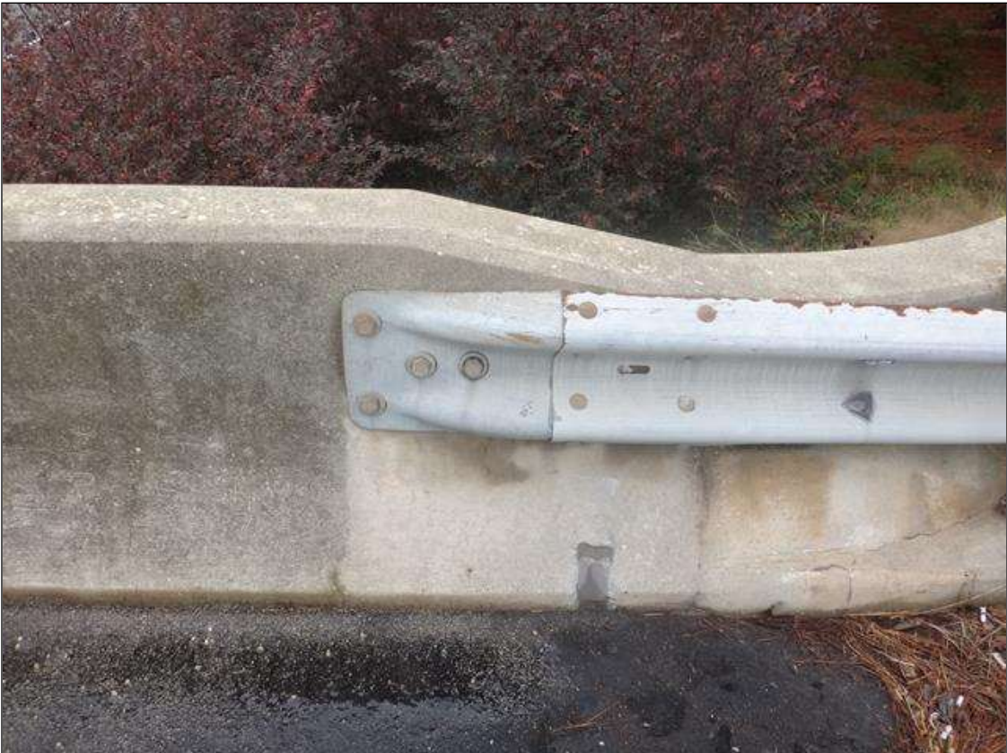
northwest guardrail attachment
