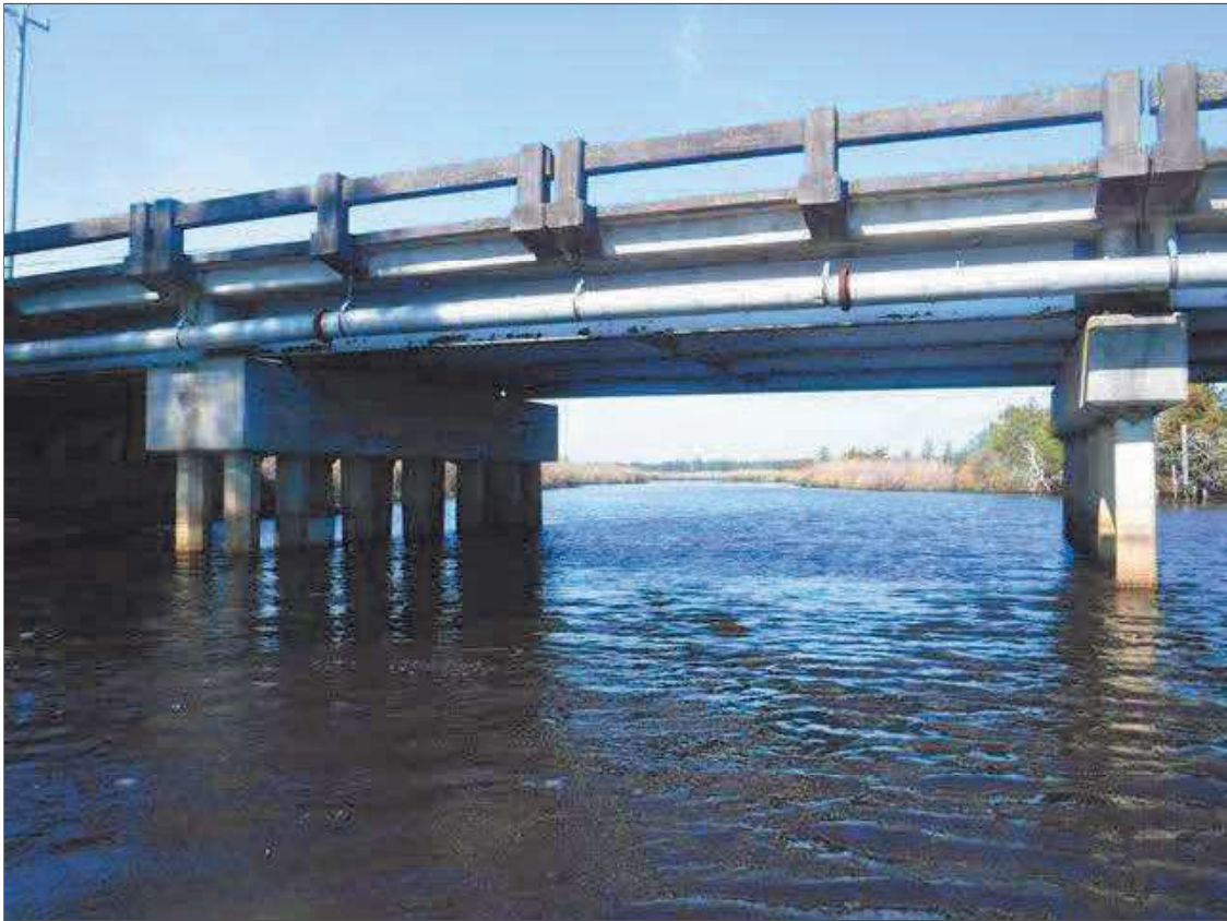
SPAN 2 UPSTREAM PROFILE, LOOKING NORTH
