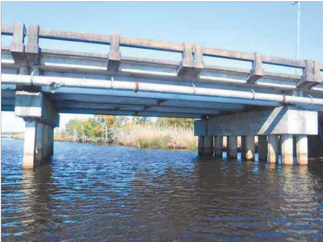
SPAN 3 UPSTREAM PROFILE, LOOKING NORTH
