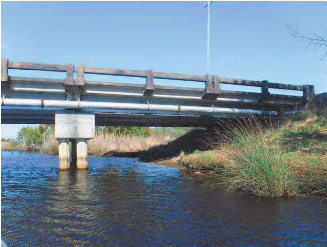
SPAN 4 UPSTREAM PROFILE, LOOKING NORTH
