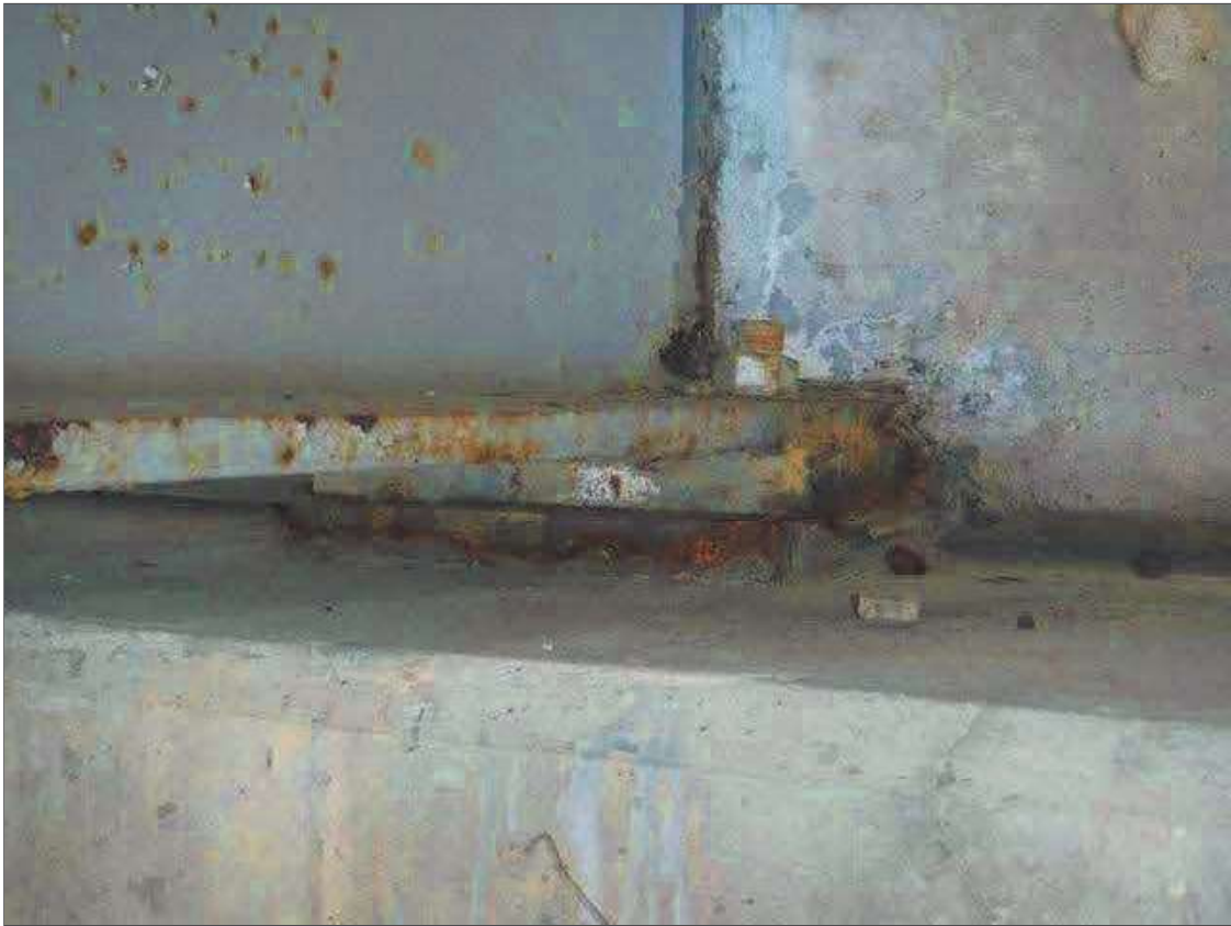
BEAM 3 BEARING AT END BENT 2, OTHERS SIMILAR AT END BENTS
