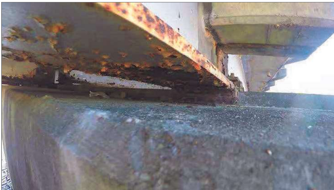
BEAM 1 BEARING AT BENT 3 IN SPAN 4, OTHERS SIMILAR AT BENTS
