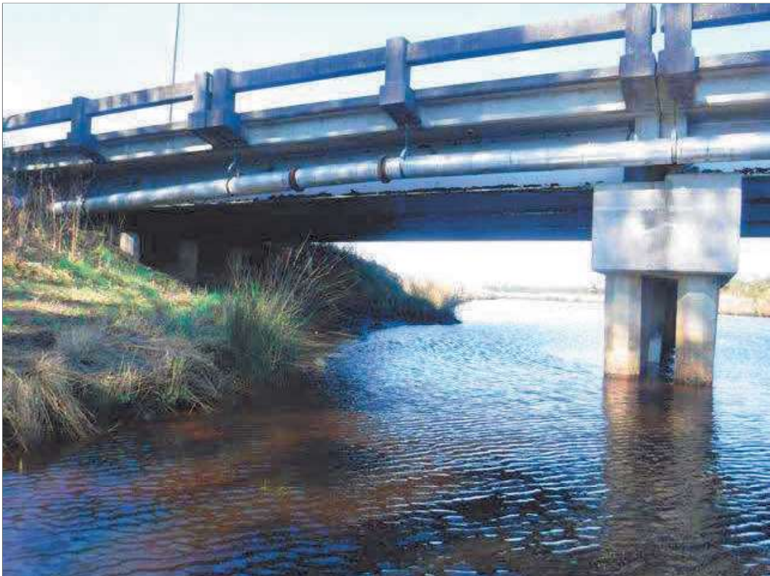
SPAN 1 UPSTREAM PROFILE, LOOKING NORTH
