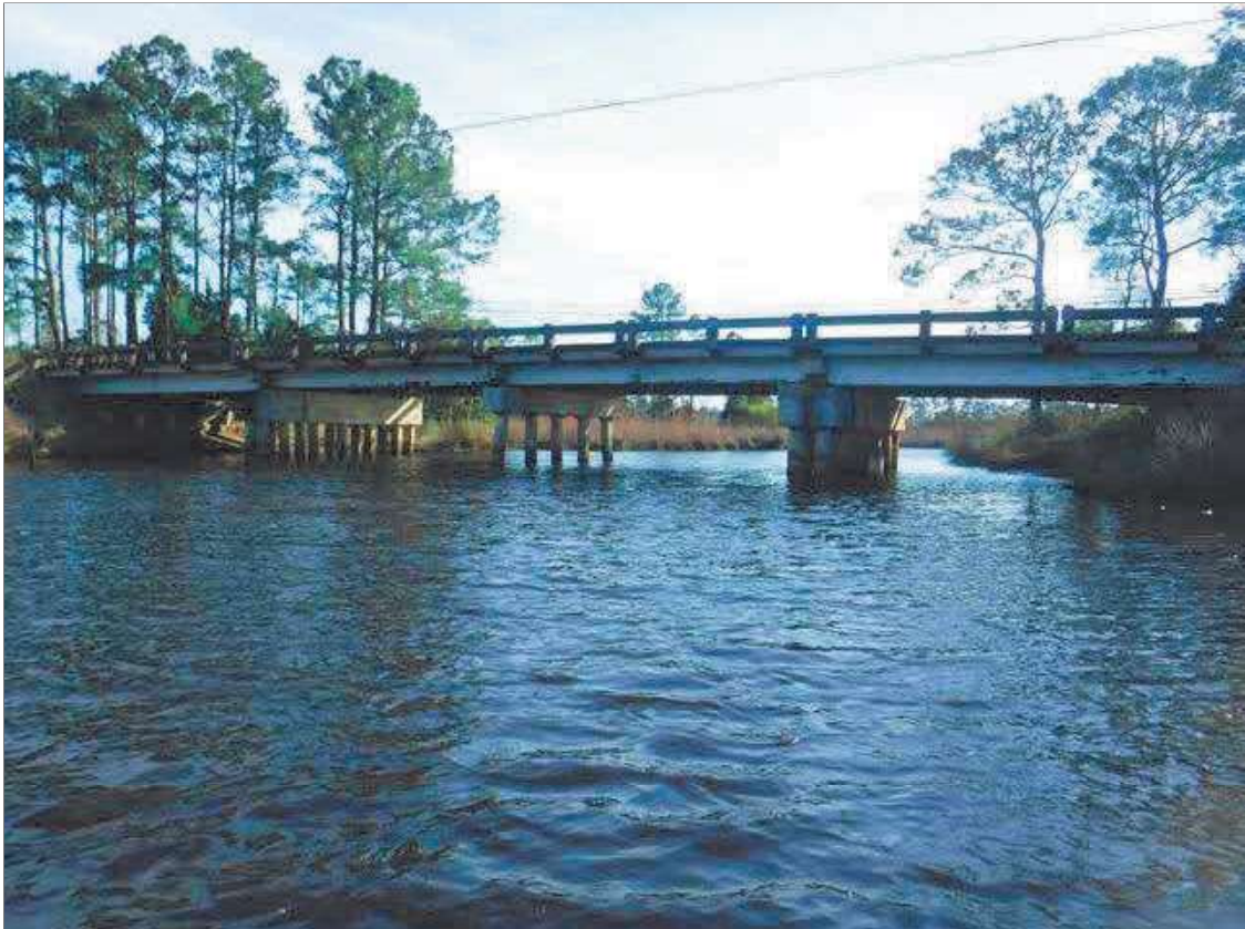
DOWNSTREAM PROFILE, LOOKING SOUTH
