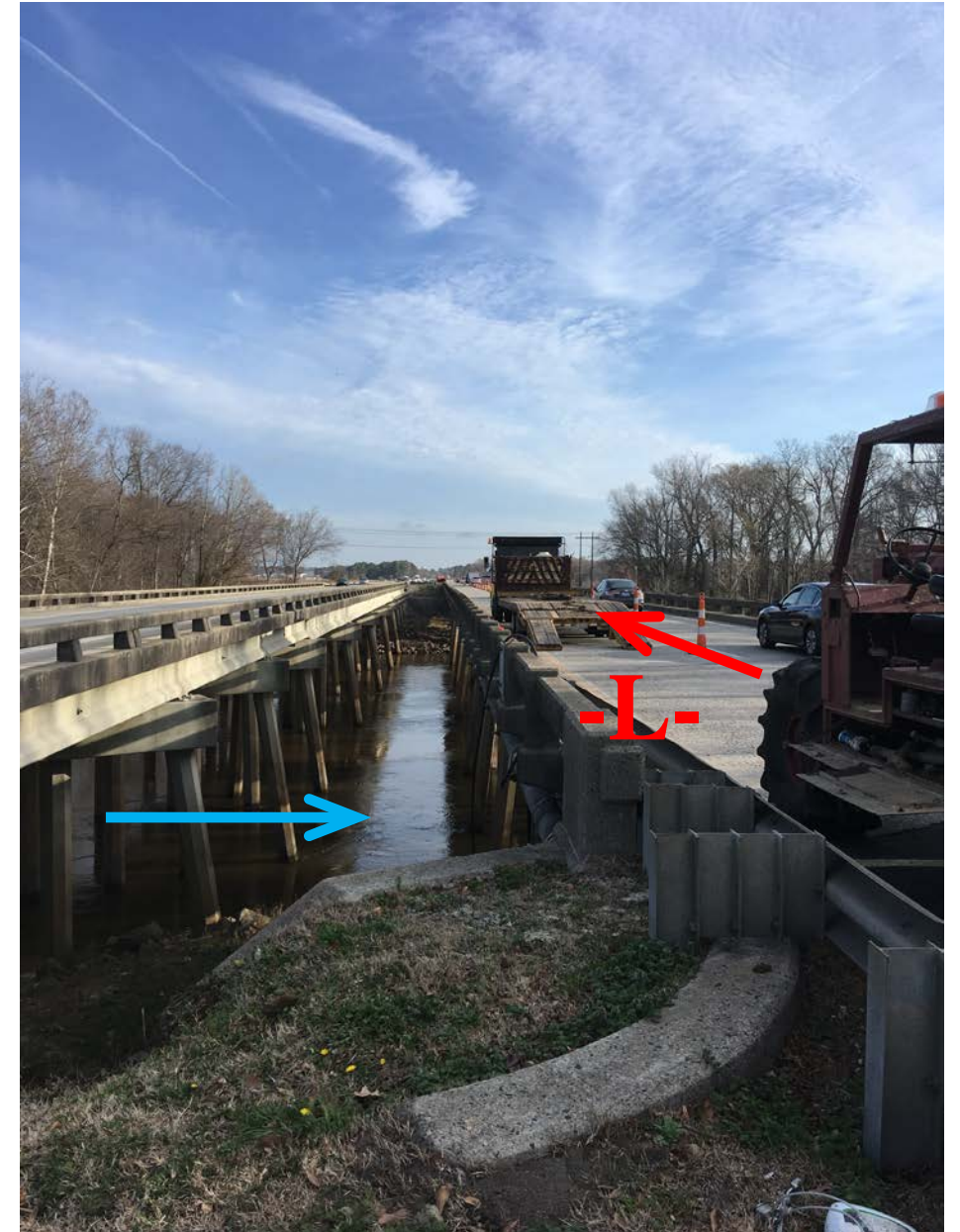
Looking Northeast towards End Bent 2
