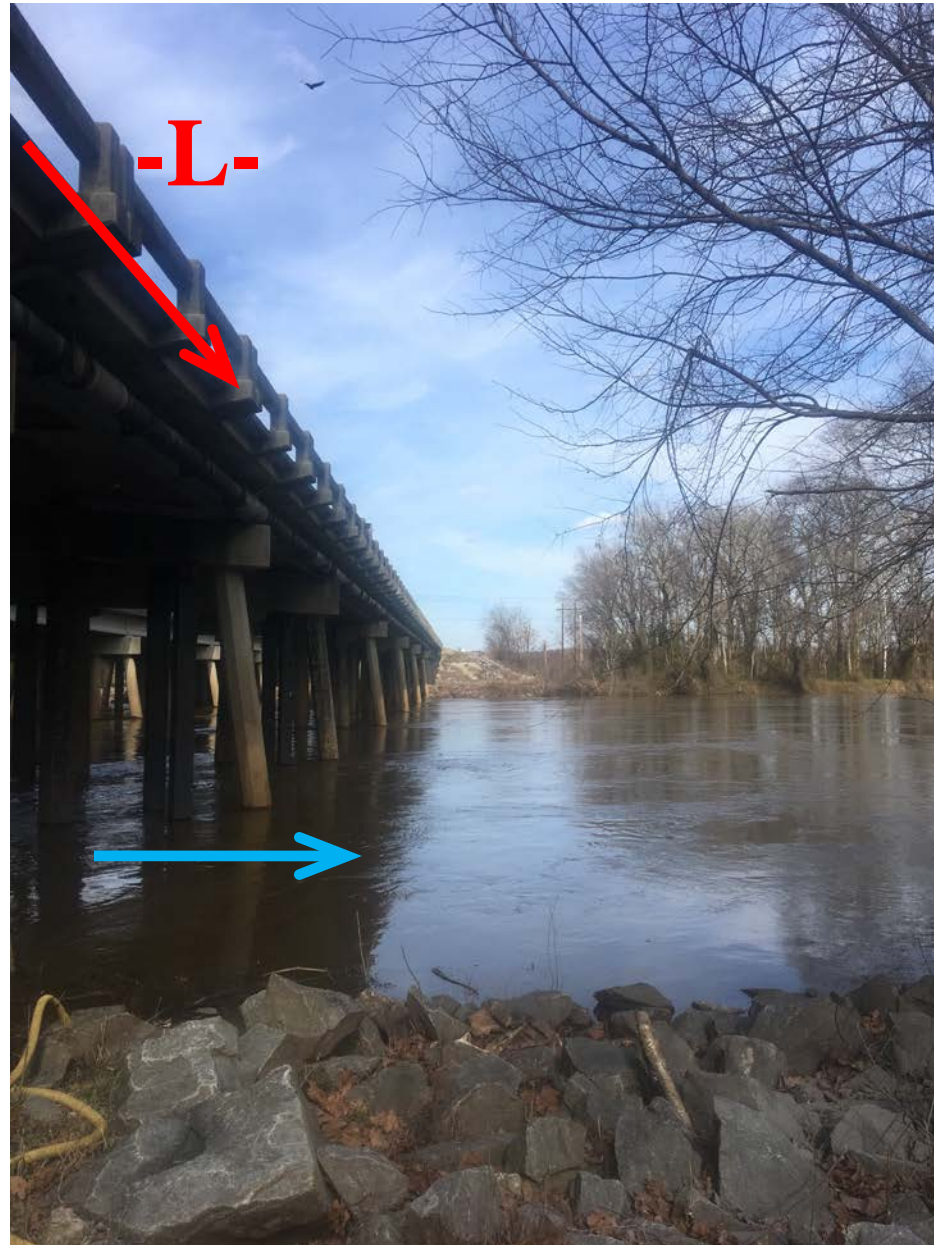
Looking Northeast towards End Bent 2
