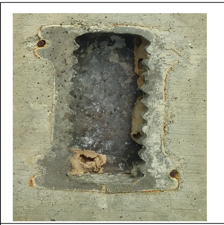
EXIST. CONCRETE INSERTS IN THE BRIDGE OVERHANG
