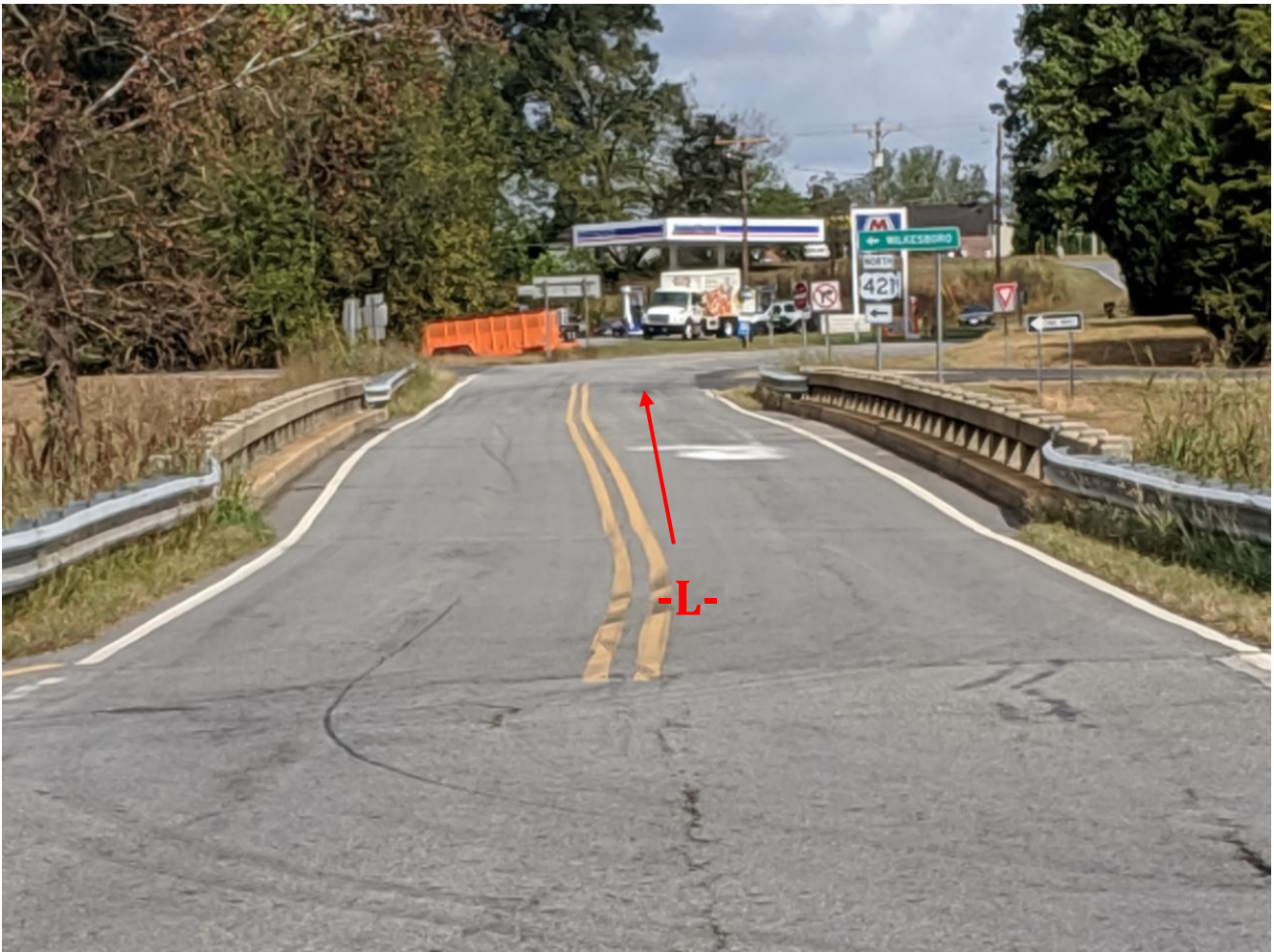
Photograph No. 1: At End Bent 1 looking towards End Bent 2
