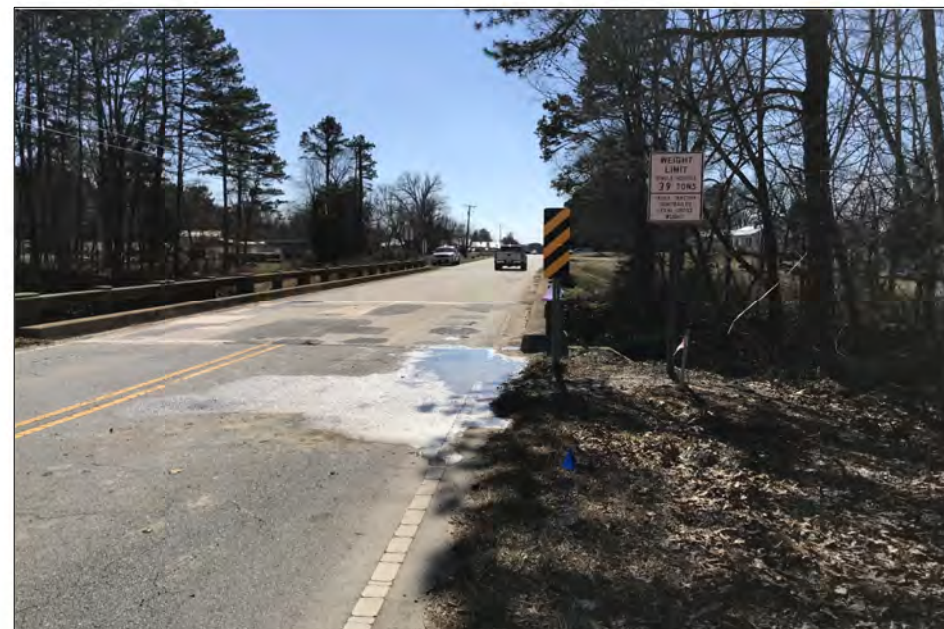
VIEW DOWNSTATION FROM END BENT 2 TOWARD END BENT 1
