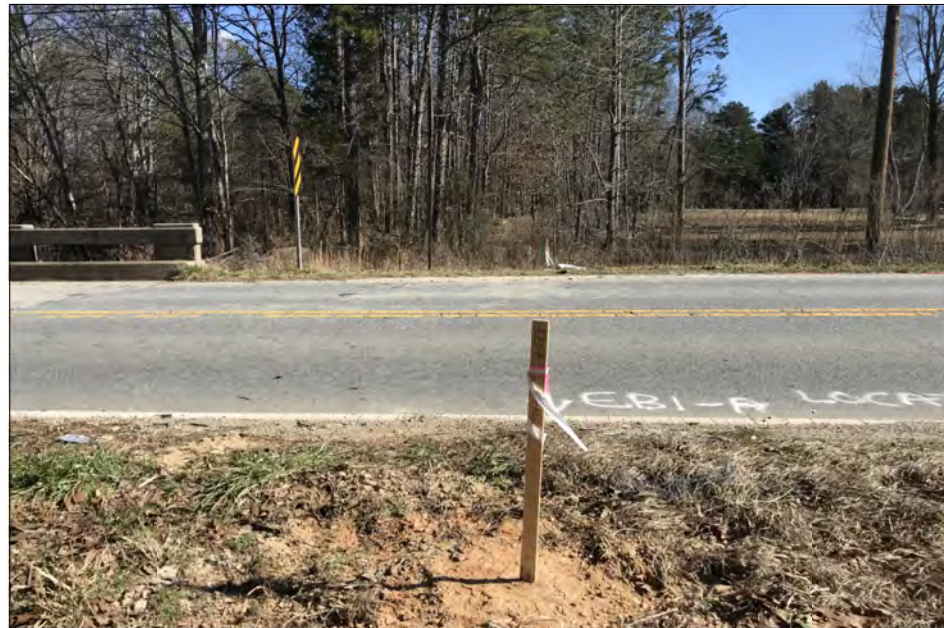
VIEW ALONG END BENT 1 FROM EB1-A TOWARD EB1-B
