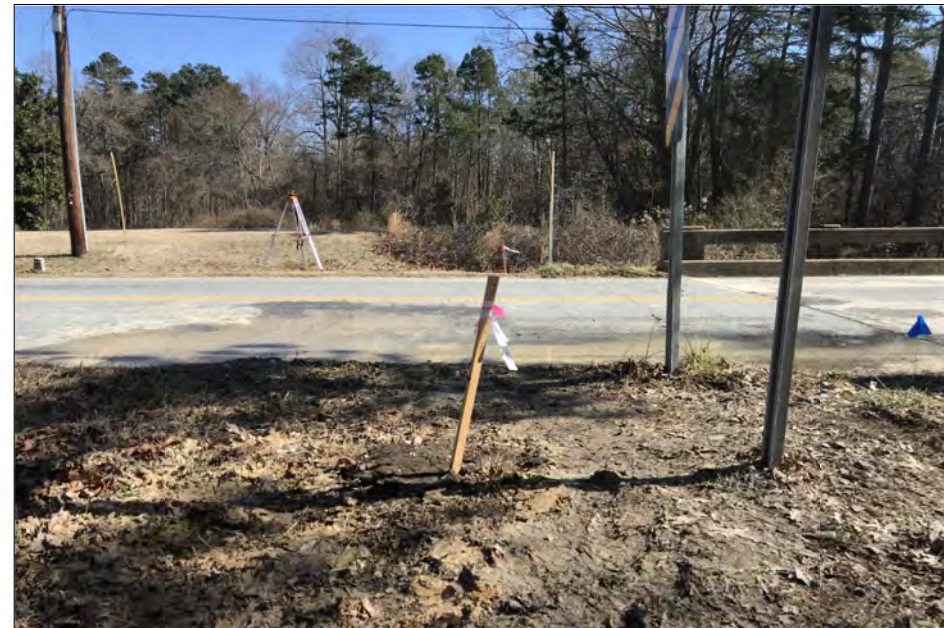
VIEW ALONG END BENT 2 FROM EB2-A TOWARD EB2-B
