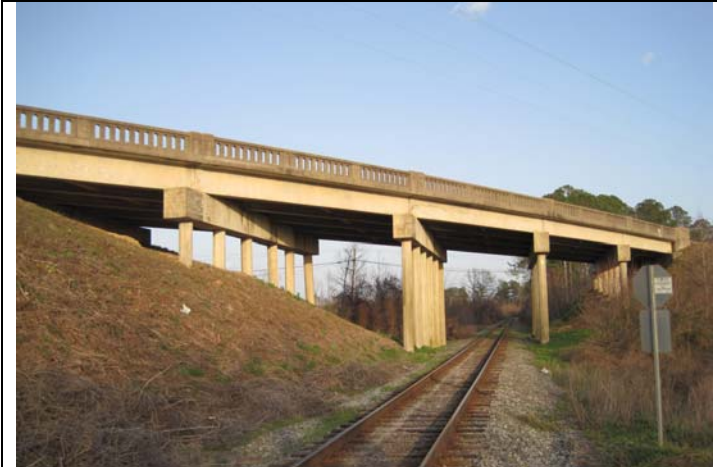
Bridge 87: Looking southward toward Bridge 87.
