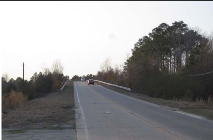
Bridge 87: Looking westward toward Bridge 87.
