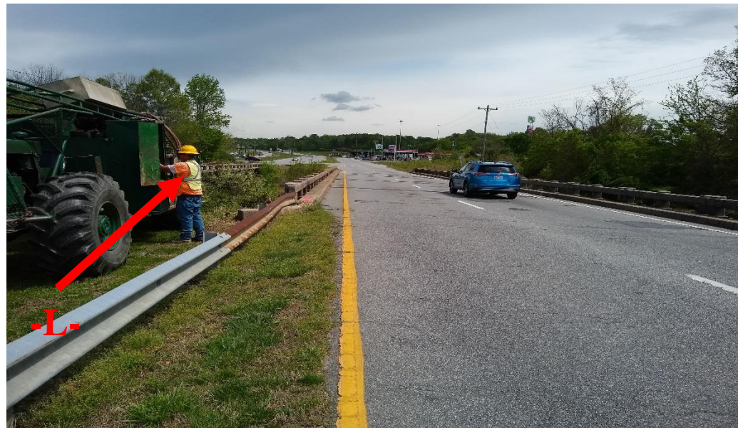
View Along Bridge 109 Looking Upstation from End Bent 1
