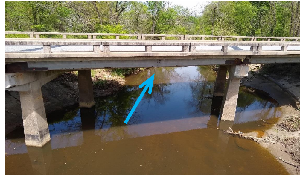
View Looking Downstream from Bridge 109
