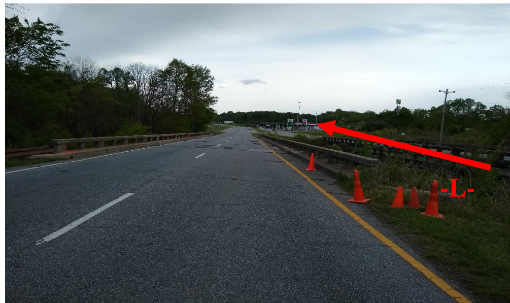
View of Along Bridge 121 Looking Upstation from End Bent 1
