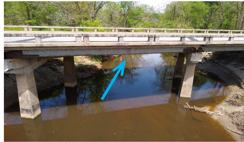
View Looking Downstream from Bridge 109
