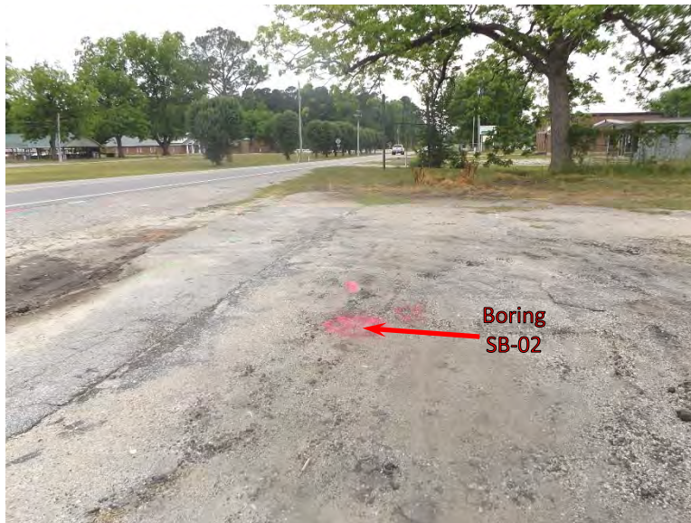
Photograph 7. GeoEnvironmental soil boring location SB-R5819-02.
