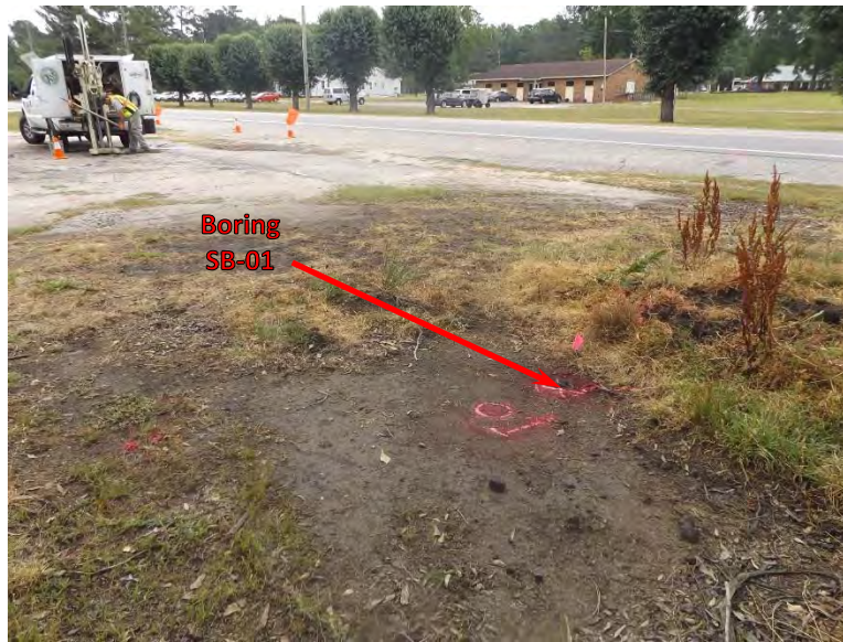
Photograph 6. GeoEnvironmental soil boring location SB-R5819-01.
